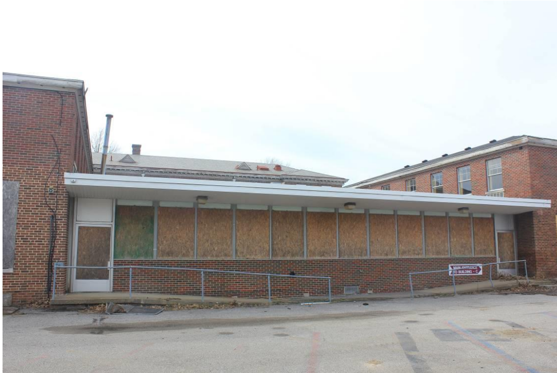
Photo #7: View of rear courtyard infill addition (ca. 1960), camera facing south
