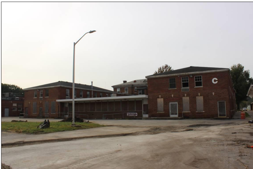
Photo 7: Rear (north) facade, camera facing south
