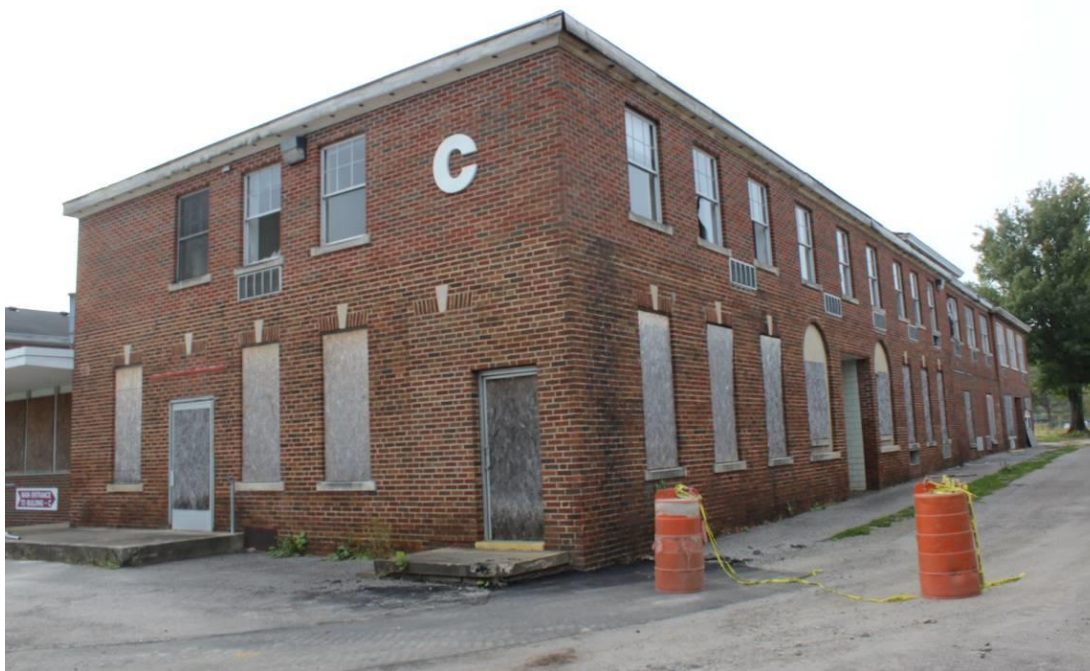
Photo #8: Oblique view of west wing, camera facing south
