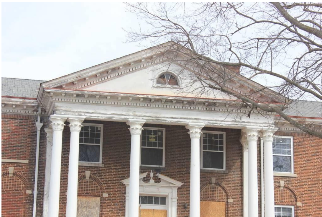
Photo #2: South Façade, portico, camera facing north
