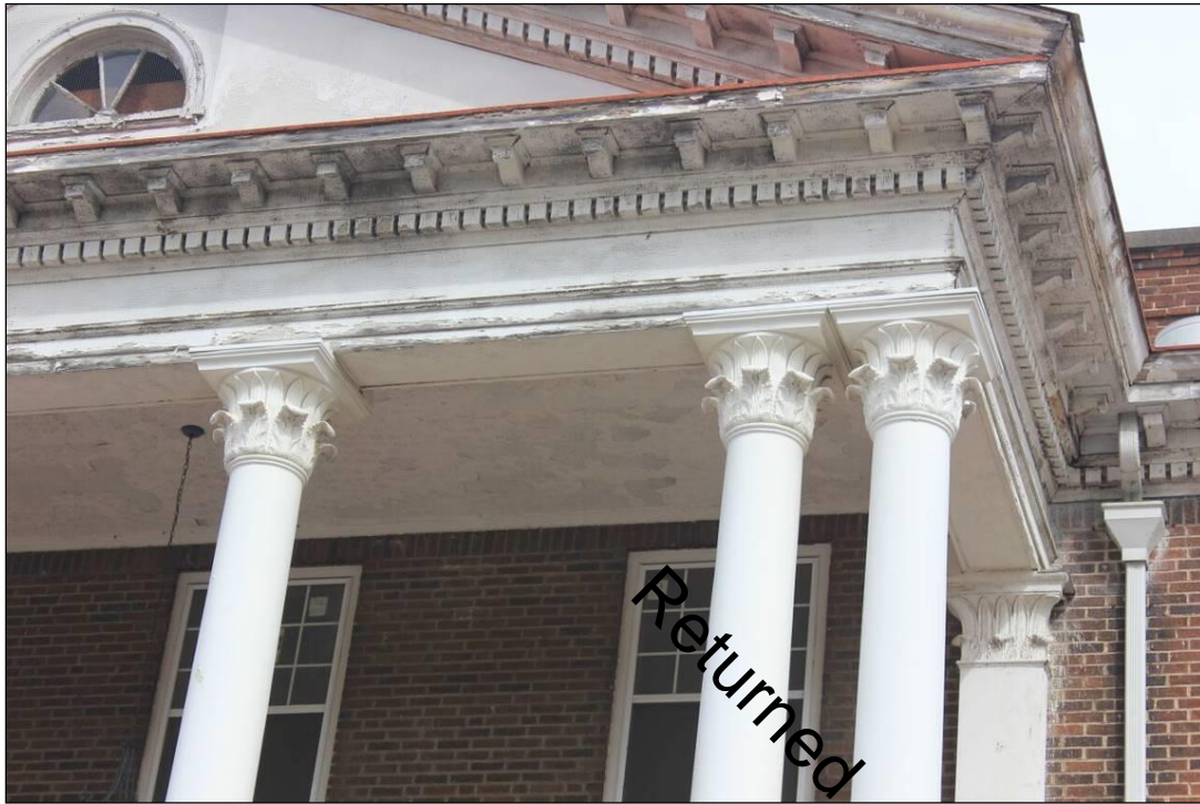
Photo 10: View of the portico architectural details, camera facing north
