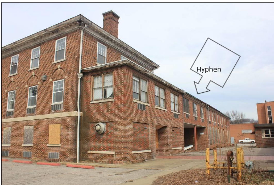
Photo 5: Side view of the east façade and wing, camera pointing northwest
