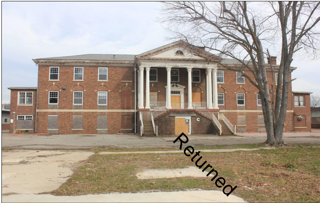
Photo 2: South façade, camera facing north
