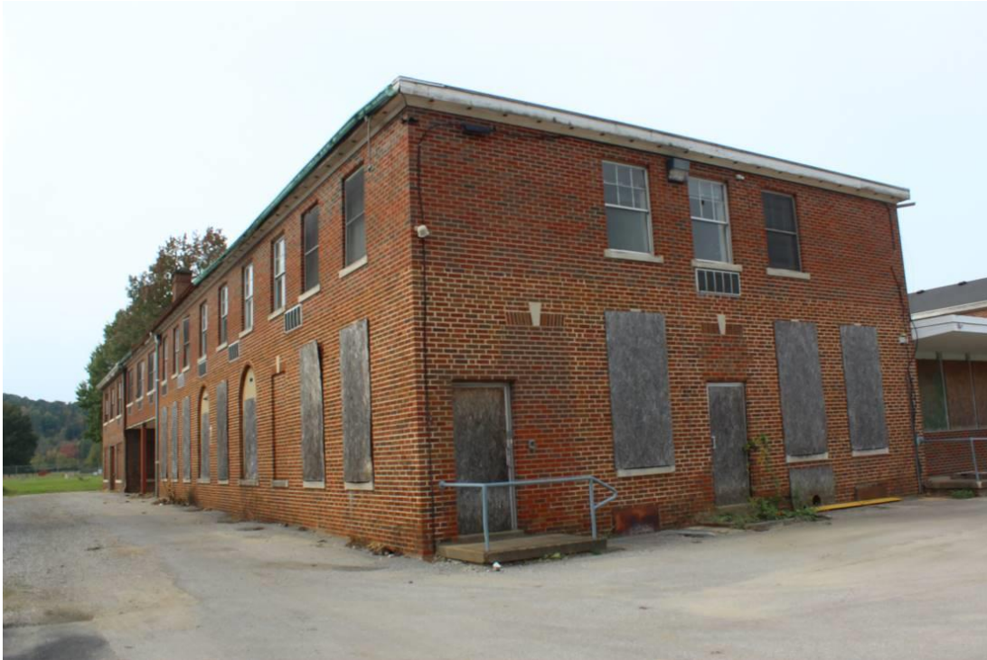
Photo #5: Oblique view of east wing, camera facing southwest
