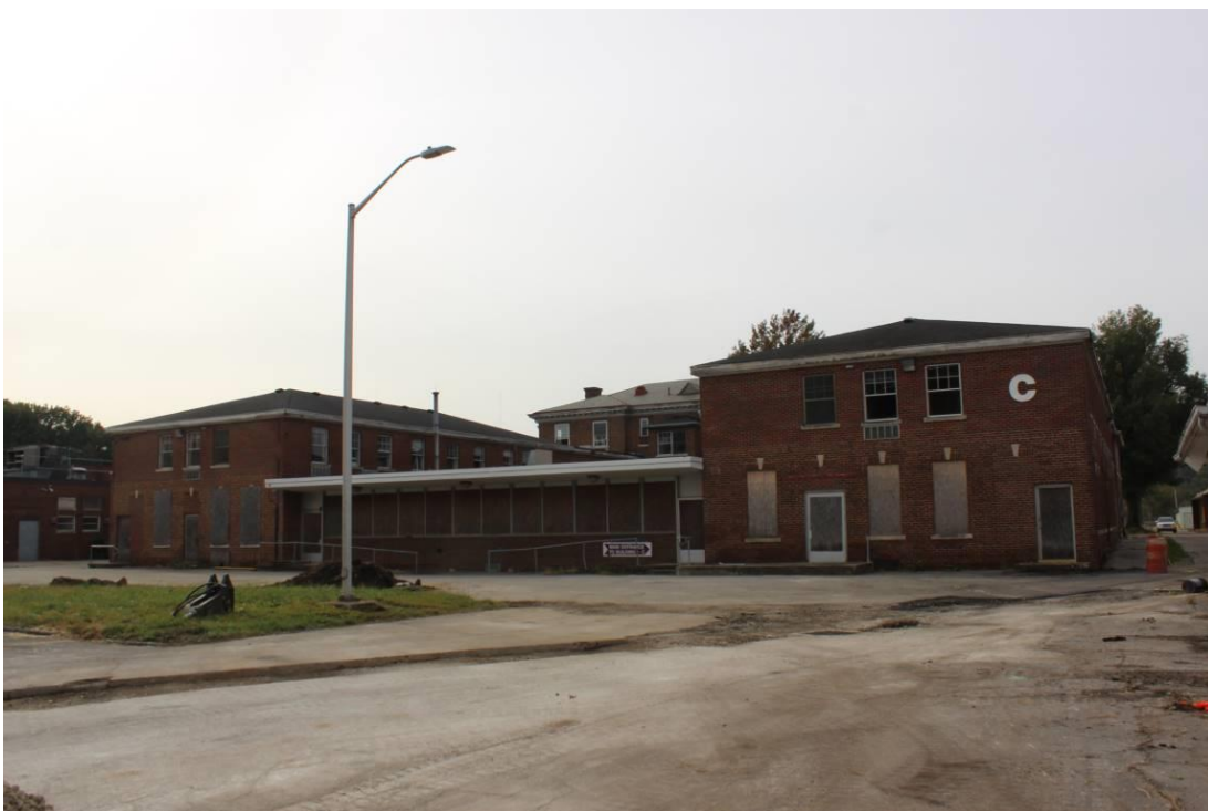
Photo #6: Rear (north) facade, camera facing south
