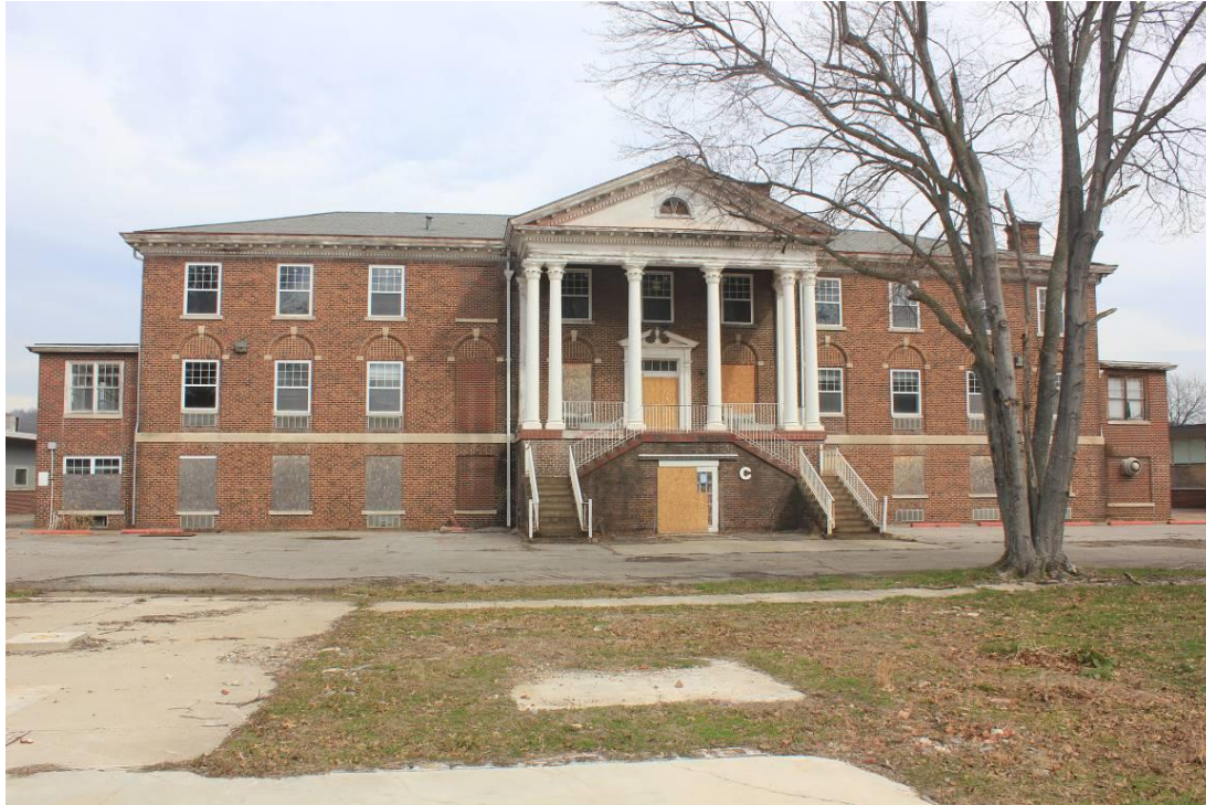
Photo 1: South façade, camera facing north
