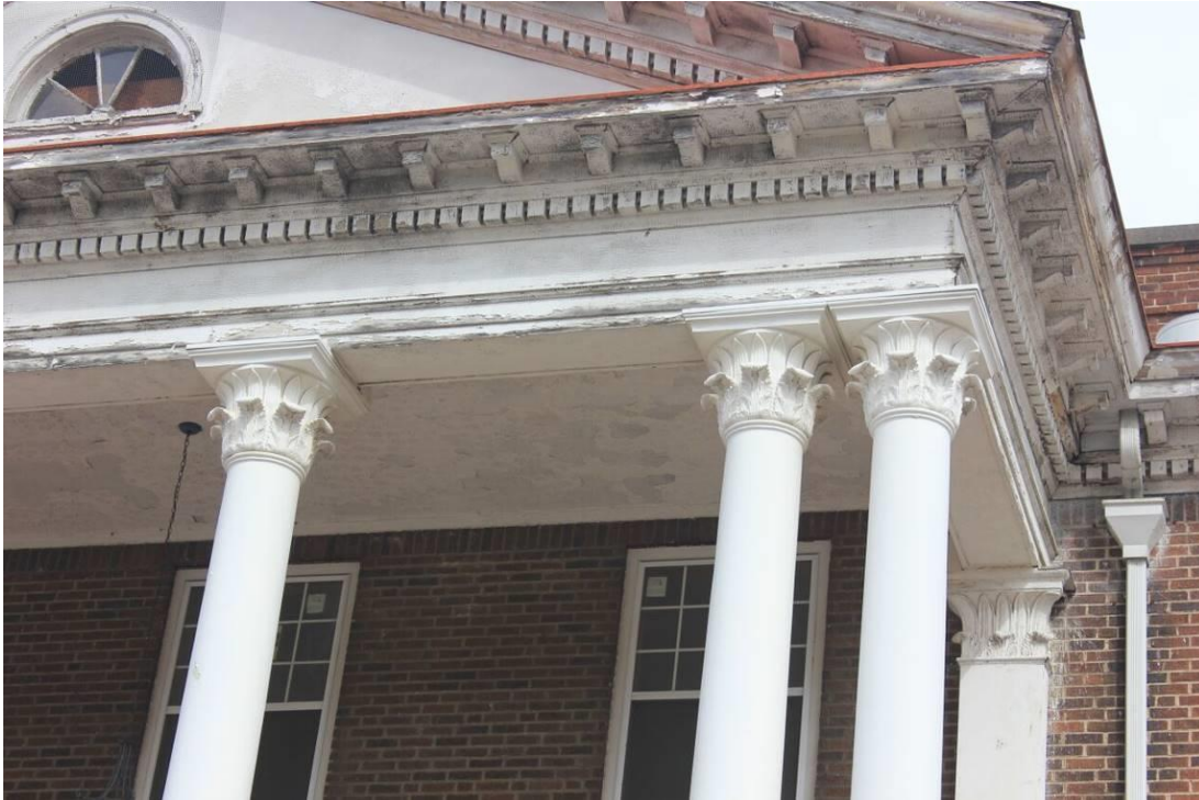
Photo #9: View of the portico architectural details, camera facing north
