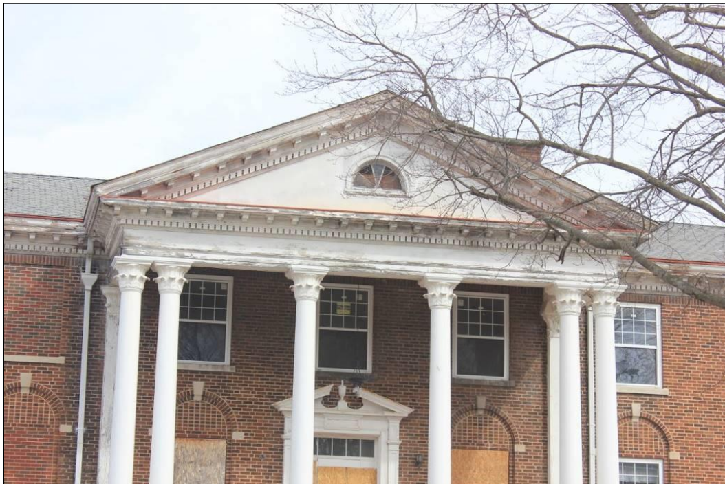
Photo 3: South Façade, portico, camera facing north
