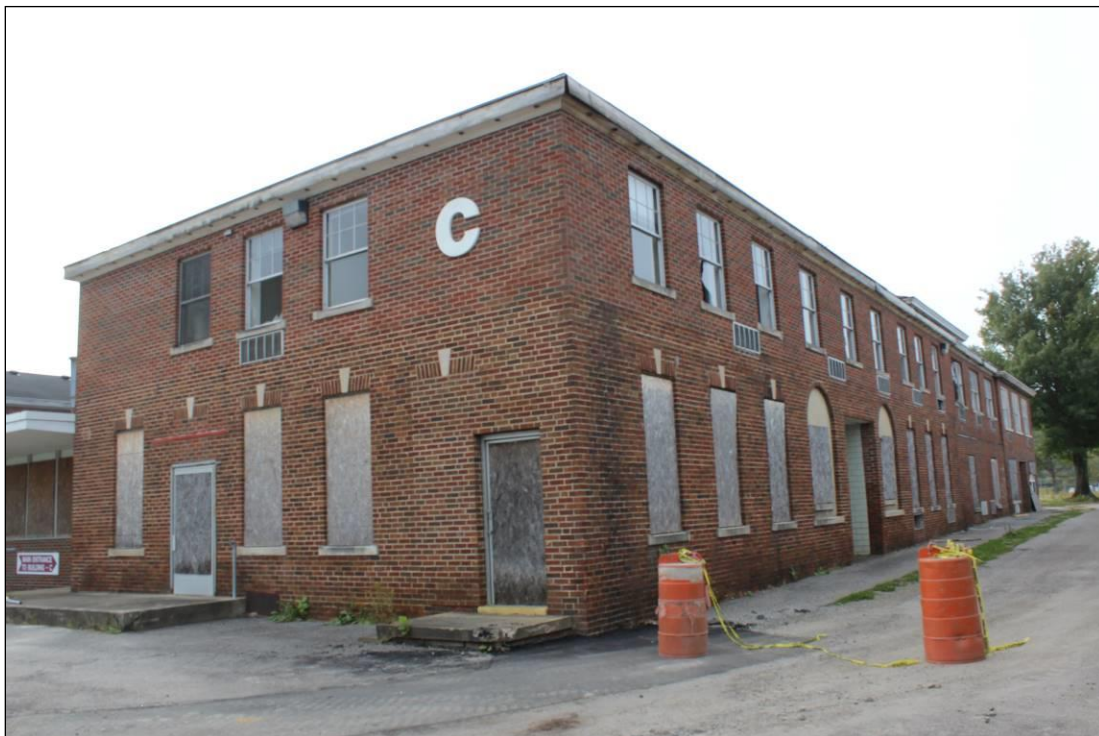
Photo 9: Oblique view of west wing, camera facing south
