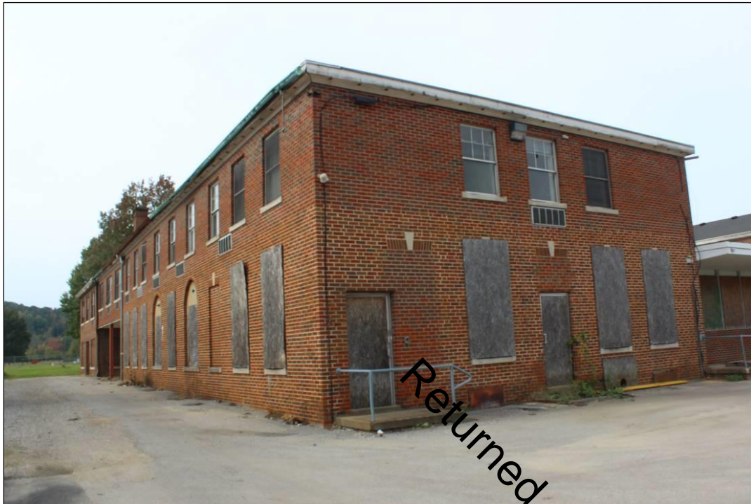
Photo 6: Oblique view of east wing, camera facing southwest
