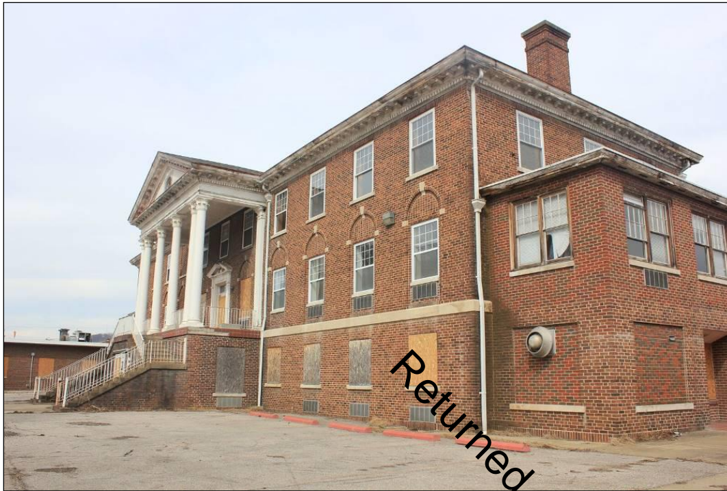
Photo 4: Oblique view of the central structure, camera pointing northwest
