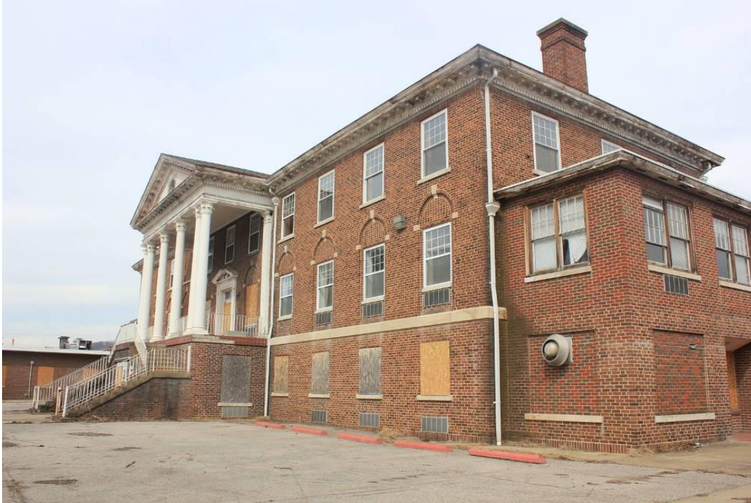
Photo #3: Oblique view of the central structure, camera pointing northwest
