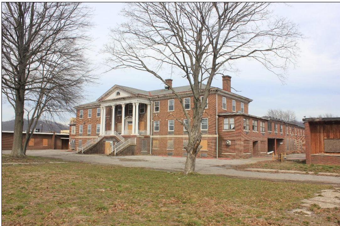
Photo 11: Overview photo, camera facing northwest
