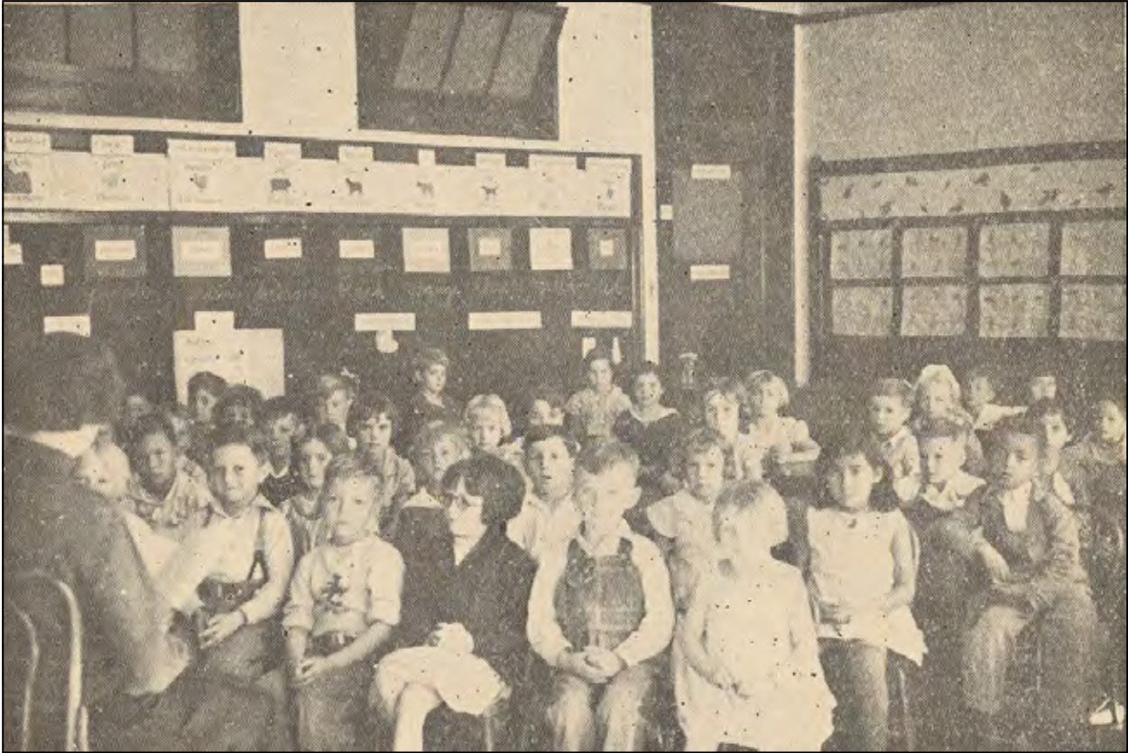
Figure 11: 1923 building classroom, 1935 (Clark County School District)
