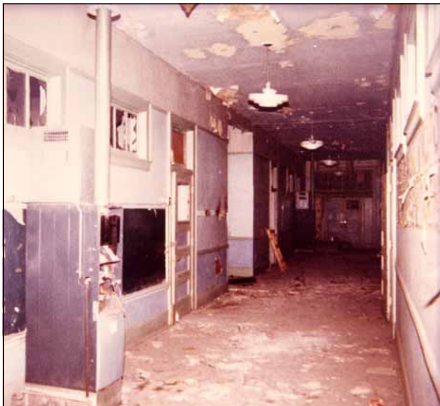
Figure 18: 1923 building corridor, 1982 (Clark County School District Archive)
