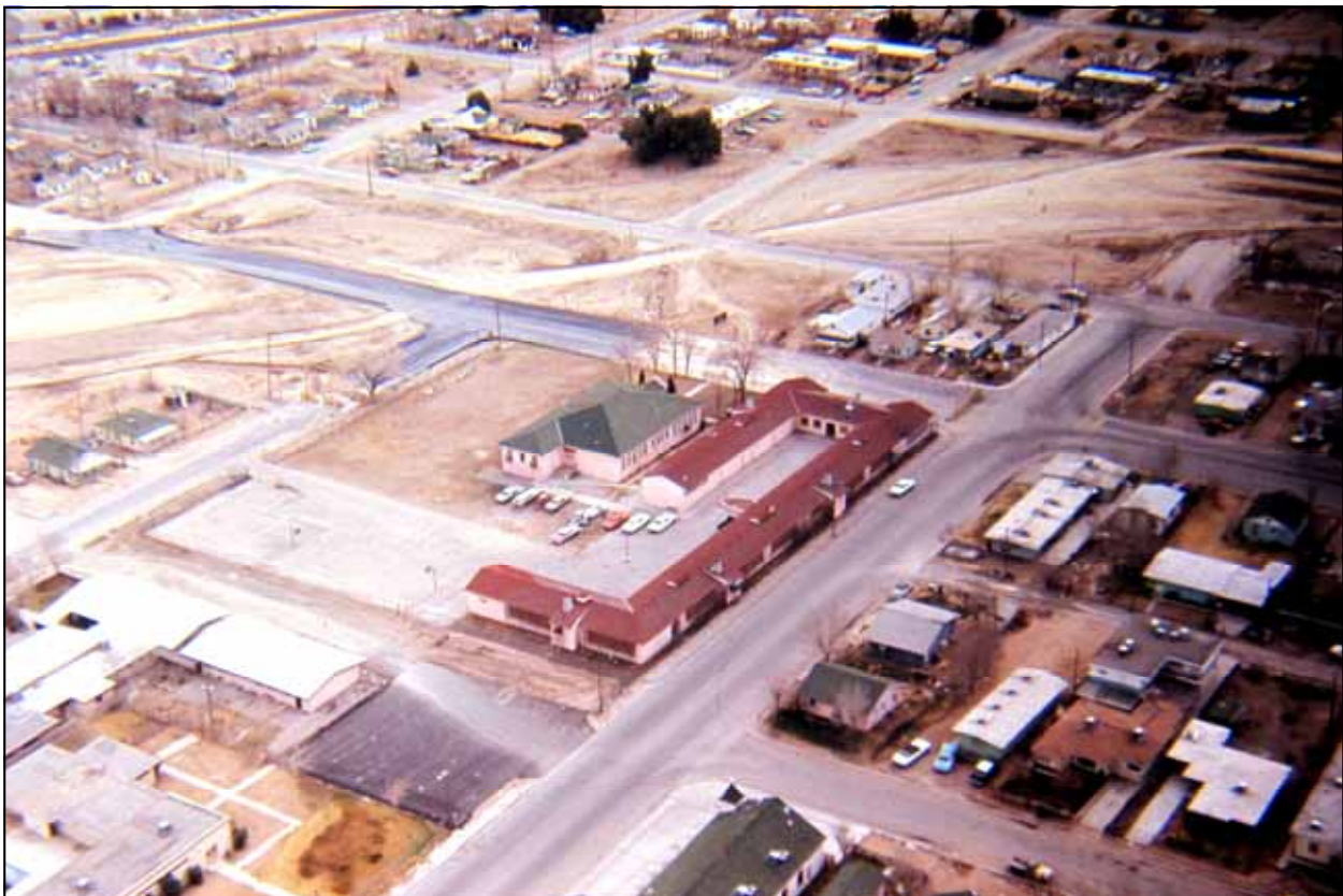
Figure 14: Aerial, view southeast, 1969 (Clark County School District Archive)
