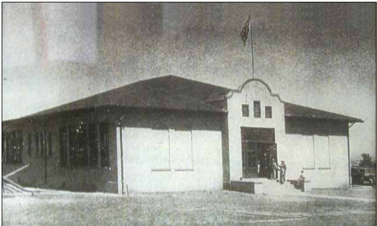
Figure 4: 1923 building, c. 1930 (Clark County School District Archive)
