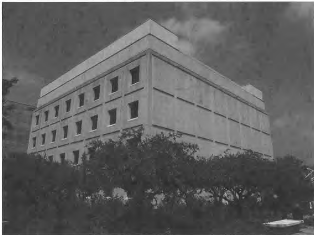
Figure 44. 1972 Addition to Building 54, south and west elevations, facing northeast
