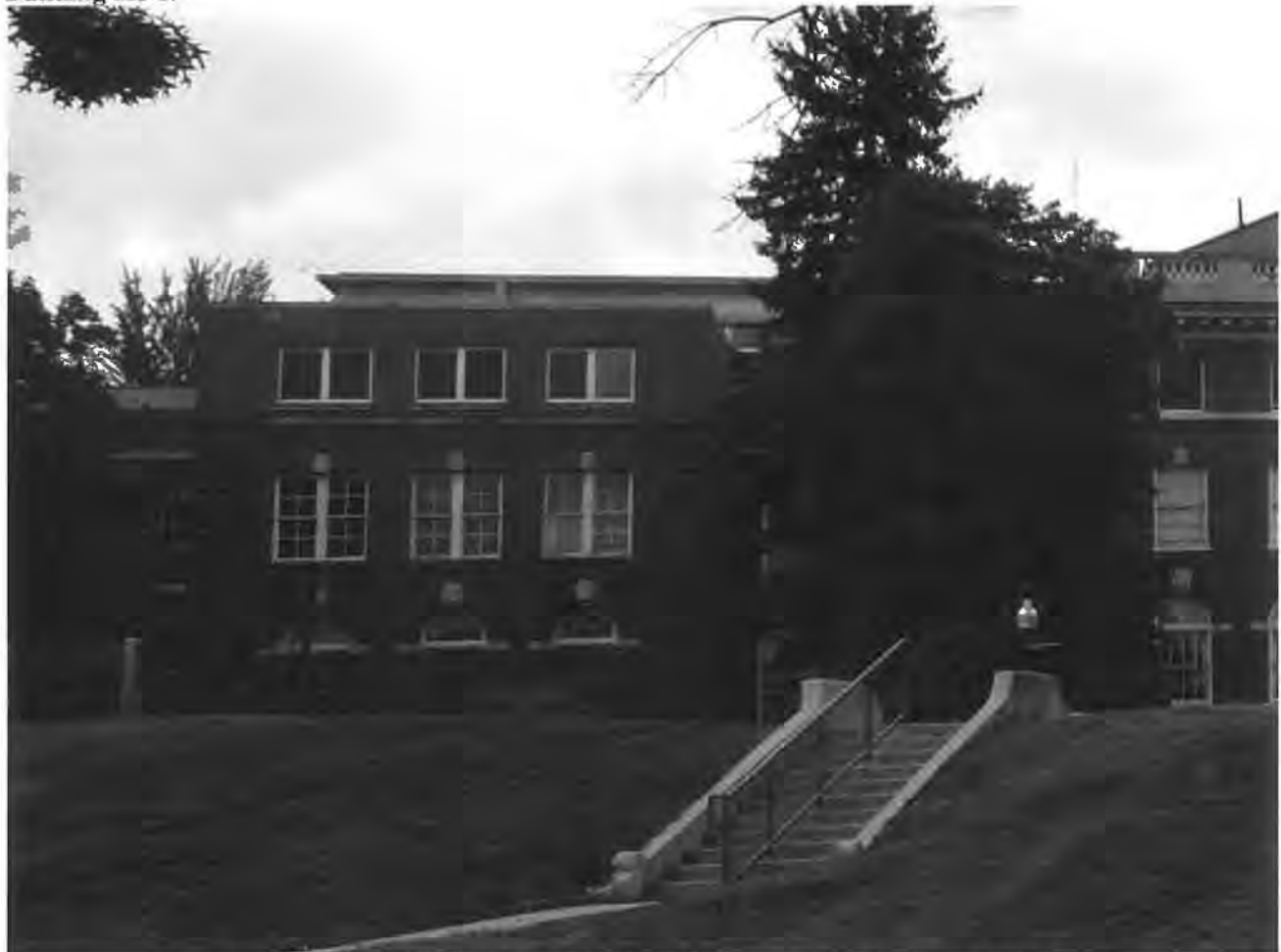
Figure 5. Main Hospital, Building 1A, West Pavilion, south elevation, facing north
