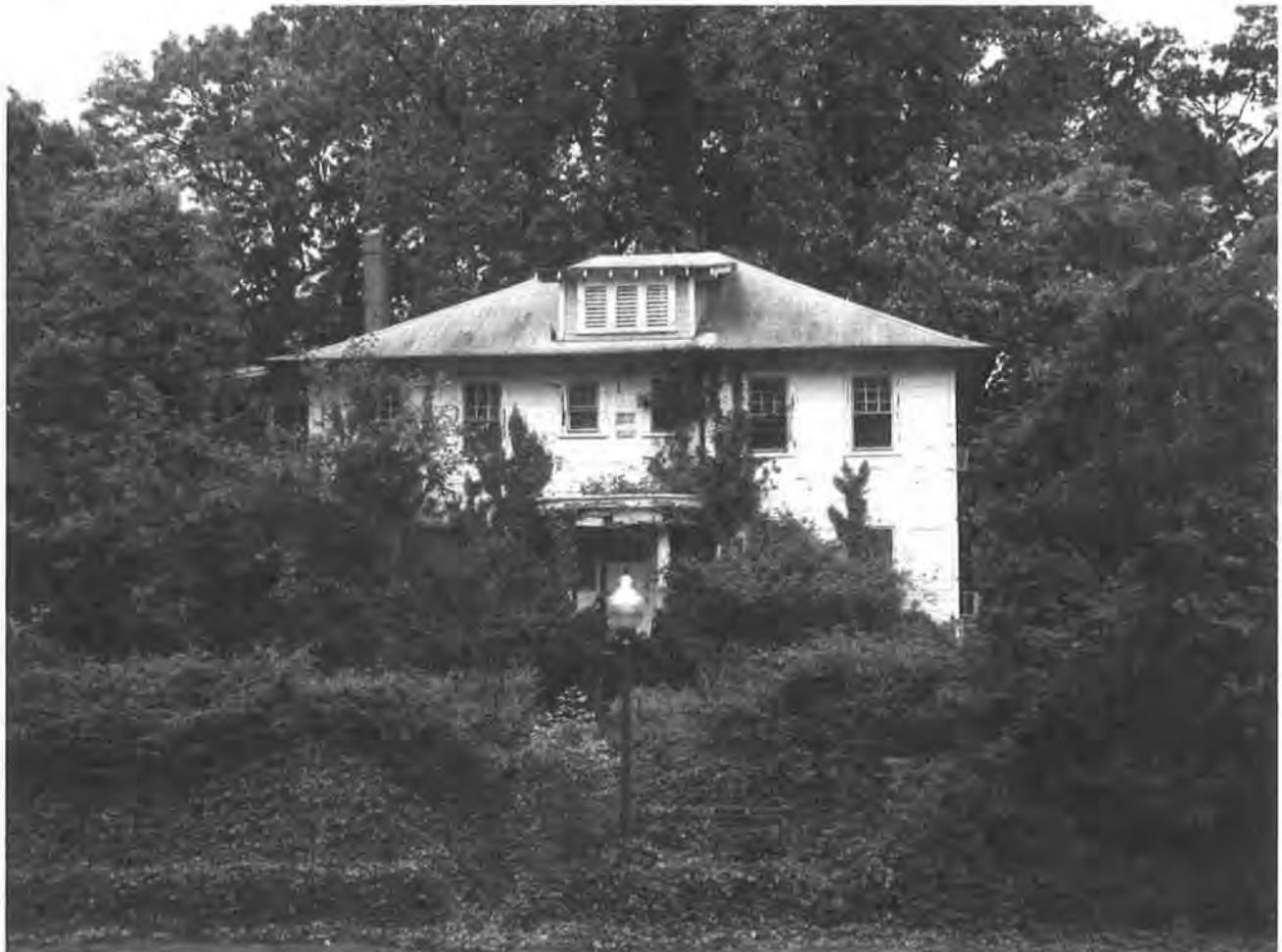
Figure 23. Building 25, east (main) elevation, facing west
