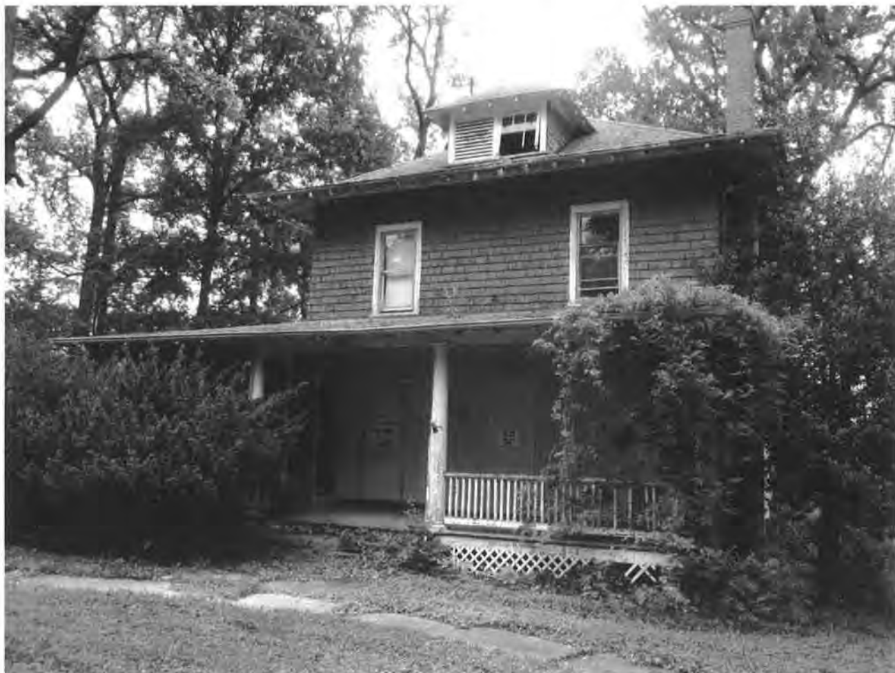
Figure 27. Building 35, northwest (main) elevation, facing southeast
