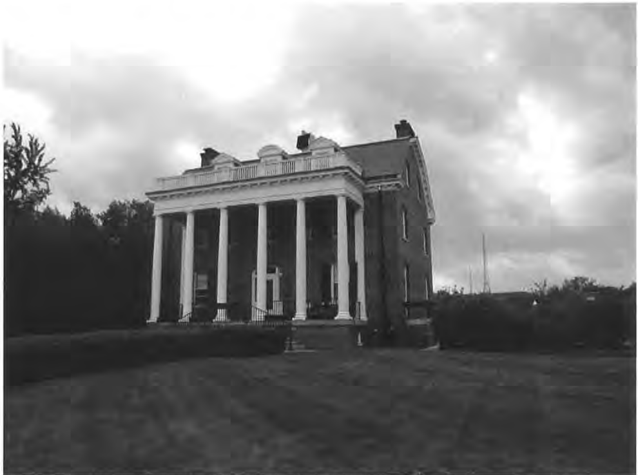
Figure 16. Building 8, Officer Quarters 1, main (north) and west elevation, facing southeast
