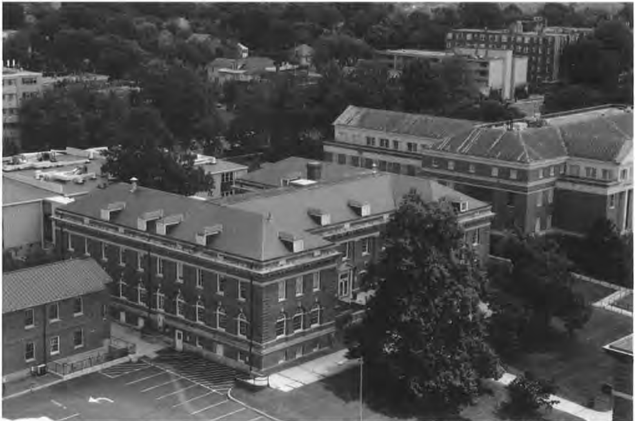
Figure 15. Barracks, Building 7, north and west elevations, facing southeast
