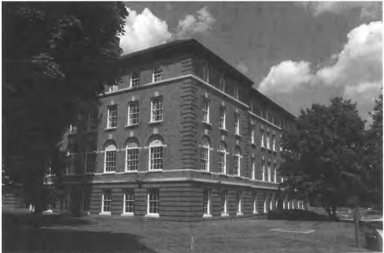
Figure 10. Main Hospital, Building 1F, East Wing, southwest corner, facing northeast
