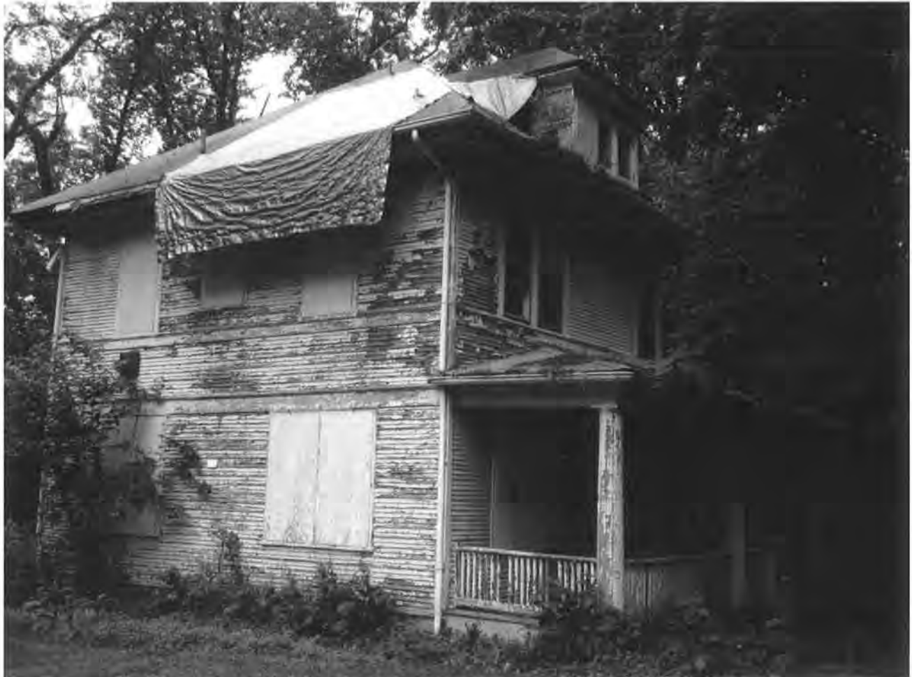
Figure 26. Building 30, north (main) and east elevation, facing southwest
