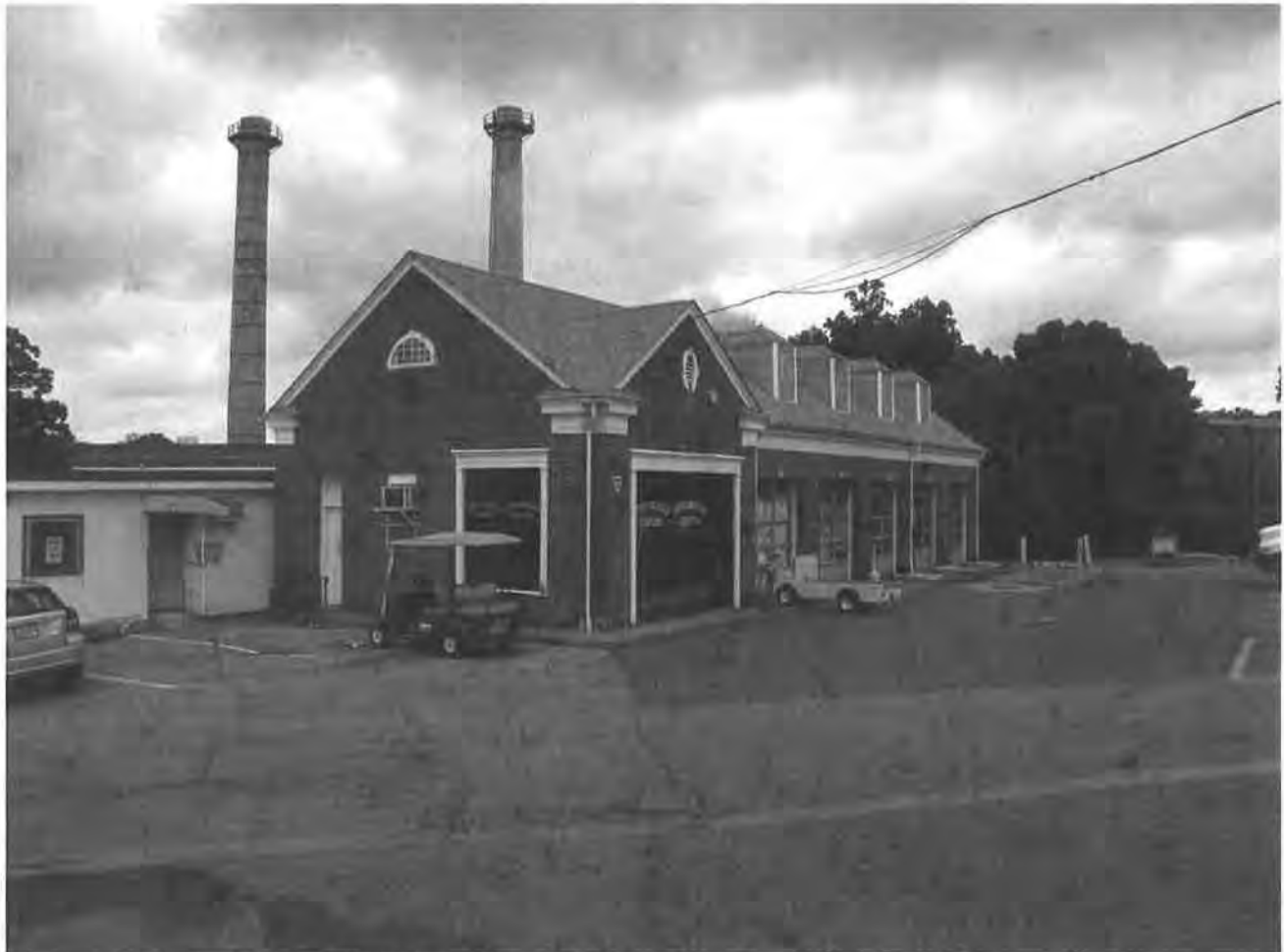
Figure 38. Building 82, northeast (main) and southeast elevations, facing southwest
