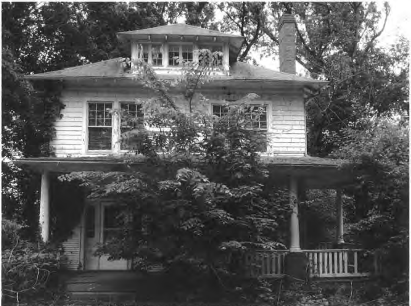
Figure 24. Building 26, north (main) elevation, facing south
