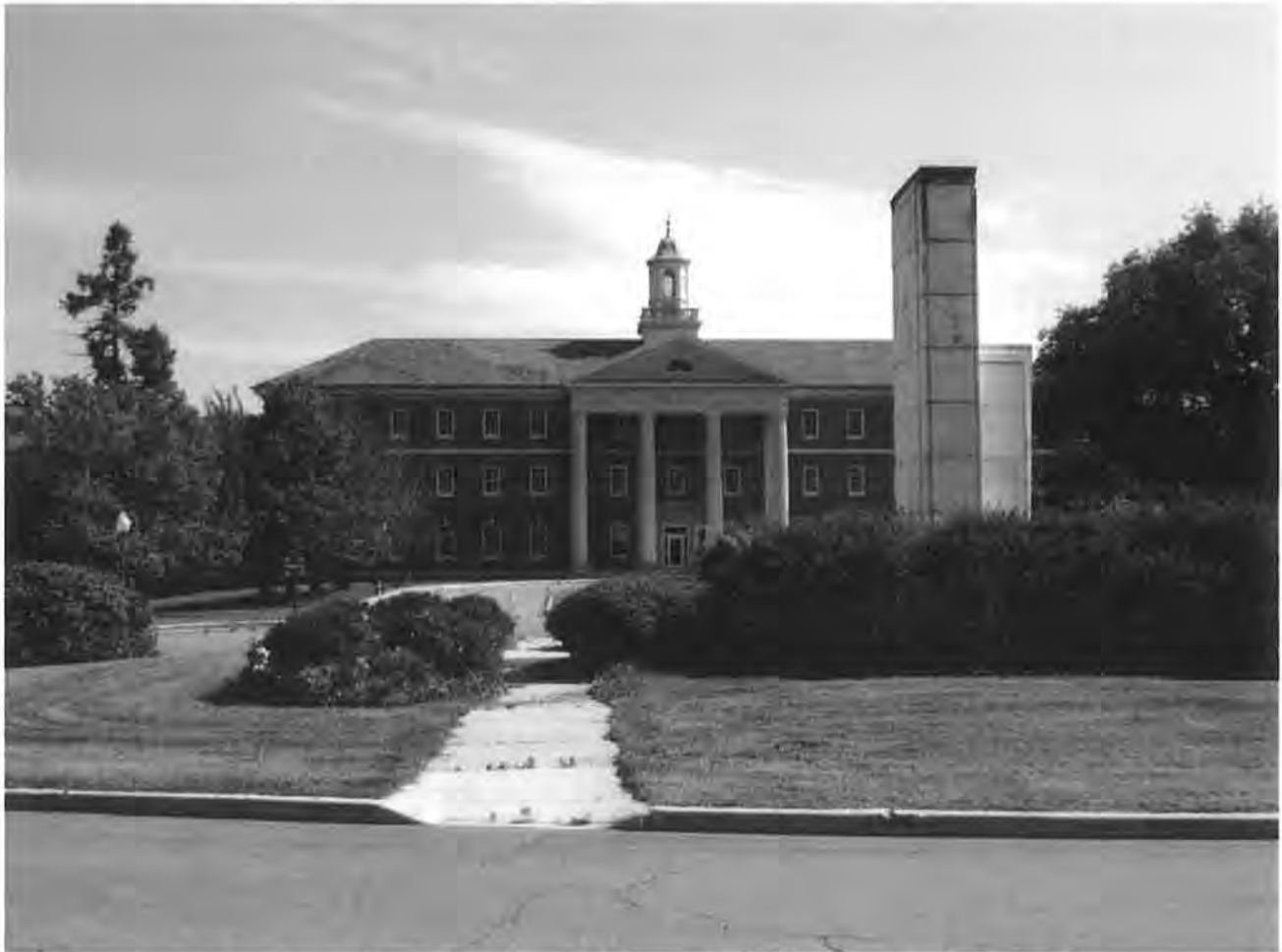
Figure 34. Building 11A, Center Wing, north (main) elevation, facing south
