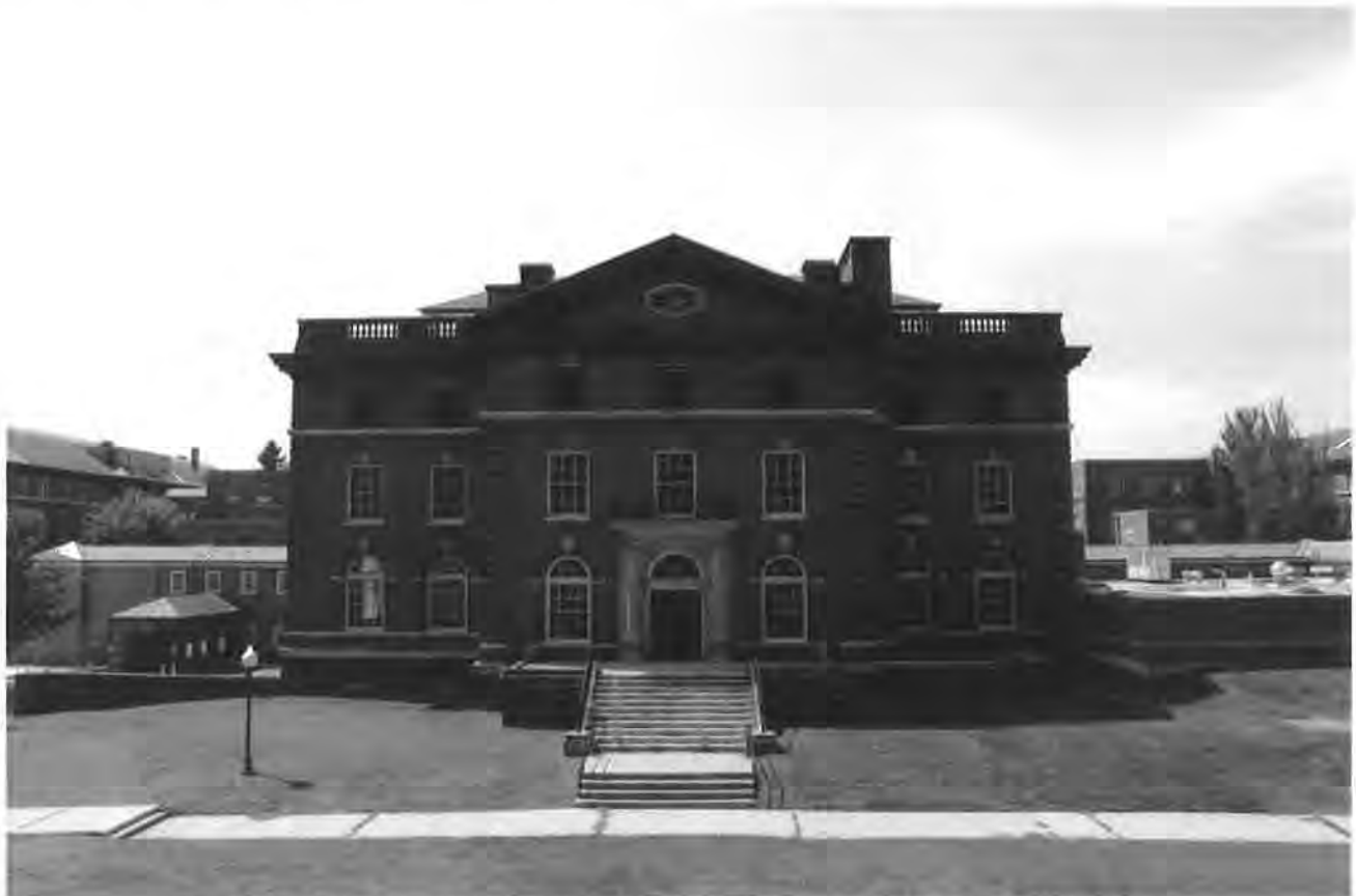
Figure 8. Main Hospital, Building 1D, North Wing, north elevation, facing south
