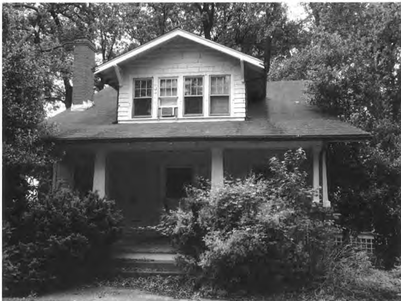
Figure 22. Building 22, north (main) elevation, facing south
