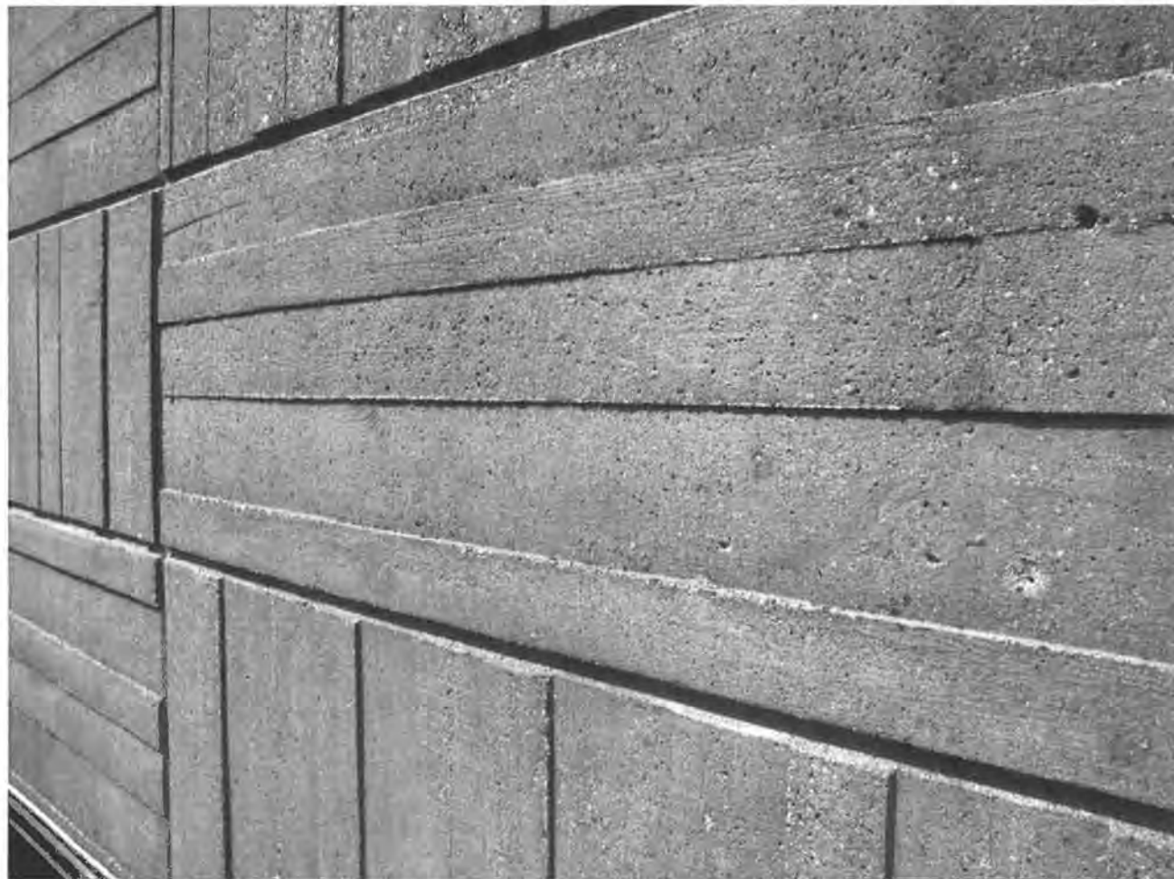
Figure 43. Distinctive texturing of concrete walls in the original block of Building 54
