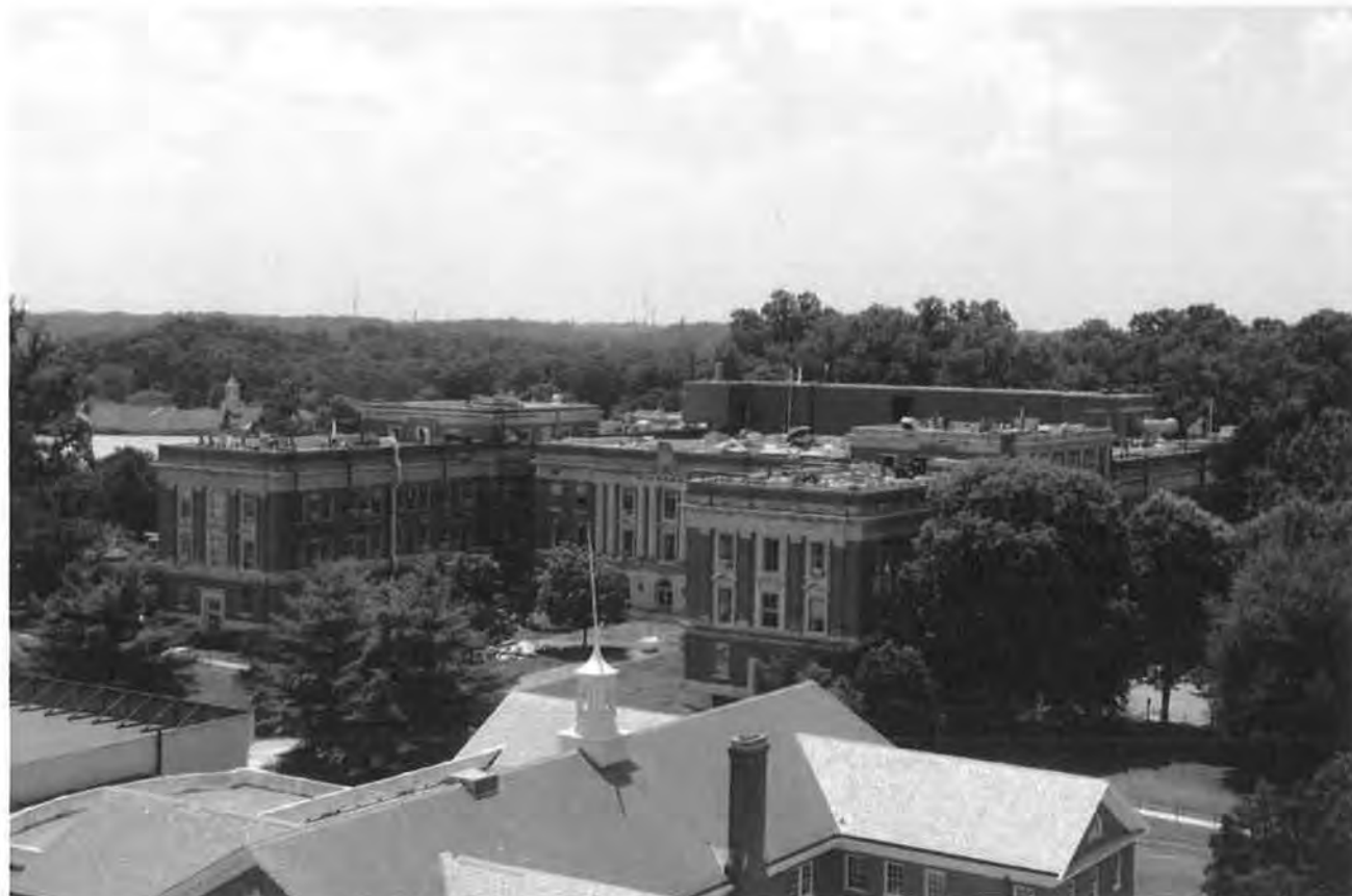
Figure 31. Buildings 40, 40A, and 40B, east and north elevations, facing southwest
