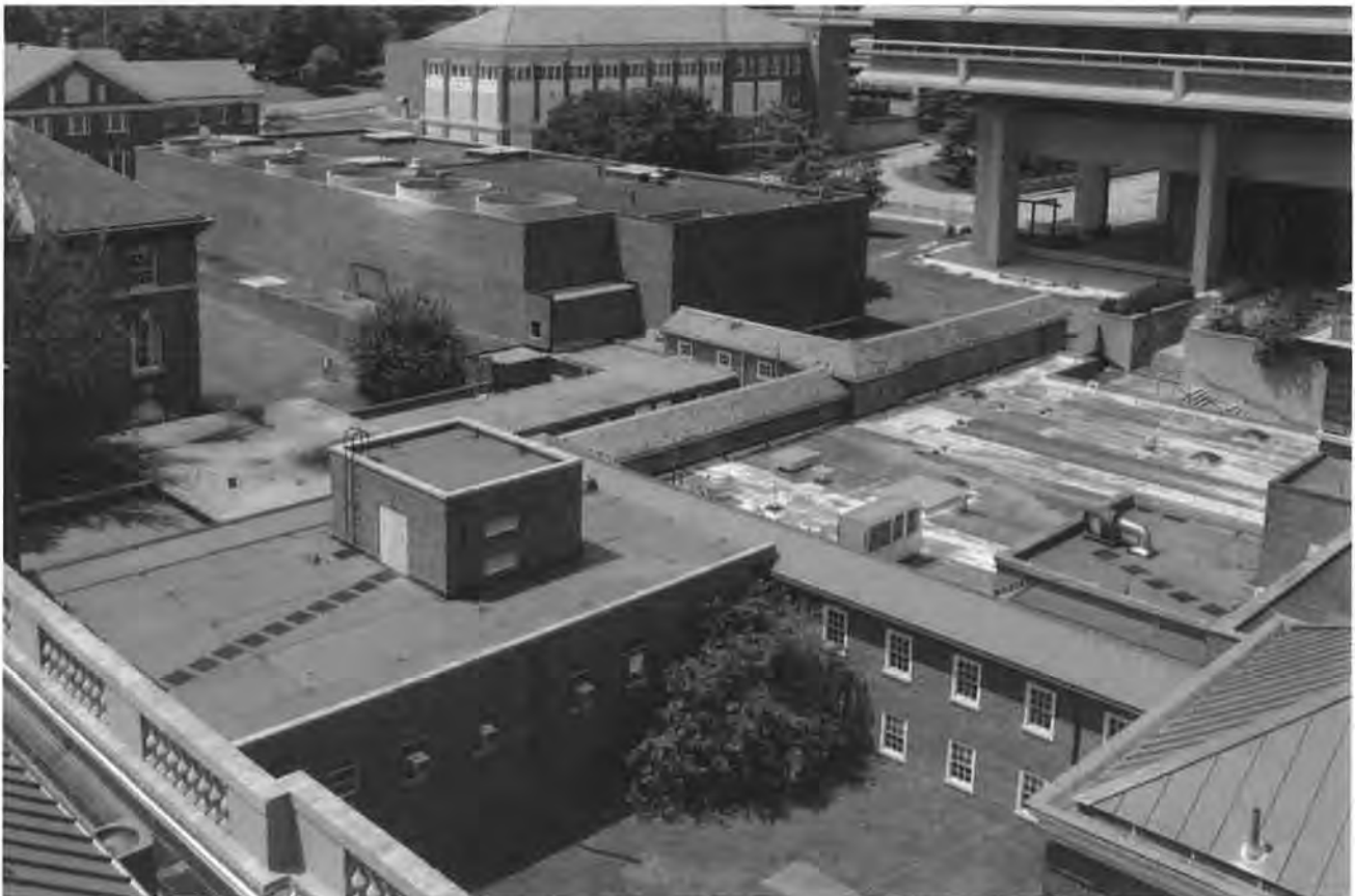
Figure 12. Main Hospital, Buildings 1J and 1K, Admissions Office, lower left of frame
