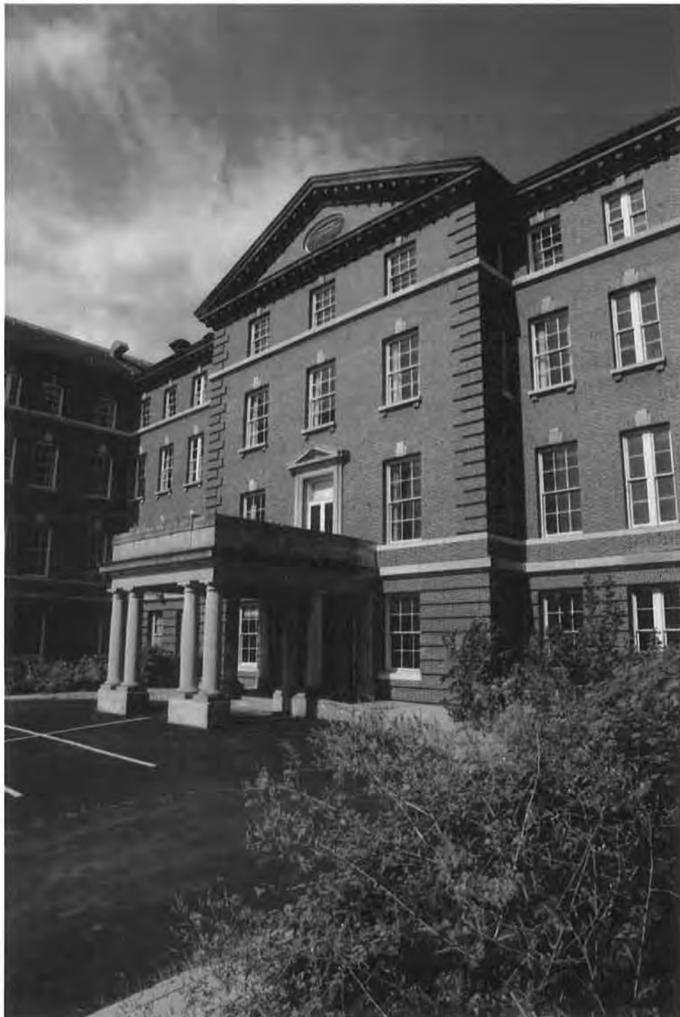
Figure 9. Main Hospital, Building 1E, West Wing, main elevation, facing northeast
