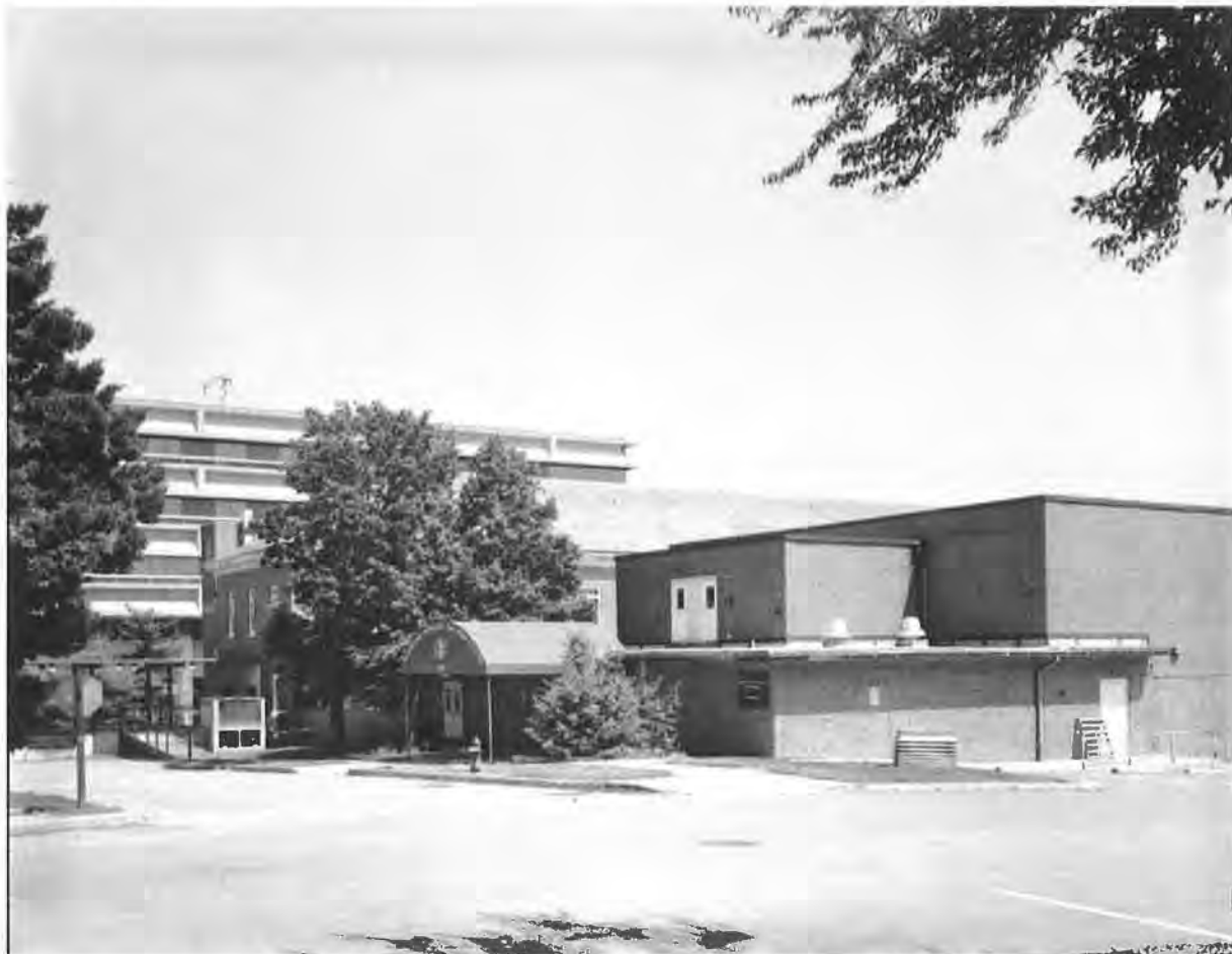
Figure 41. Building 53, north (main) and west elevations, facing east
