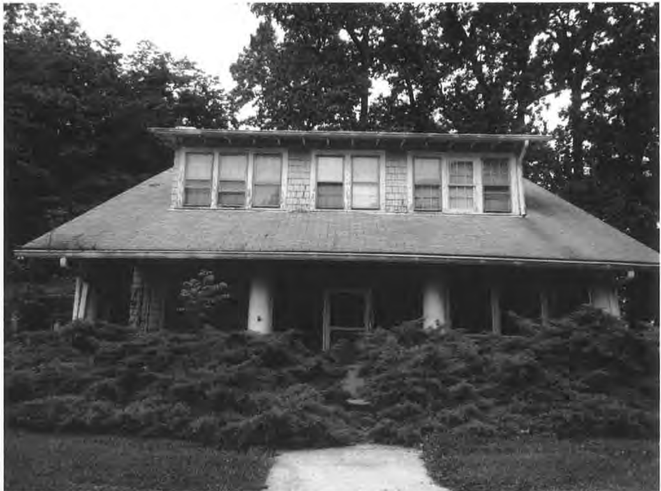
Figure 21. Building 21, east (main) elevation, facing west
