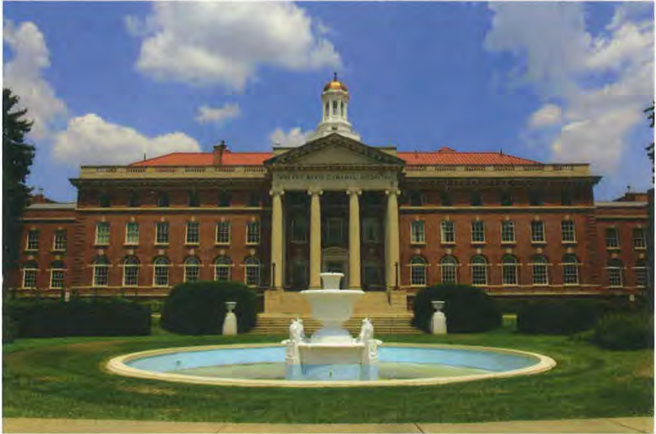
Figure 2. Main Hospital, Building 1, Main Elevation
