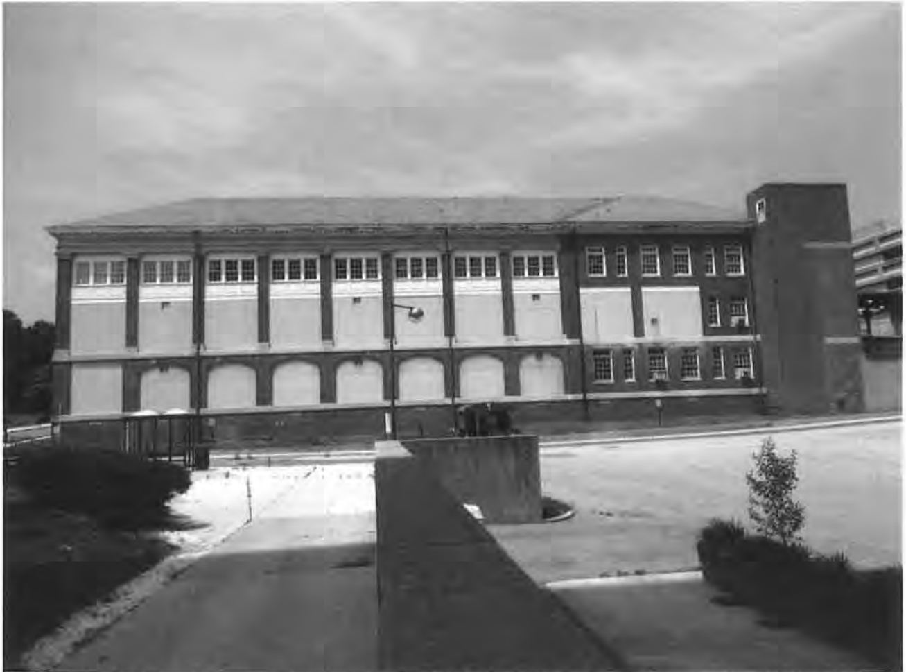
Figure 35. Building 52, east (main) elevation displaying infill of porch openings and fenestration, facing west
