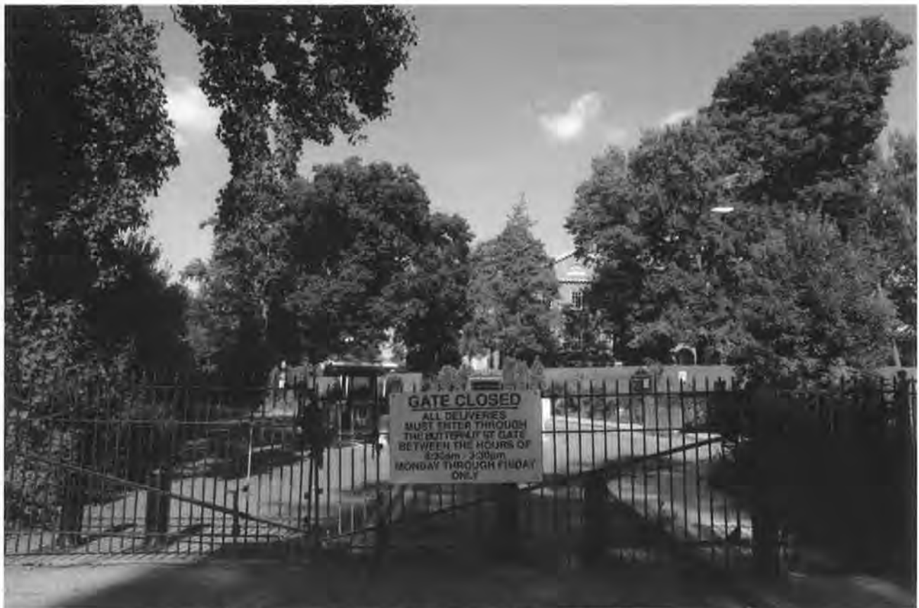
Figure 46. Structure 413, Iron Perimeter Fencing at 16th Street Entrance
