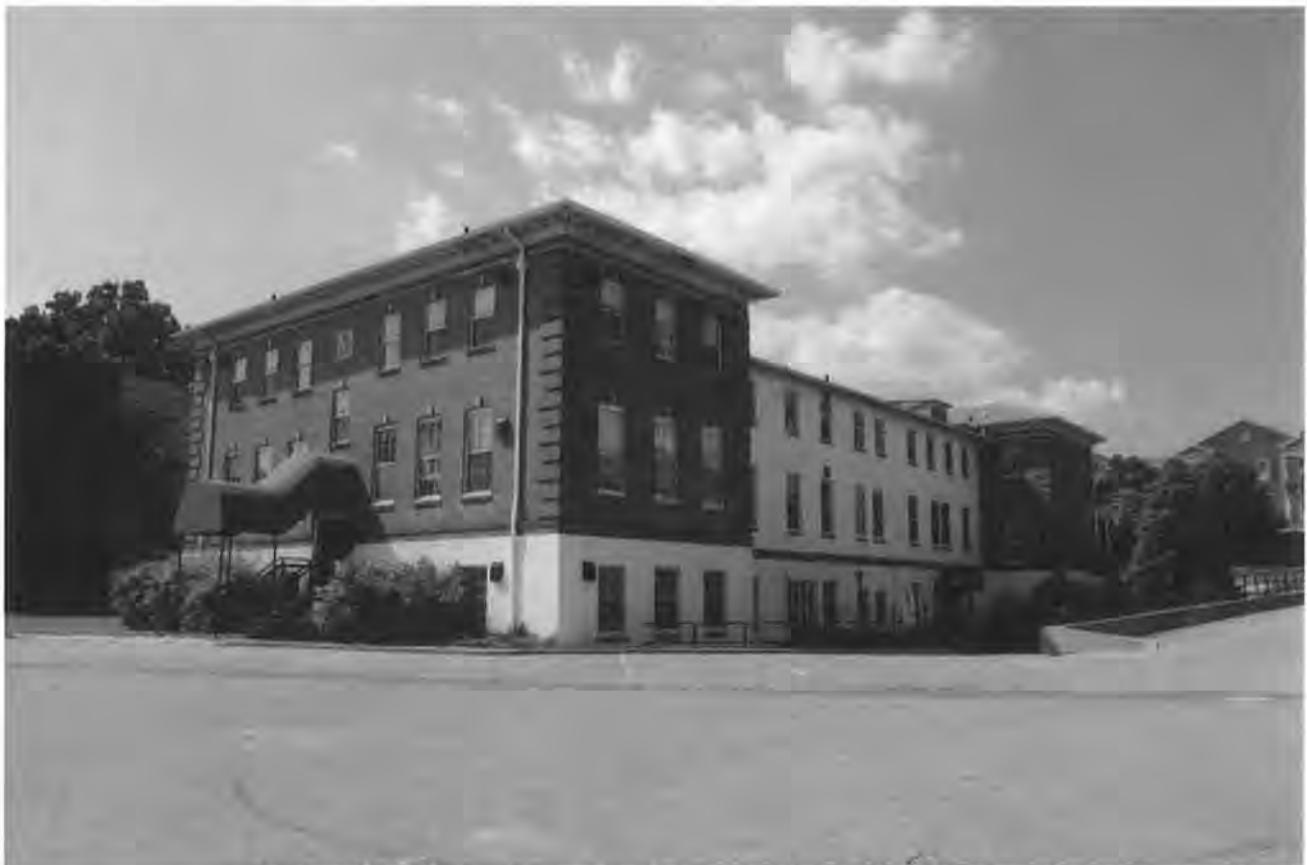
Figure 28. Building 17, south and east elevations, facing northwest
