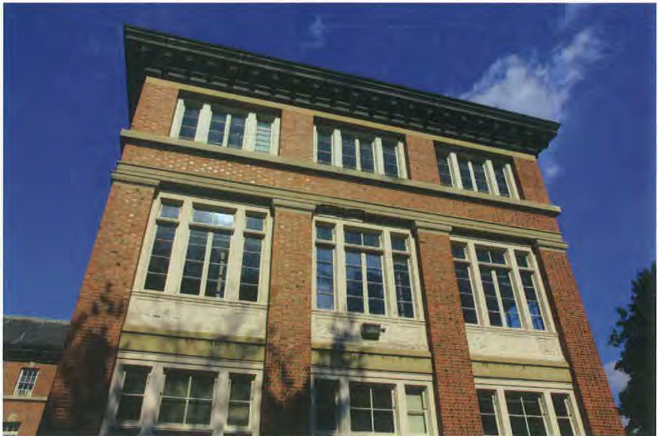
Figure 6. Main Hospital, Building 1B, East Pavilion, south elevation, facing north
