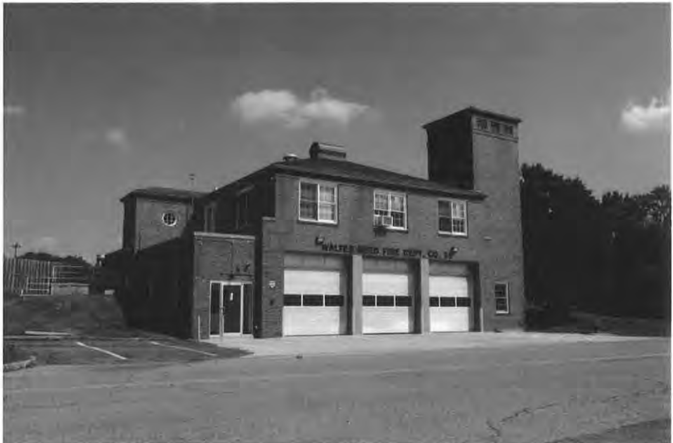
Figure 40. Building 90, south (main) and west elevations, facing northeast
