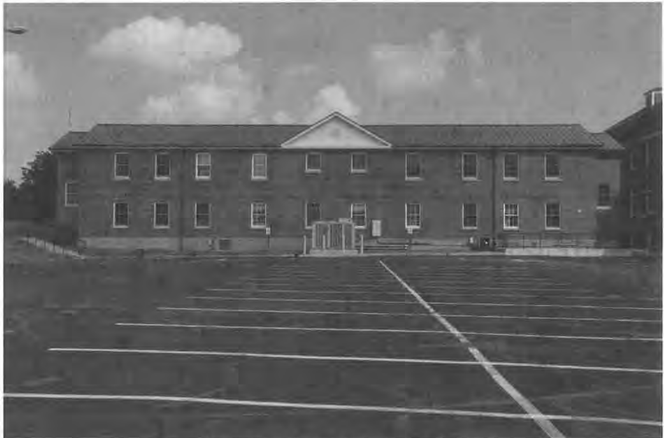
Figure 30. Building 38, west (rear) elevation, facing east
