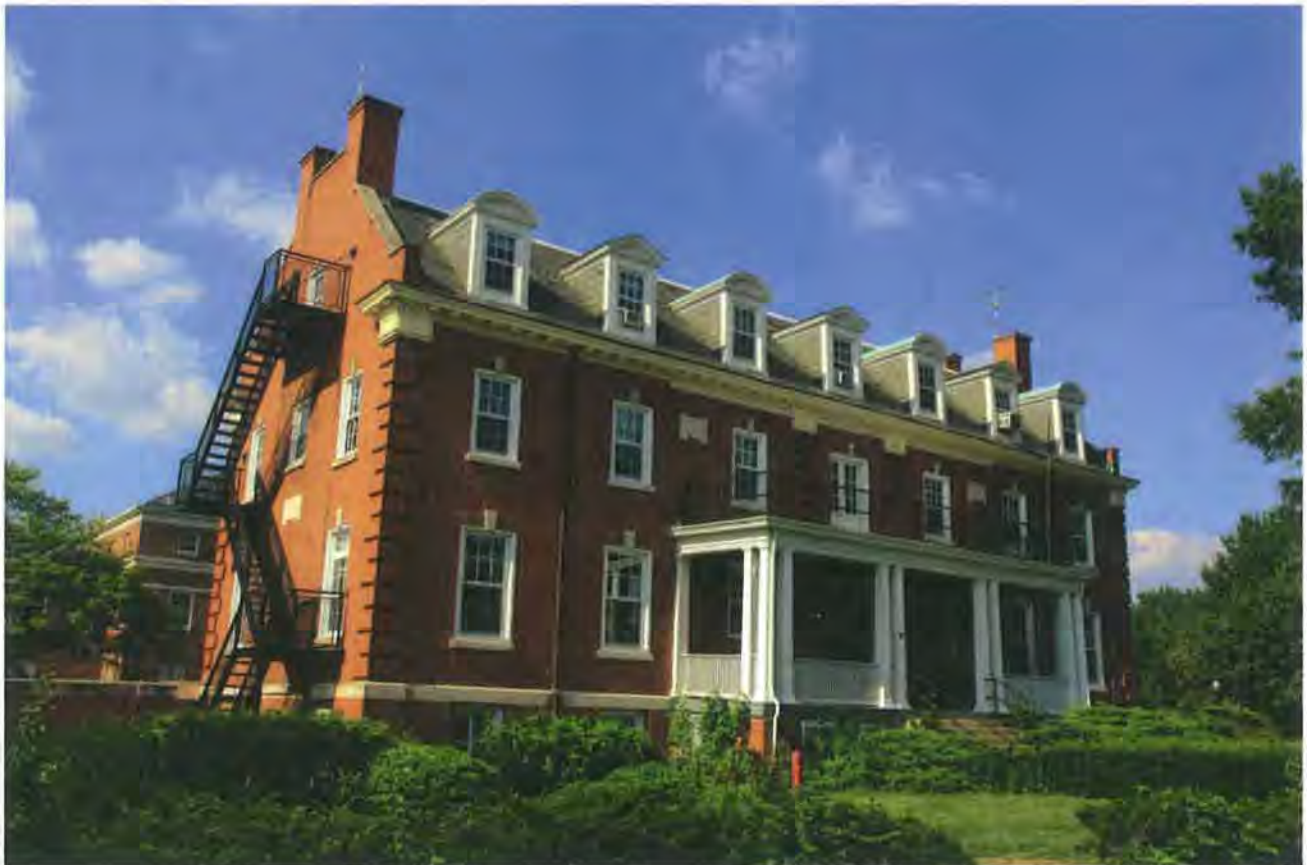
Figure 18. Building 12, south (main) and west elevation, facing northeast
