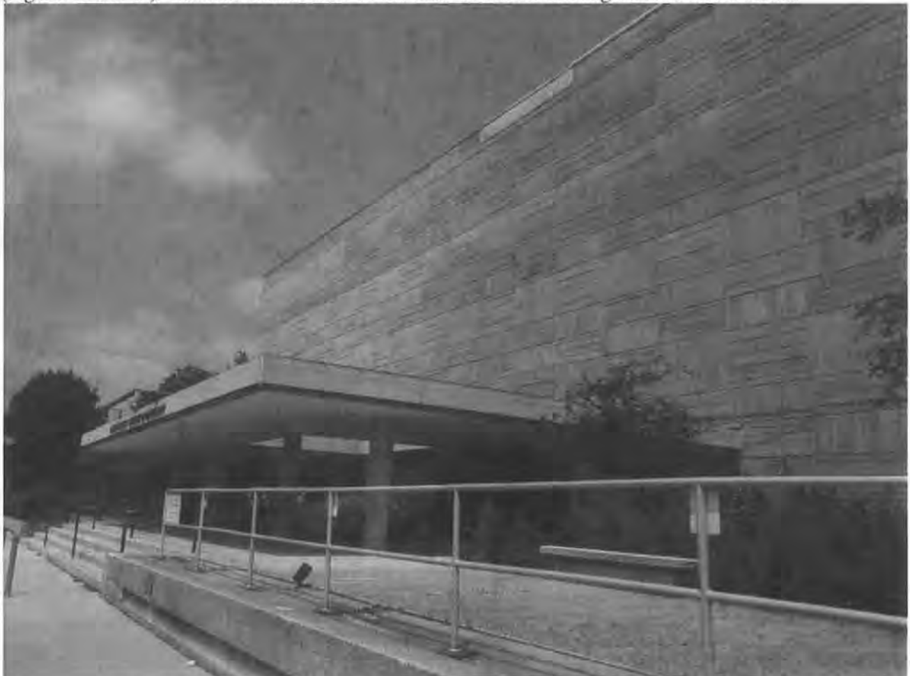
Figure 42. Building 54, west (main) elevation of the original block, facing north
