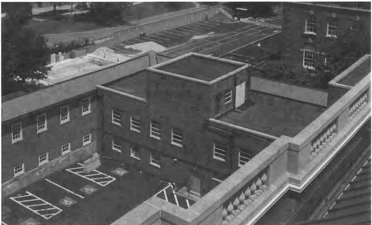
Figure 13. Main Hospital, Building 1L, Cardio-Vascular and Physical Medicine Clinics, center of frame
