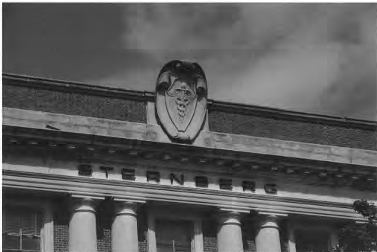
Figure 32. Detail of stone cartouche at front entrance of Building 40A (Sternberg Crossbar Wing)
