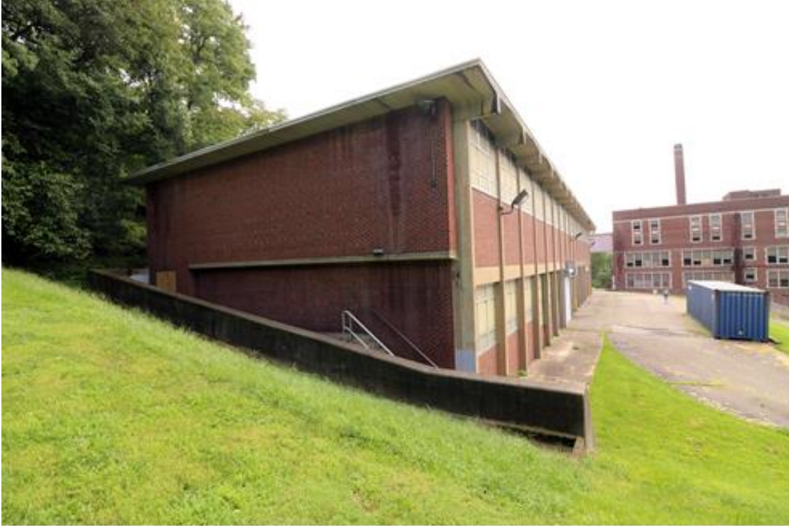
Photo 19: Exterior View, 1914 - 1924 Building, 1965 Non-Contributing Addition, North and West Elevations, Looking Southeast
