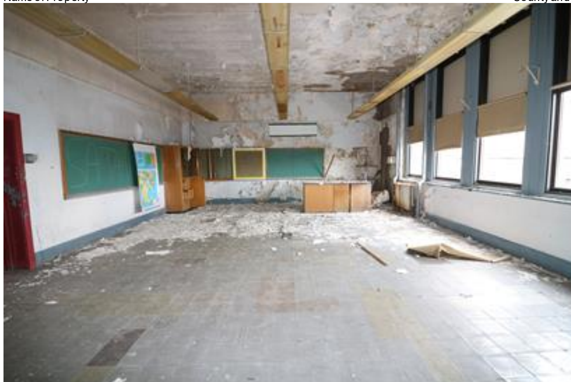
Photo 15: Interior View, 1914 - 1924 Building, Second Floor, Classroom, Looking South
