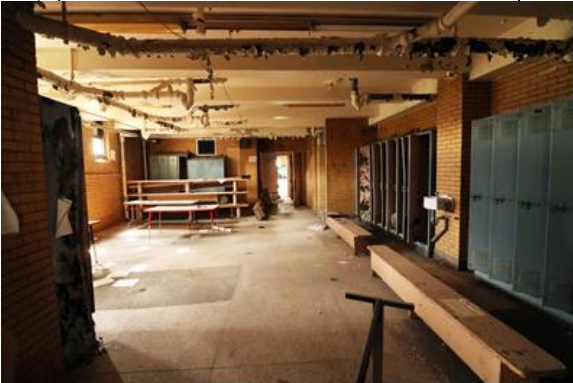
Photo 31: Interior View, 1926 Building, Second Floor, locker room, looking West
