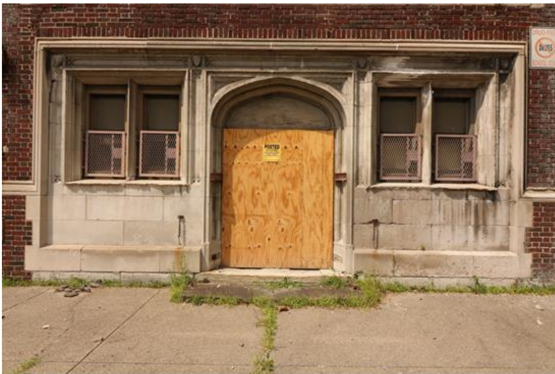
Photo 5: Exterior View, 1914 - 1924 Building, South Elevation Entry, Looking North
