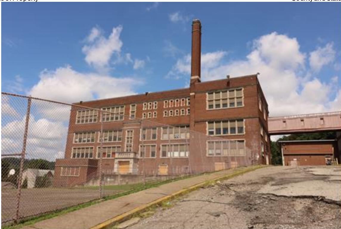
Photo 24: Exterior View, 1926 Building, South Elevation, Looking Northwest
