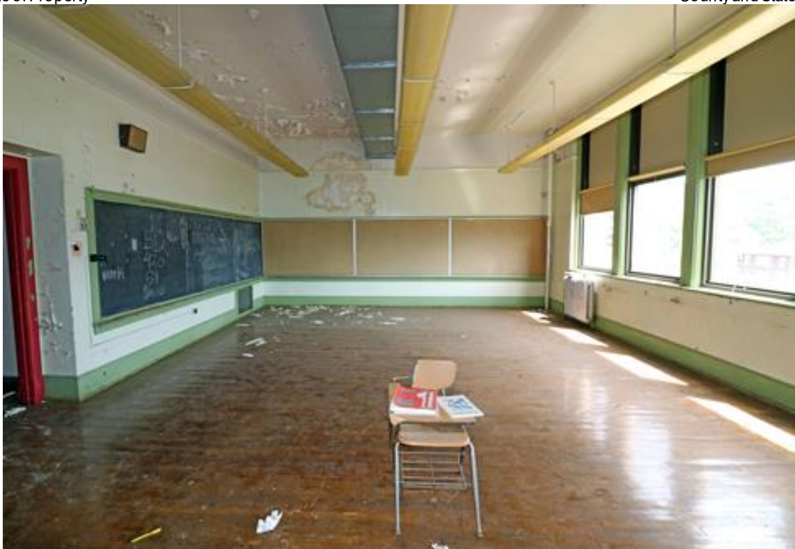
Photo 29: Interior View, 1926 Building, First Floor, Typical Classroom, Looking West.
