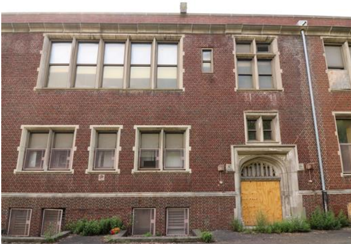
Photo 10: Exterior View, 1914 - 1924 Building, East Elevation at Center, Looking West
