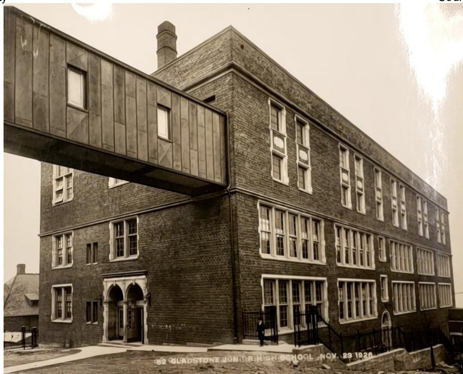
Figure 11: Photograph showing a rear view of the completed Annex Building and Skybridge c.1926.
