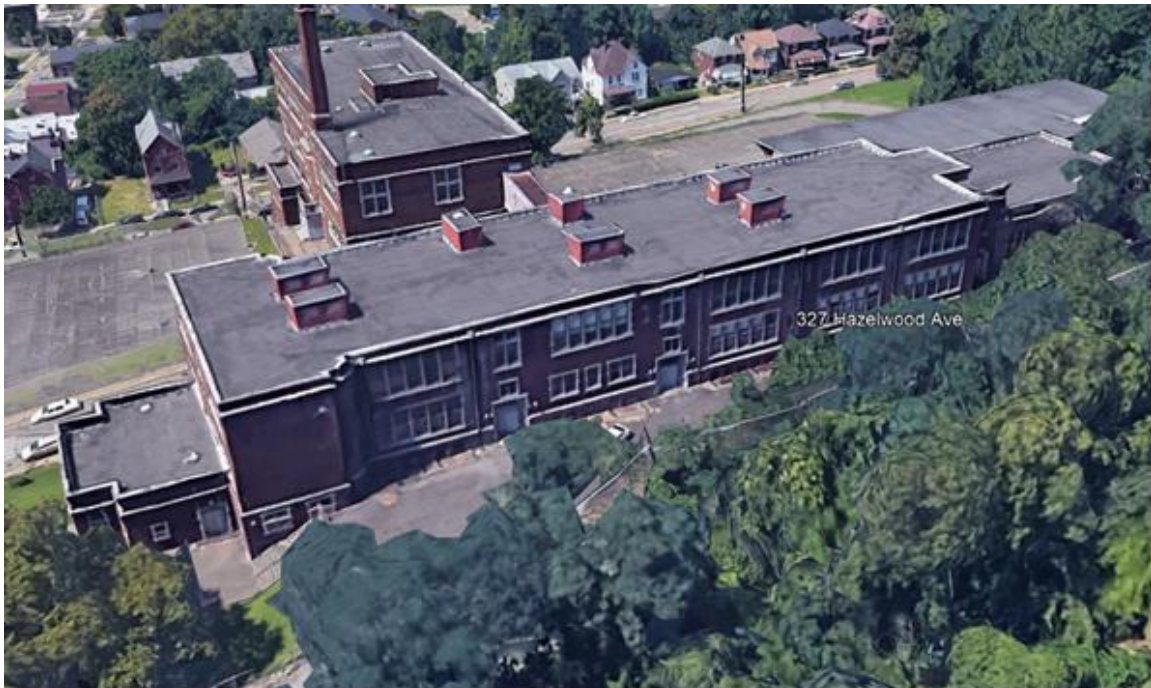
Figure 2: Aerial View of the east elevation, looking west. Image Source: Google Earth
