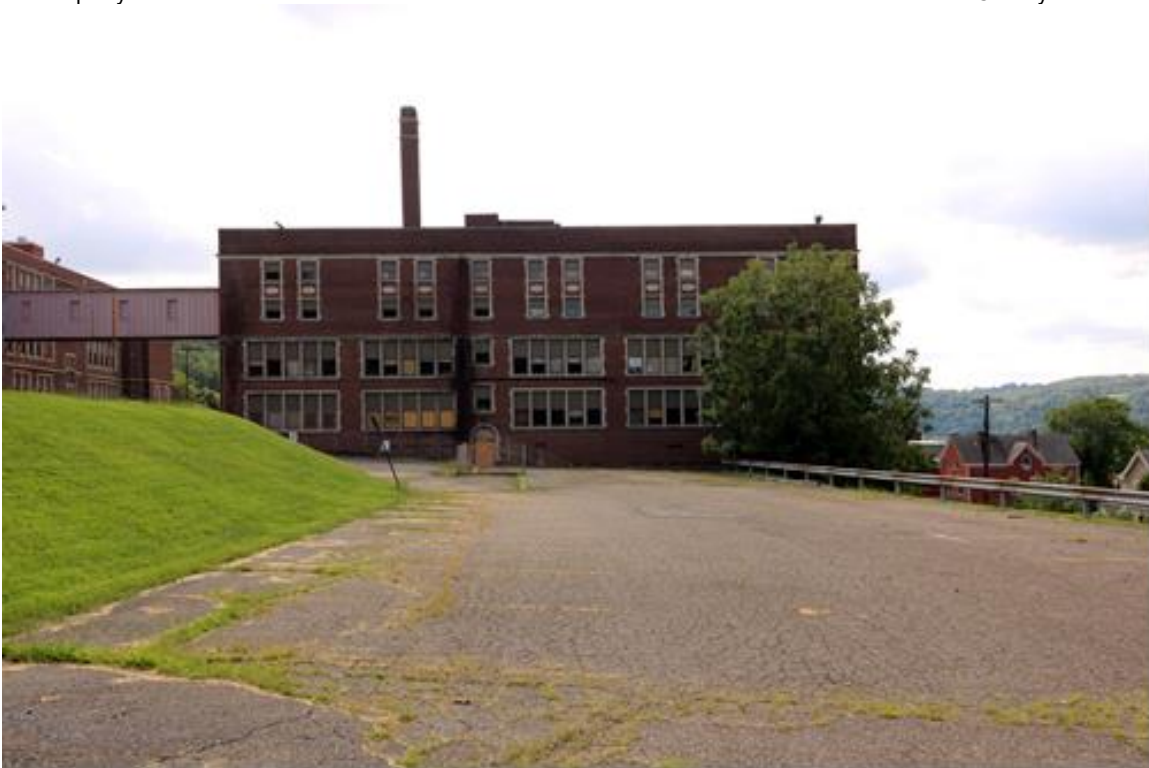
Photo 26: Exterior View, 1926 Building, North Elevation, Looking South
