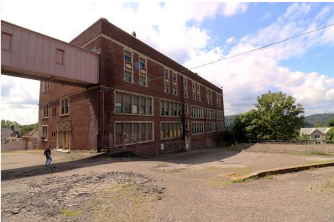
Photo 27: Exterior View, 1926 Building, North and East Elevations, Looking Southwest
