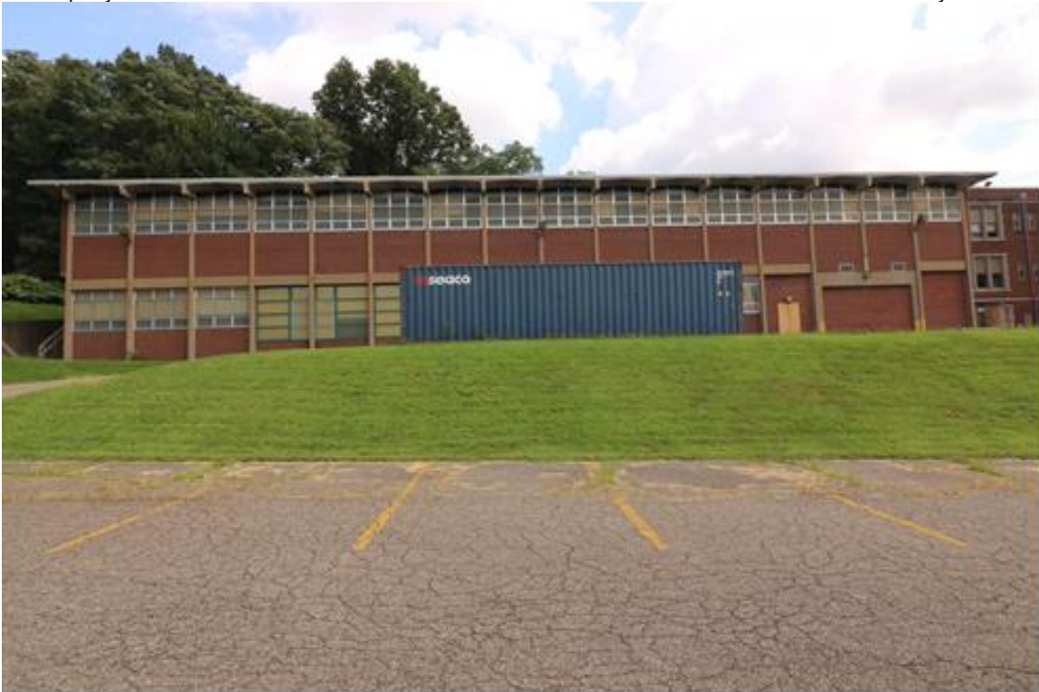
Photo 18: Exterior View, 1914 - 1924 Building, 1965 Addition, West Elevation, Looking East
