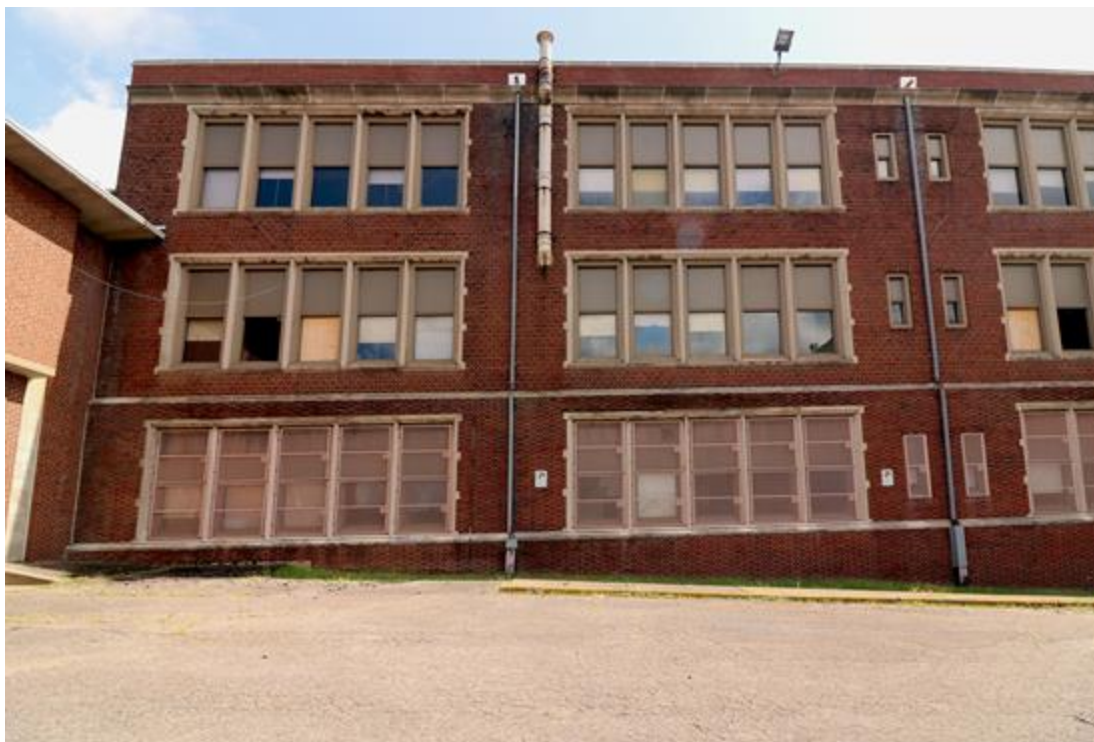
Photo 8: Exterior View, 1914 - 1924 Building, West Elevation at North, Looking East
