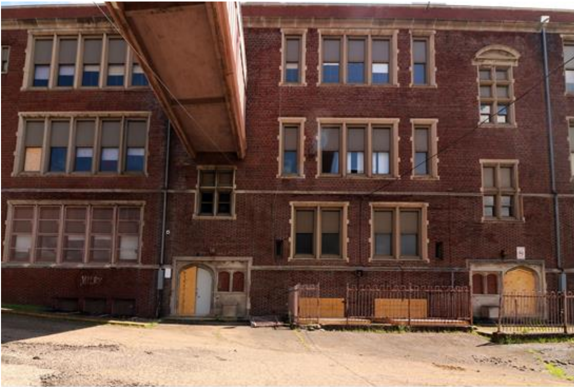
Photo 7: Exterior View, 1914 - 1924 Building, West Elevation at Center, Looking East
