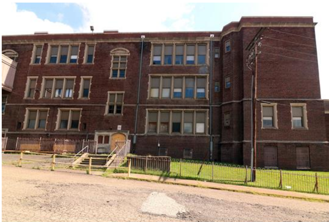
Photo 6: Exterior View, 1914 - 1924 Building, West Elevation, Looking East
