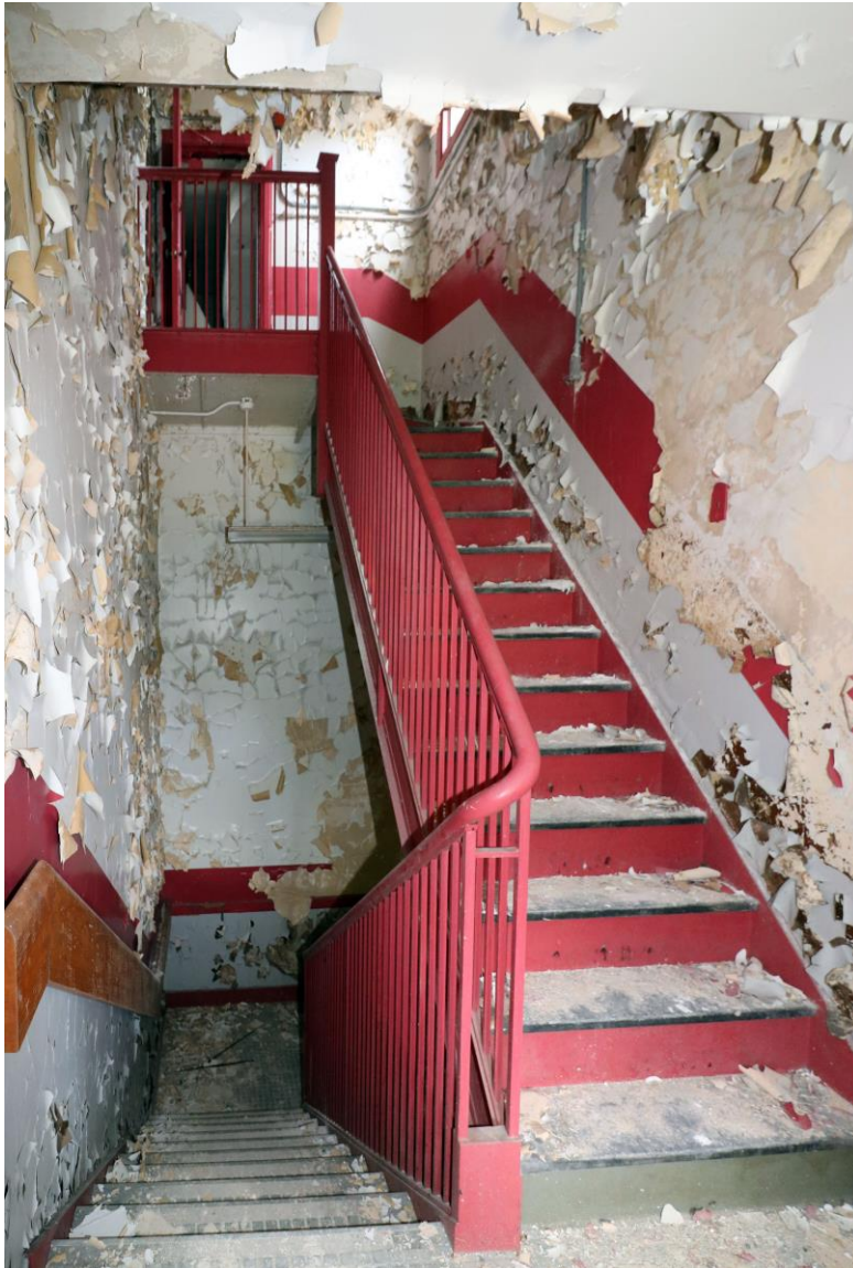
Photo 33: Interior View, 1926 Building, Second Floor, Stair, looking North
