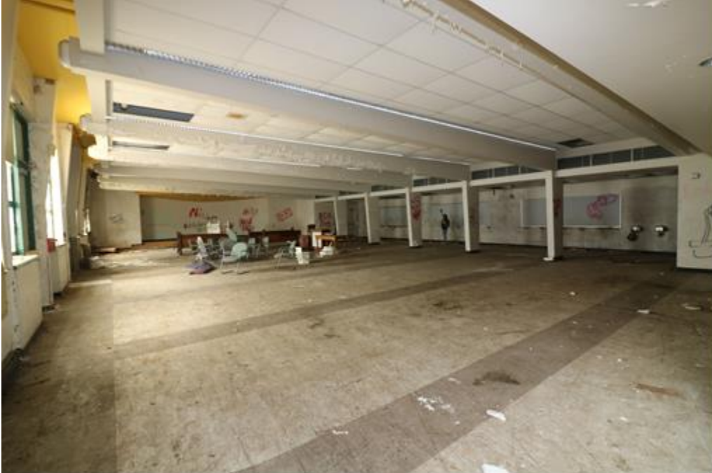
Photo 21: Interior View, 1914 - 1924 Building, 1965 Non-Contributing Addition, Ground Floor, Cafeteria, Looking Northwest
