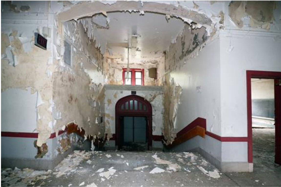
Photo 12: Interior View, 1914 - 1924 Building, First Floor, Hallway at South Center, Looking East
