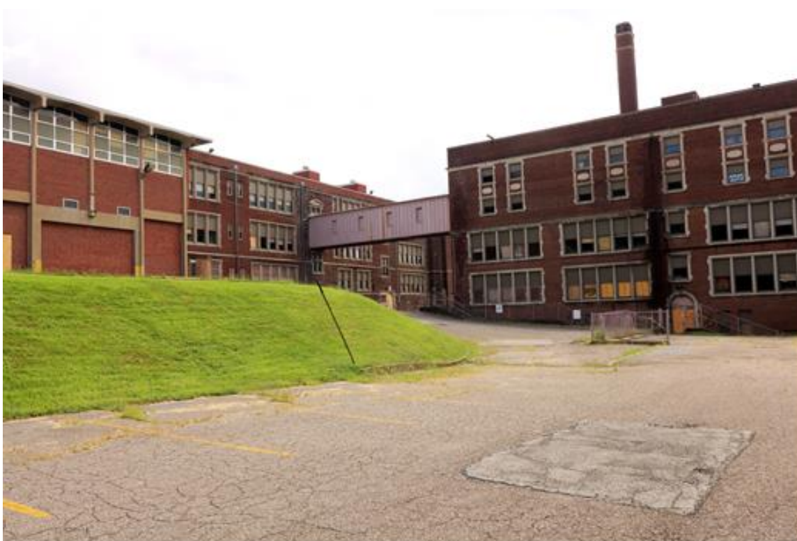
Photo 2: Site View, Looking Southeast from the rear parking lot, showing the 1914-1924 Building (left), 1926 Building (right), and skybridge (center)
