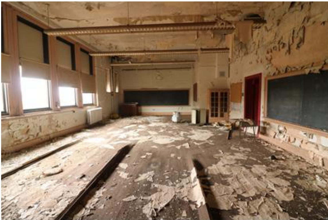
Photo 14: Interior View, 1914 - 1924 Building, First Floor, Classroom, Looking North
