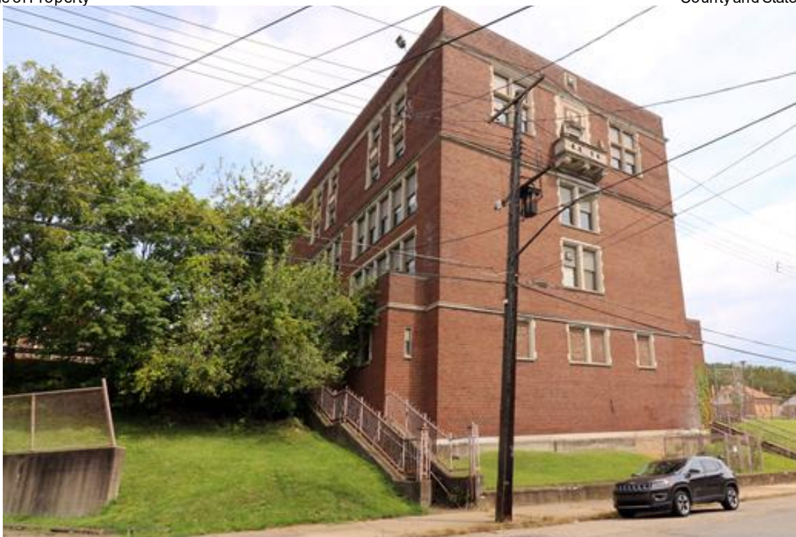
Photo 25: Exterior View, 1926 Building, West Elevation, Looking Southeast
