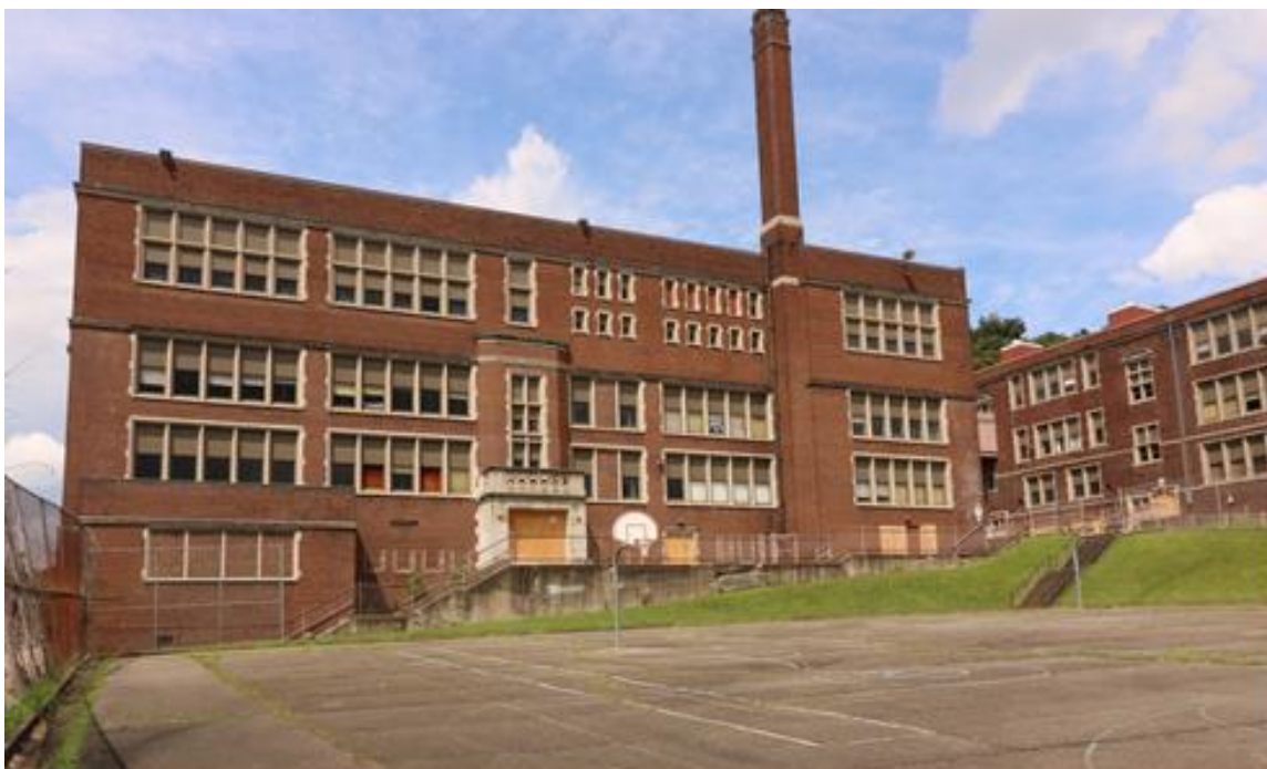
Photo 23: Exterior View, 1926 Building, South Elevation, Looking North
