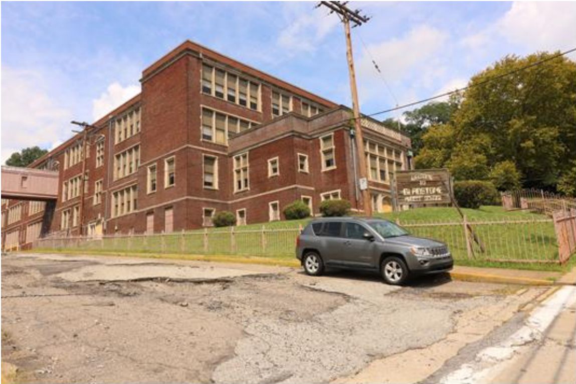
Photo 4: Exterior View, 1914 - 1924 Building, West and South Elevations, Looking Northeast
