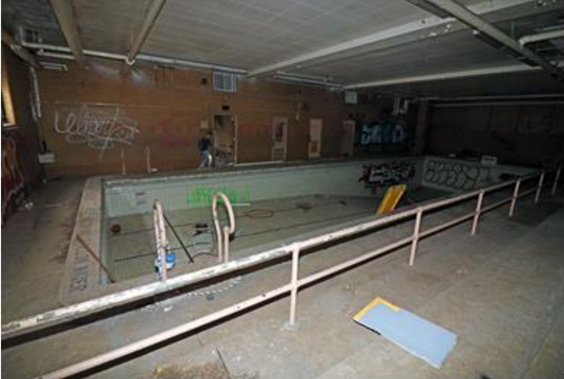
Photo 34: Interior View, 1926 Building, Basement, Pool, looking Southeast
