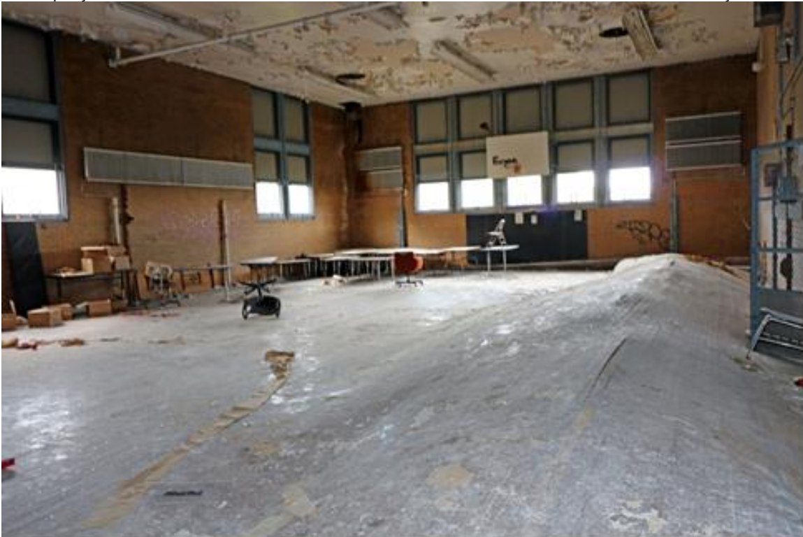
Photo 30: Interior View, 1926 Building, Second Floor, Gymnasium, Looking Southeast.
