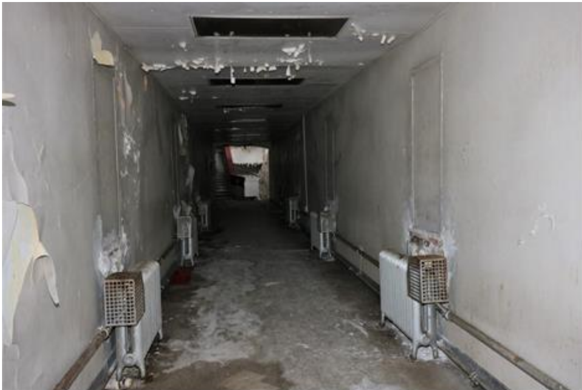
Photo 36: Interior View, Skybridge, looking East.
