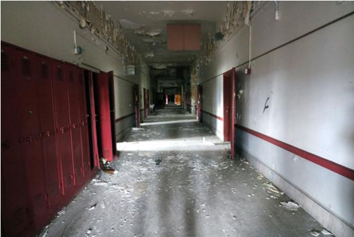
Photo 11: Interior View, 1914 - 1924 Building, First Floor, Hallway at South, Looking North
