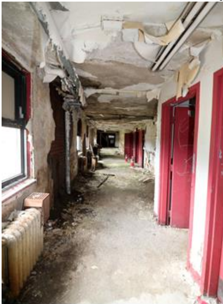
Photo 32: Interior View, 1926 Building, Second Floor Corridor, looking East towards pedestrian bridge
