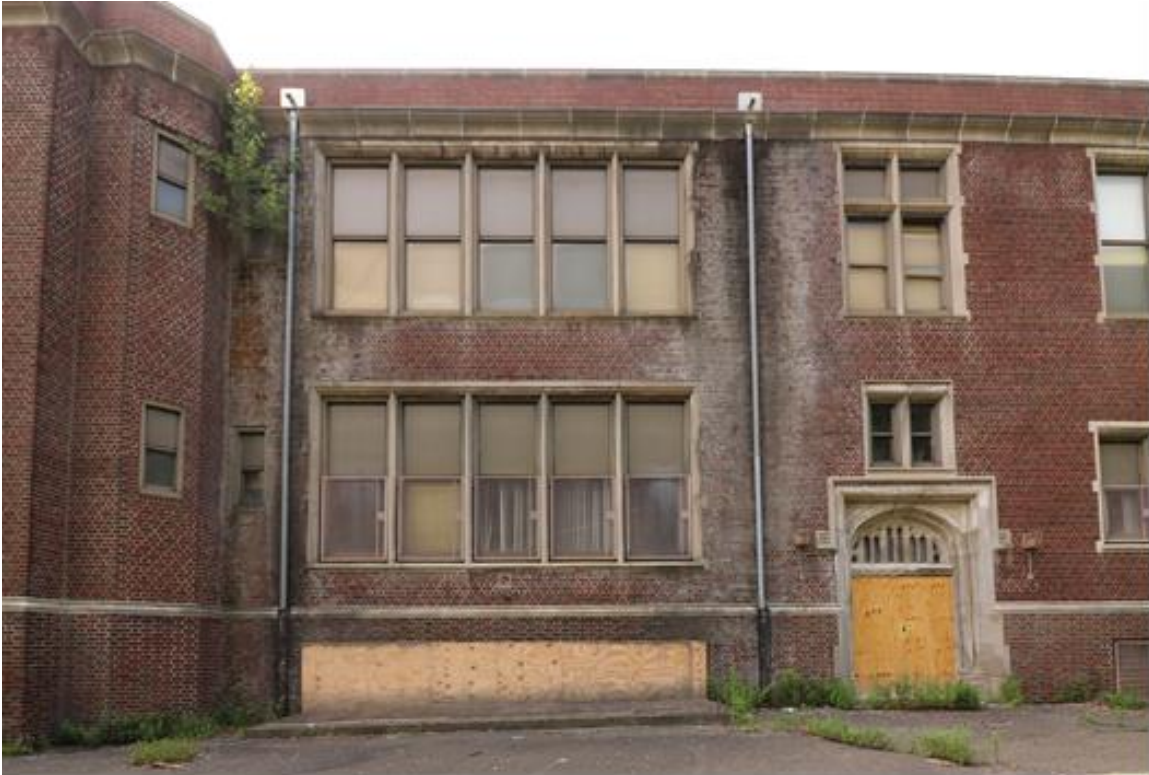
Photo 9: Exterior View, 1914 - 1924 Building, East Elevation, Looking West
