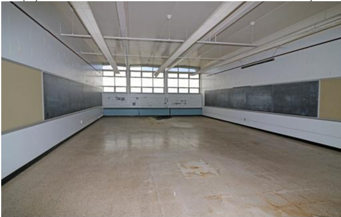
Photo 22: Interior View of a Typical classroom, 1914 - 1924 Building, 1965 Non-Contributing Addition, First Floor, Classroom, Looking West
