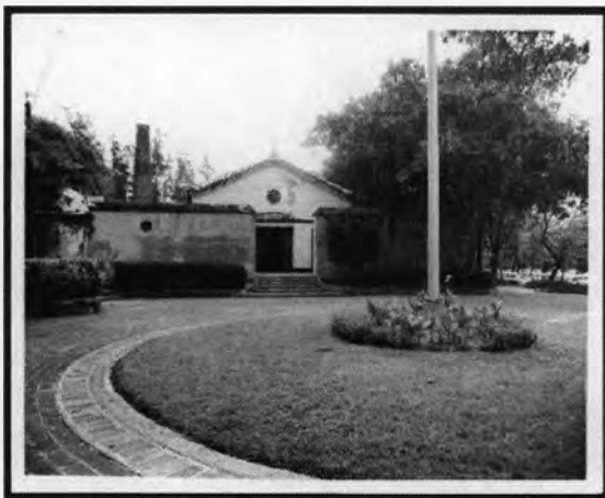
Fig. 7 Entrance to San Geronimo Powderhouse, 1967 9 .
