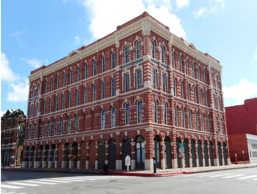
Photo 19 The Kauffman and Runge Building at 220 22 nd Street, looking northeast.
