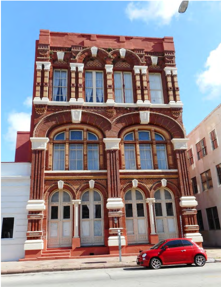
Photo 18 The Galveston News Building at 2110 Mechanic, looking north.
