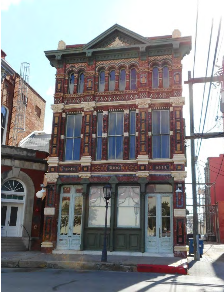
Photo 20 The Truheart and Company Building at 212 22 nd Street, looking east.
