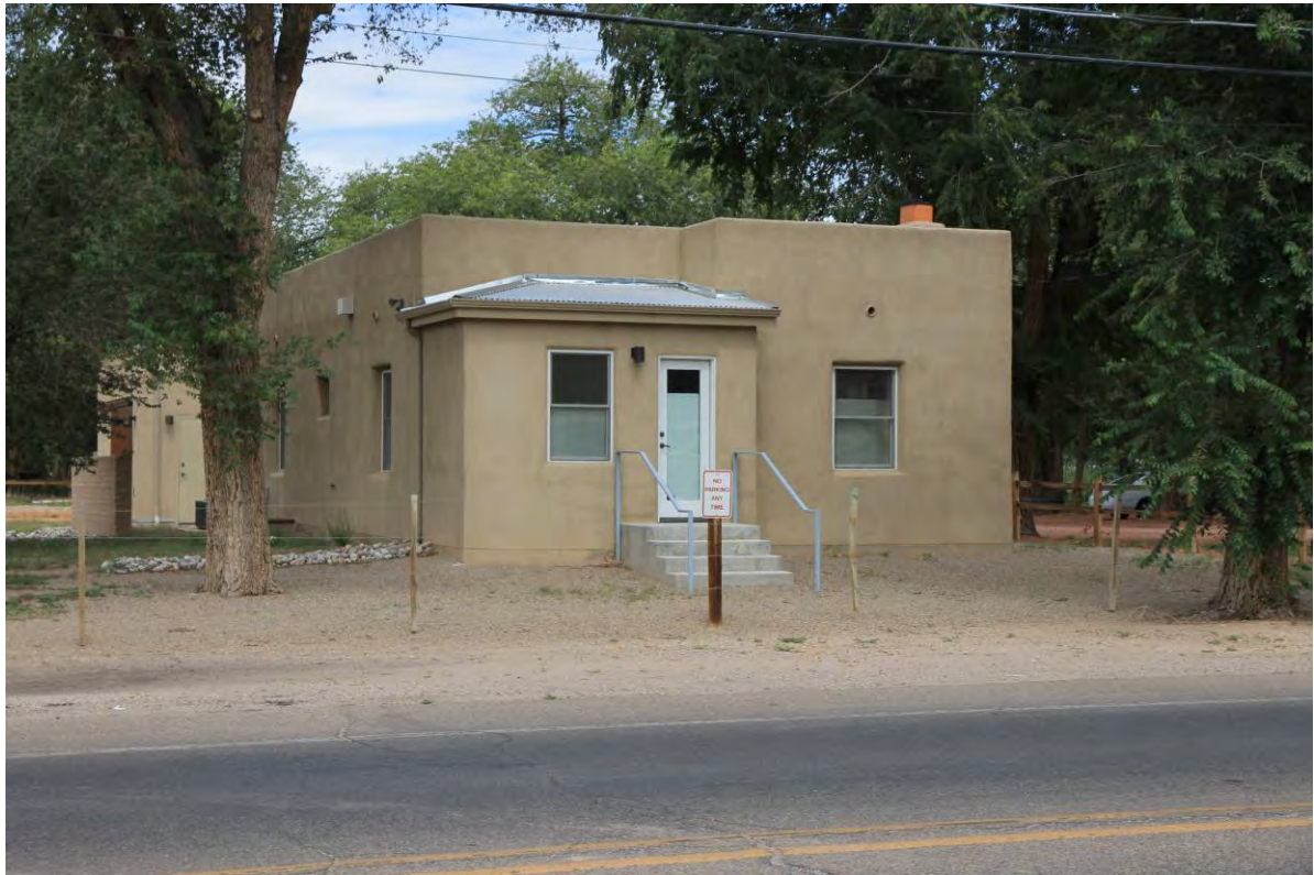
23 of 27. Casita, main (west) and south facades, photographer facing northwest.
