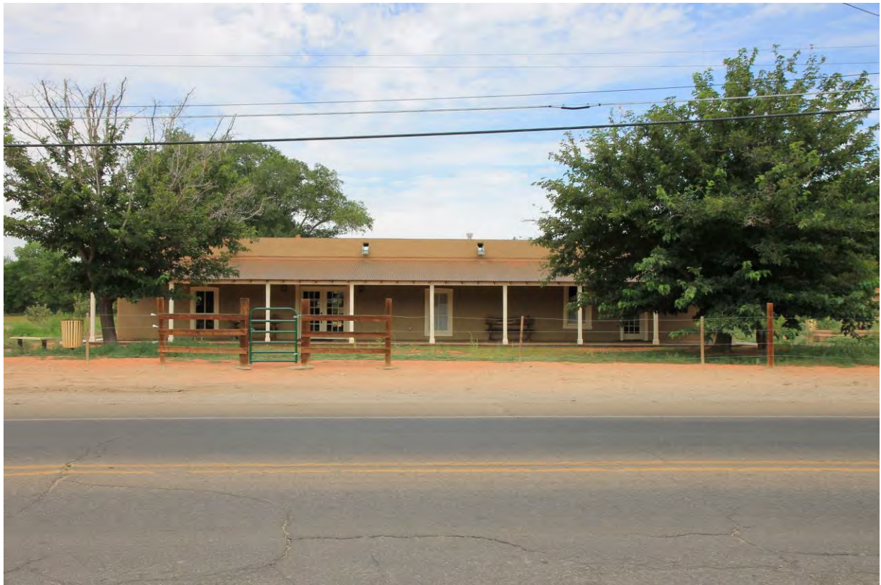
1 of 27. Main house, main (east) façade, photographer facing west.
