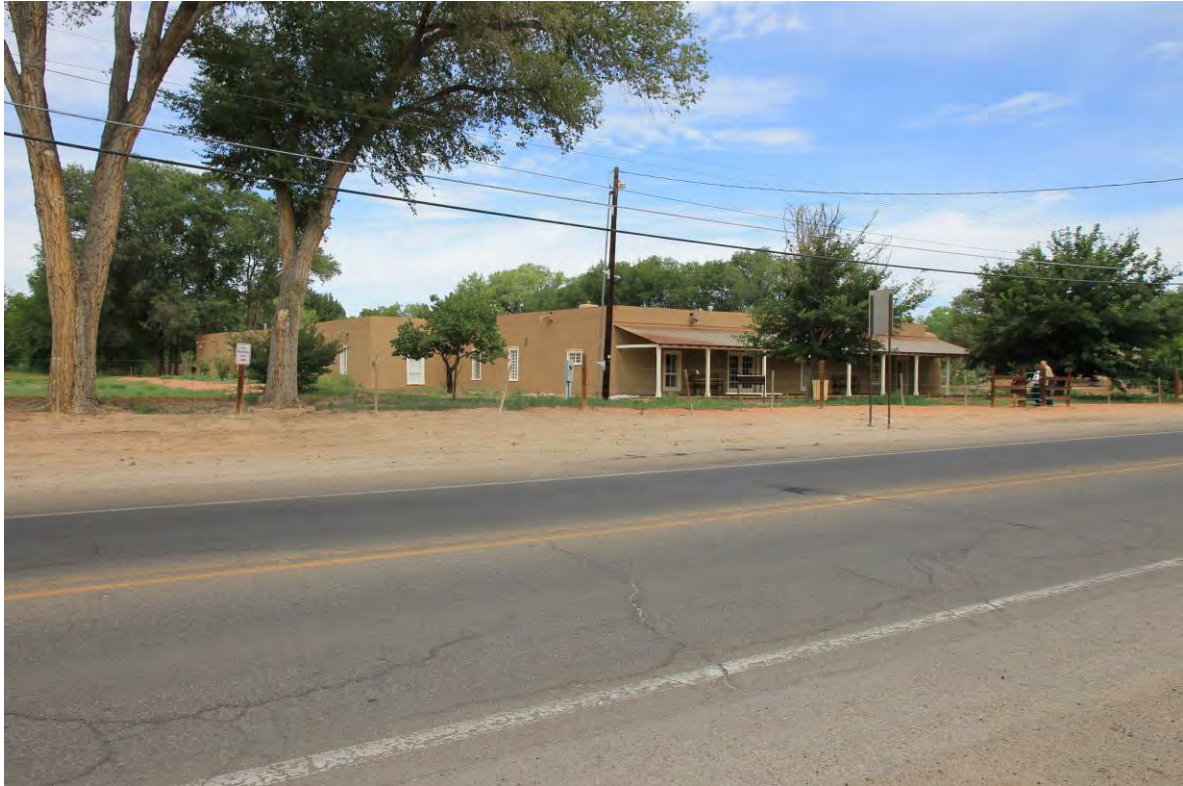
3 of 27. Main house, main and south facades, photographer facing northwest.
