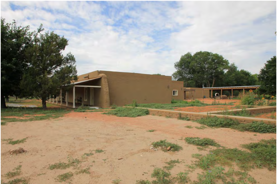
8 of 27. Main house, main and north facades with site of mercantile (right), photographer is facing southwest.
