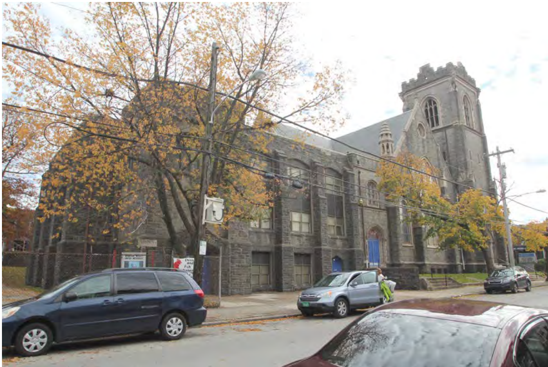
Photograph 4 – North and west elevations, view southeast
