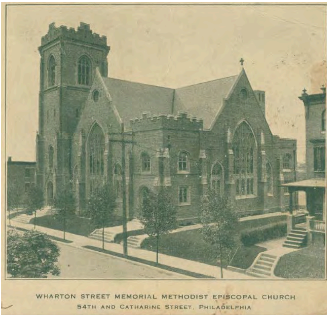
Figure 2 – 1911, Wharton Street Memorial Methodist Episcopal Church.
