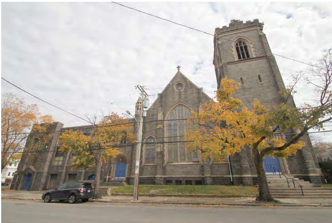
Photograph 2 – West elevation, view east
