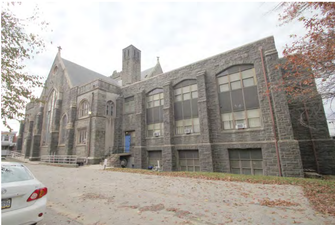
Photograph 6 – East elevation, view southwest
