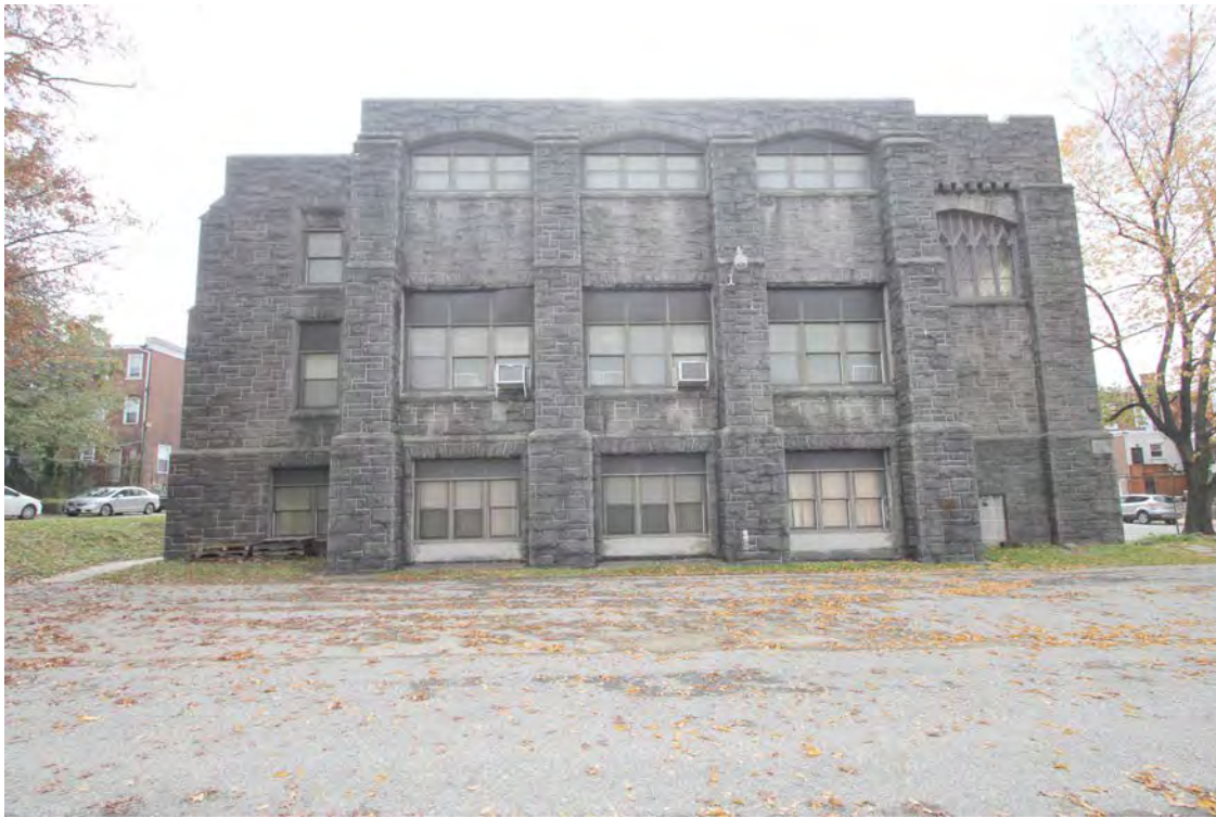
Photograph 5 – North elevation, view south
