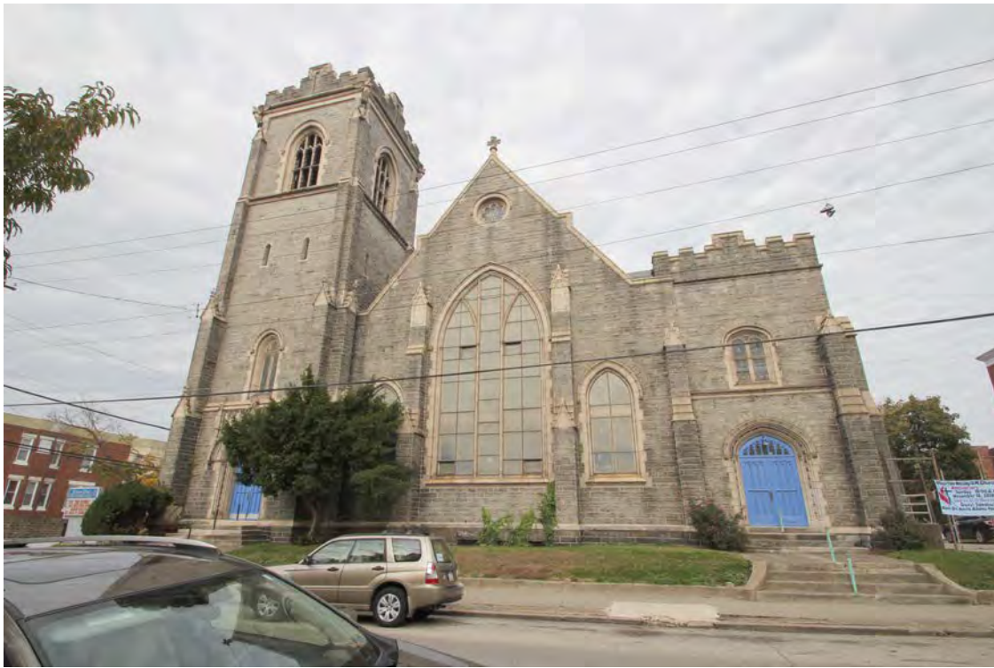
Photograph 1 – South elevation, view northwest
