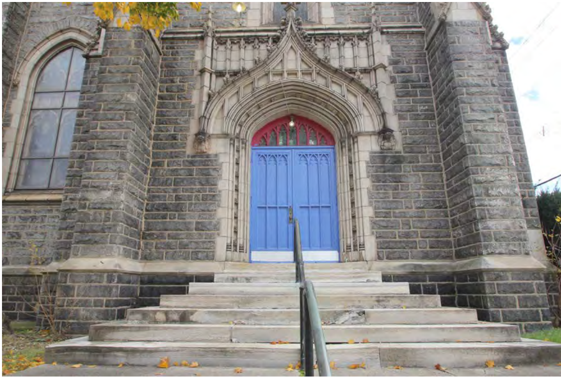
Photograph 3 – West elevation, Entrance, view east
