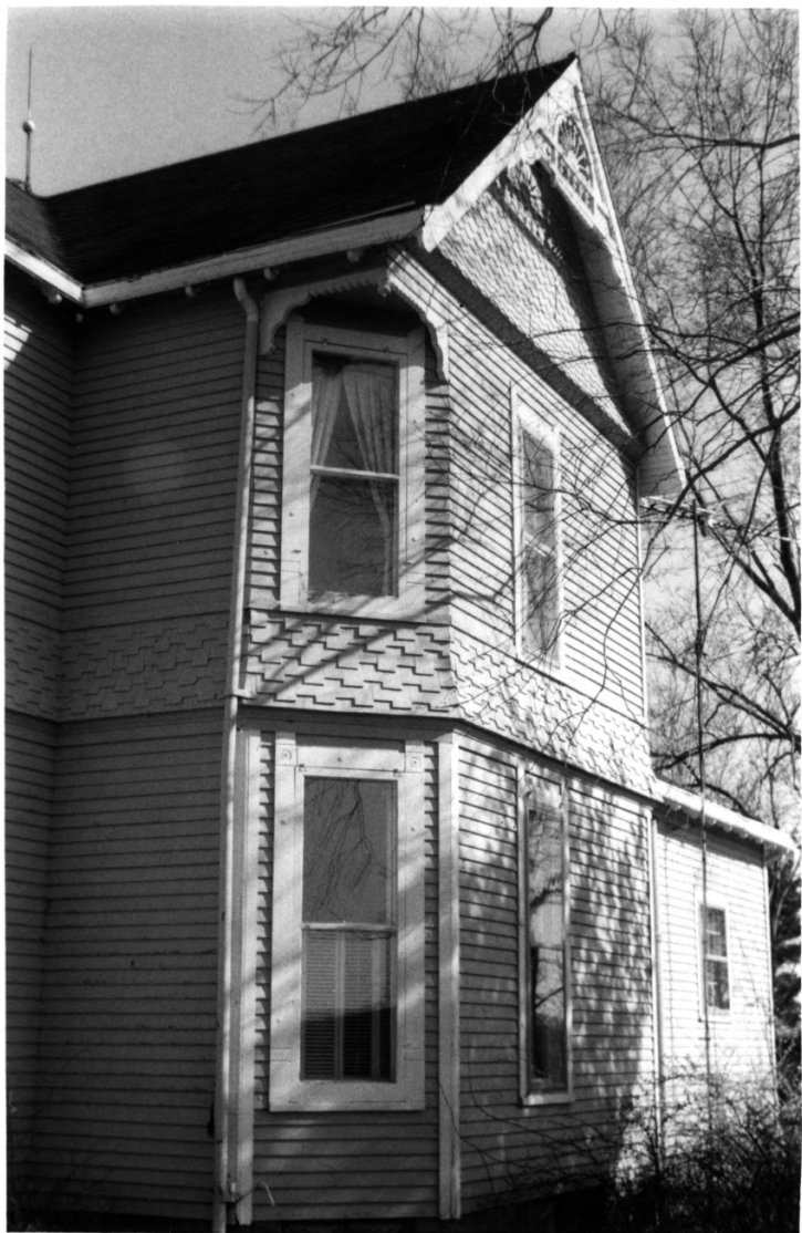
HEBLER, CLINTON F., HOUSE FOUNTAIN COUNTY, IN PHOTO # 13
