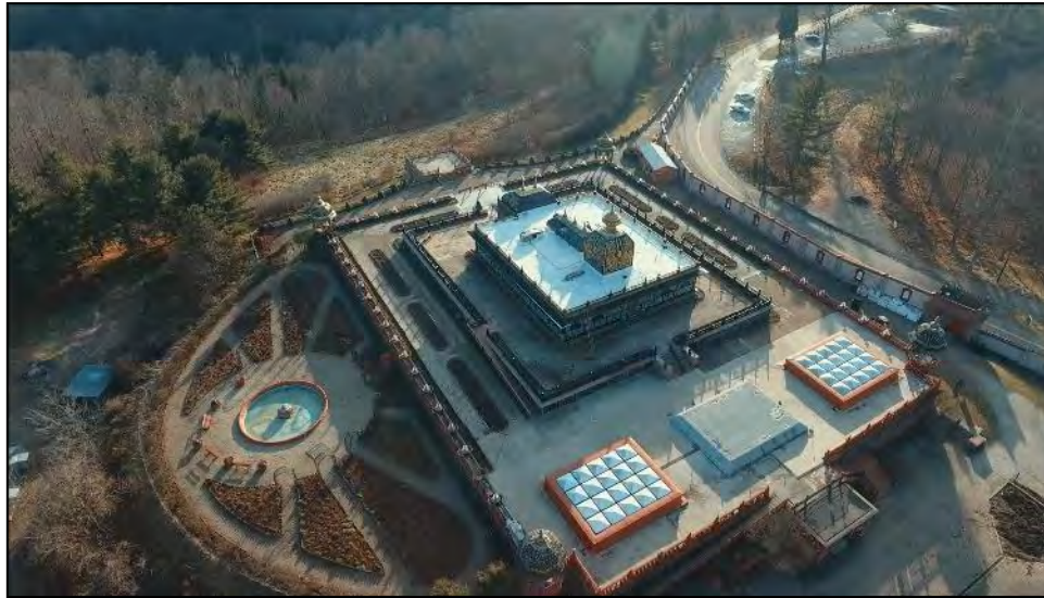
Photo 3. Aerial overview, facing southwest
