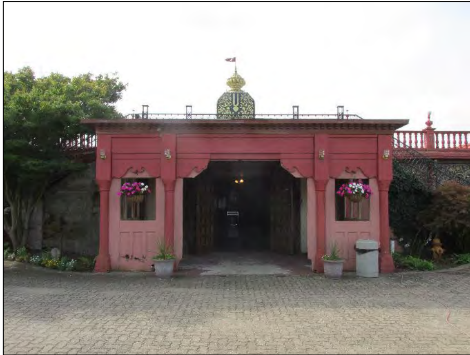
Photo 13. Entrance to basement level, facing south
