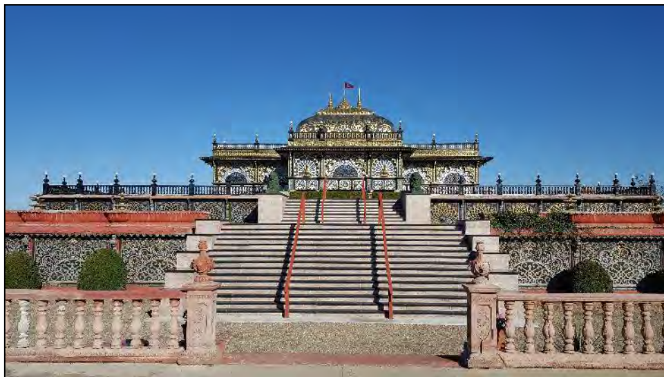
Photo 14. South elevation, facing north
