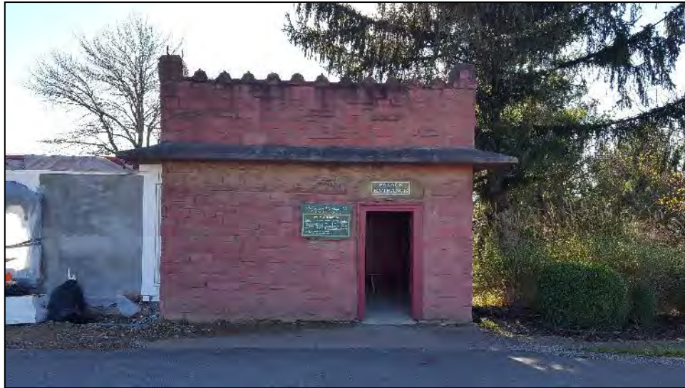
Photo 29. West elevation, southern guardhouse, facing west
