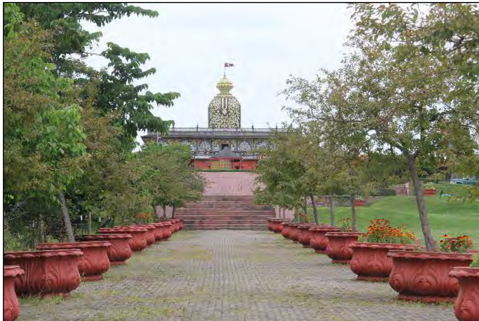
Photo 7. North elevation of palace, facing south
