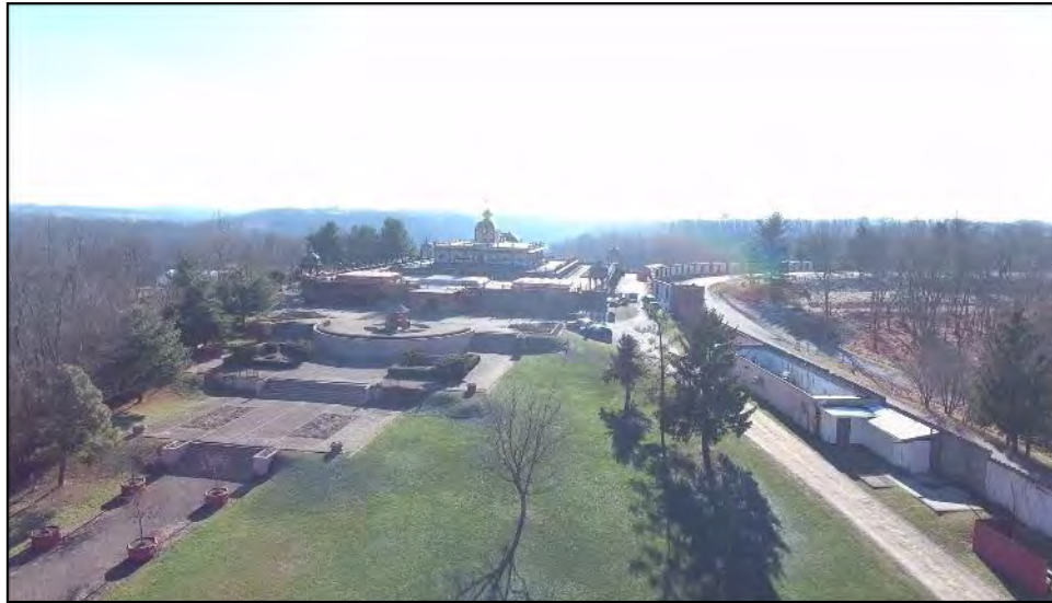
Photo 1. Aerial overview, facing south
