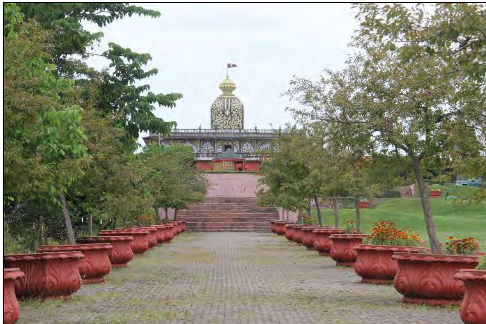
Photo 7. North elevation of palace, facing south
