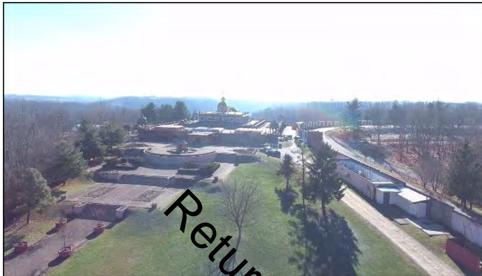
Photo 1. Aerial overview, facing south
