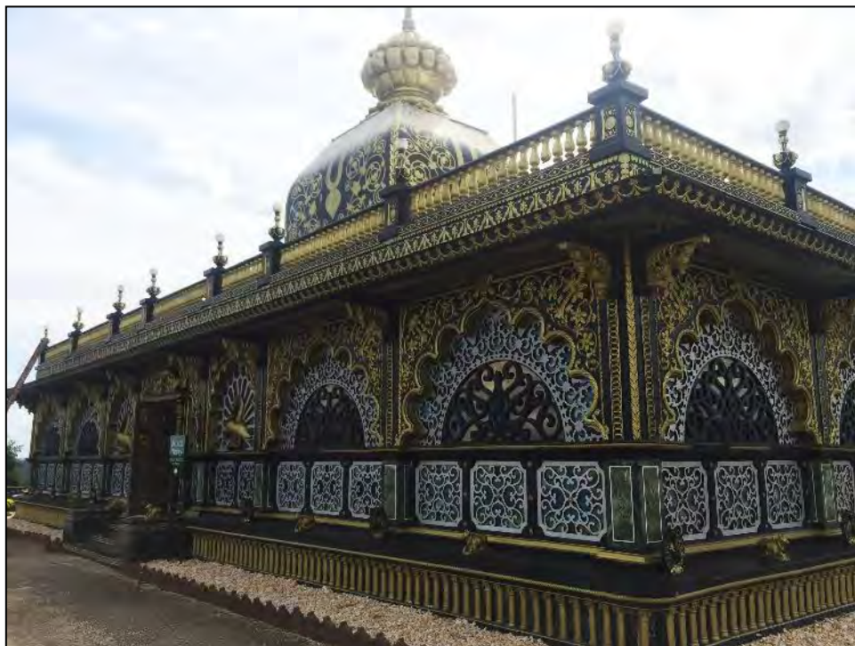
Photo 16. Detail of south elevation, facing southeast
