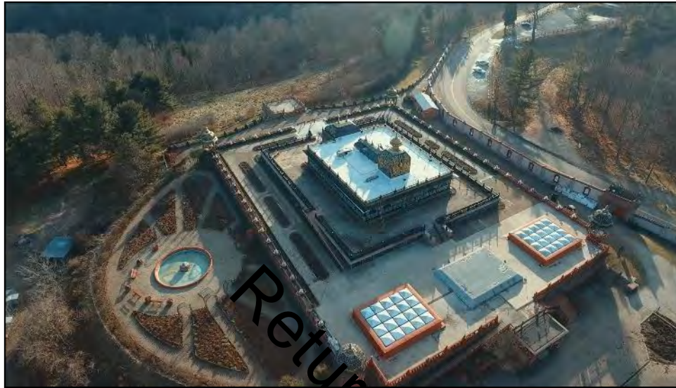
Photo 3. Aerial overview, facing southwest
