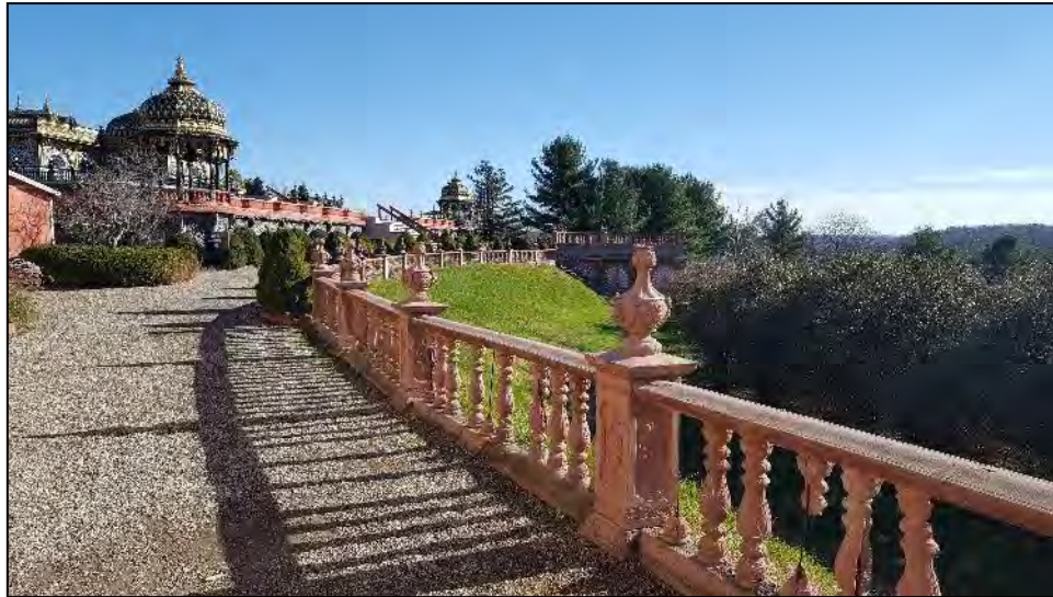
Photo 31. Overview of south wall, facing northeast
