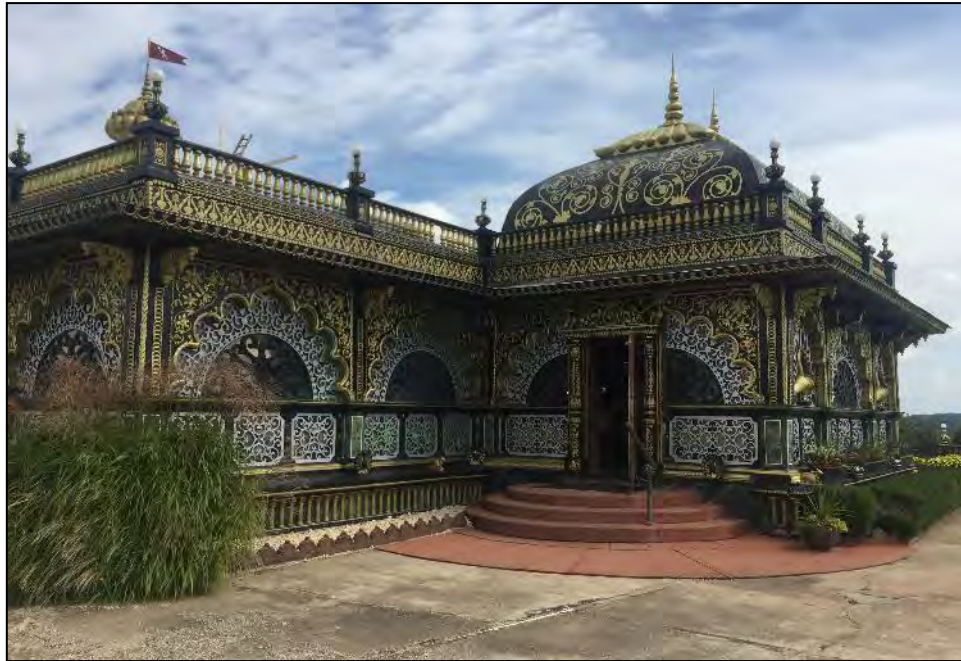
Photo 15. Entry door on west side of entry hall, facing northeast
