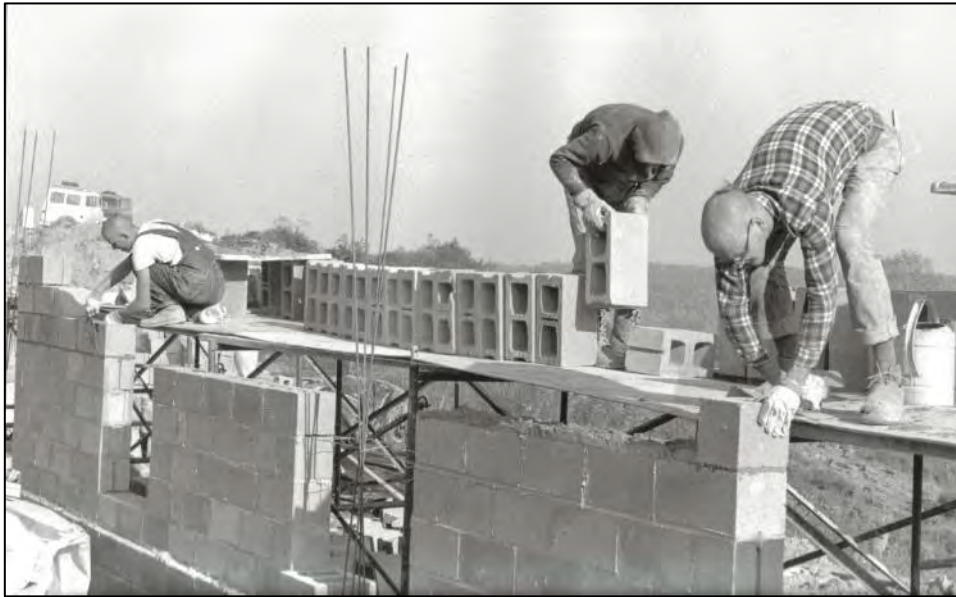
Figure 5. Hare Krishna devotees construct the west wall, c. 1978. Image courtesy ISKCON.
