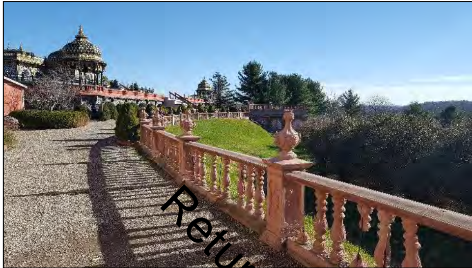
Photo 31. Overview of south wall, facing northeast
