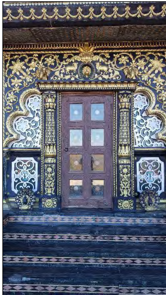
Photo 32. Detail of exterior door on north elevation
