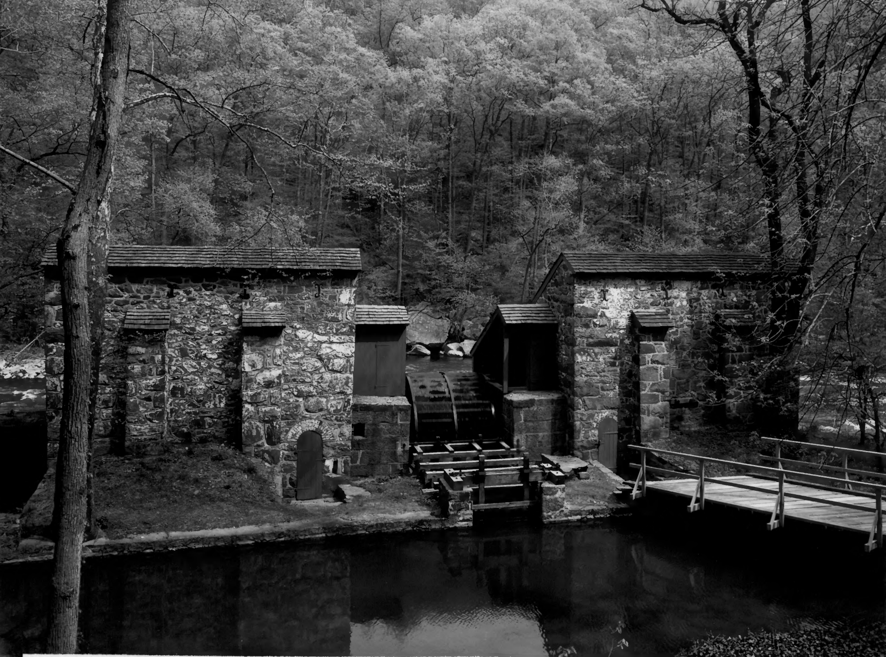
S-24. Birkenhead Mills - Drawn and photographed by HABS during the Depression. Waterwheel restored 1966 and rebuilt 1983. Race M-2 in foreground. The bridge is an insignificant modern addition near the site of an original lattice truss bridge.
