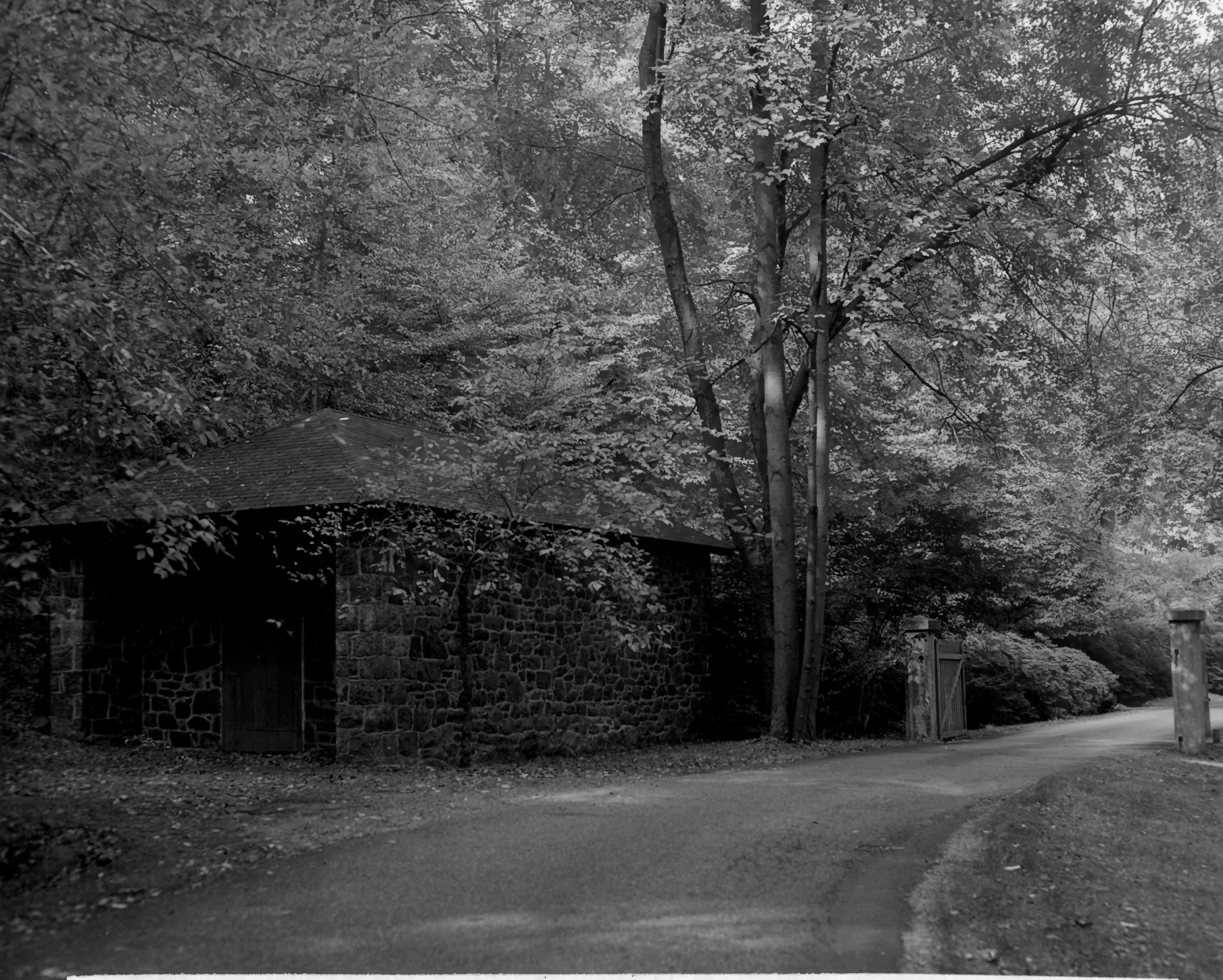
S-27. Rebel Shanty - Original walls dating from before the Civil War. The roof is an old (20th century) improper replacement. Gates to right are post-yard closing.
