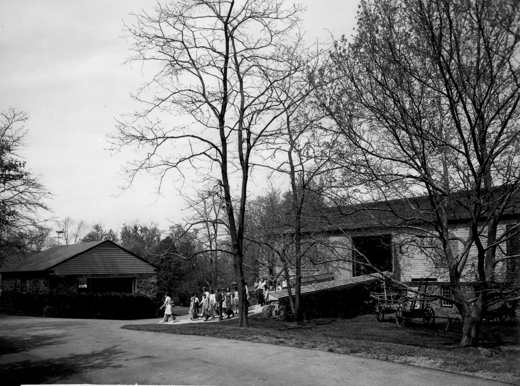
S-37. & S-38. Barn and Carriage House - The barn is virtually identical to its appearance in the sketches and late 19th century photographs. The carriage house was part of a three-building complex and originally had a second story which burned about 50 years ago.
