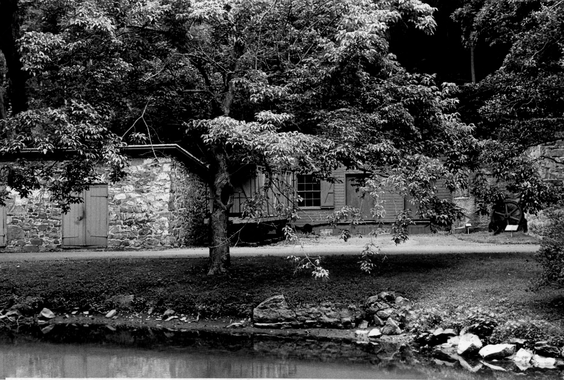
S-18,S-19,S- 20. Press House (S-19) contains original powder press. Railroad car slated for moving in 1984. It was built by American Car & Foundry in Wilmington and is like magazine cars pictured on the property. This particular car came from Carney's Point.
