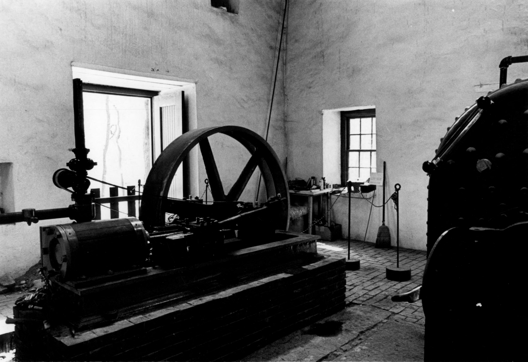
S-25 Engine House interior restoration with antique boxbed slide valve engine. Engine is run daily for visitors.
