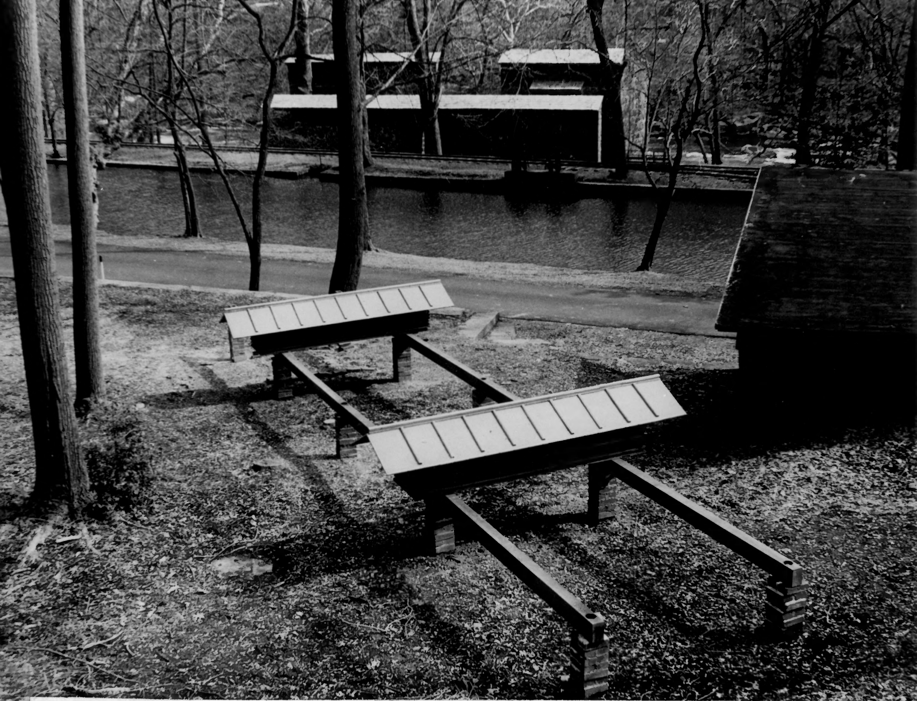
R-12, R-14, S-20. Restored drytable (one of 10 on site). Wheel mills #3 and 4 in background. Bucket house at right. Race (part of M-2) runs through the center.
