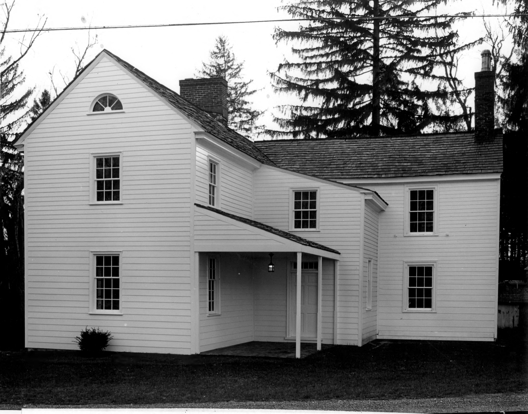
S-15. Belin House - Photo taken in 1974 during renovations. House now has shutters and is painted yellow to conform to the original color.
