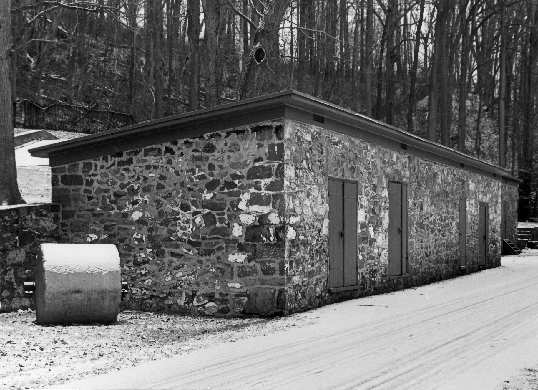
S-18. Store House - S-20. Bucket House at right. Large stone object at left is original road roller minus its wood box frame.
