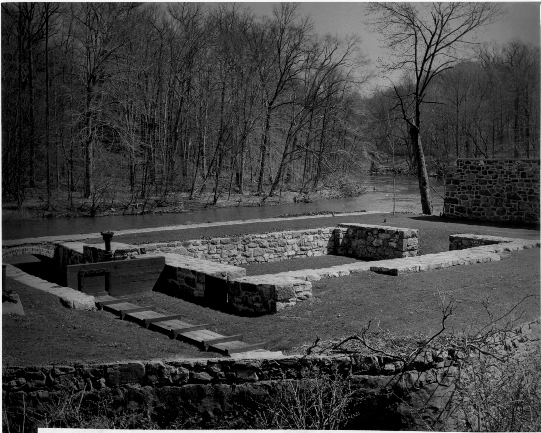
R-18. Dust Mill foundations and original 1860 vintage Tyler scroll case turbine. Race (M-3) in foreground.
