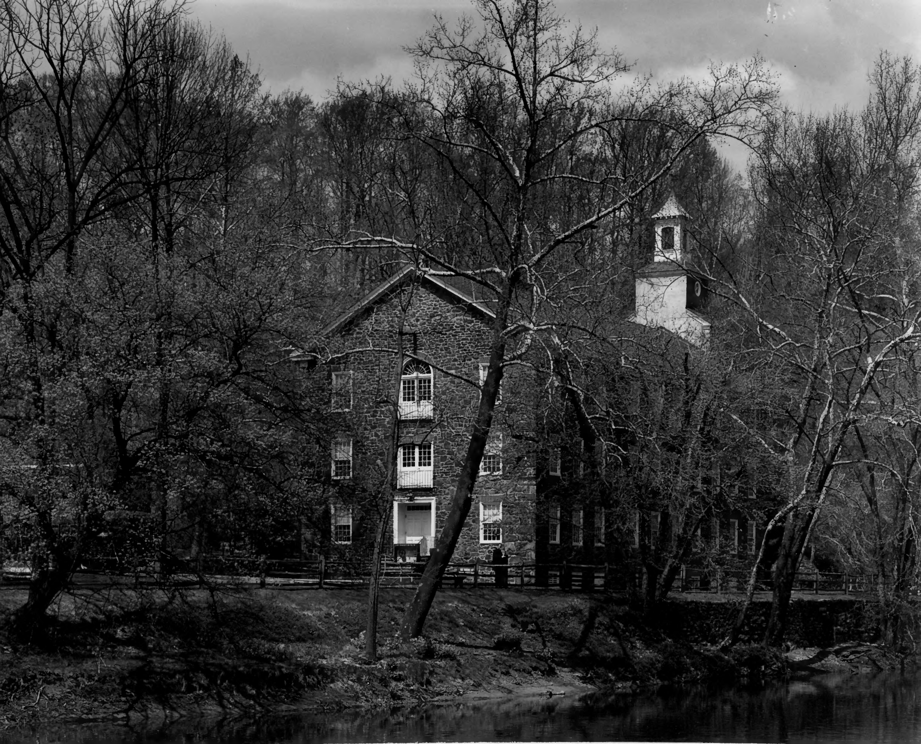
S-3. Henry Clay Factory - Now Museum's Main Exhibit Building.
