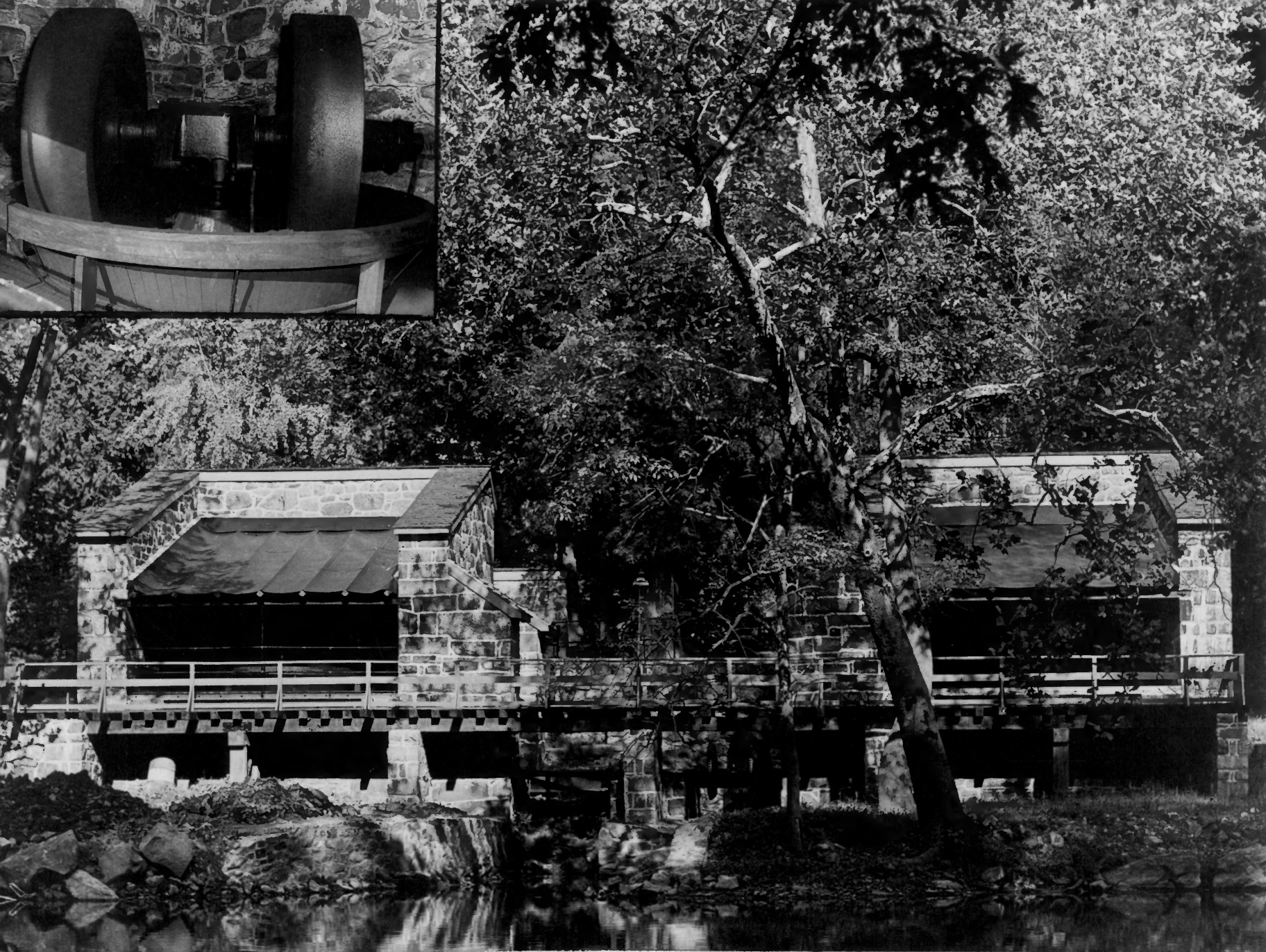
S-7. Restored Wheel Mills - Inset shows pair of 8-ton wheels. Mill is operated daily for visitors powered by a water turbine.
