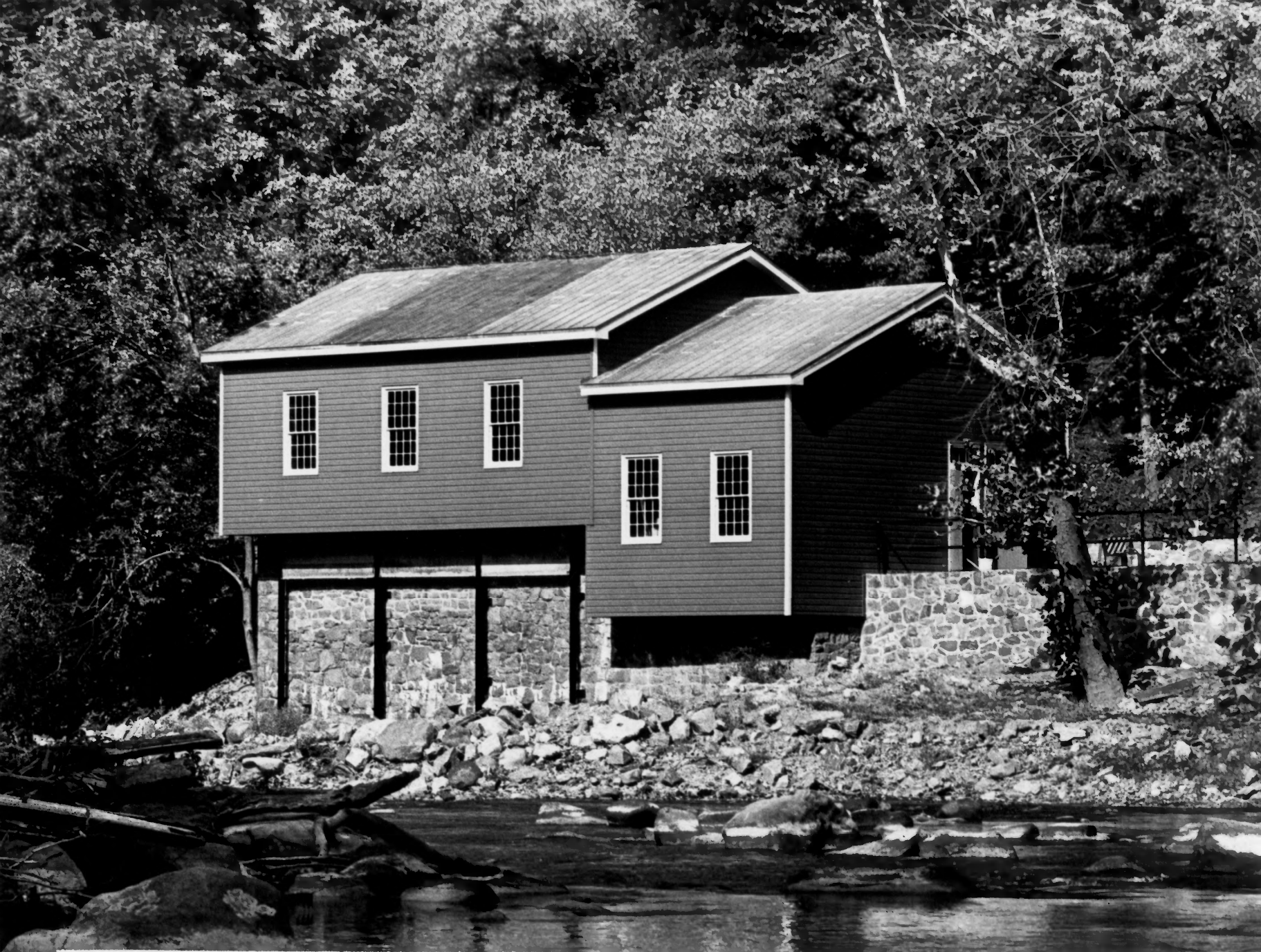
S-4. New Century Hydro Plant - Foundations original, building 1976 replica scaled from original photographs. This hydroplant produces power for the Foundation property. Depending on the season and time of day, additional power is bought from Delmarva Power and Light or surplus power is sold to them.
