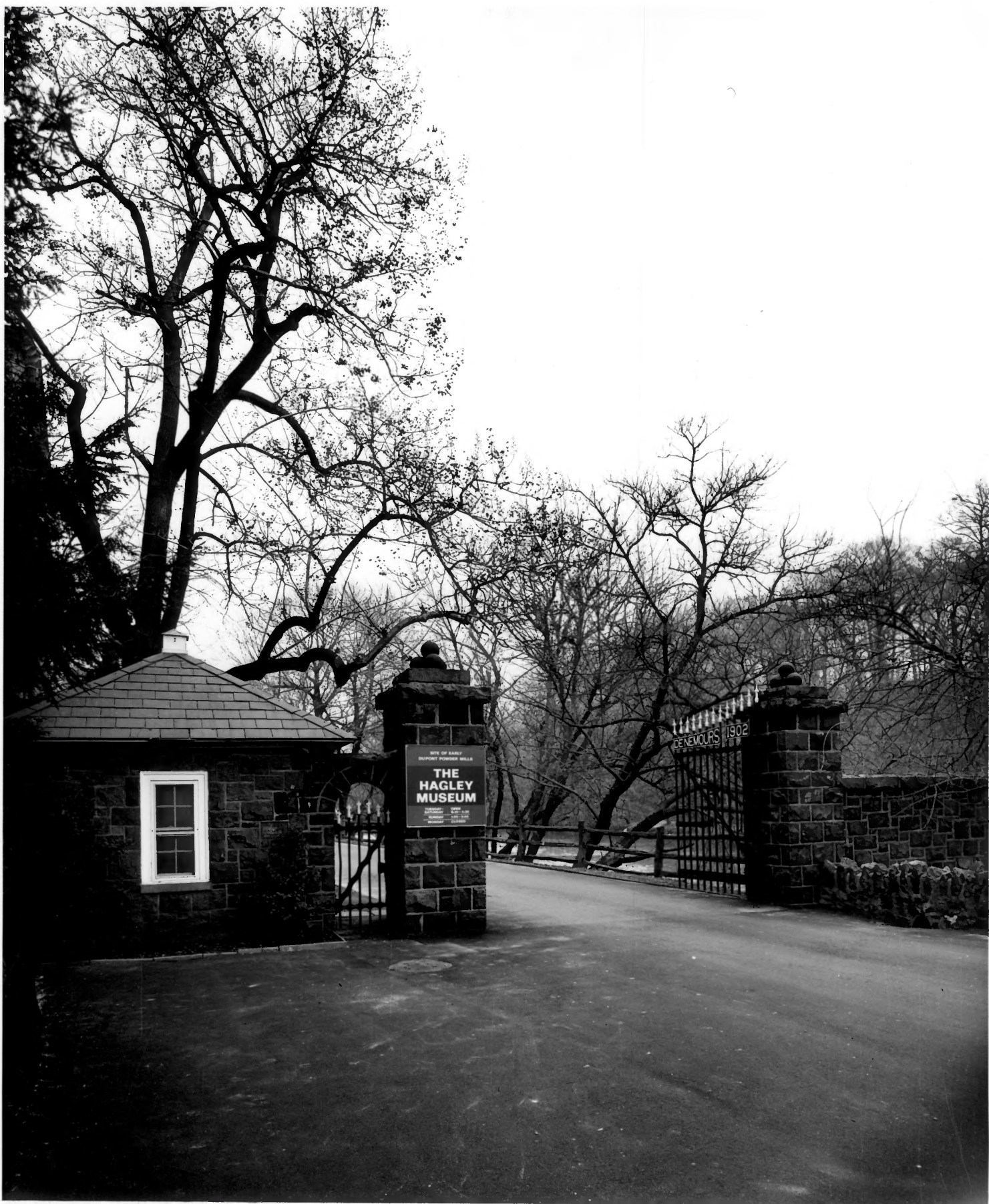
S-1. Gates and Gate House - The access gates moved as the yard expanded. This is the final location. The stone work is original; the gates have been restored twice, but retain some of the original fabric. Original construction drawings in Hagley Museum files.
