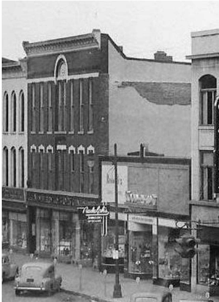
Detail, previous image. Note the undulating storefronts, typical of 1930s-era retail designs.
