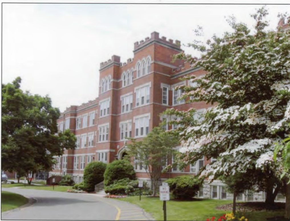
Photo 0008: Exterior view of Mercy Hall (Administration), east and north elevations
