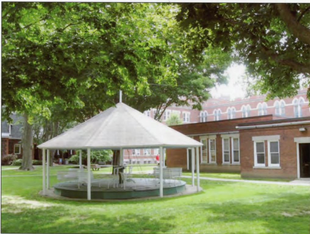
Photo 0014: Exterior view of the Taylor Carousel with the Boiler Room at right (north and west elevations) and Mercy Hall and Chapel in the background (west and north rear elevations)
