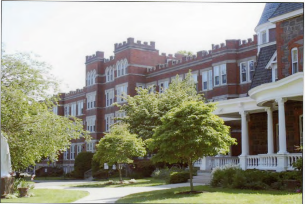
Photo 0007: Exterior view of Mercy Hall (Administration) and adjacent Lauralton Hall (Mansion), east and north elevations
