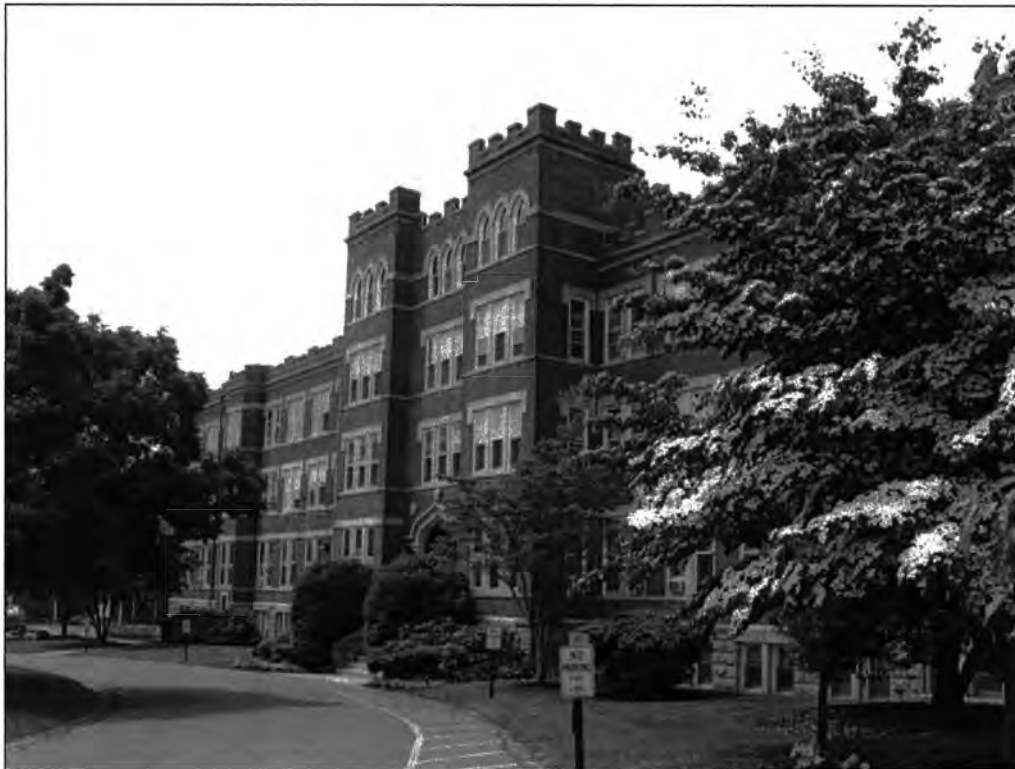
Photo 0008: Exterior view of Mercy Hall (Administration), east and north elevations
