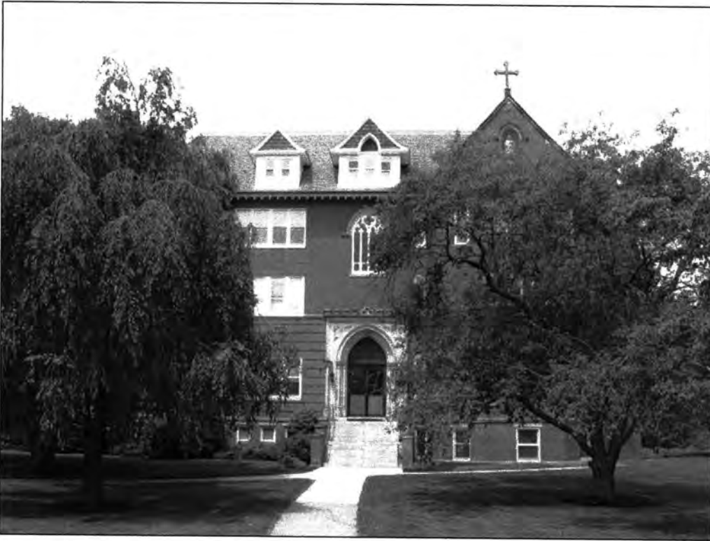
Photo 0005: Exterior view of St. Joseph Hall, east elevation
