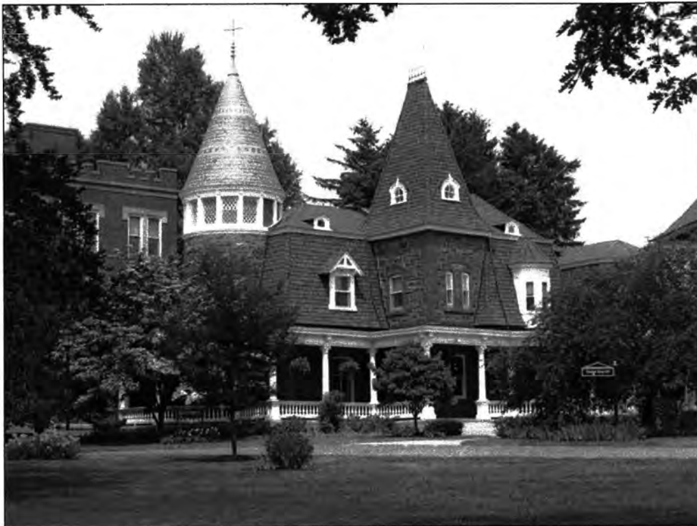
Photo 0004: Exterior view of Luralton Hall (Mansion), south and east elevations
