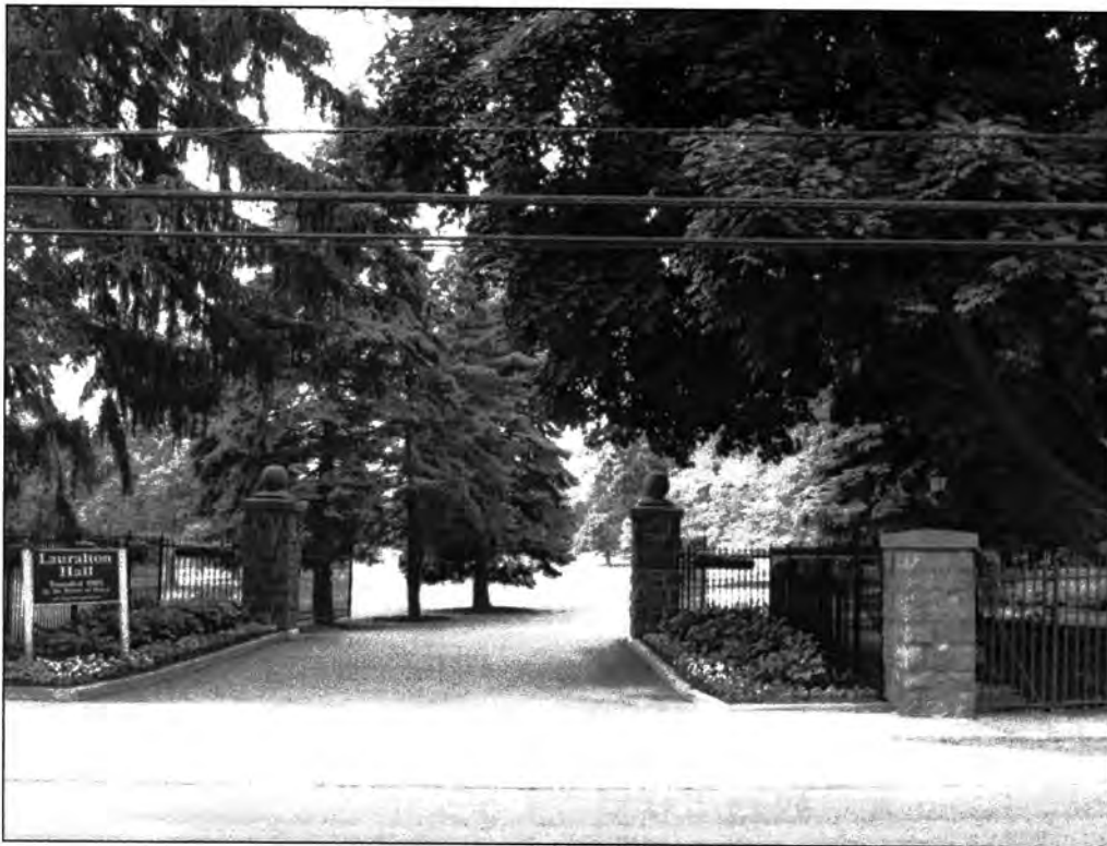
Photo 0001: Entrance to the Academy of Our Lady of Mercy / Luralton Hall, 200 High St., Milford, CT – view looking west from High St.
