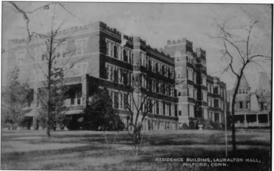
Historic View I: View of Mercy Hall, south and east elevations, c. 1920
