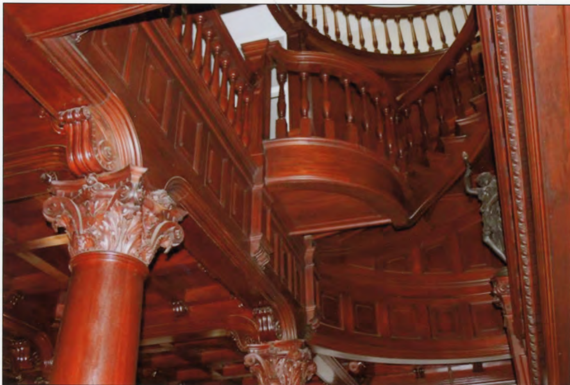
Photo 0018: Interior view of the Grand Staircase at Lauralton Hall, looking up from the 1 st landing
