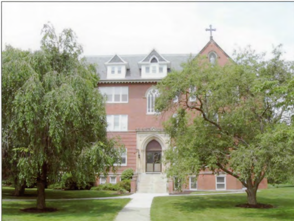
Photo 0005: Exterior view of St. Joseph Hall, east elevation
