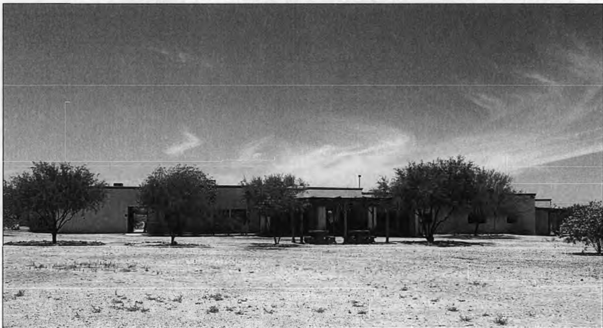
Figure 14. Robles Ranch House, north facade, view to south, June 9, 2010.
