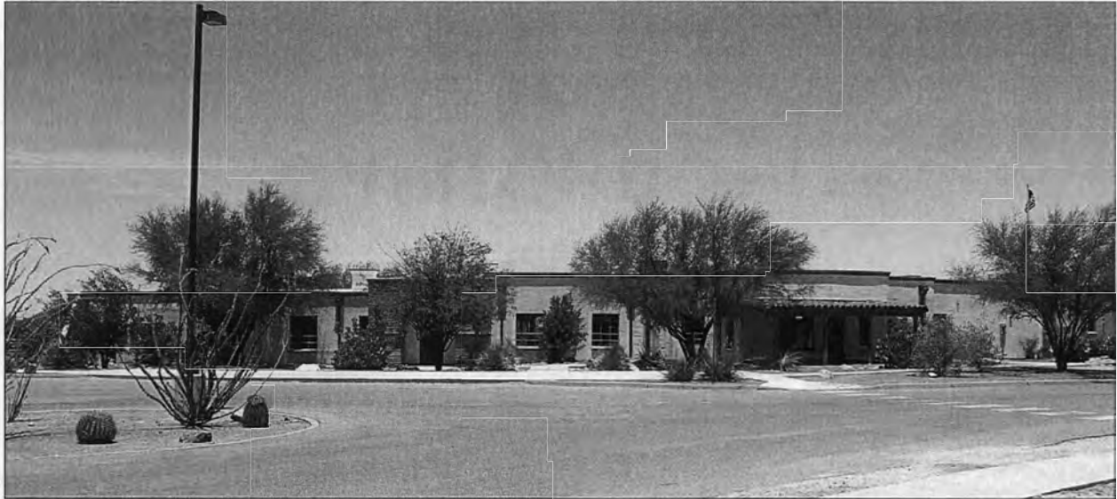
Figure 13. Robles Ranch House, south facade, view to north, June 9, 2010.
