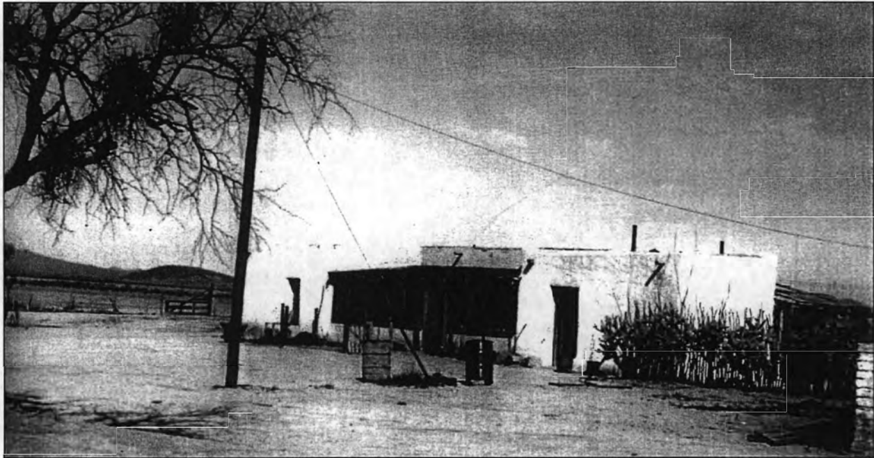
Figure 11. West house, view to northwest, ca. 1943 (Doyle and Associates 1999:Figure 3).
