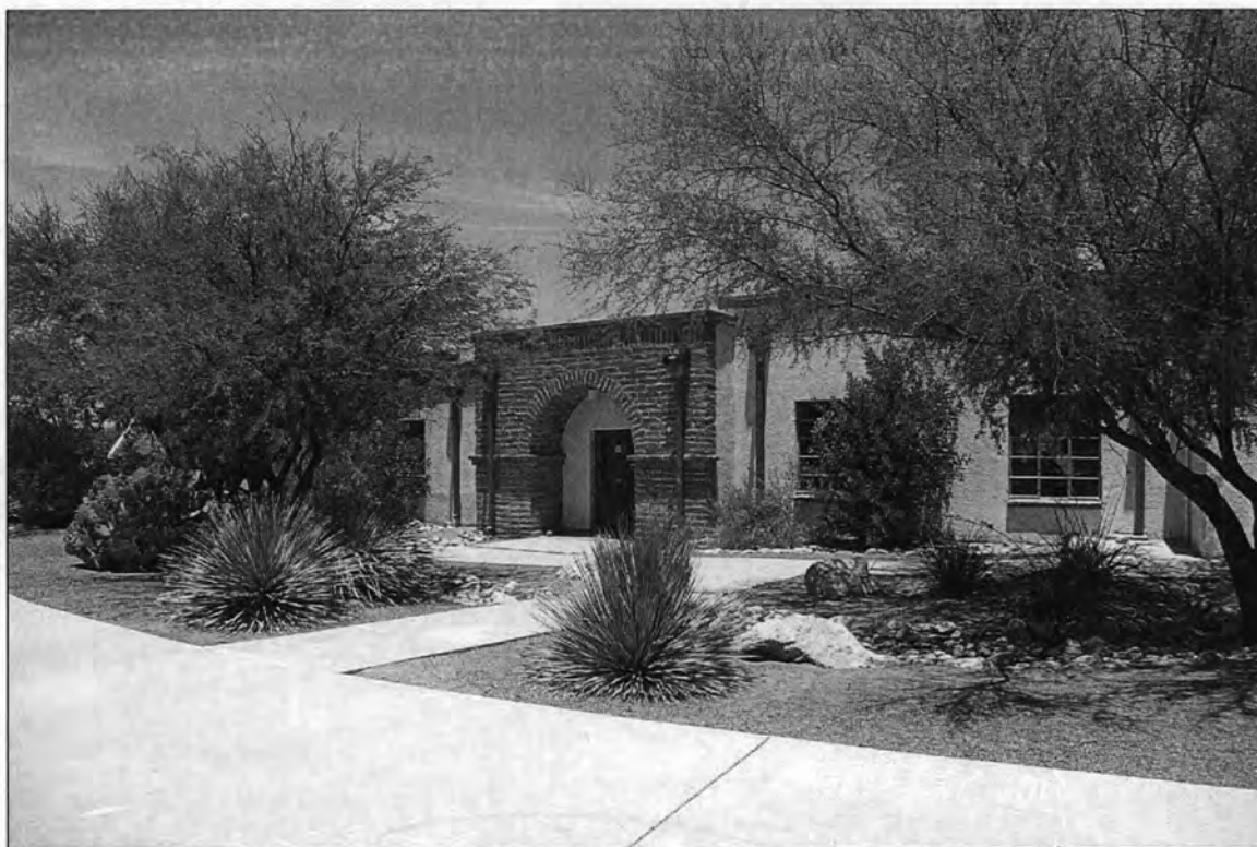
Figure 15. Detail of entry, south facade, view to north-northwest, June 9, 2010.
