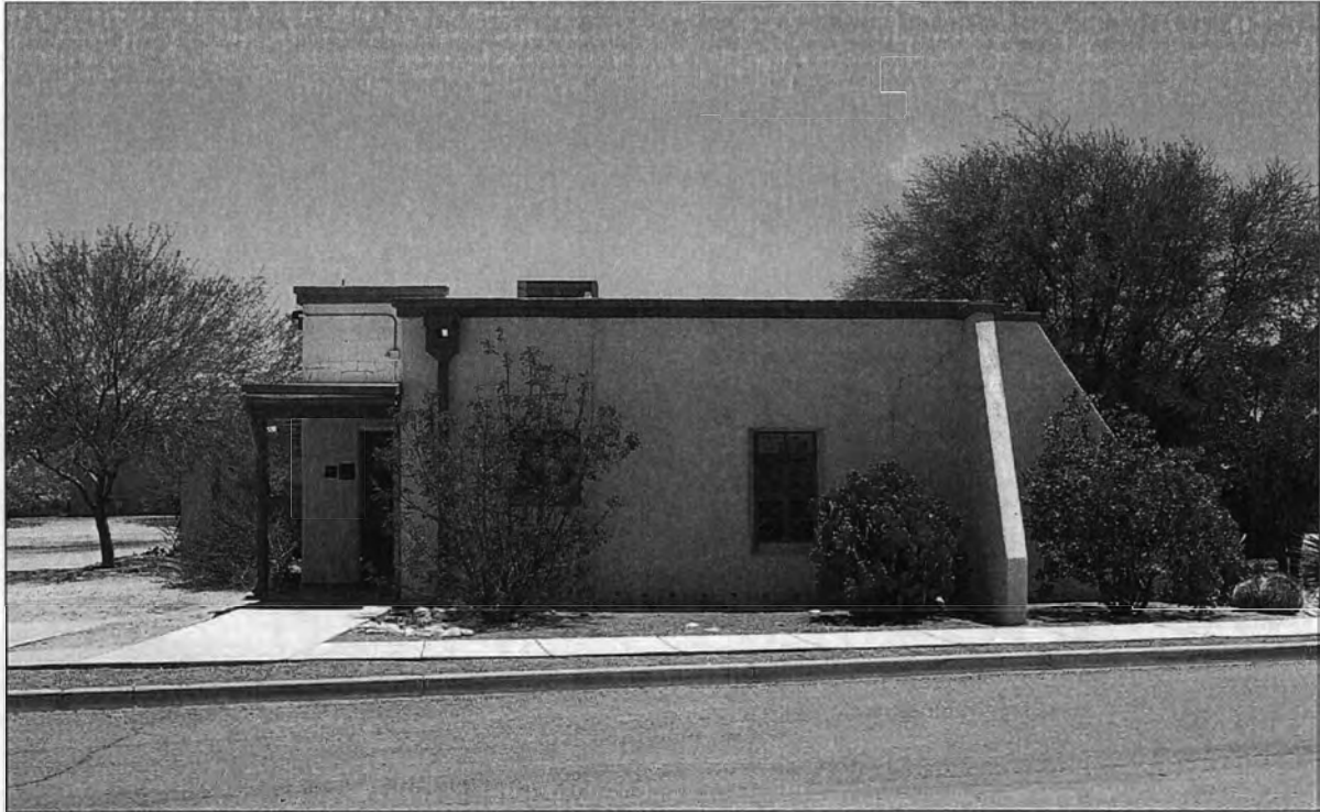
Figure 17. Robles Ranch House, west facade showing corner buttresses, view to east, June 9, 2010.
