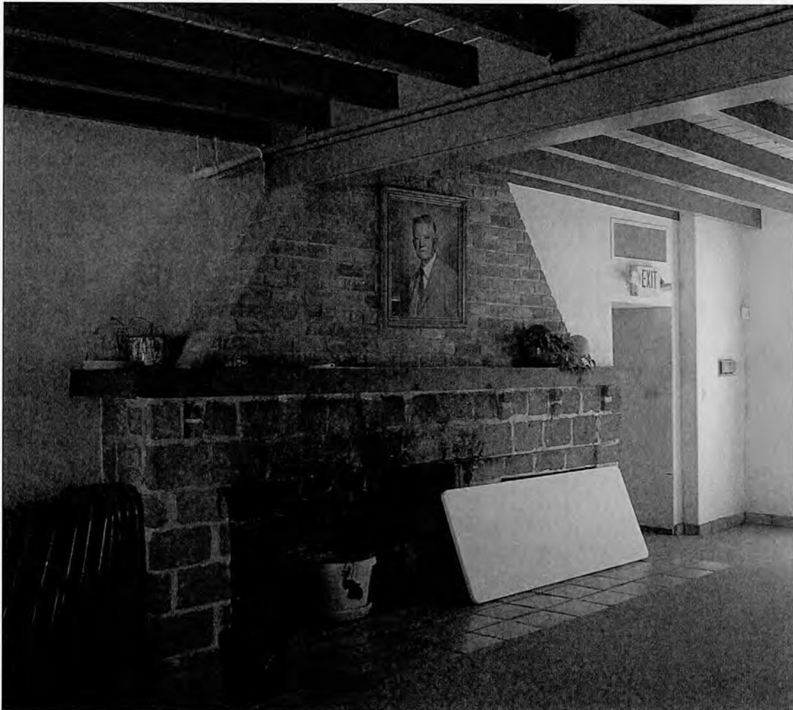
Figure 21. Detail, east wall, Meeting Room, showing fireplace, June 9, 2010.
