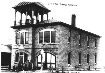
FIGURE 4: Tigerton Village Hall and Engine House Tigerton, Shawano County, Wisconsin Early View
