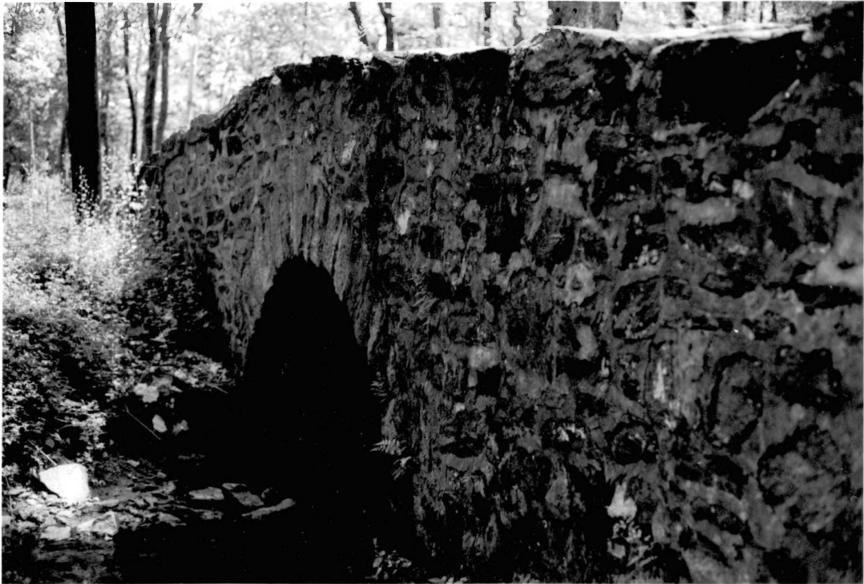
FROG HOLLOW ROAD BRIDGE, TEWKSBURY TWP., HUNTERDON CO. PHOTO 4 of 5
