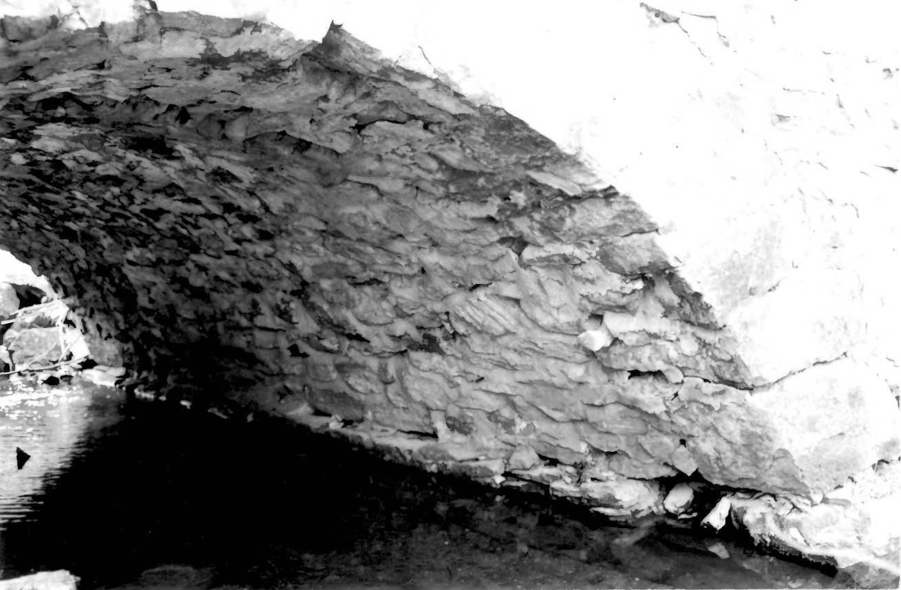
FROG HOLLOW ROAD BRIDGE, TEWKSBURY TWP., HUNTERDON CO.
