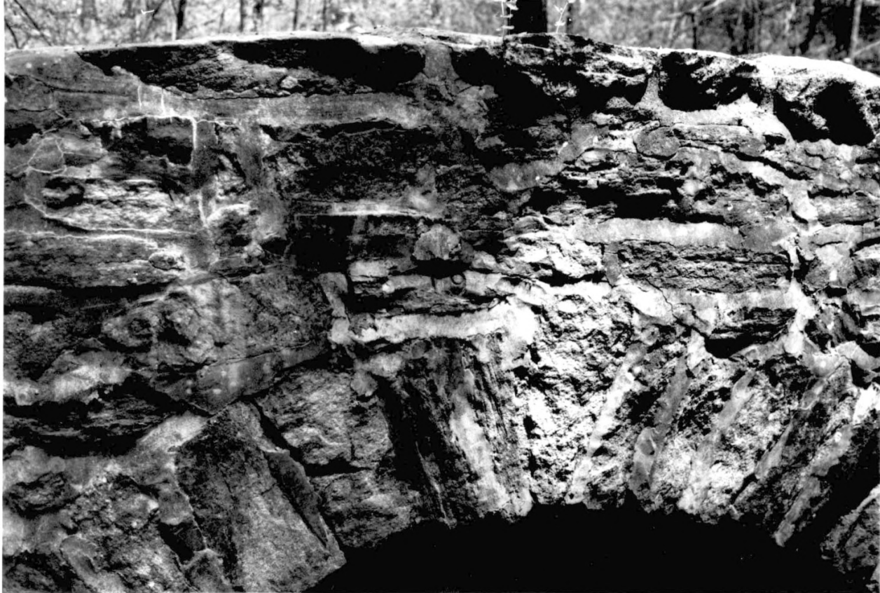
FROG HOLLOW ROAD BRIDGE, TEWKSBURY TWP, HUNTERDON CO. PHOTO 5 of 5
