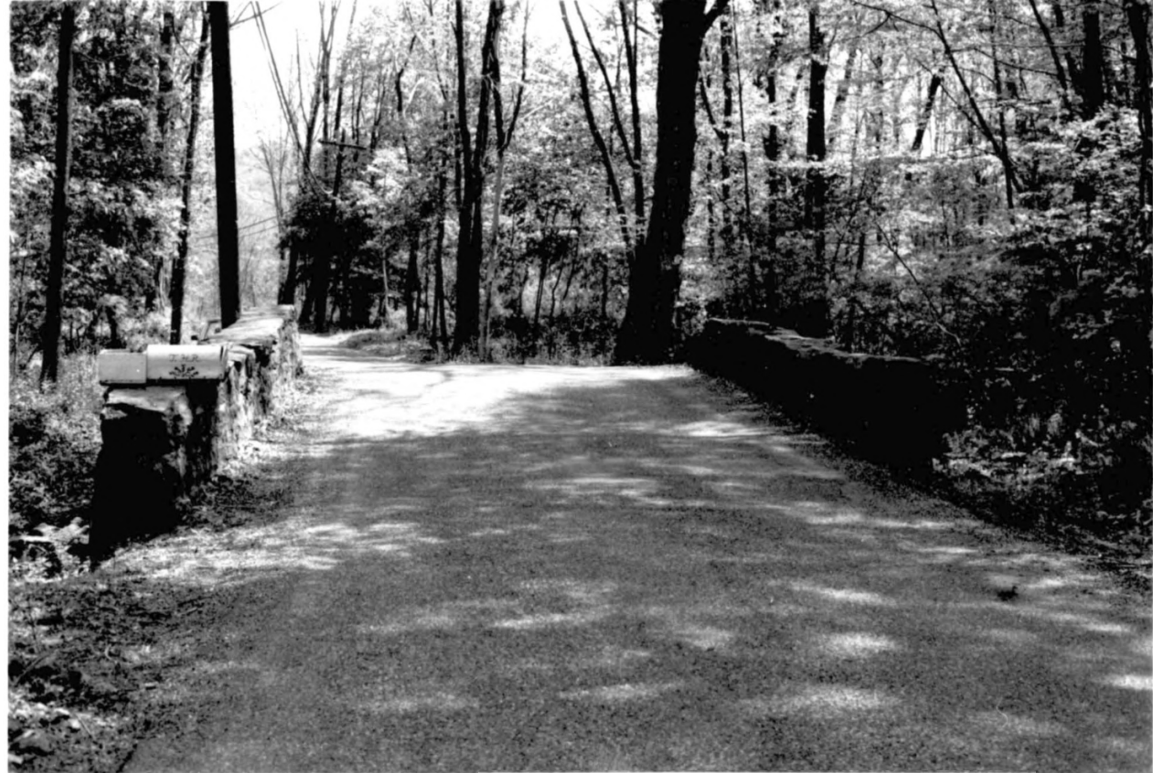
FROG HOLLOW ROAD BRIDGE, TEWKSBURY TWP., HUNTERDON CO. PHOTO 2015
