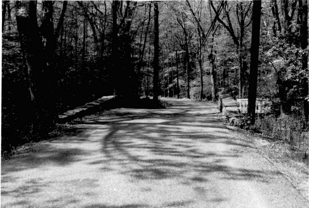
FROG HOLLOW ROAD BRIDGE, TEWKSBURY TWP., HUNTERDON CO. PHOTO 1 OF 5
