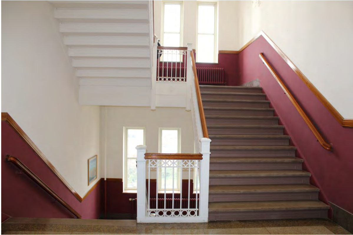
20 of 20 Main stair
