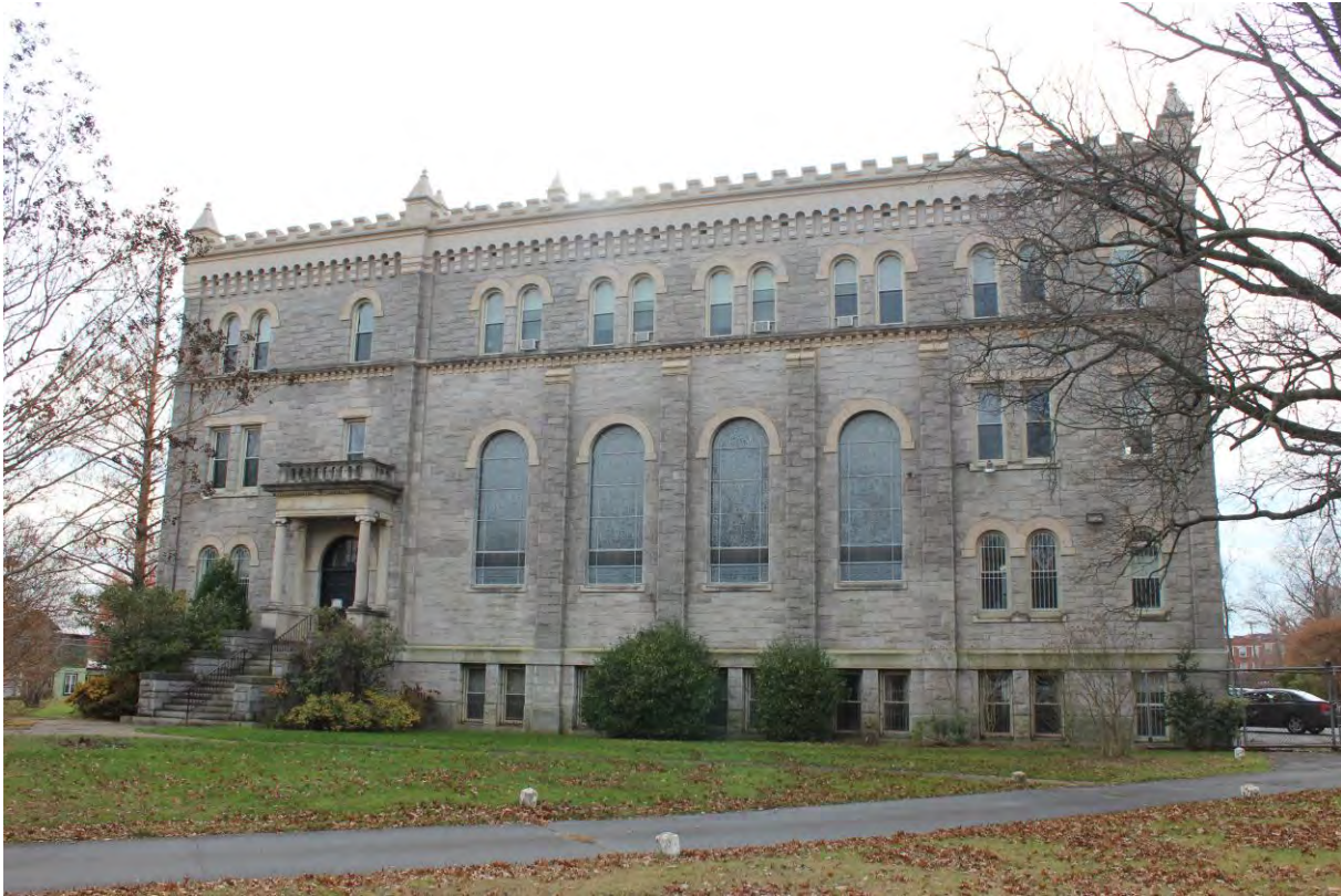
2 of 20 North (side) elevation, facing south
