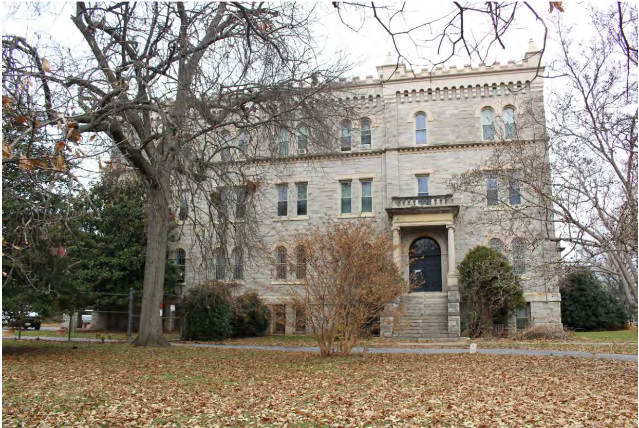
3 of 20 South (side) elevation, facing north
