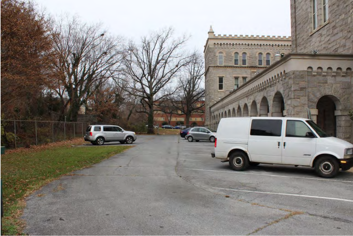
14 of 20 Rear parking lot, facing north
