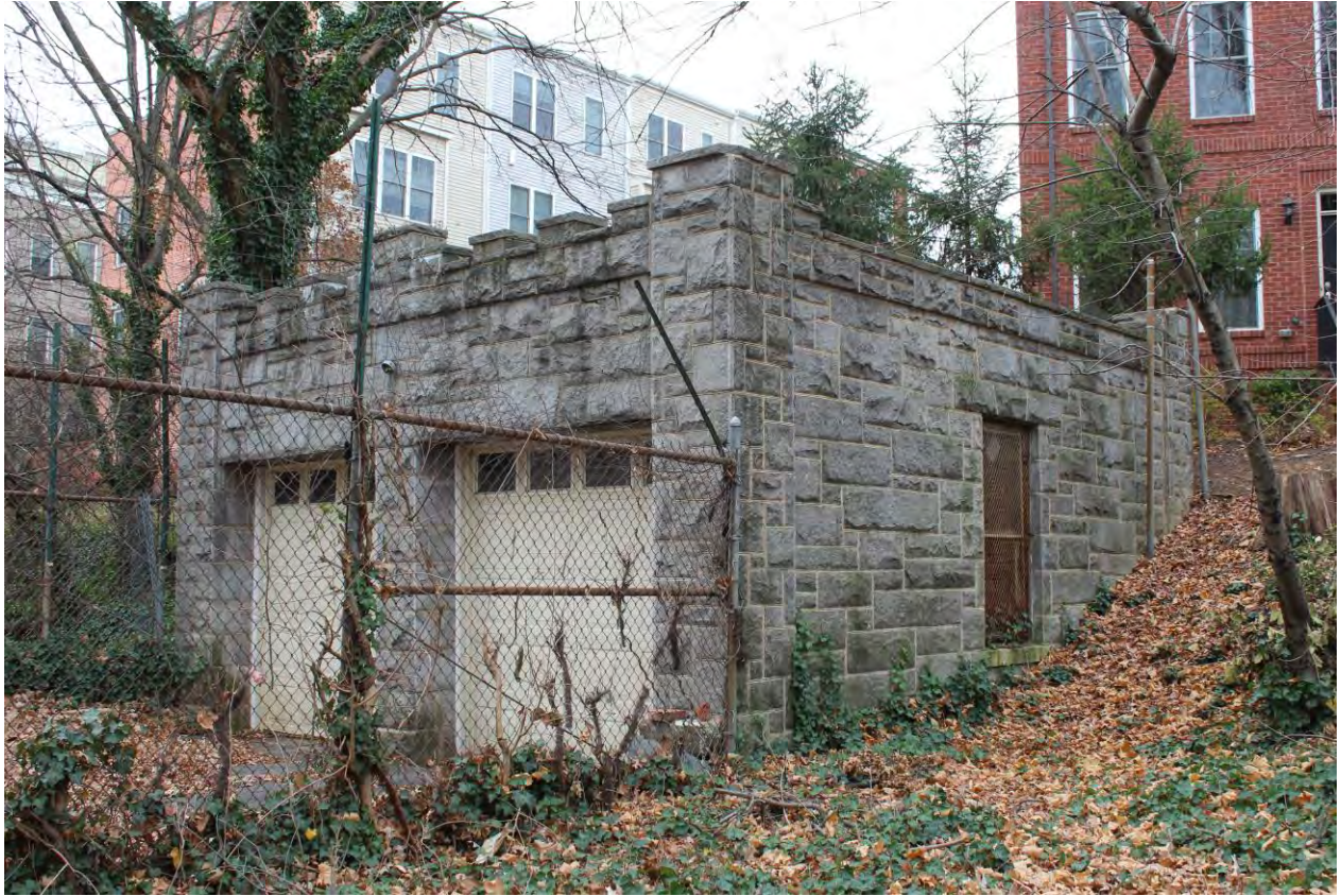
15 of 20 Garage, facing southwest
