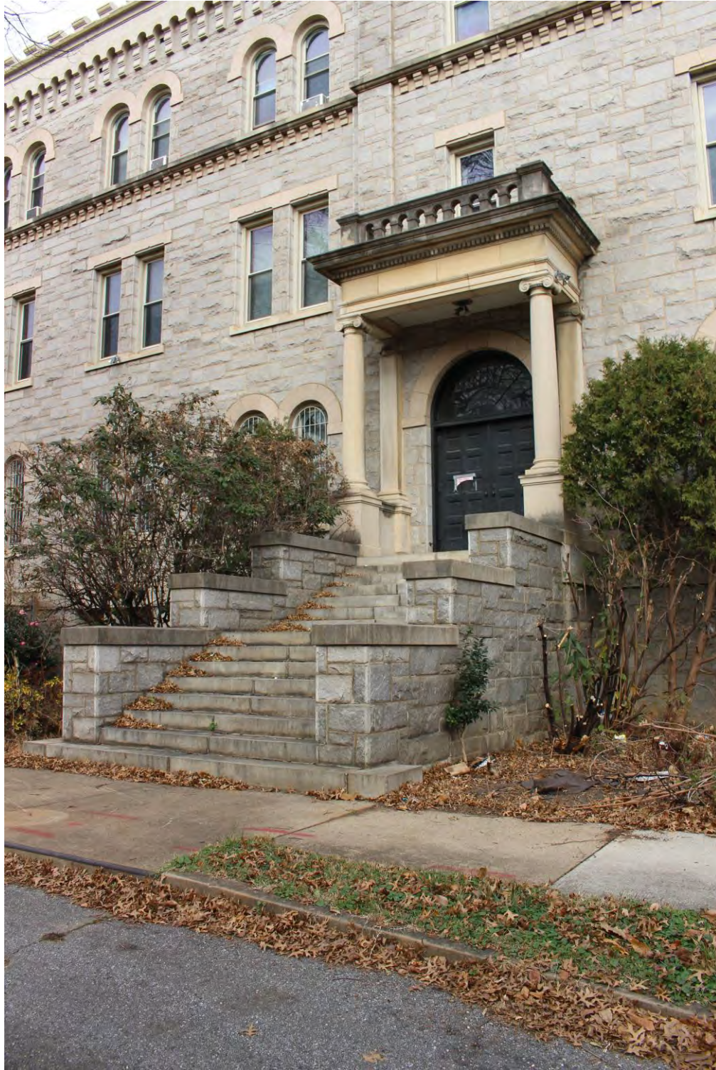
9 of 20 South entrance, facing northwest
