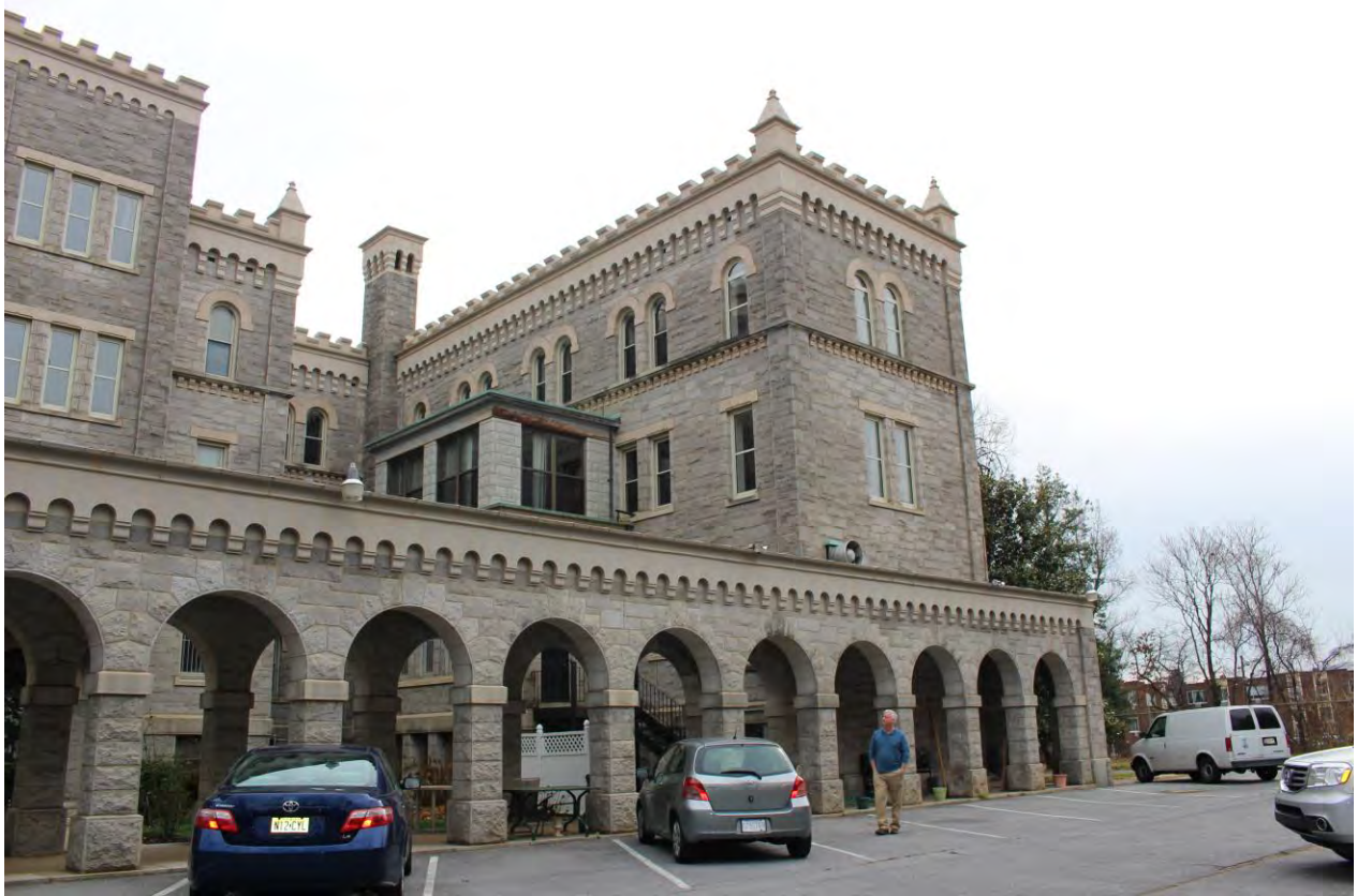
6 of 20 West (rear) elevation, facing southeast
