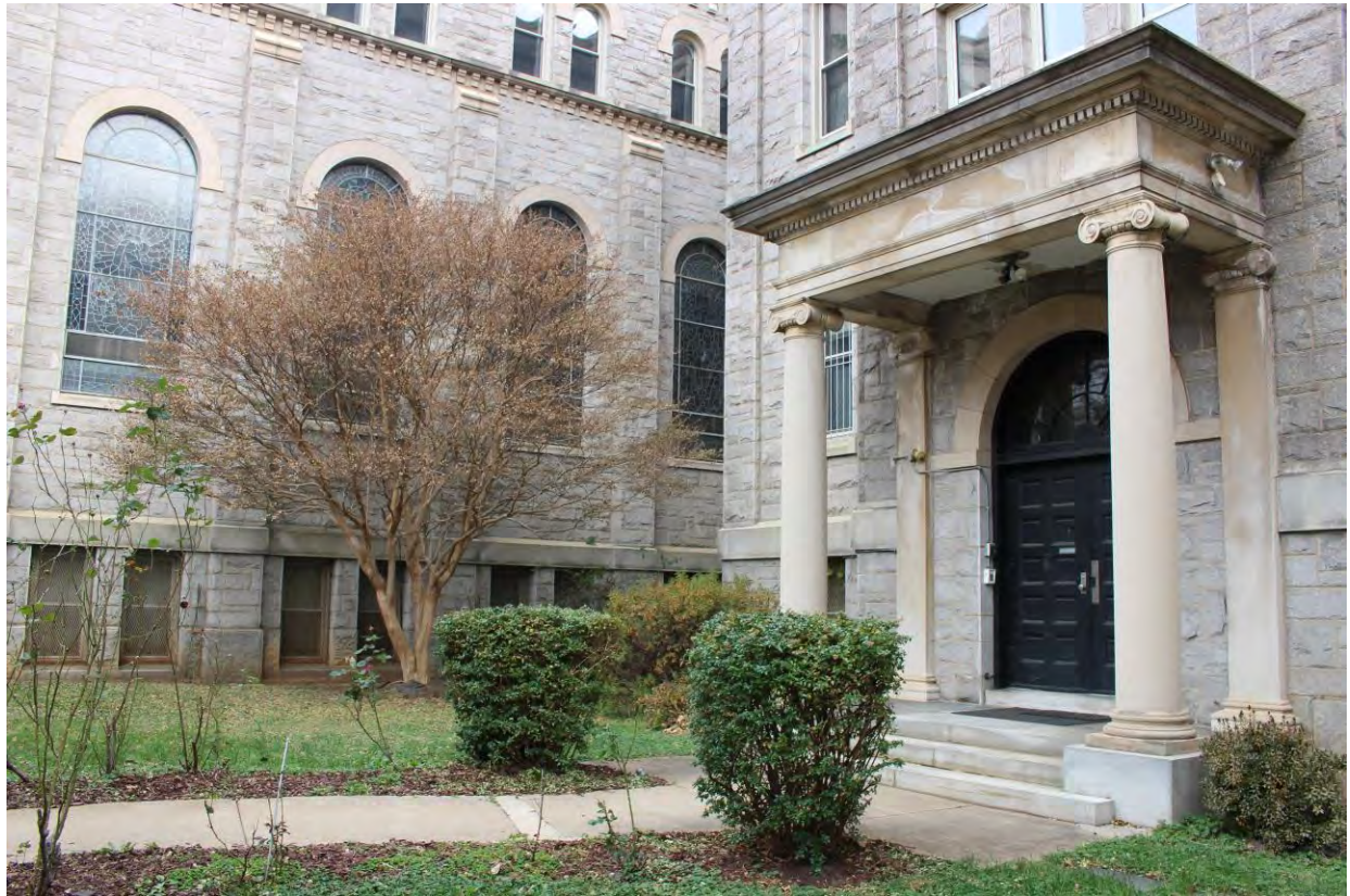
13 of 20 Rear courtyard with entrance, facing northeast
