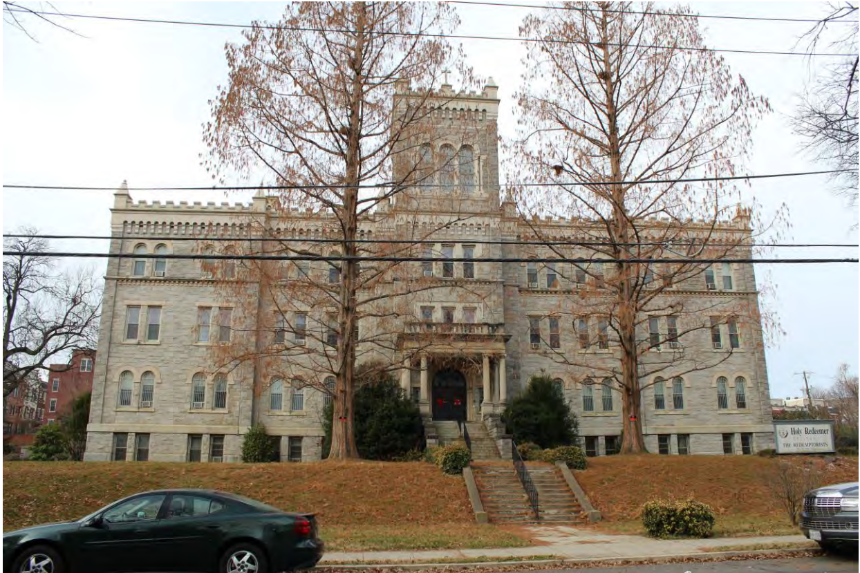
1 of 20 Front (east) elevation, facing west
