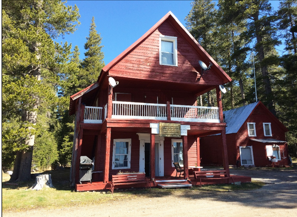
Photo 1: Webber Lake Hotel, south elevation, looking northeast
