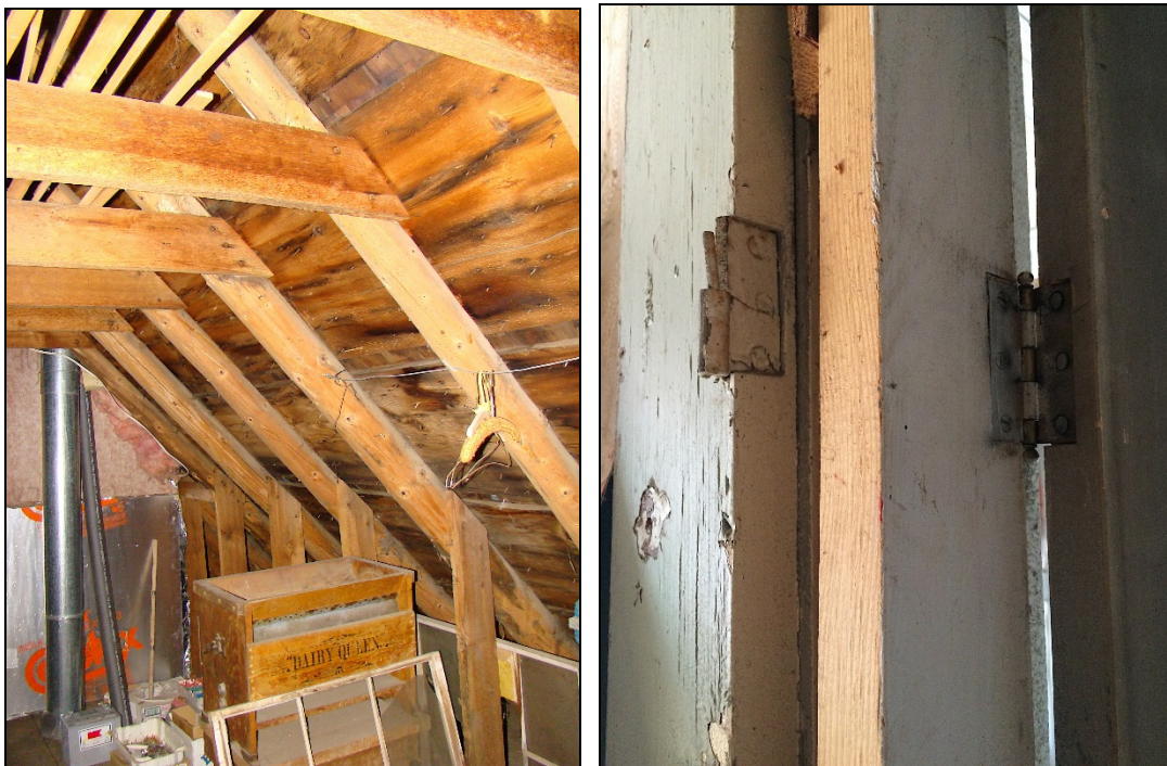
Photo 14: Webber Lake Hotel 4-panel door in Room 209, looking west (right)
