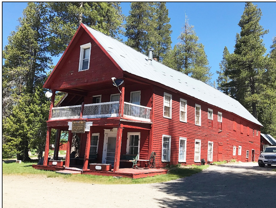
Photo 3: Webber Lake Hotel east elevation, looking northwest
