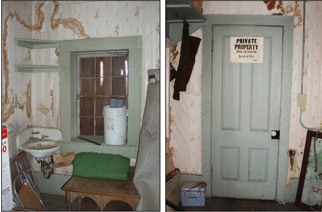
Photo 13: Webber Lake Hotel sink, shelf, and window in Room 209, looking east (left)
