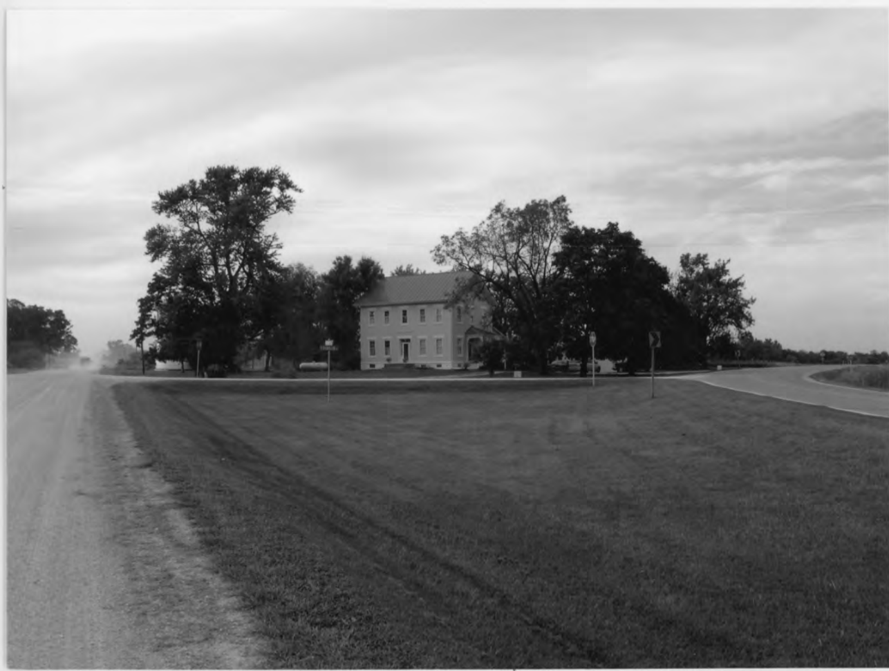
Cook-Johnson House, Salem, Henry County, Iowa, Photograph 1
