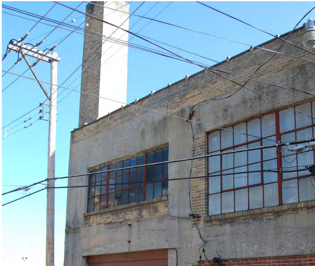
Figure 8. Second story windows, west elevation, are original.
