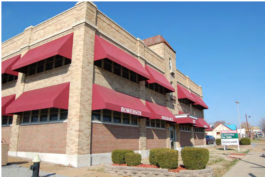
Figure 2. First-floor display windows have been partially infilled on the east and south elevations with brick and bands of one-over-one windows. View is northwest.
