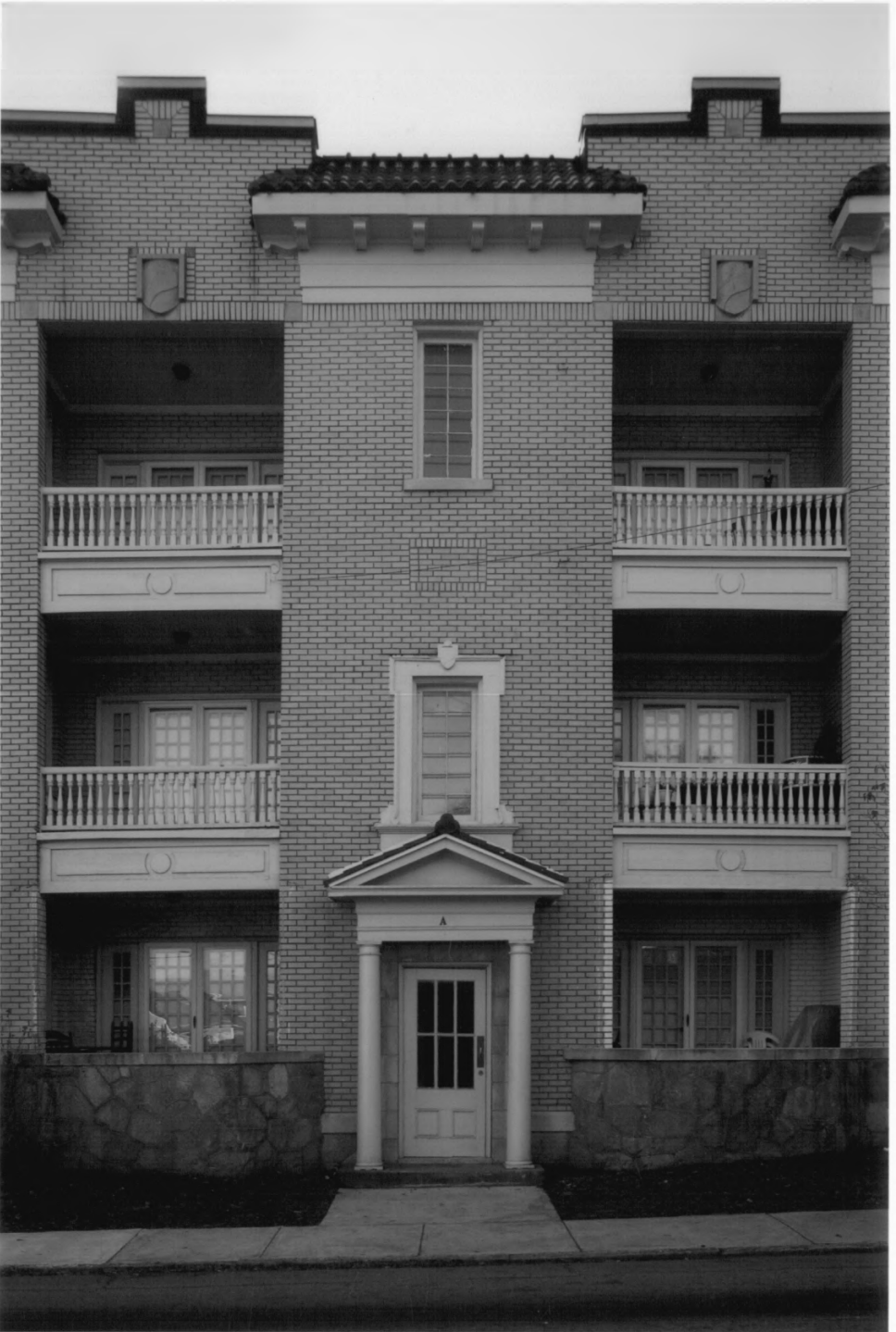
Marian Apartments Spalding County, Georgia Photograph 7 of 15
