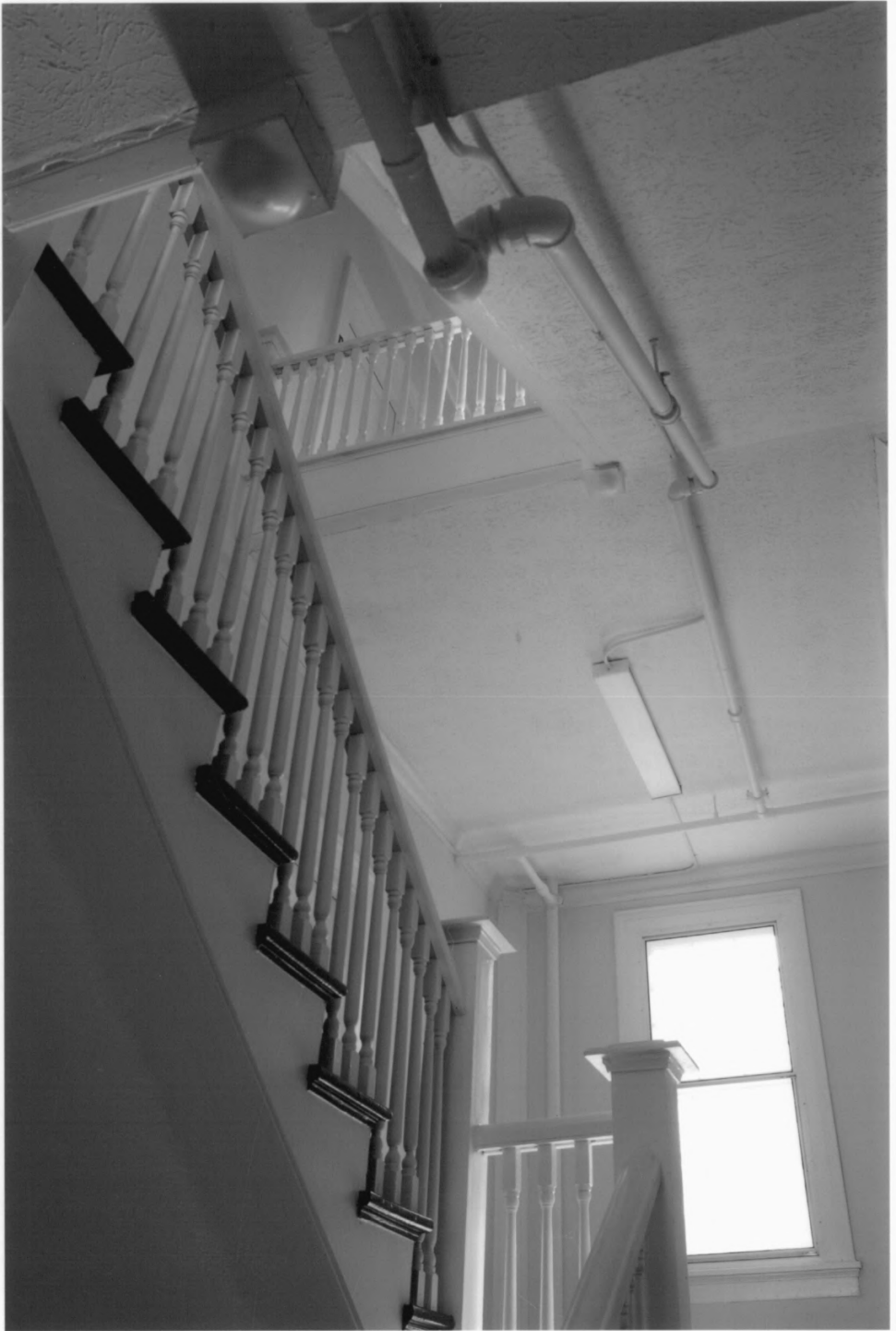
Marian Apartments Spalding County, Georgia Photograph 12 of 15
