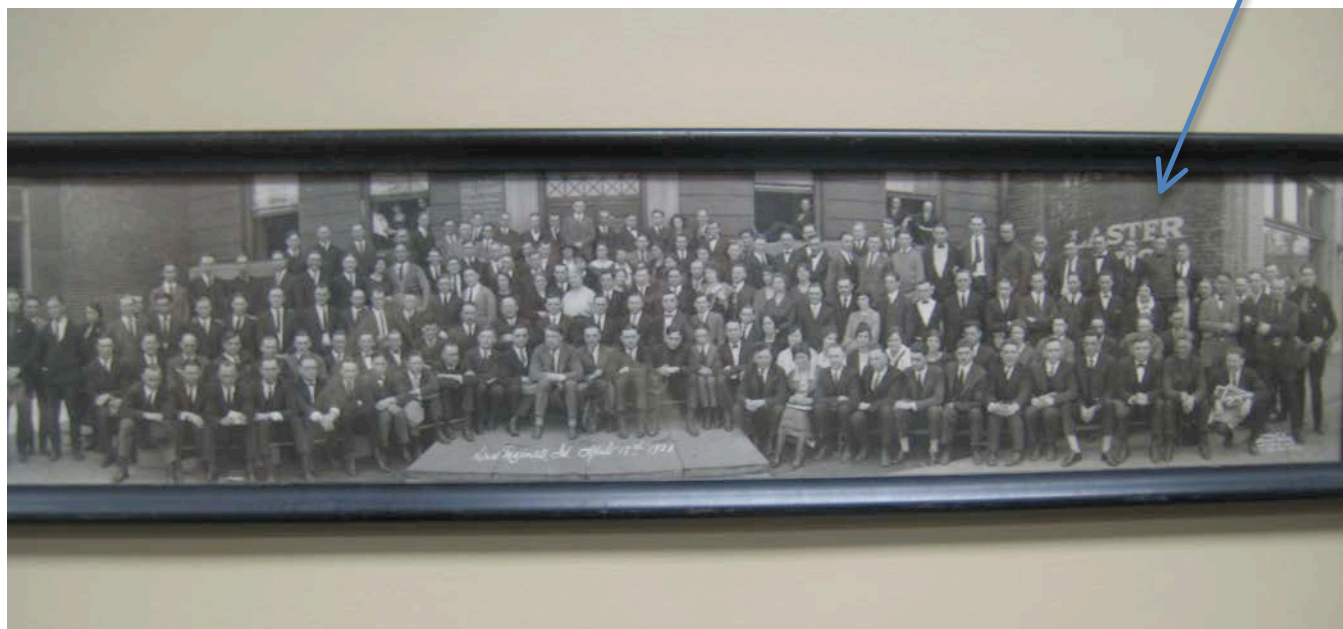
Figure 6. HISTORIC IMAGE – G.W. Jones Building, 1430 Locust Street, April 1923
