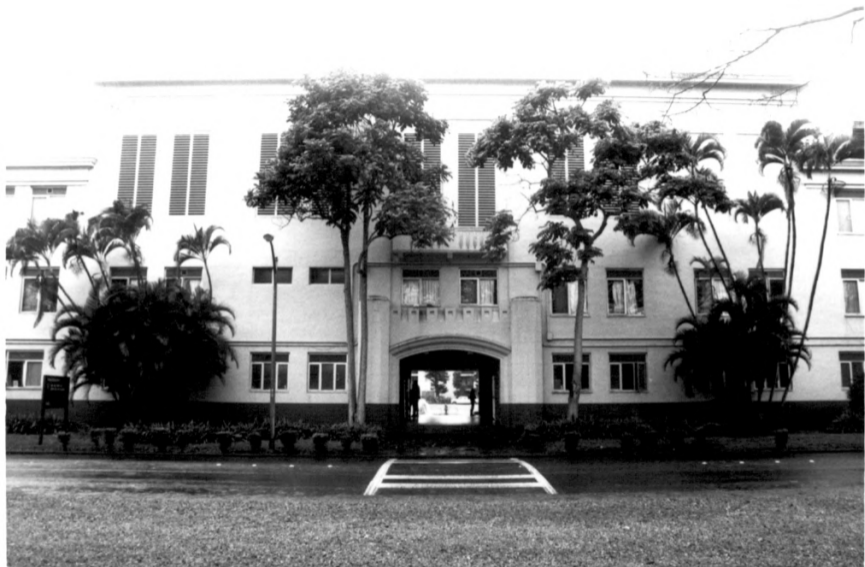
Building 649, Schotfield Barracks Historic District Honolulu County, Hawaii Photo 20
