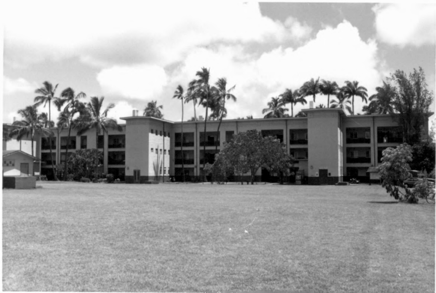
Buildings 846; Schofield Barracks Historic District Honolulu County, Hawaii Photo 28
