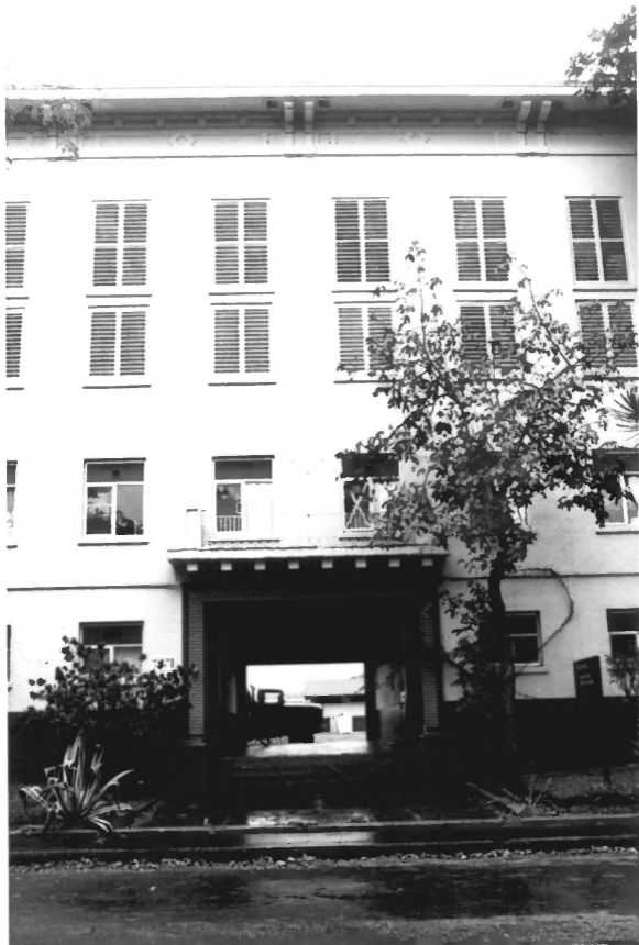
Building 845 - Schofield Barracks Historic District Honolulu County, Hawaii Photo 30
