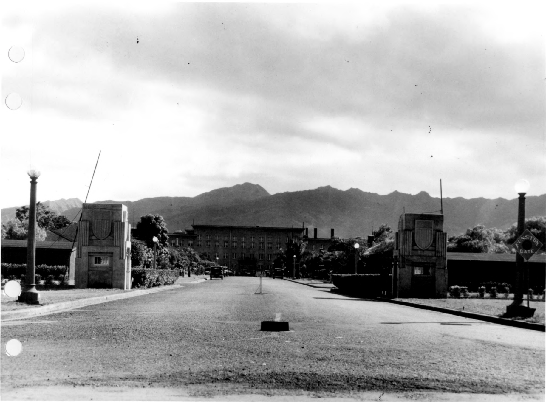
Funston Gate, Schofield Barracks Historic District Honolulu County, Hawaii photo 64
