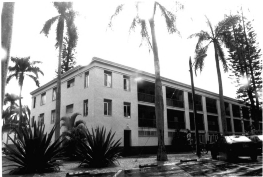
Building 651; Schofield Barracks Historic District Honolulu County, Hawaii Photo 19
