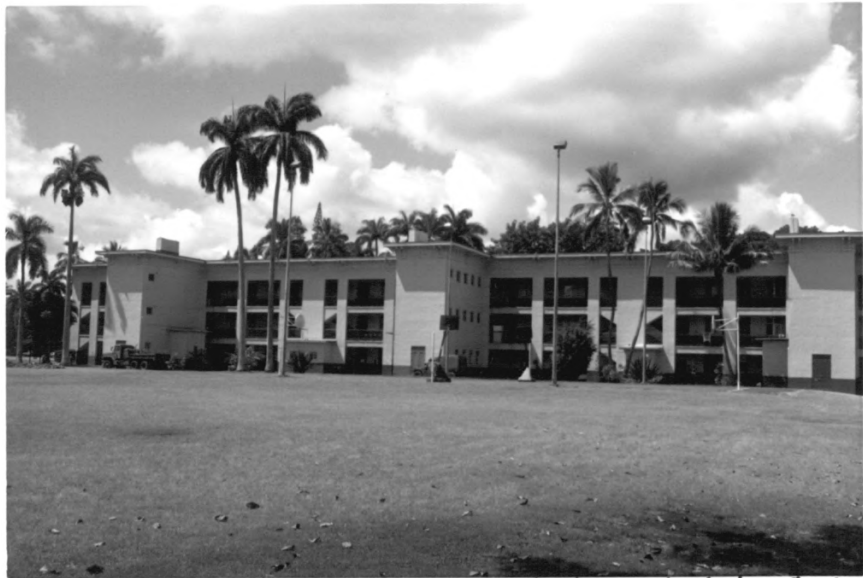
Building 747, Schofield Barracks Historic District Honolulu County, Hawaii photo 23
