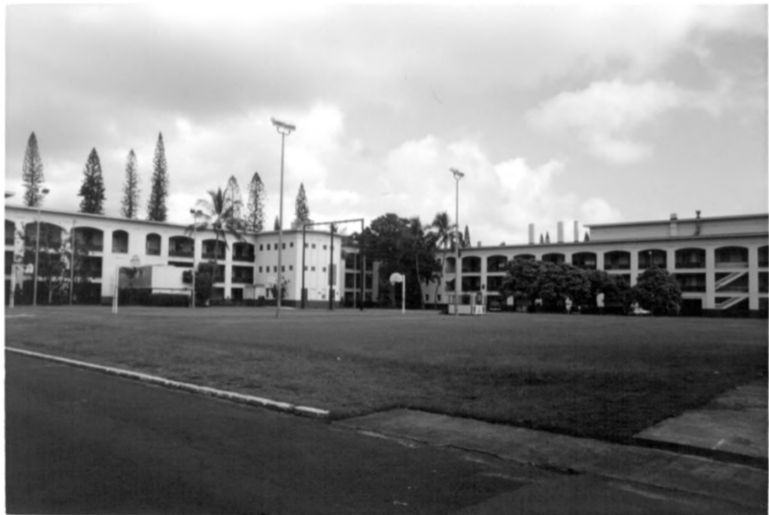
Buildings 449, 451; Schofield Barracks Historic District Honolulu County, Hawaii Photo # 13
