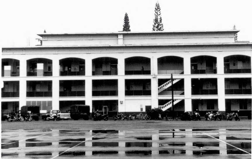
Building 155, Schofield Barracks Historic District Honolulu County, Hawaii Photo # 6
