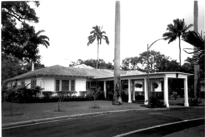
Building 227, Schotfield Barracks Historic District Honolulu County, Hawaii Photo 35
