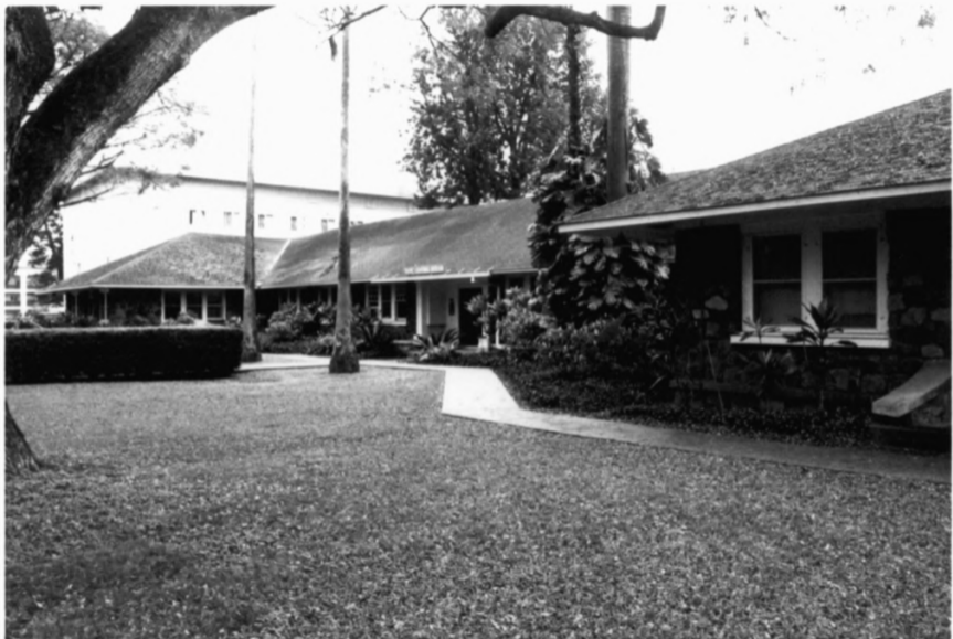
Building 361, Schofield Barracks Historic District Honolulu County Photo # 3
