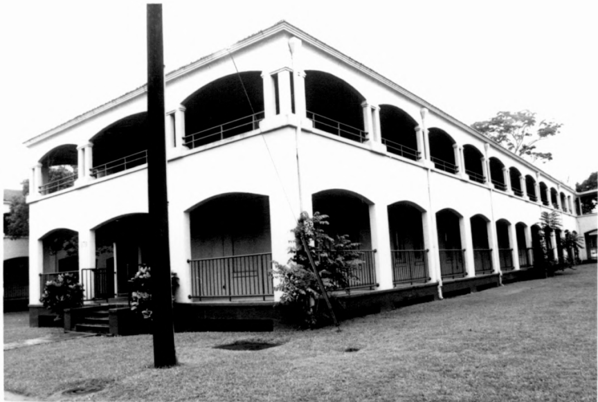
Building 678, Schofield Barracks Historic District Honolulu County, Hawaii photo 47
