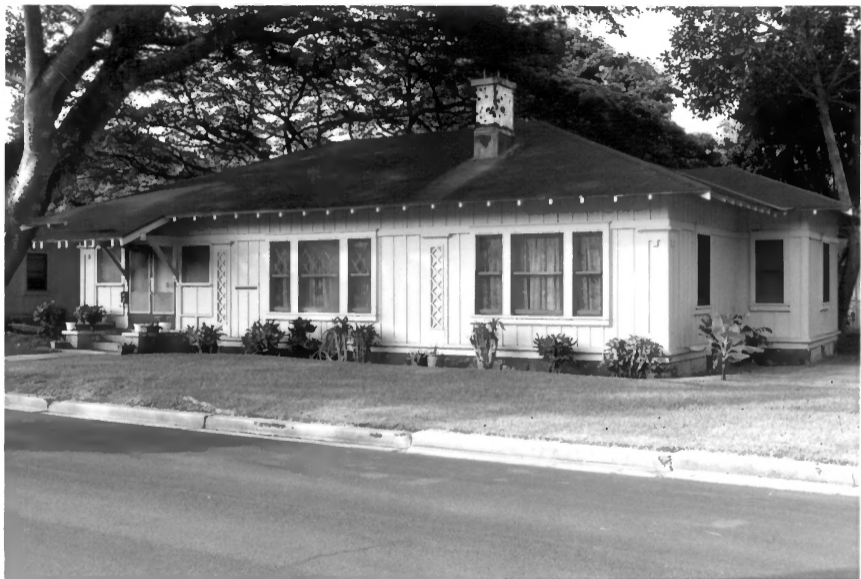
Building 735, Schofield Barracks Historic District Honolulu County, Hawaii Photo 38
