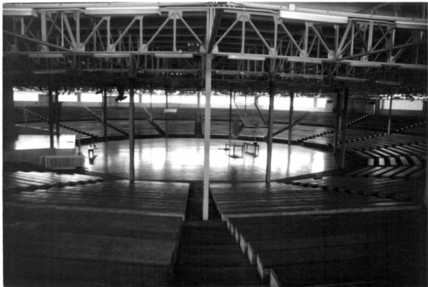
Building 55, Schofield Barracks Historic District Honolulu County, Hawaii photo 55
