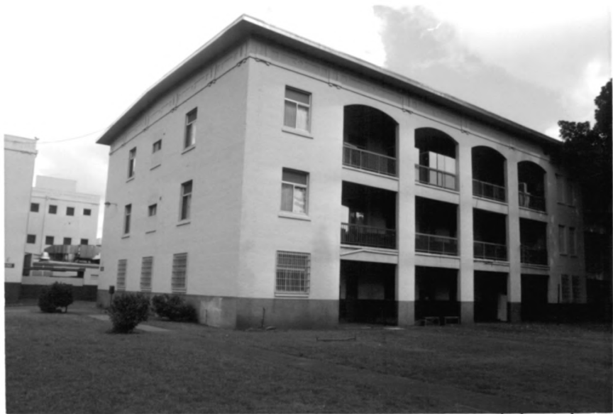
Building 552; Schofield Barracks Historic District Honolulu County, Hawaii Photo # 18
