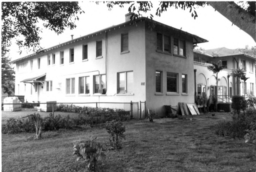
Building 692, Schofield Barracks Historic District Honolulu County, Hawaii Photo 49
