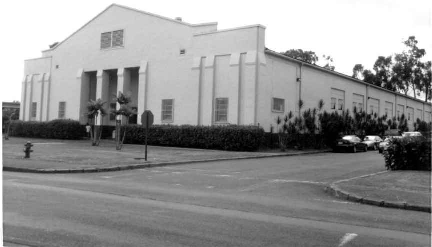
Building 582, Schofield Barracks Historic District Honolulu County, Hawaii photo 57
