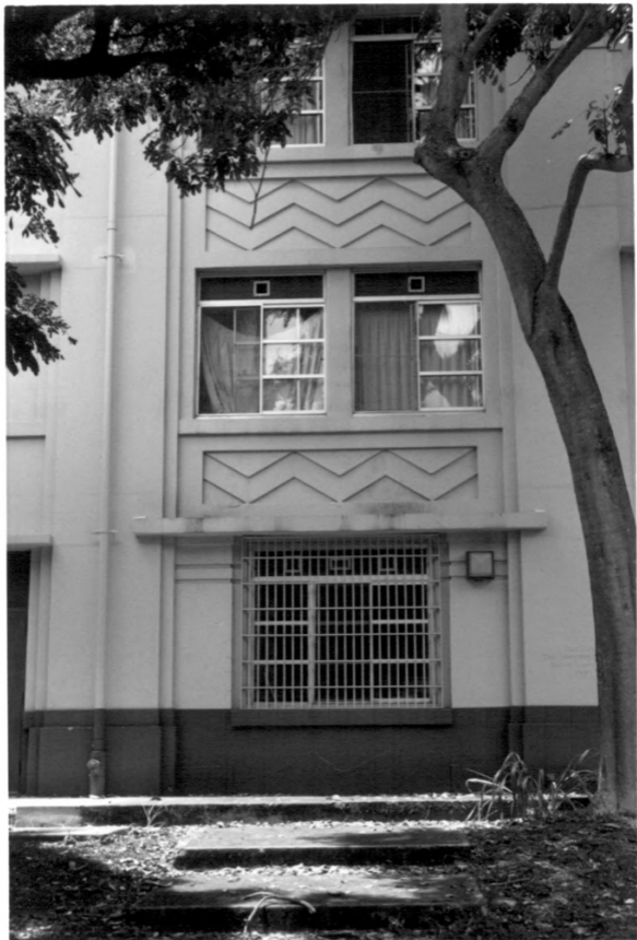
Building 660, Schofield Barracks Historic District Honolulu County, Hawaii Photo 34
