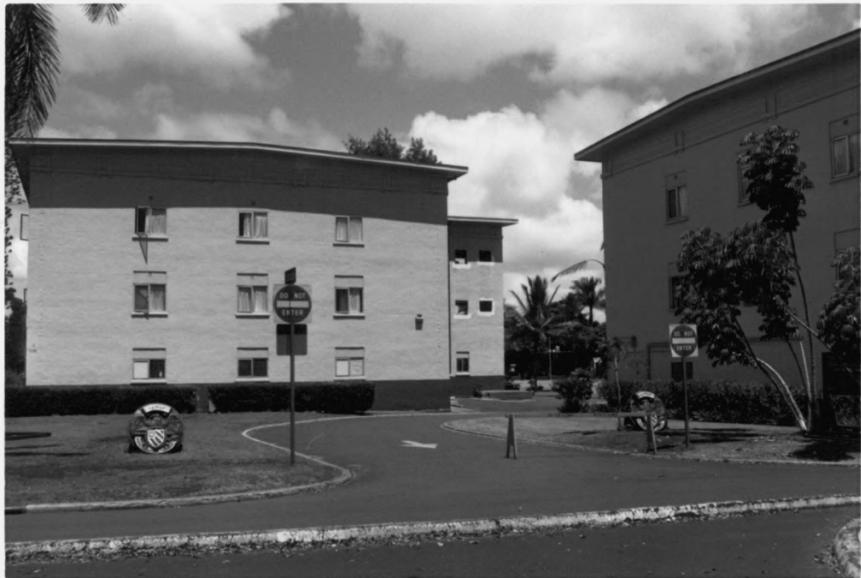
Buildings 847, 845; Schofield Barracks Historic District Honolulu County, Hawaii Photo 27
