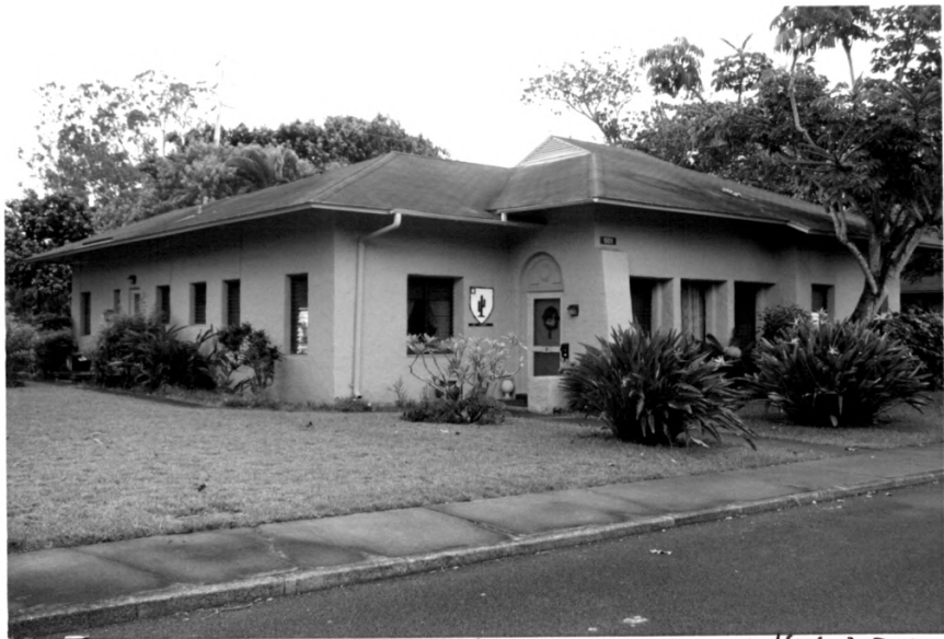
Building 601, Schofield Barracks Historic District Honolulu County, Hawaii Photo 43
