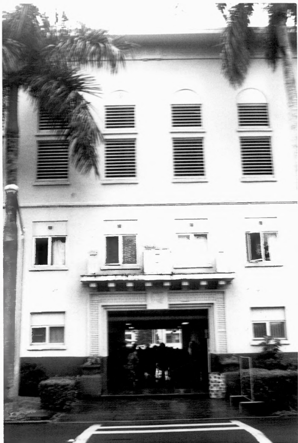
Building 355, Schofield Barracks Historic District Honolulu County, Hawaii Photo # 12
