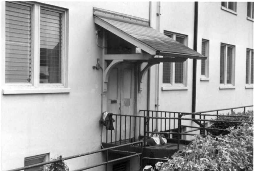
Building 692, Schofield Barracks Historic District Honolulu County, Hawaii Photo 50
