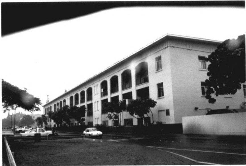
Building 450; Schofield Barracks Historic District Honolulu County, Hawaii photo #15
