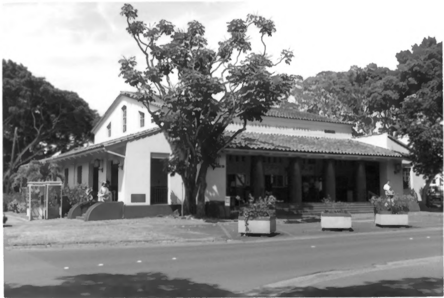
Building 258, Schofield Barracks Historic District Honolulu County, Hawaii Photo 51
