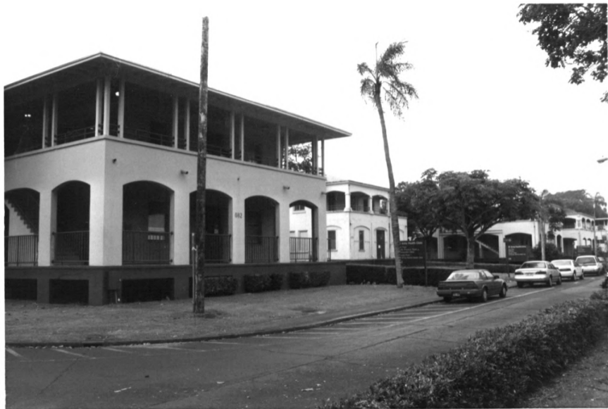
Building 682, Schofield Barracks Historic District Honolulu County, Hawaii Photo 46
