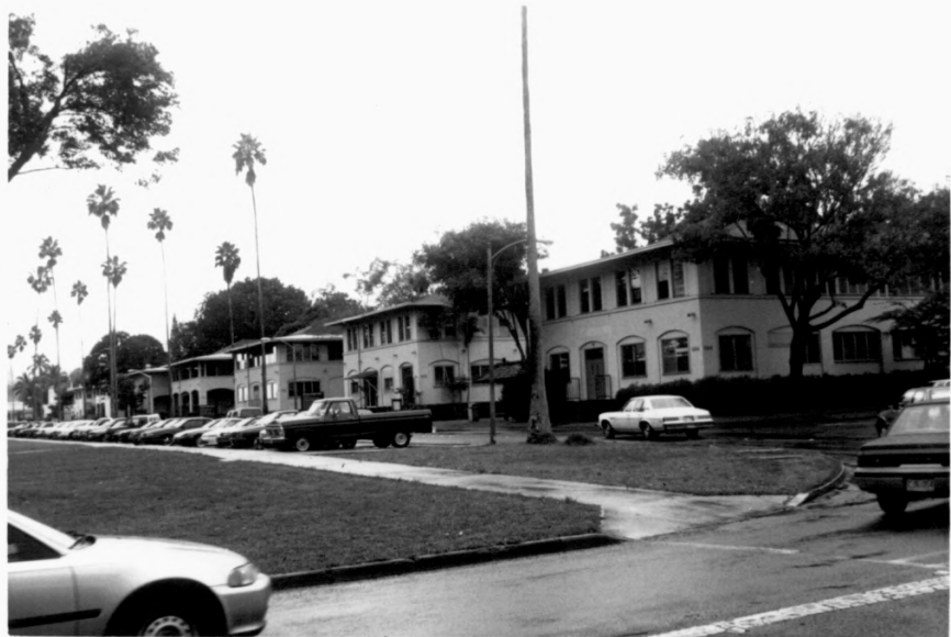
Building 5 684-687, Schofield Barracks Historic District Honolulu County, Hawaii Photo 44
