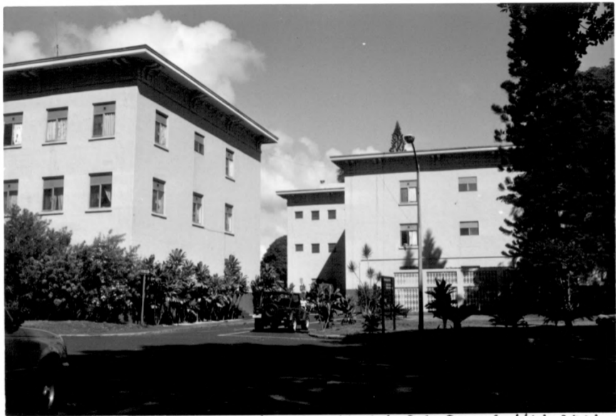
Buildings 745 746 : Schofield Barracks Historic District Honolulu County, Hawaii Photo 26
