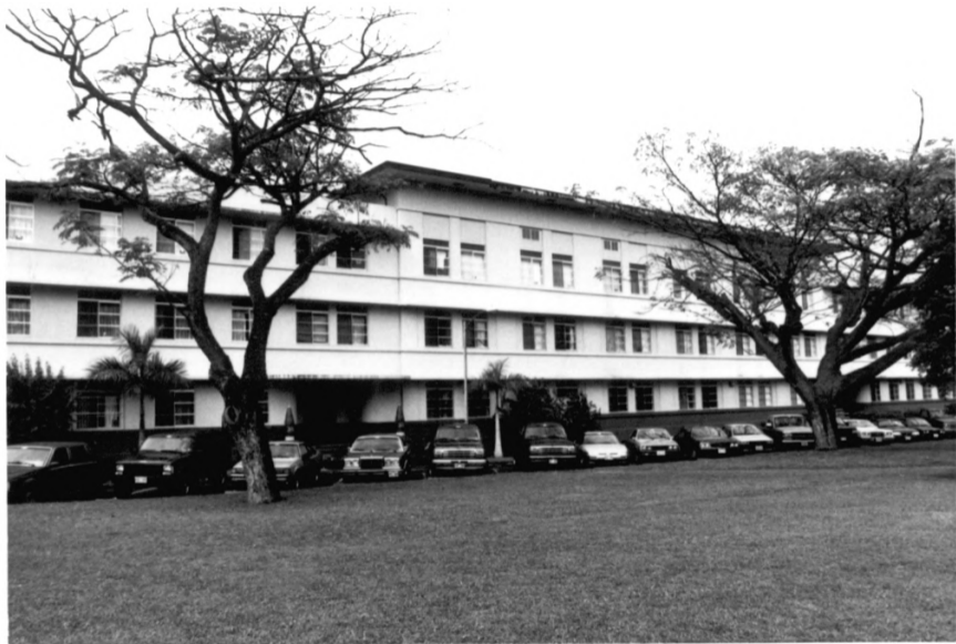
Building 860, Schofield Barracks Historic District Honolulu County, Hawaii Photo 33
