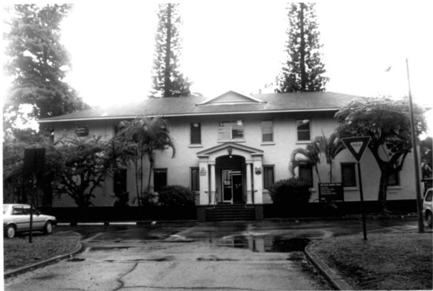
Building 683, Schofield Barracks Historic District Honolulu County, Hawaii Photo 45
