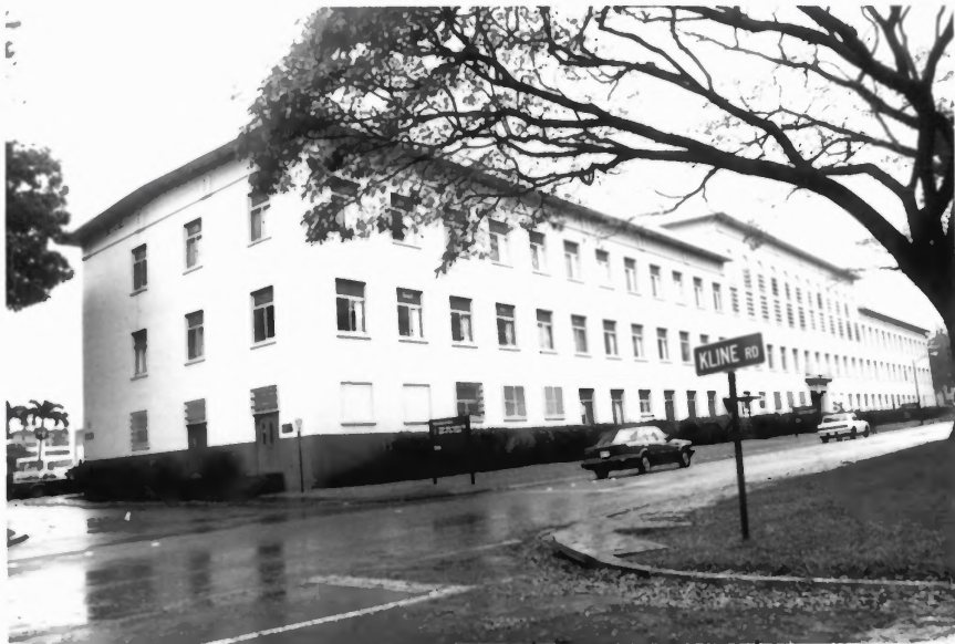
Building 549, Schofield Barracks Historic District Honolulu County, Hawaii photo # 17
