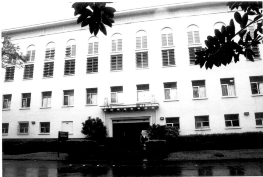
Building 449; Schiefel Barracks Historic District Honolulu County, Hawaii Photo # 16
