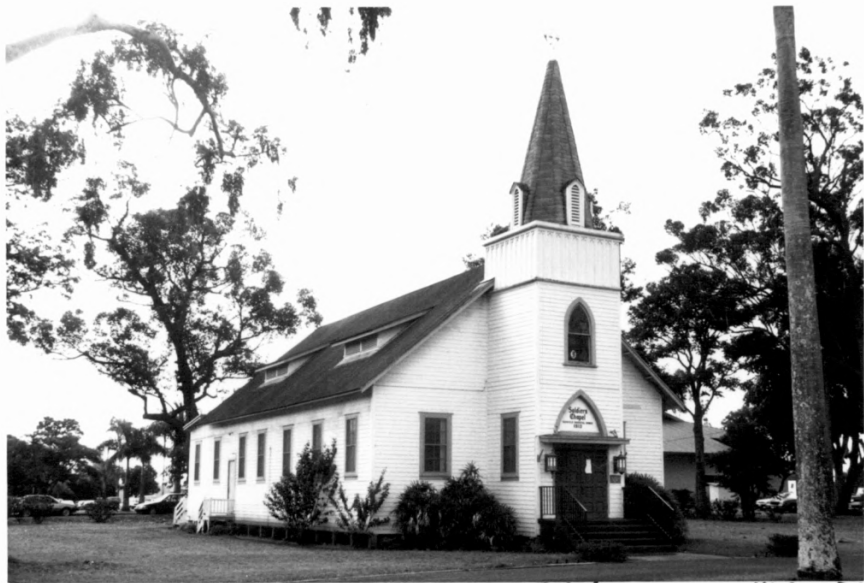
Building 590, Schofield Barracks Historic District Honolulu County Photo 59
