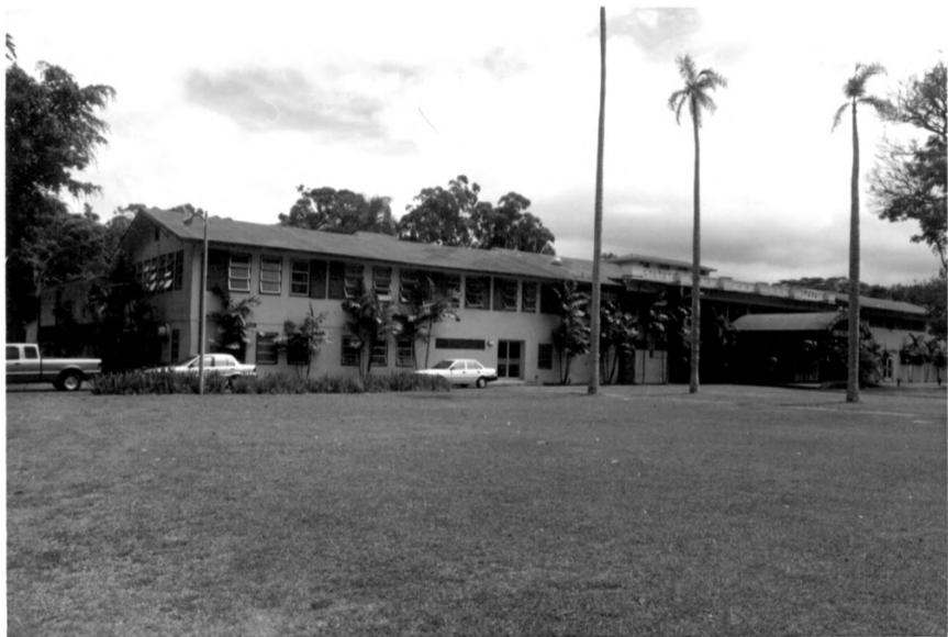
Building 750, Schofield Barracks, Historic District Honolulu County, Hawaii Photo 63
