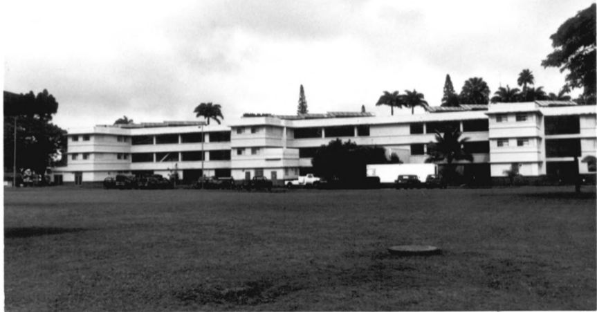
Building 859, Schofield Barracks Historic District Honolulu County, Hawaii photo 31
