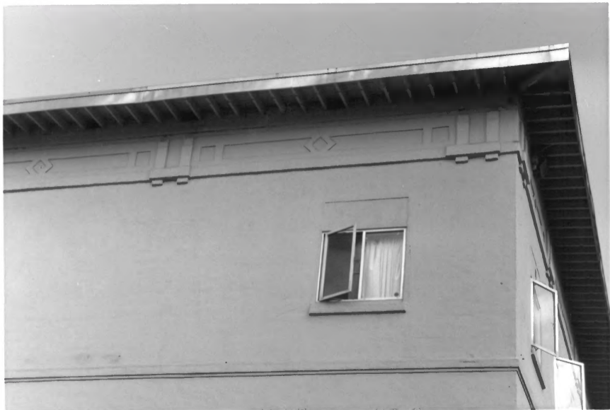
Building 357, Schofield Barracks Historic District Honolulu County, Hawaii Photo # 11
