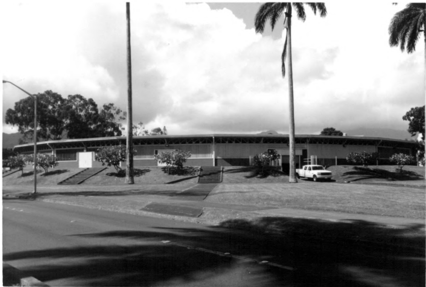
Building 555, Schofield Barracks Historic District Honolulu County, Hawaii Photo 54
