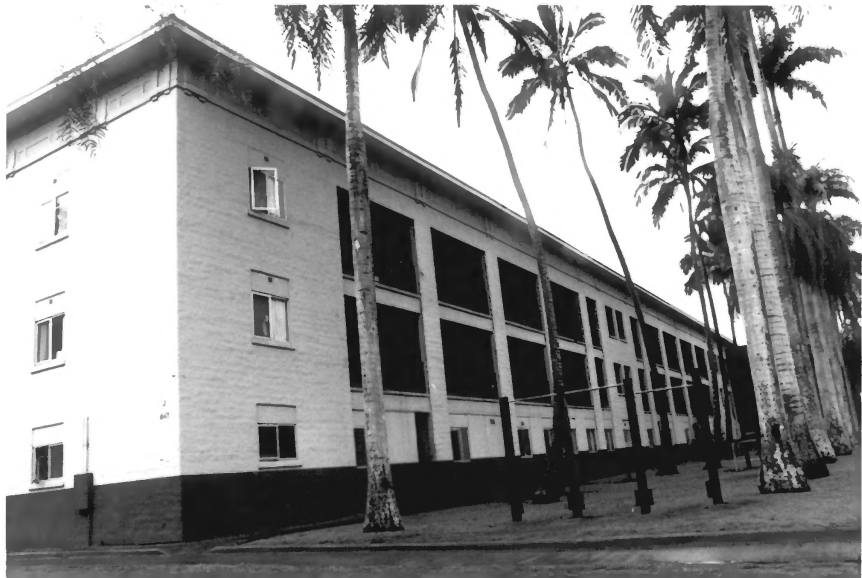
Building 747, Schofield Barracks Historic District Honolulu County, Hawaii PHOTO 25
