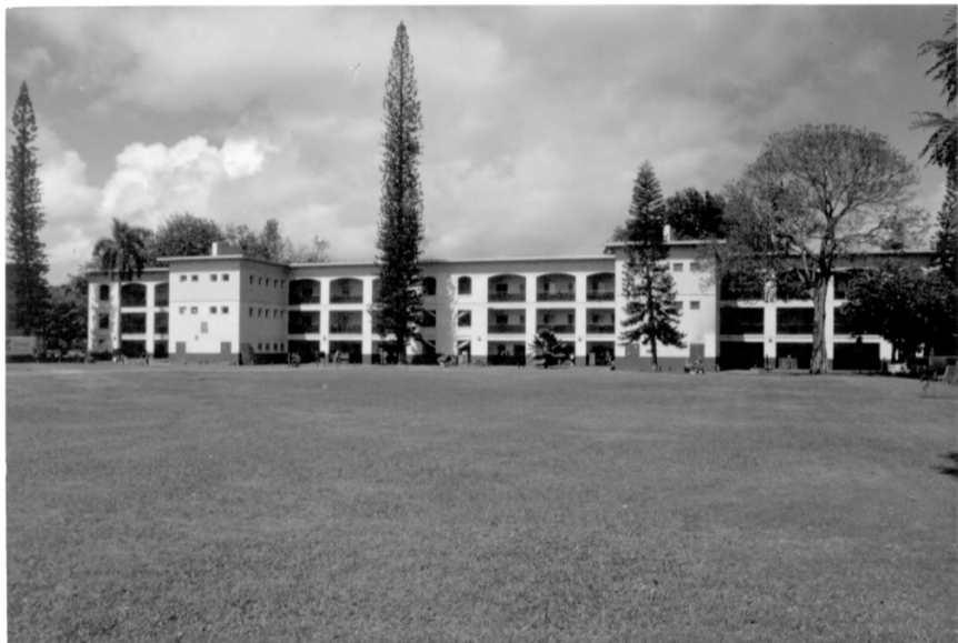
Building 256, Schofield Barracks Historic District Honolulu County, Hawaii photo 49
