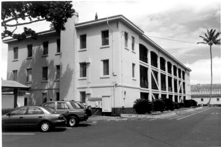
Building 690, Schofield Barracks Historic District Honolulu County, Hawaii Photo 62
