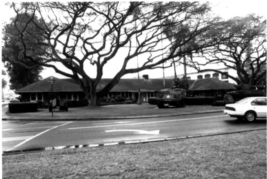
Building 361, Schofield Barracks Historic District Honolulu County, Hawaii Photo #4
