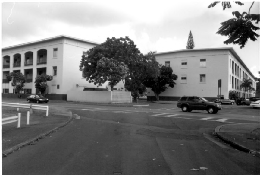
Buildings 450, 452; Schofield Barracks Historic District Honolulu County, Hawaii photo # 14
