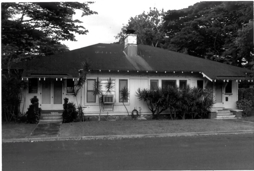
Building 844 ; Schofield Barracks Historic District Honolulu County, Hawaii Photo 37
