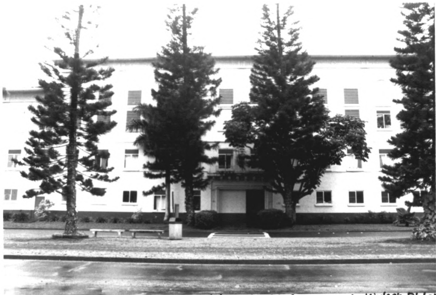
Building 155, Schiefel Barracks Historic District Honolulu County, Hawaii Photo #7
