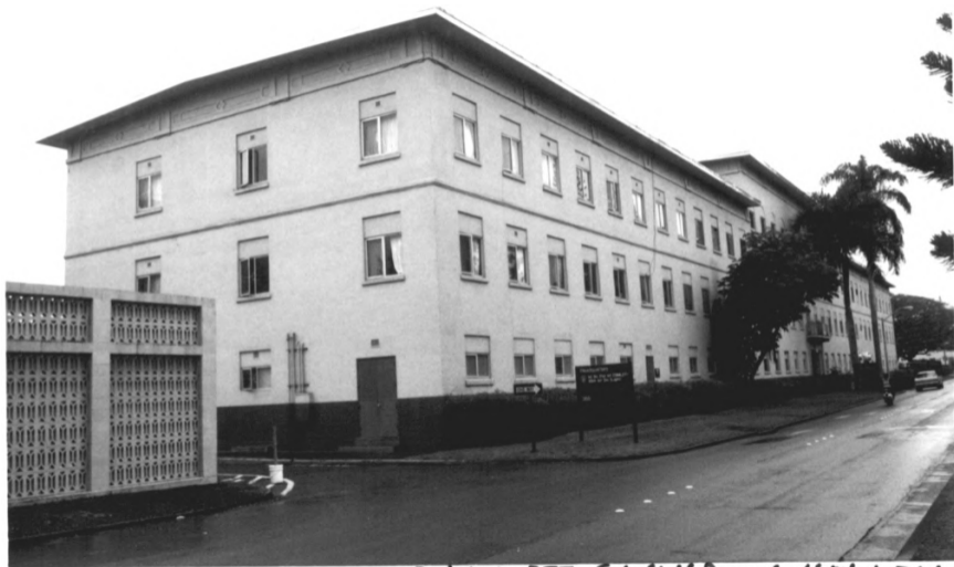
Building 355, Schofield Barracks Historic District Honolulu County, Hawaii Photo # 10
