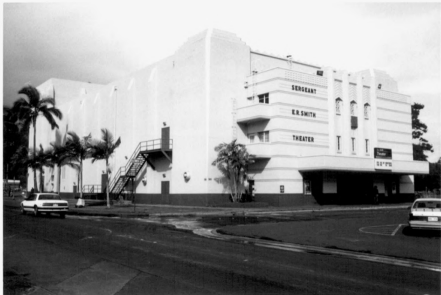
Building 583, Schofield Barracks Historic District Honolulu County, Hawaii photo 53
