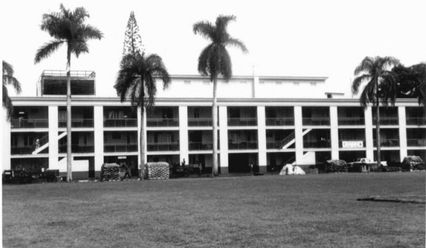
Building 649, Schofield Barracks Historic District Honolulu County, Hawaii photo 22
