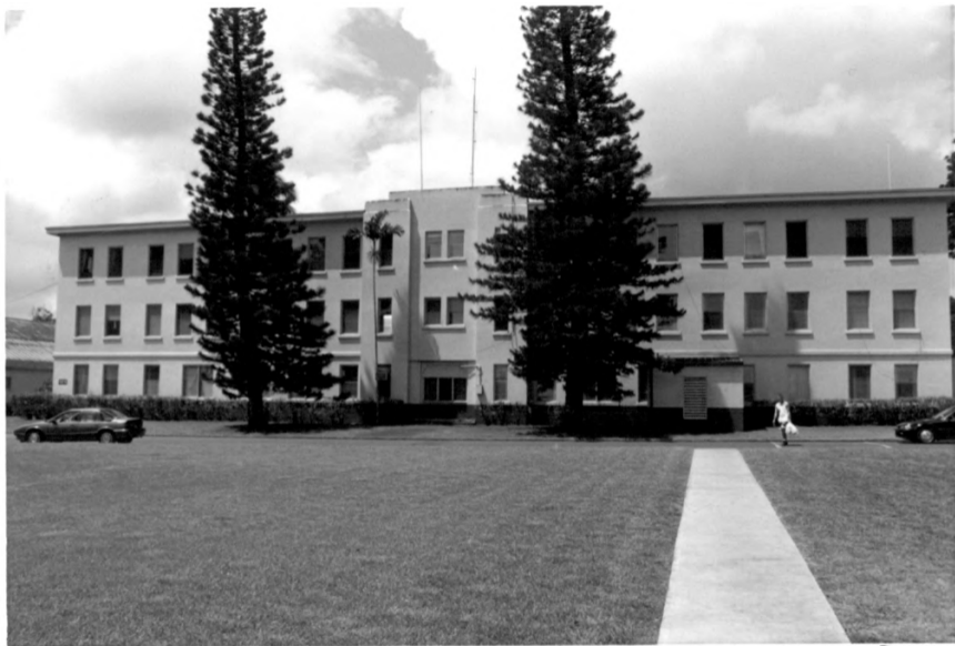
Building 690, Schofield Barracks Historic District Honolulu County, Hawaii Photo 61
