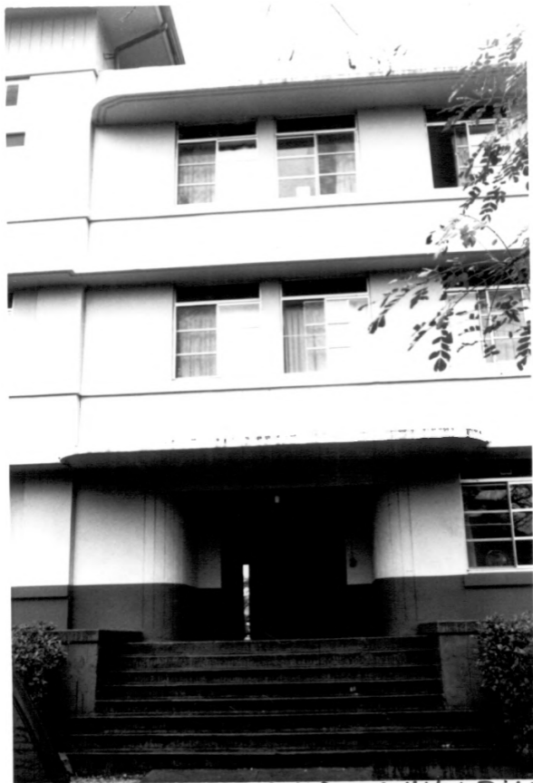
Building B59, Schofield Barracks Historic District Honolulu County, Hawaii photo 32
