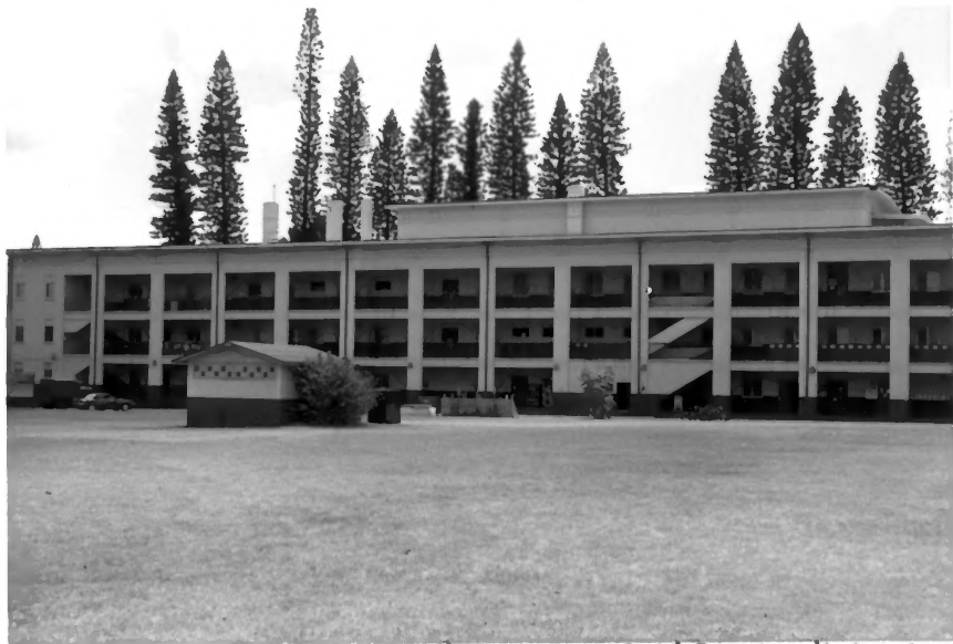
Building 845; Schofield Barracks Historic District Honolulu County, Hawaii Photo 29
