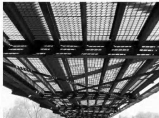
South Span Floor System Looking North
