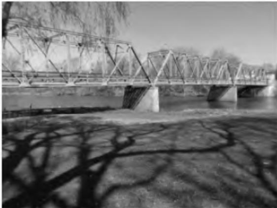
East Elevation from South Embankment
