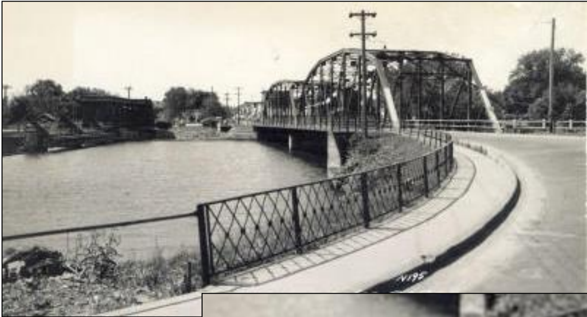
Figure 7: Comparison historic view of Iowa 346, Cedar River Bridge, Nashua, Iowa (nonextant); built 1921 by Illinois Steel Bridge Co., similar details to Third Street SE Bridge, Waverly also based on a design by Iowa State Highway Commission. Note the similarity of the sidewalk balustrade enlargement below that is identical to Third Street SE Bridge in Waverly; see plan design Figs. 6-2 and 6-5. (Photo source: Bridgehunters/com).
