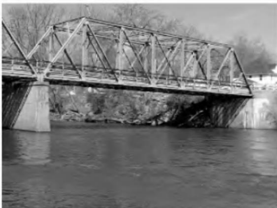
East Elevation North Span
