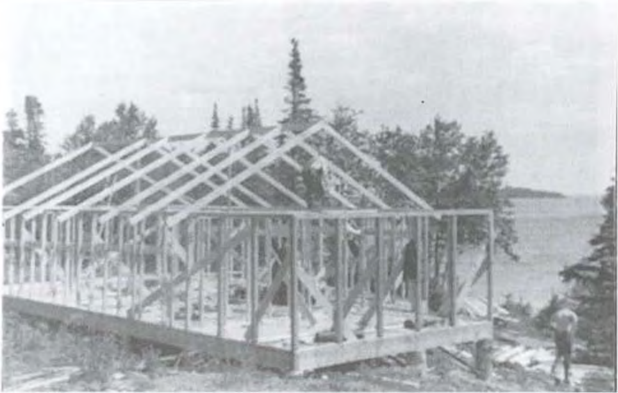
Figure 20. Gale cottage under construction in 1937. Gale Family Photo
