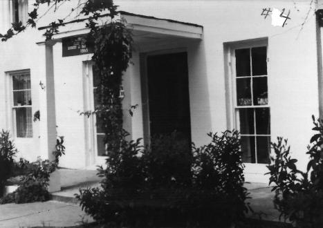
East side of house (front) when the addition was added to the South side, the original porch was removed and this stoop was placed in front of the entrance.
