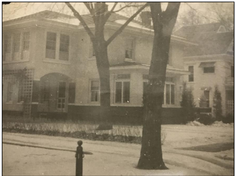
Figure 6: Chain House, looking NW, unknown date.
