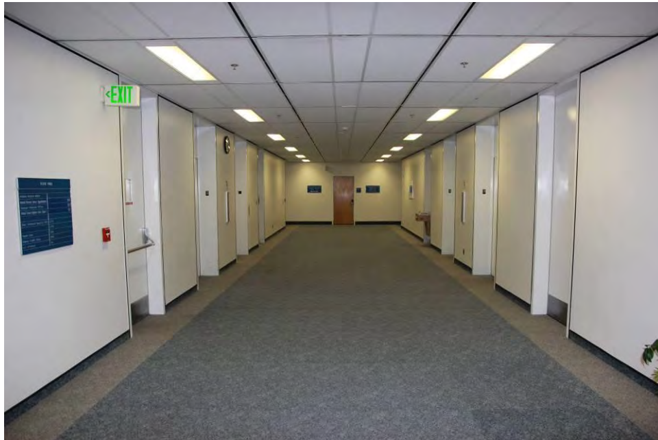
Photo 17 of 26: Typical elevator lobby interior (third floor shown), camera facing west.
