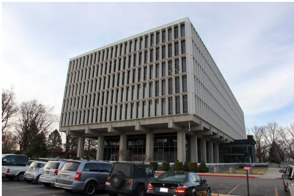
Photo 6 of 26: North elevation and parking lot, camera facing southeast.
