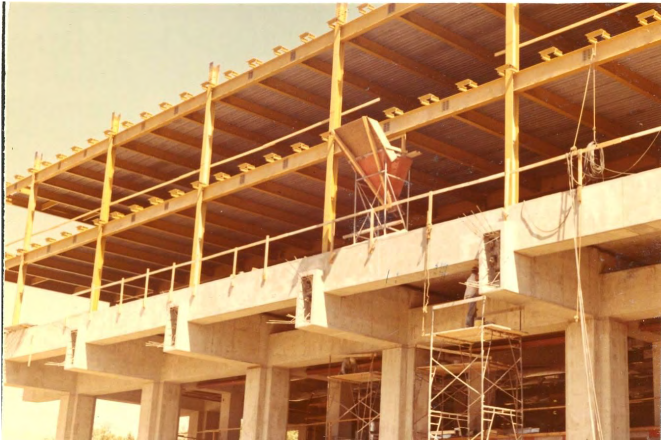
Figure 11: Historic Image, Construction of upper floor systems, 1966 (GSA Archives)
