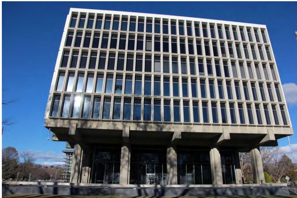
Photo 4 of 26: South elevation, camera facing north.
