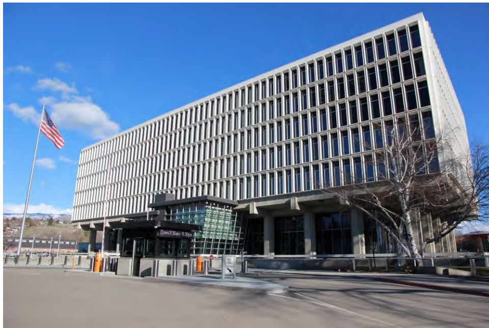
Photo 2 of 26: Primary/west elevation showing entry addition with vehicular entry guard booth in foreground, camera facing northeast.
