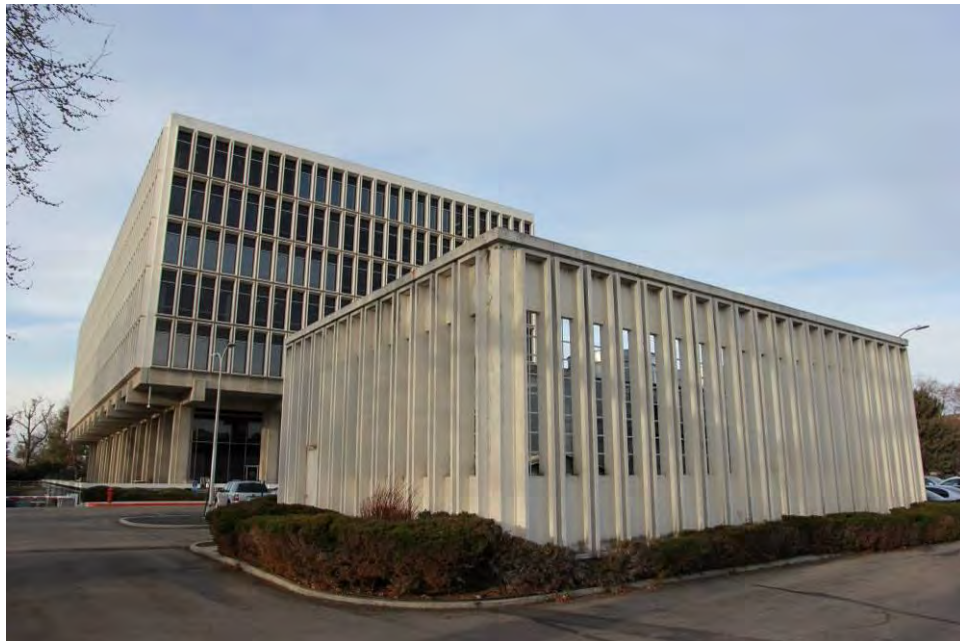
Photo 9 of 26: Mechanical enclosure in north parking lot, camera facing southwest.
