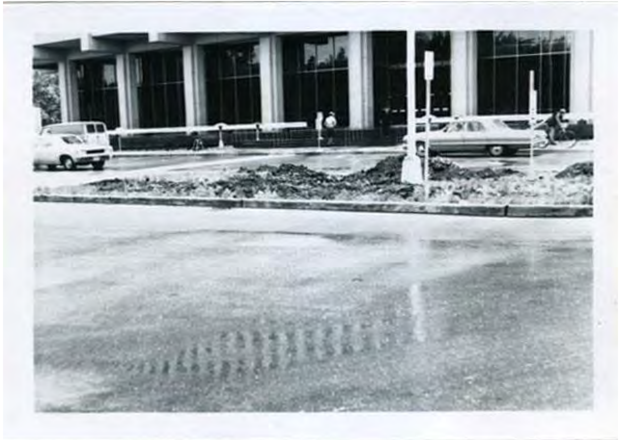
Figure 6: Historic Image, original west stair, podium, and first floor entry configuration, 1967
