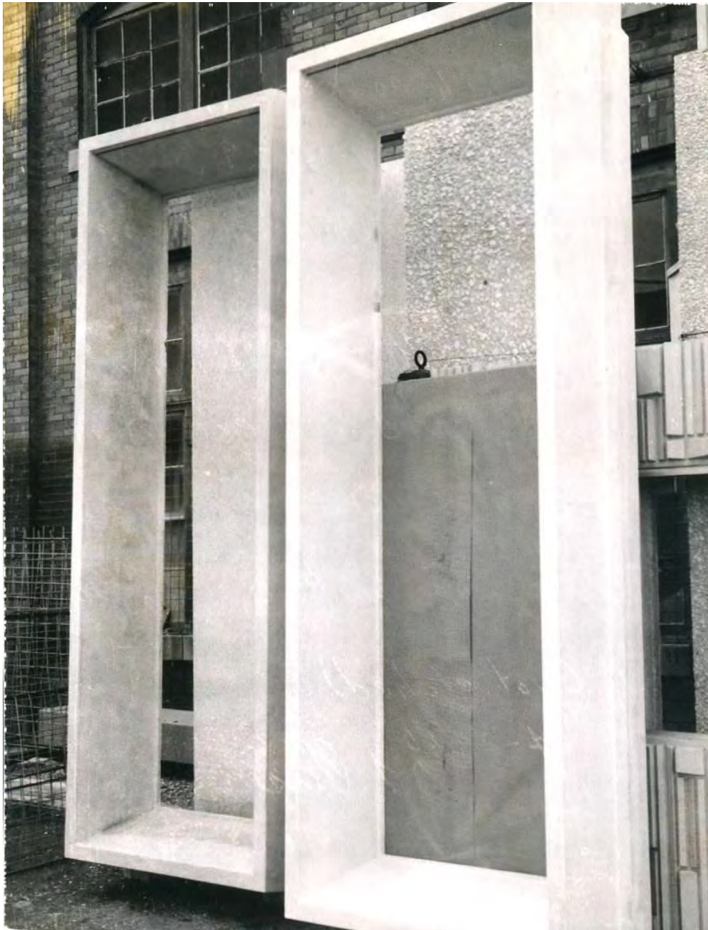
Figure 13: Historic Image, precast concrete window module before installation, 1966 (GSA Archives)
