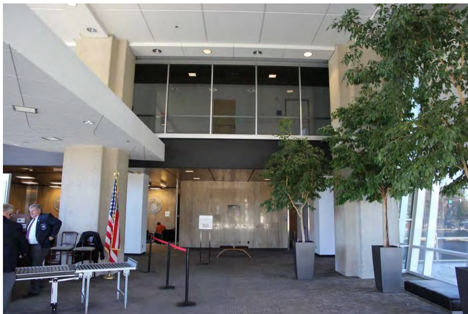
Photo 12 of 26: 2004 west entry addition lobby, camera looking east toward historic west lobby and showing formerly exterior pilotis and two bays where original entry and curtain wall were removed.
