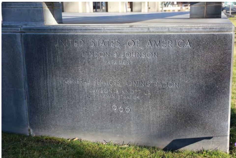
Photo 10 of 26: Granite corner stone at southwest corner of podium, camera facing east.
