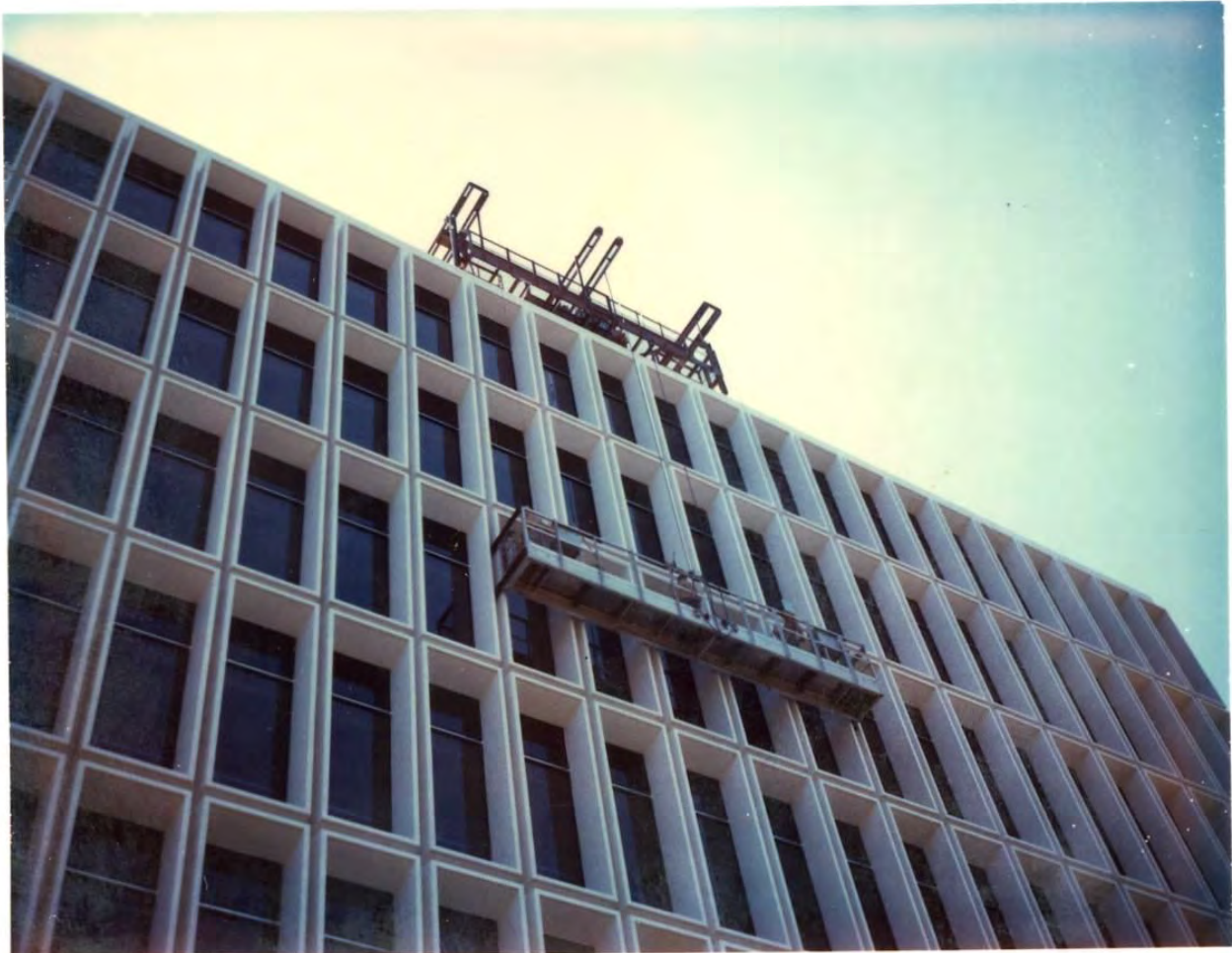
Figure 15: Historic Image, roof top window washing scaffold system, 1967 (GSA Archives)
