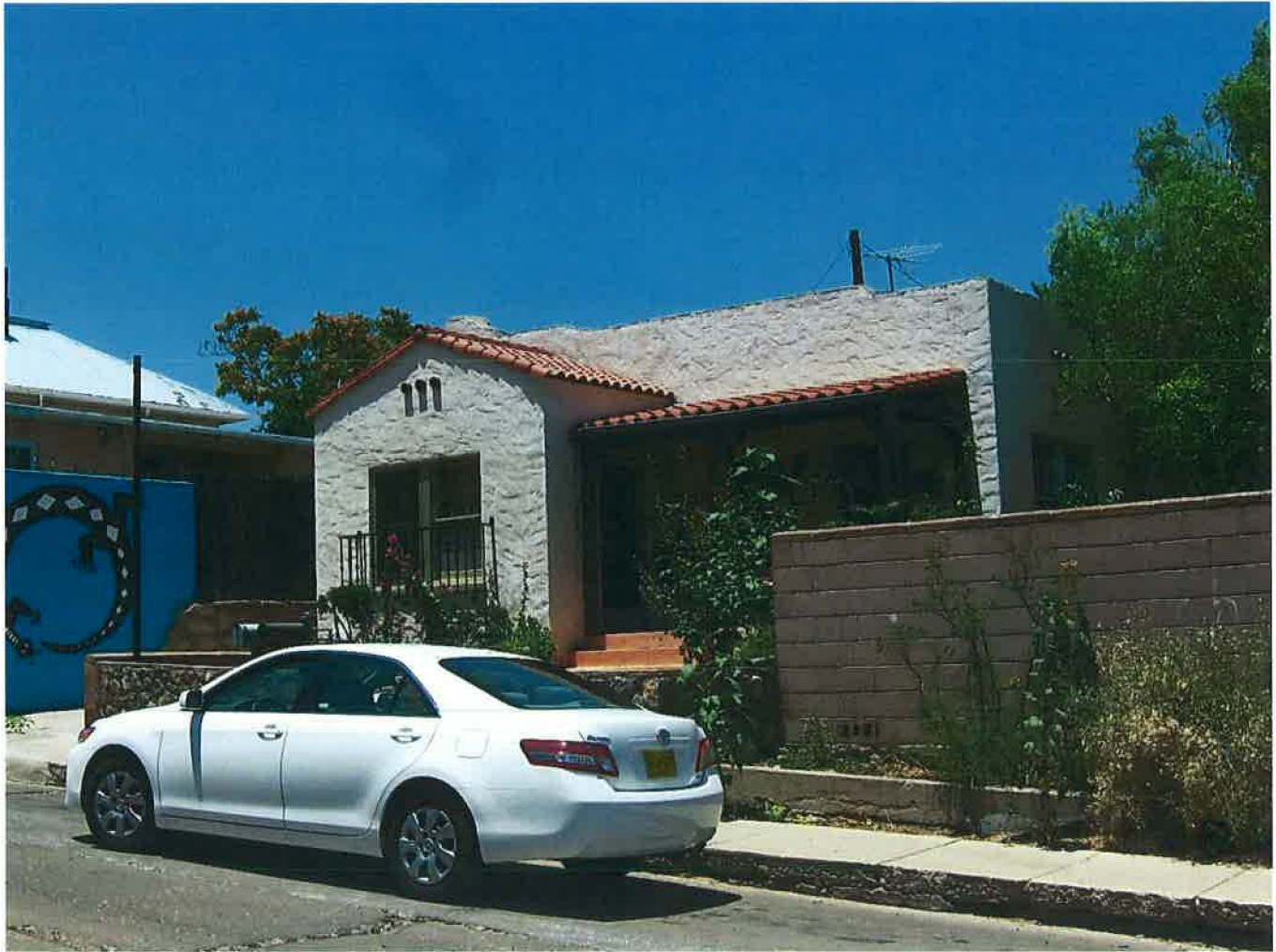
23 of 24 Dr. Frazin Office, 204 West Market, South (front) elevation; looking north
