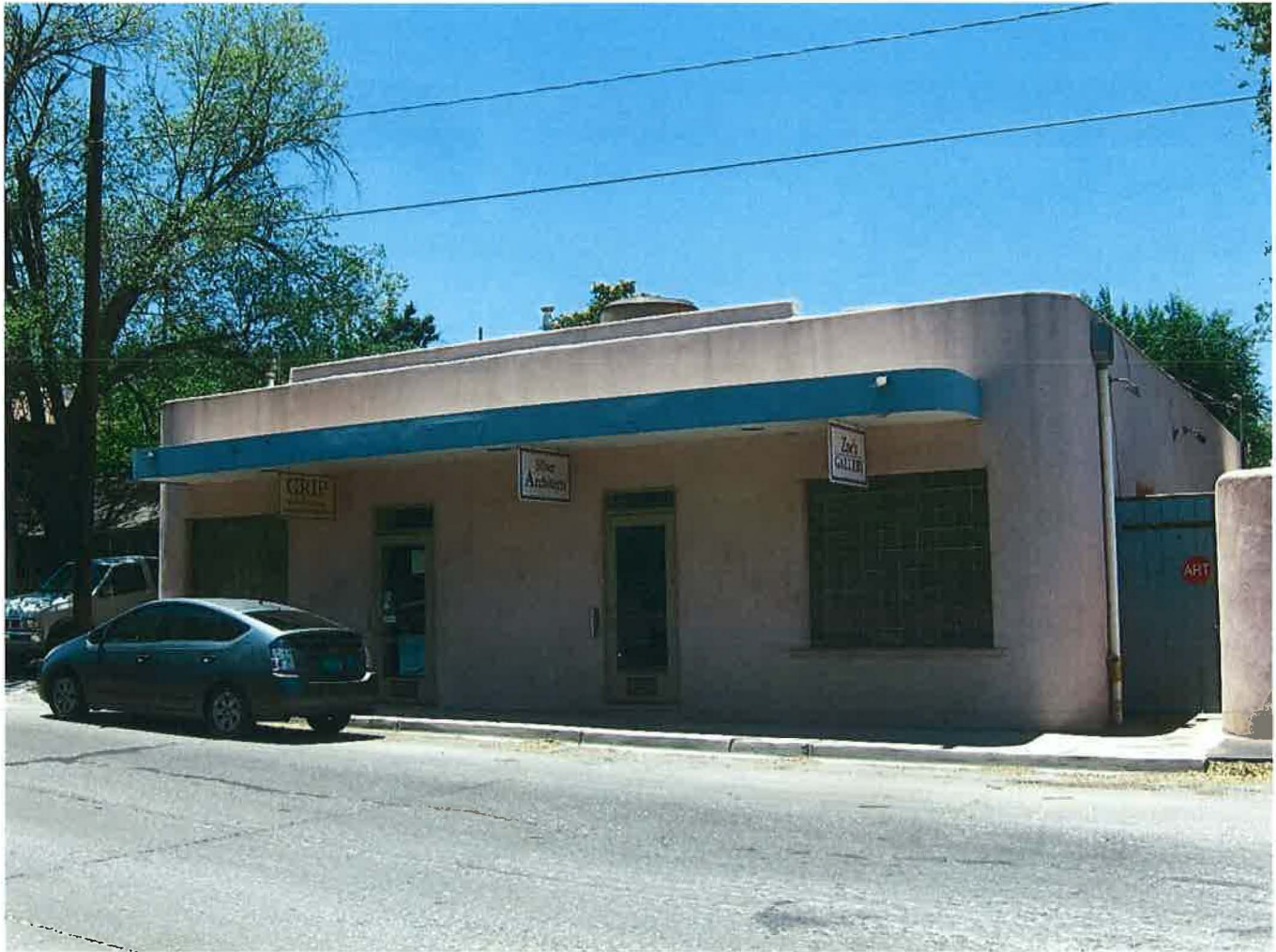
21 of 24 Food Locker Plant, 305 North Cooper Street, East (front) elevation; looking west
