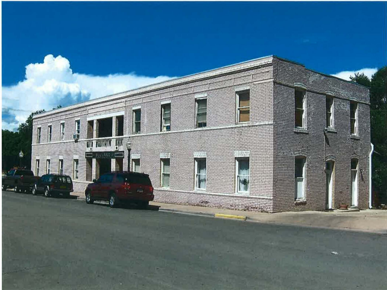
6 of 24 Bullard Hotel, 105 South Bullard, West (front) and north elevations; looking southeast (2010)
