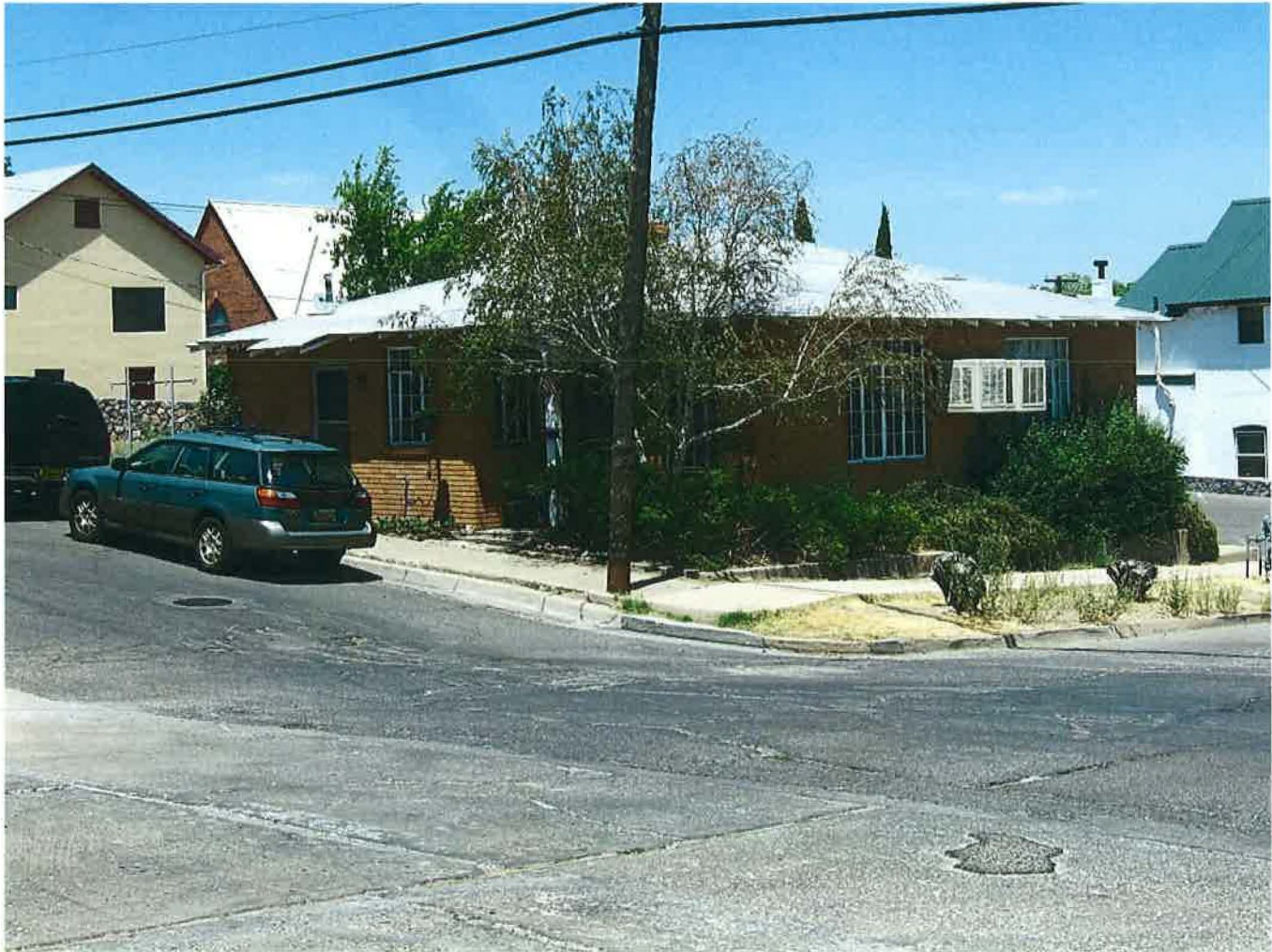
11 of 24 Duplex, 602 North Arizona Street, West and south elevations; looking northeast
