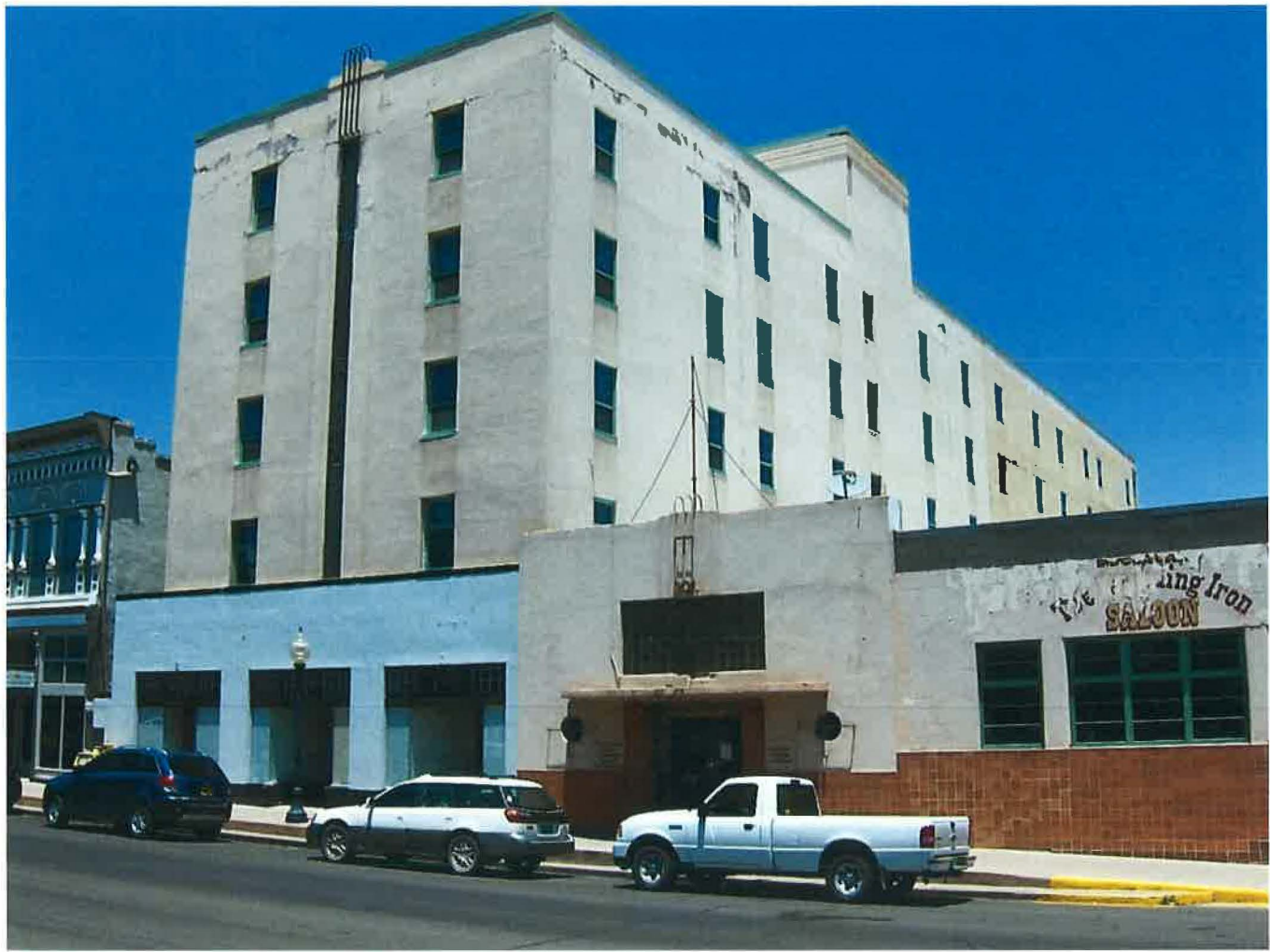
13 of 24 Murray Hotel, 200-206 West Broadway, South (front) and east elevations; looking northwest
