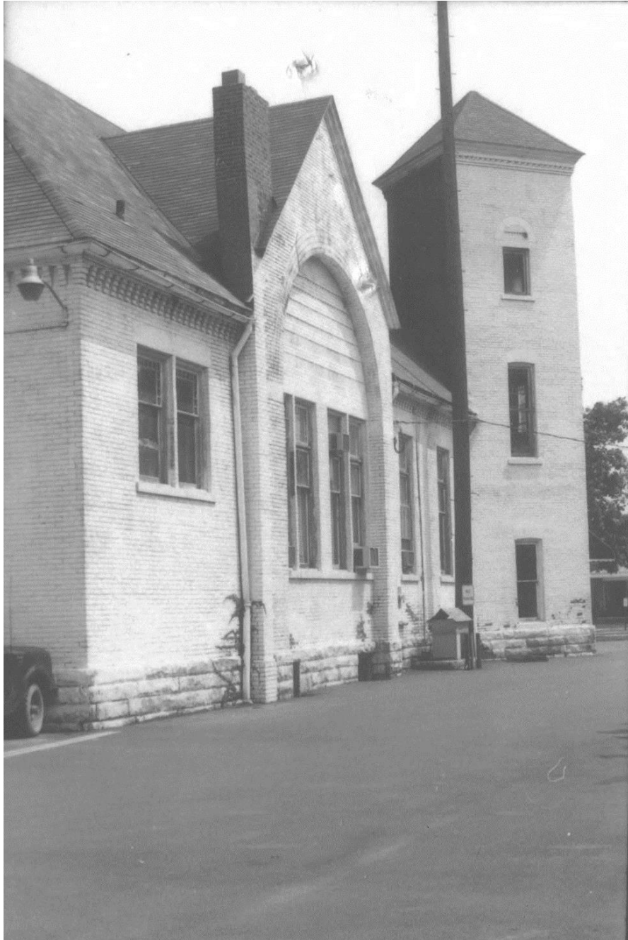
Figure 7: Mentor City Hall, 1972, Old Mentor Foundation survey, west elevation. Lake County Historical Society
