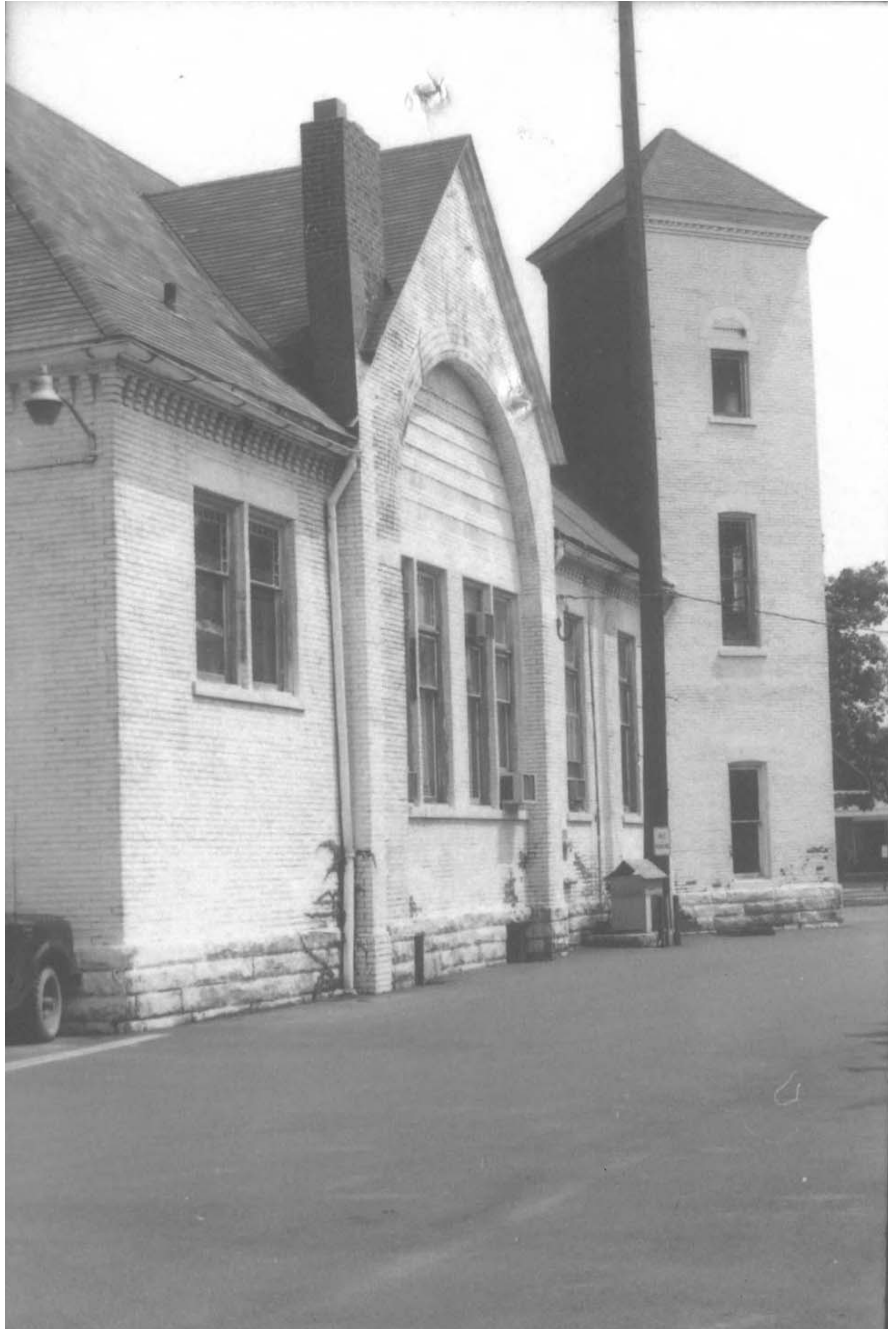
Figure 7: Mentor City Hall, 1972, Old Mentor Foundation survey, west elevation. Lake County Historical Society
