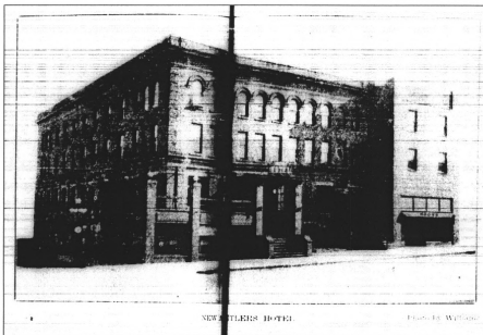
Figure 10: The newly-completed annex ( Spirit Lake Beacon , November 13, 1930)
