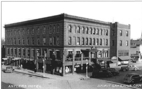
Figure 3: Antlers Hotel, c.1950, view southeast (note how the basement-level west storefronts were advanced south between the rebuilt veranda and the 1930 south addition) ( www.pbase.com/luckybreak/okoboji.jpg )
