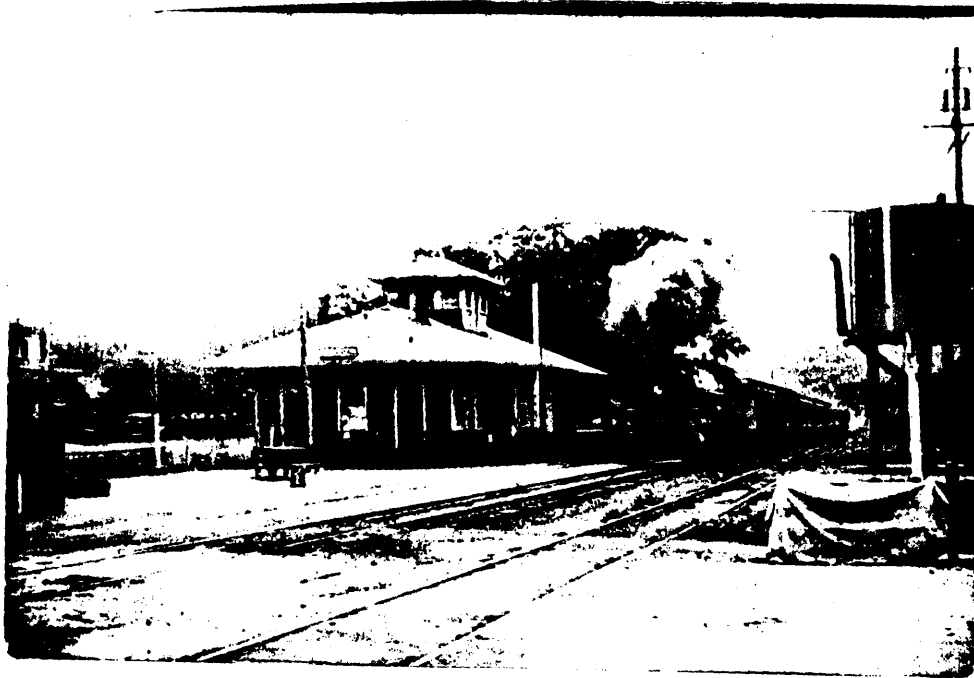
Print of Southern Depot at Leeds about 1930 showing west and south sides with platform and cupola. Present depot to be restored like picture.
