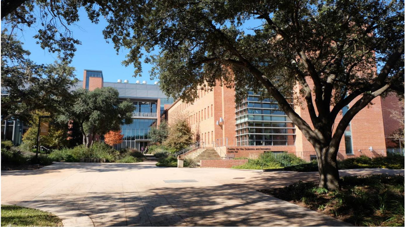
Photo 64. The Center for the Sciences and Innovation (looking west)
