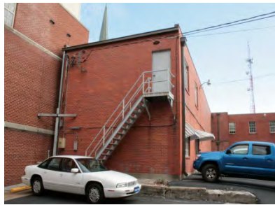
Back of the Building Photo 8
