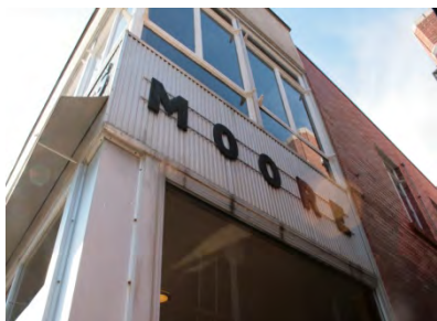
Right Exterior Wall (photo 5)
