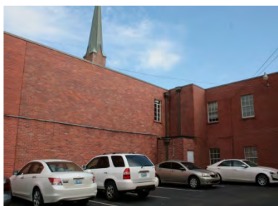
Back of the Building Photo 7
