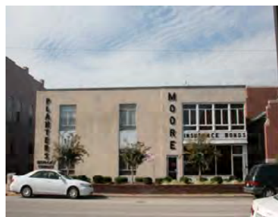
Street Facing Facade (Photo 3)
