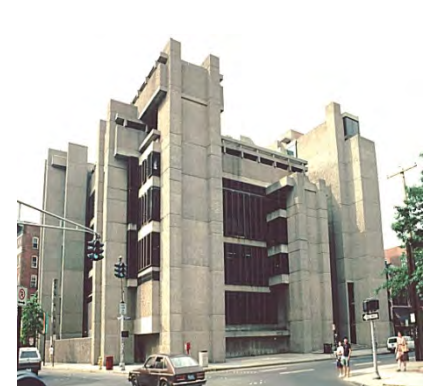
Yale Art and Architecture Bldg.
