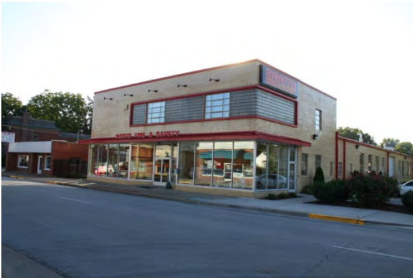
Gallaway Farm Equipment Building (1948)
