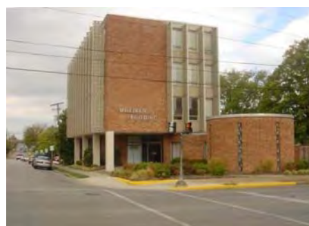
Milliken Building (1963) Photo 12
