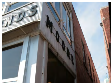
Right Exterior Wall (photo 6)
