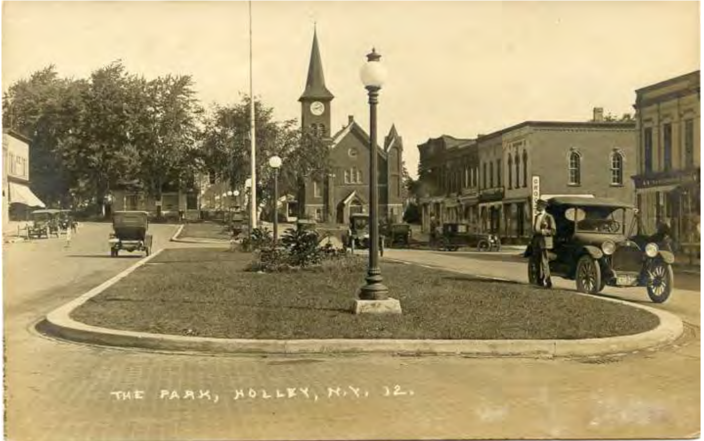
View looking north at Public Square (ca. 1914) This image shows the new brick paving installed at the square in 1913-14.
