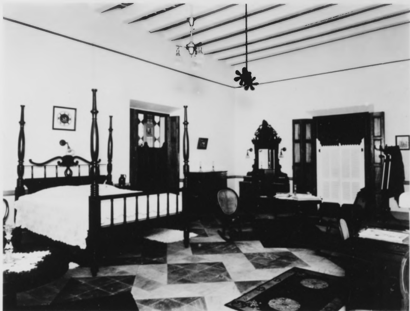
Bedroom in La Fortaleza showing type of ceiling construction being replaced with reinforced concrete
