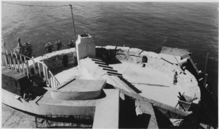
Top of NW tower showing in the parapet loopholes for both bow and arrow and harquebus
