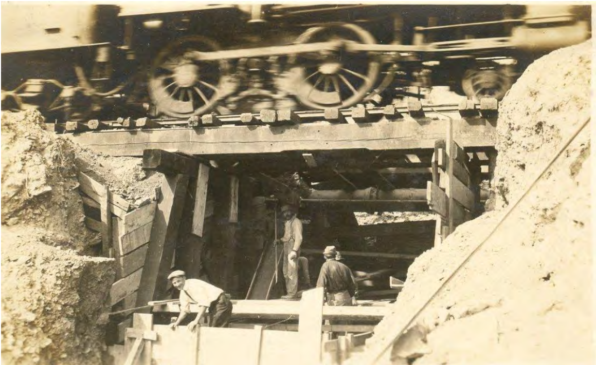
Figure 13. Circulating water pipe trench below train trestle, June 1913. Photo courtesy of Robert Abbott.
