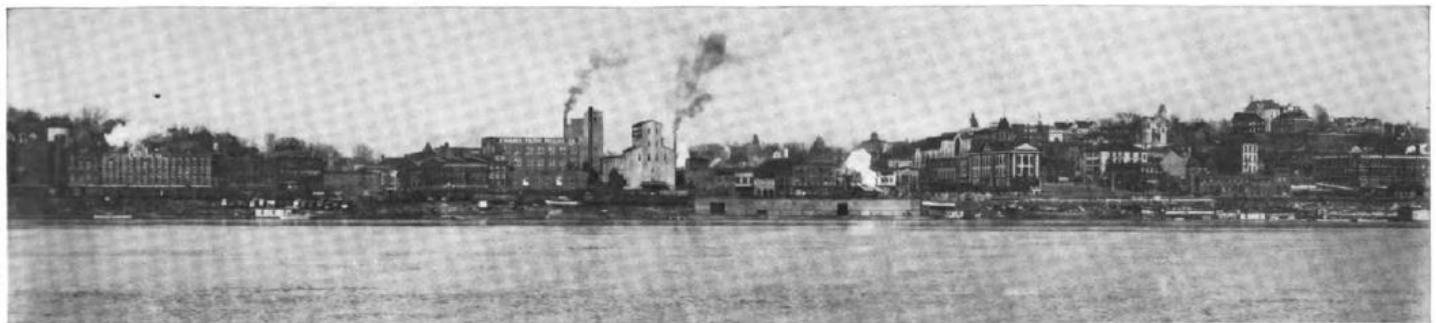
A HALF MILE OF THE PRESENT ALTON WATER FRONT.
