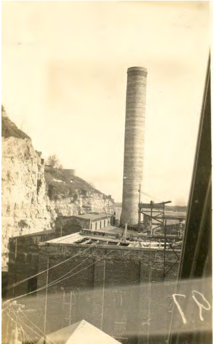
Figure 6. Power House and Transformer House, November 1913, view is southeast. Note smoke stack which was one of the first components constructed. Photo courtesy of Robert Abbott.
