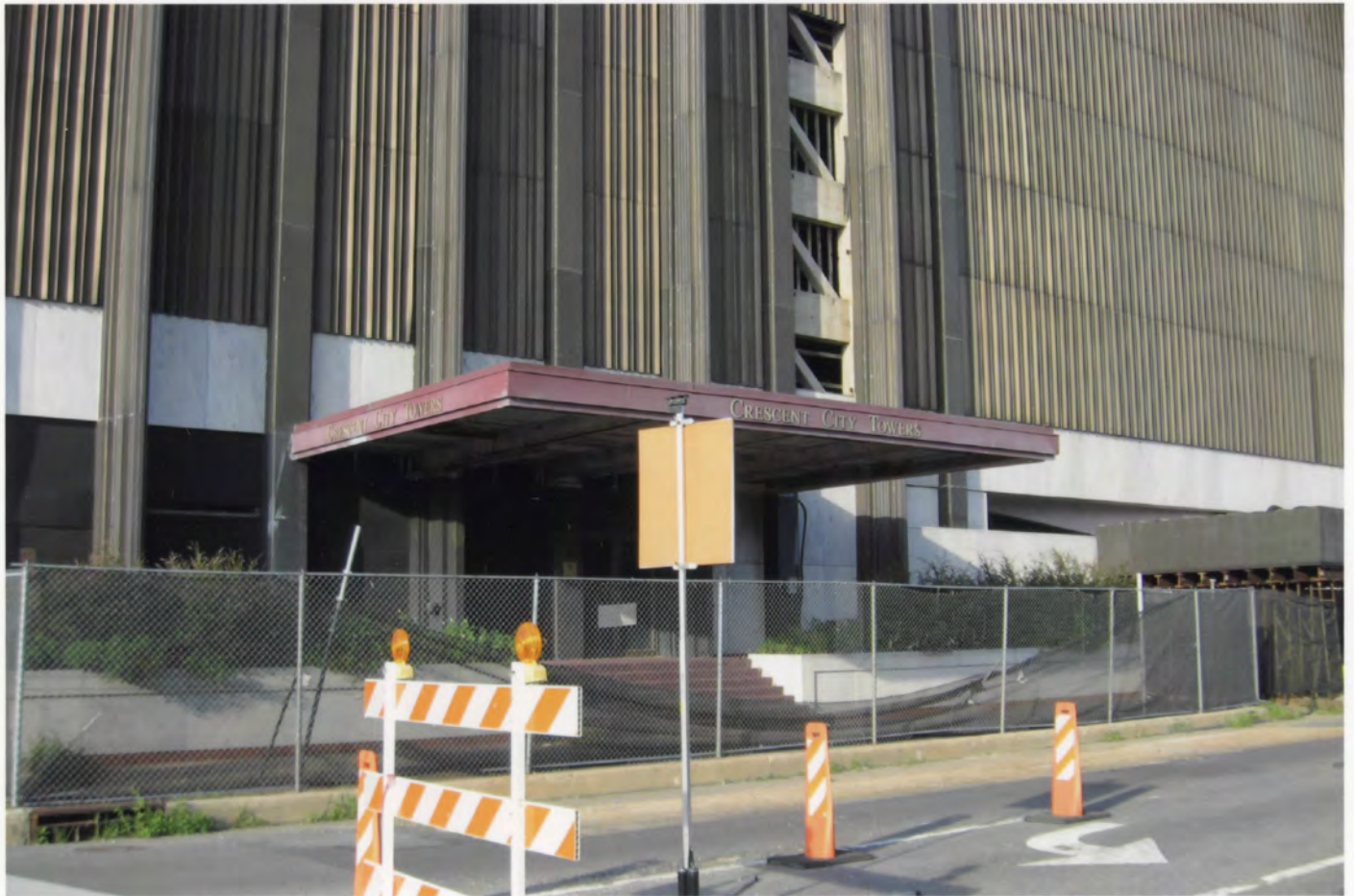
Plaza Tower New Orleans, Orleans Parish, LA Mary Lane Carleton June 13, 2012
