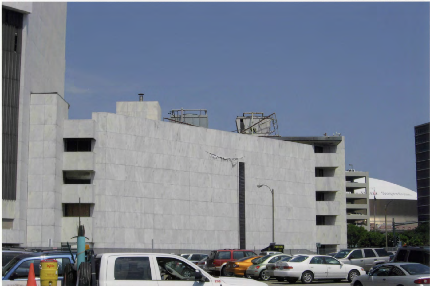
Plaza Tower New Orleans, Orleans Parish, LA Mary Lane Carleton June 14, 2012
