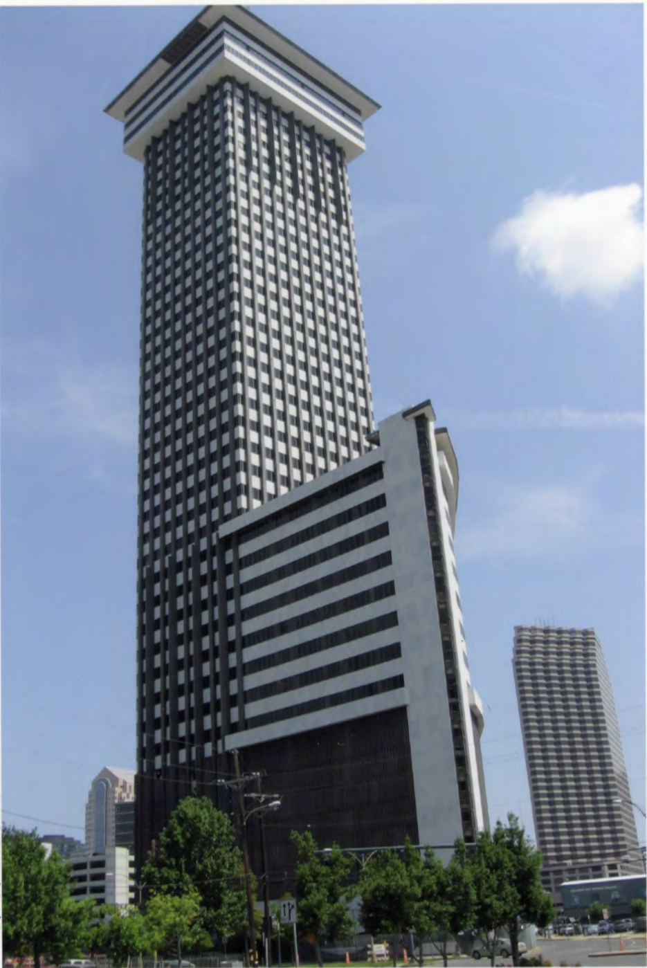
Plaza Tower New Orleans, Orleans Parish, LA Mary Lane Carleton June 14, 2012
