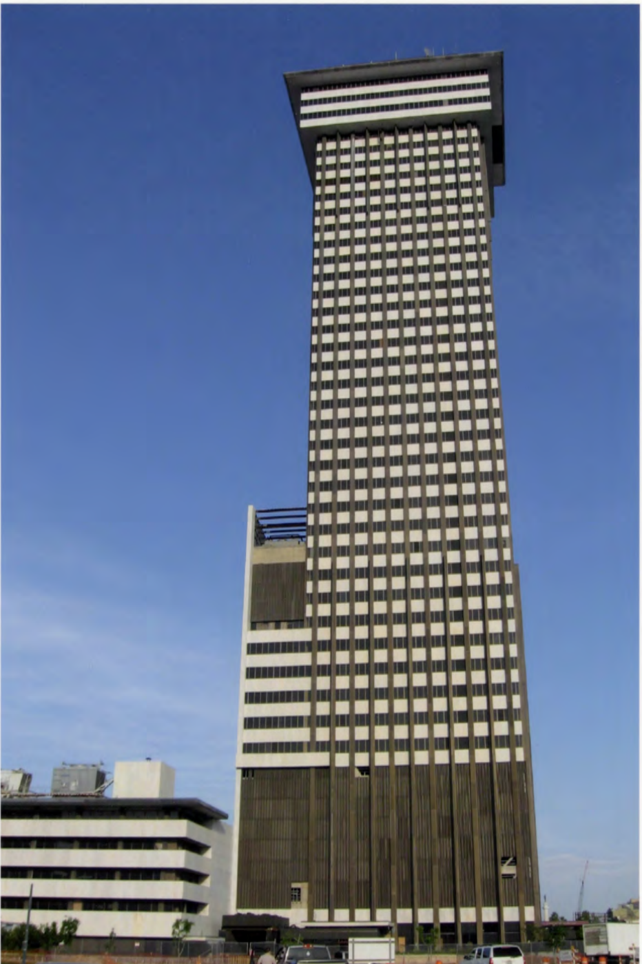
Plaza Tower New Orleans, Orleans Parish, LA Mary Lane Carleton June 13, 2012
