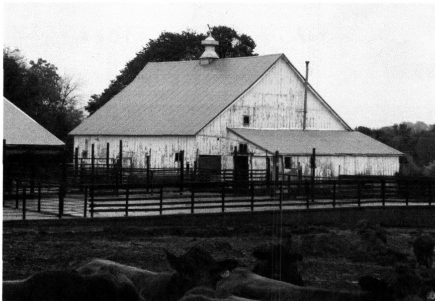
Figure 18 Large barn (#3), south gable and west long side, looking northeast over the feed lot. Tallgrass Historians L.C., 2008
