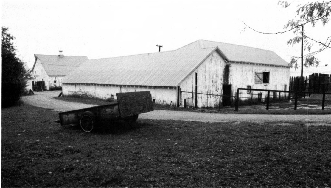
Figure 25 The horse barn's (#6) location (here looking to the southeast at its north and west sides) in the center of the farmstead has become awkward, necessitating a dangerous curve and exposing drivers and pedestrians to blind spots. This position suggests it was once the western edge of farmstead, early in the twentieth century, and is an indicator of a once compact farmstead. Roswell Garst and his descendants' agricultural pursuits expanded the farmstead well beyond the horse barn by mid-century. Tallgrass Historians L.C., 2008
