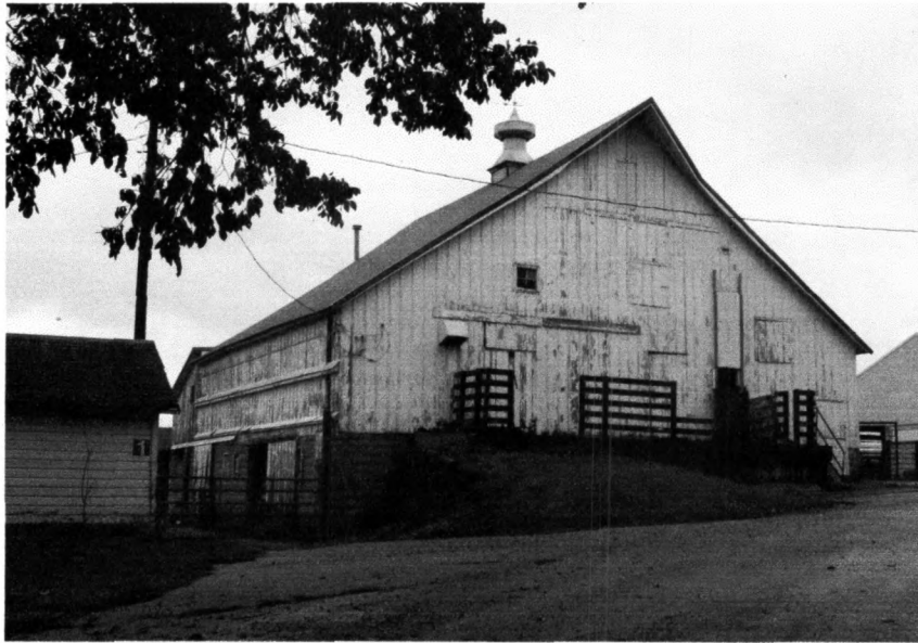
Figure 17 Large barn (#3), north gable end and east long side, looking southwest. Also visible on the left is a small outbuilding (#4). Tallgrass Historians L.C., 2008
