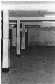
Figure 5: Basement columns and beams, view west (Jacobsen, 2006)
