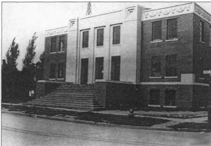
Figure 10: Original façade and entryway, 1938, view southwest, note the antenna base and the absence of a flag pole (1938 Iowa National Guard Historical Annual, p. 149).
