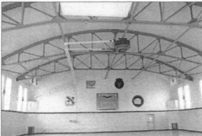
Figure 7: Drill hall interior, view west, c. 1999 (Photo, Iowa National Guard)
