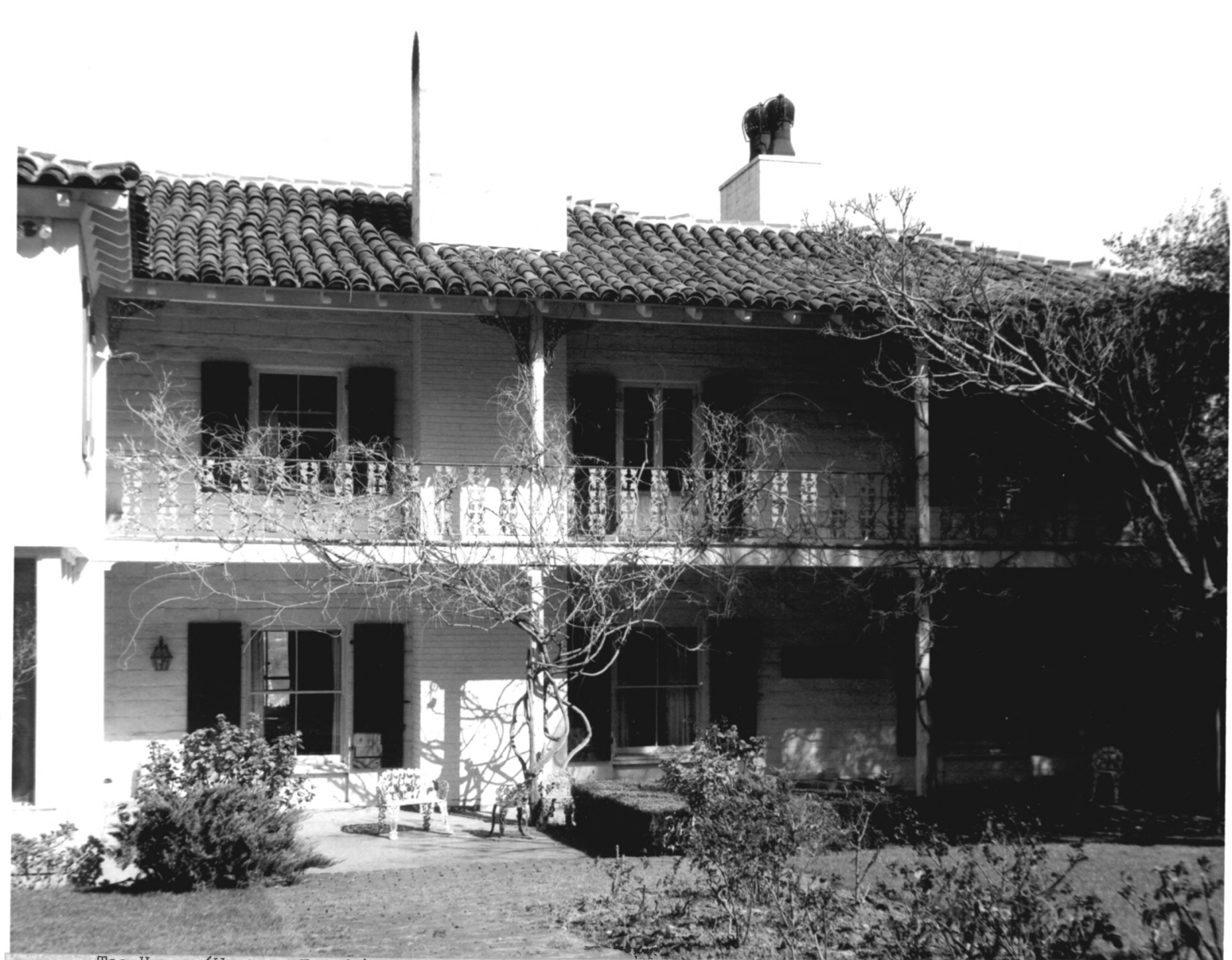
Tao House (Western Facade) near Danville, California
