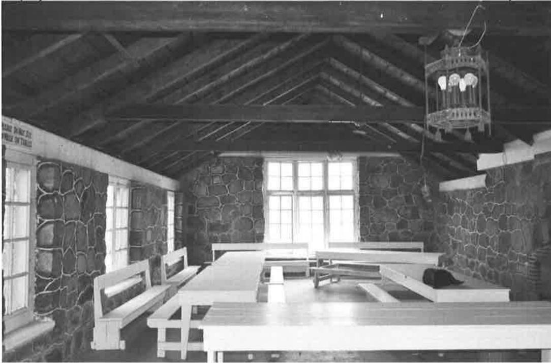
(Image 15) Interior of Stone Shelter House showing original light fixture, open beamed ceiling, original windows and stone interior.
