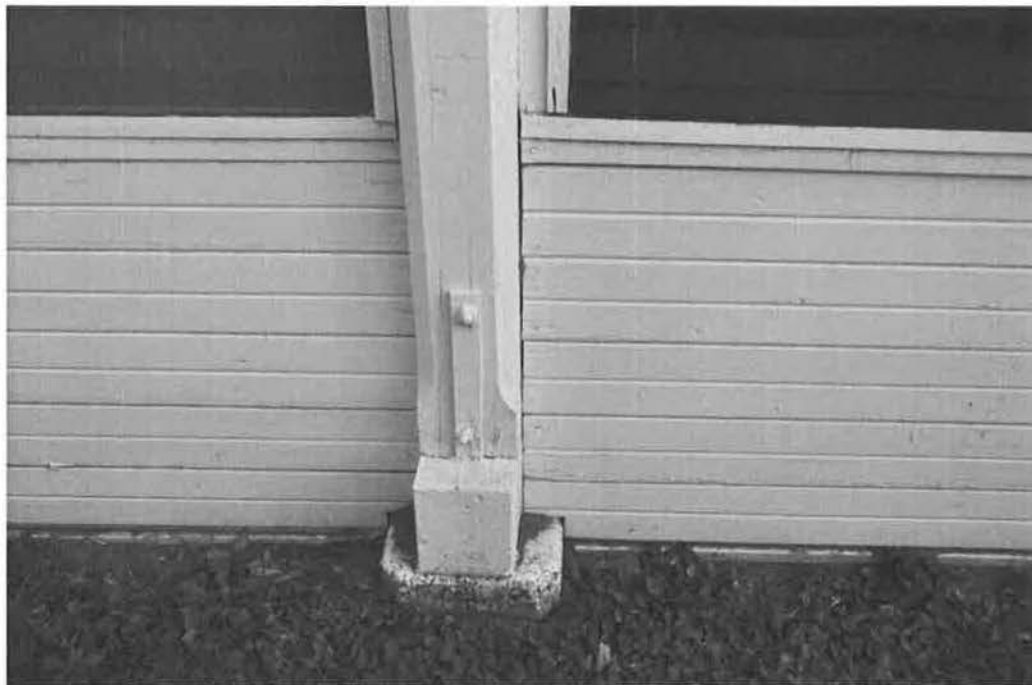
(Image 3) Wood support beams on concrete footings support the Auditorium's structure.
