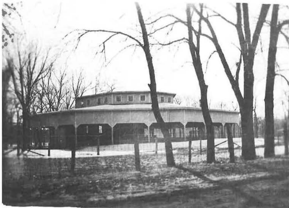
(Image 28) 1912 Photograph shows the majestic structure and open sides.
