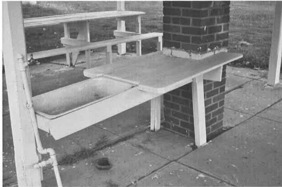
(Image 17) Close-up of original sink and counter next to brick chimney in fish cleaning shelter. The wood-burning stove that once was in shelter is gone.
