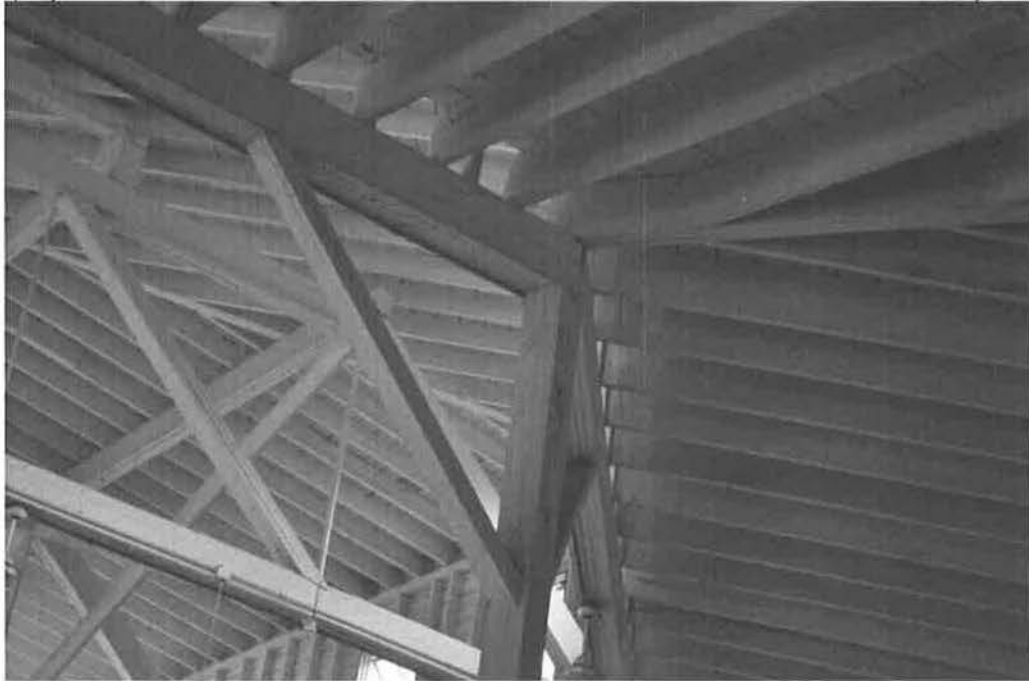
(Image 5) Another view of exposed beams in the Chautauqua Auditorium.
