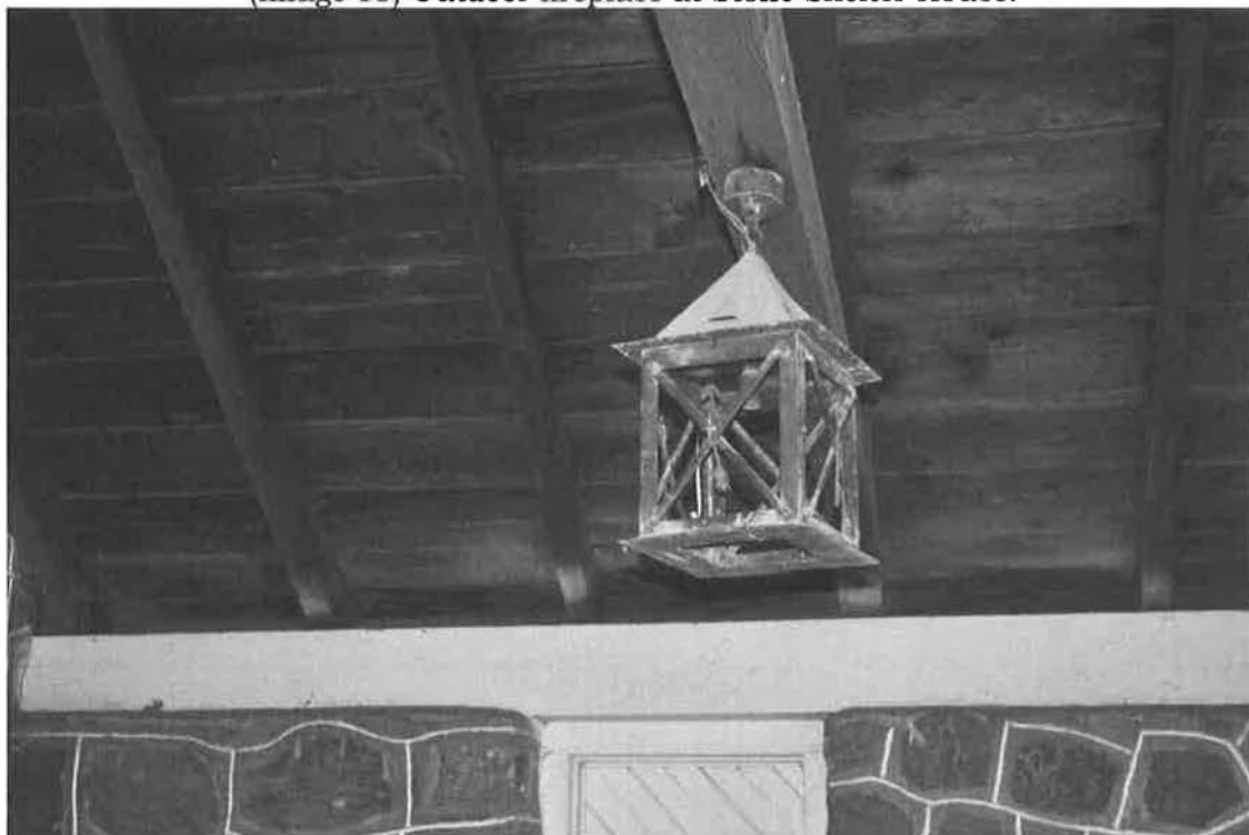
(Image 14) Open beam ceiling and original light fixture in open area of Stone Shelter House.
