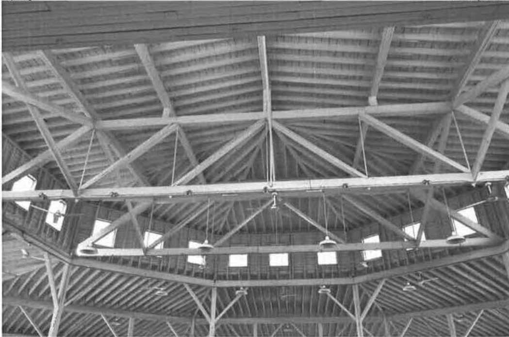
(Image 7) Performers' view looking at ceiling and upper ventilation windows.
