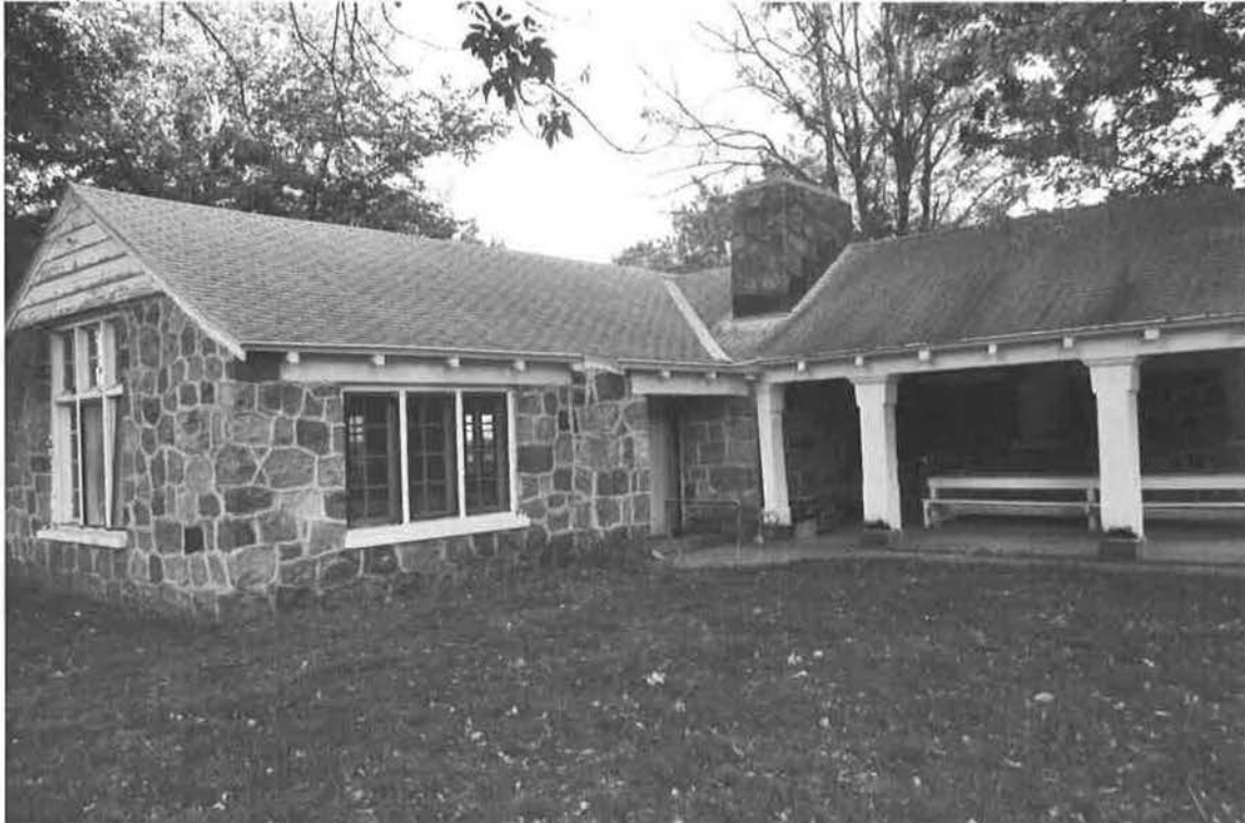
(Image 11) Stone Shelter House today. Note some water damage on the wood pillars. Stone work is in good condition.
