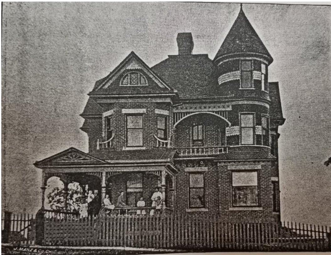
Figure 2: George E. Dovey House; West Elevation, c1892 (owner's private collection).
