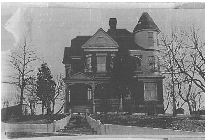
Figure 3: George E. Dovey House, West Elevation. c1915 (owner's private collection).
