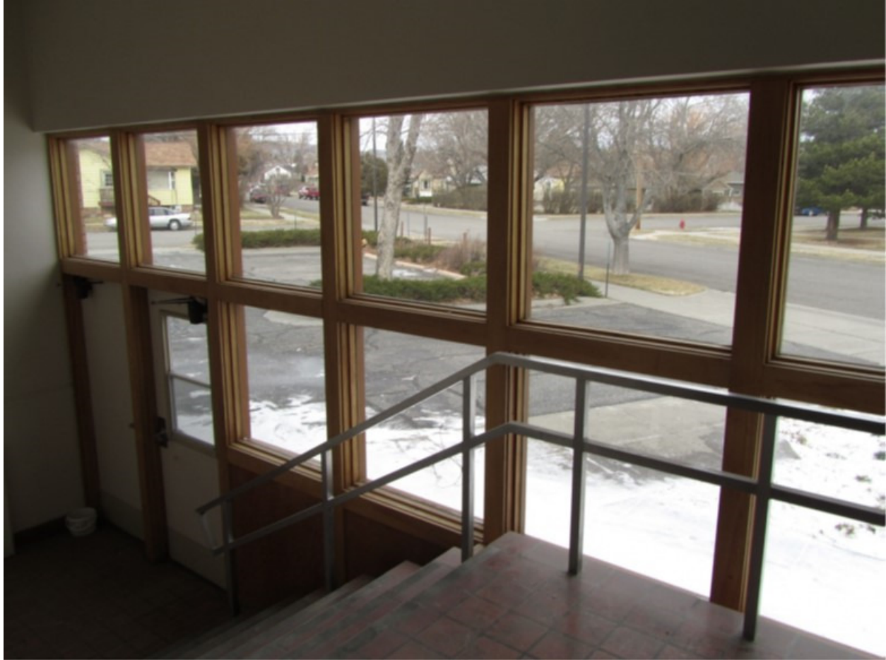
Photo 48: Administrative Corridor, Main Entrance Foyer, Aspect: N
