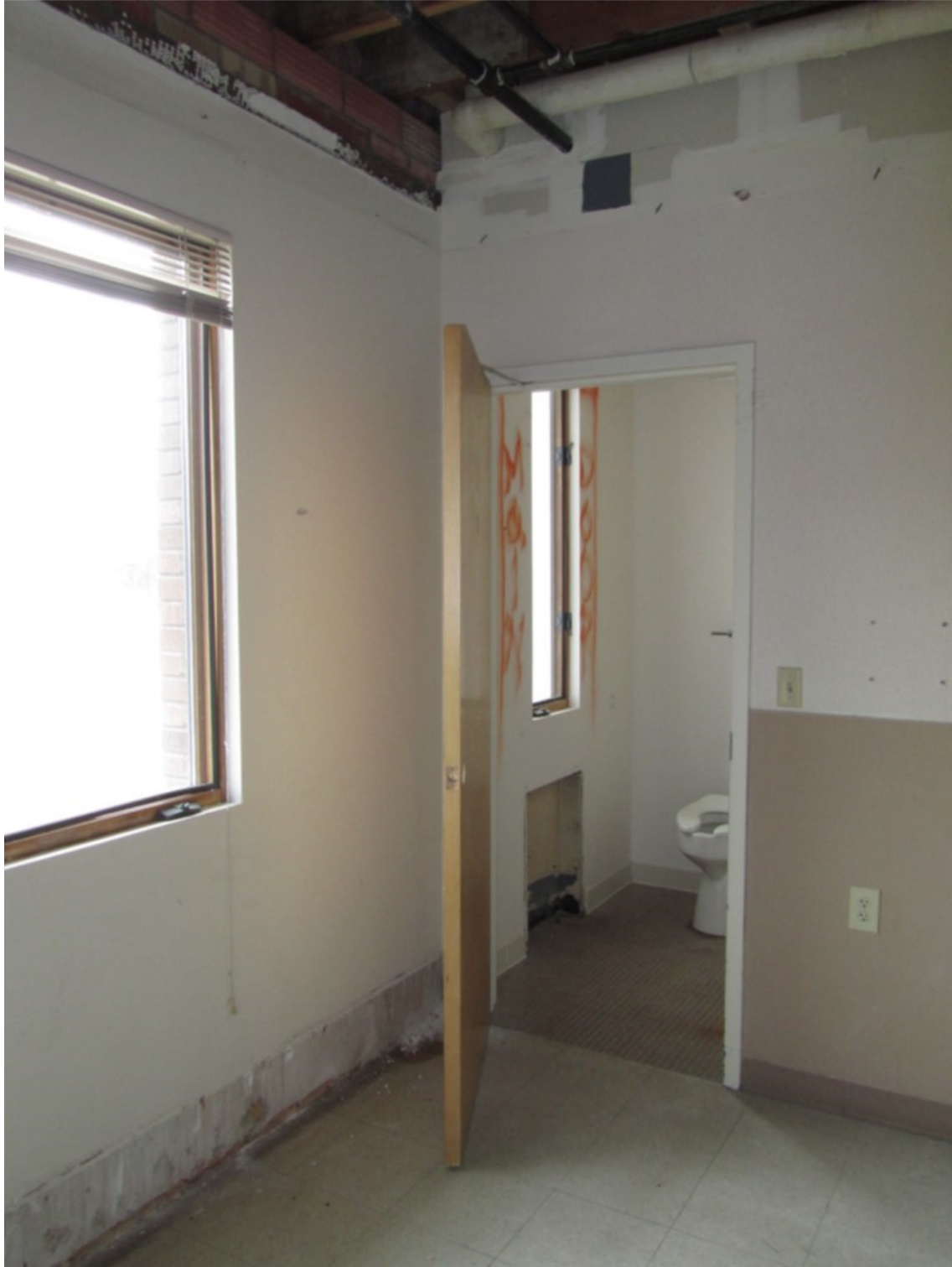
Photo 70: Nursing Corridor, Patient Room, Aspect: S
