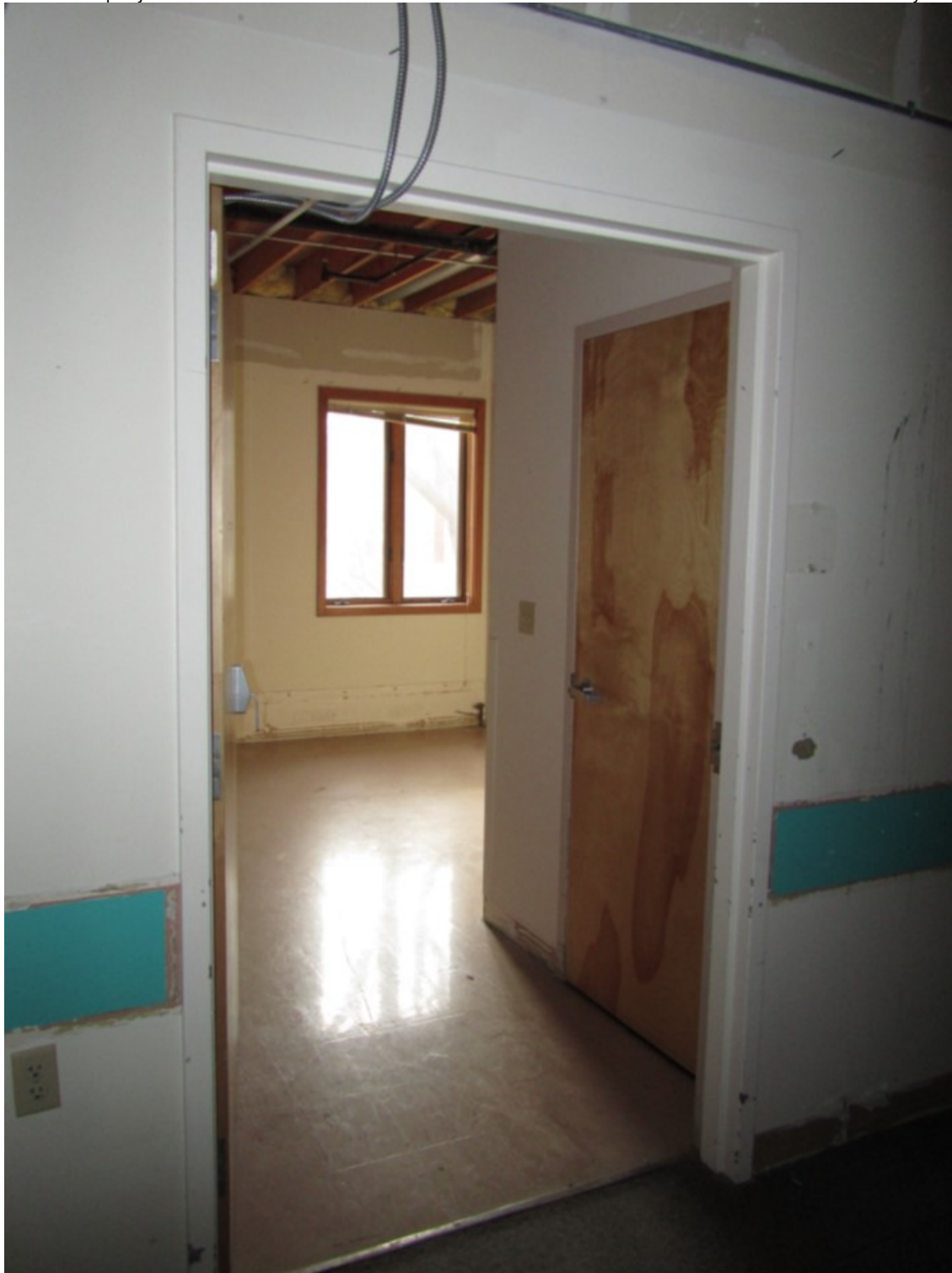
Photo 60: Rooms Addition Corridor, Patient Room, Aspect: W
