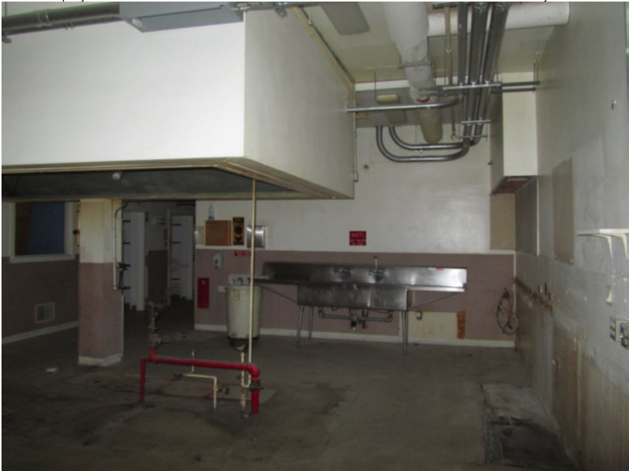
Photo 78: Basement, Primary Corridor (SW side), Cafeteria, Aspect: W
