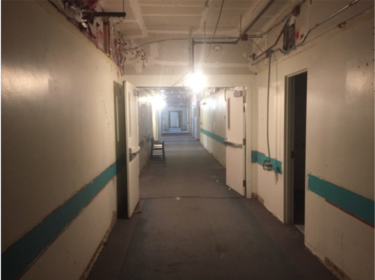
Photo 32: Primary Corridor, Hospital Core, Aspect: NE
