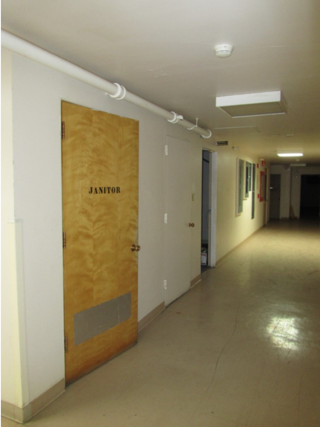
Photo 73: Basement, Main Corridor, Aspect: SW
