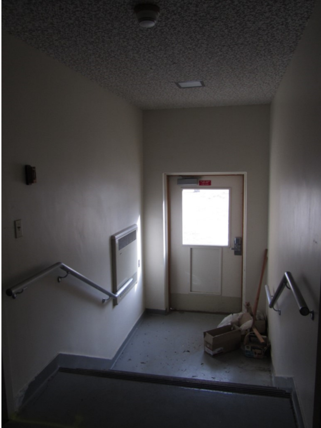
Photo 71: Nursing Corridor Entrance, Aspect: SE
