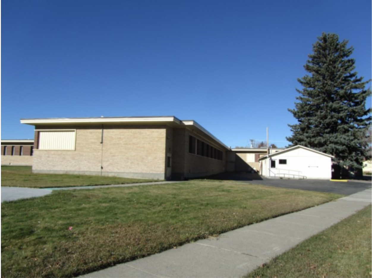
Photo 08. SE Elevation of Pediatric Wing (foreground), Aspect: NW
