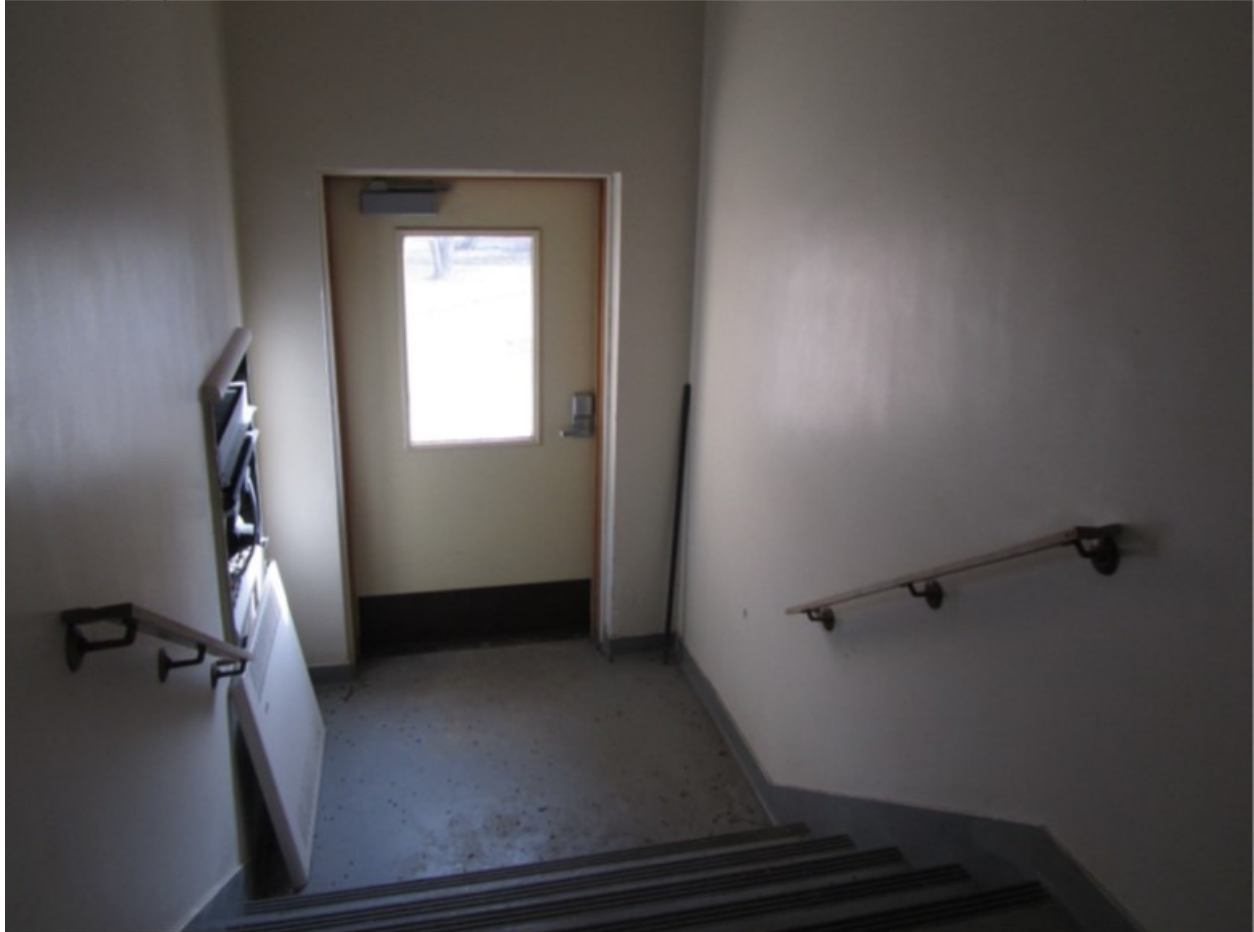
Photo 65: Maternity Corridor Entrance, Aspect: SE
