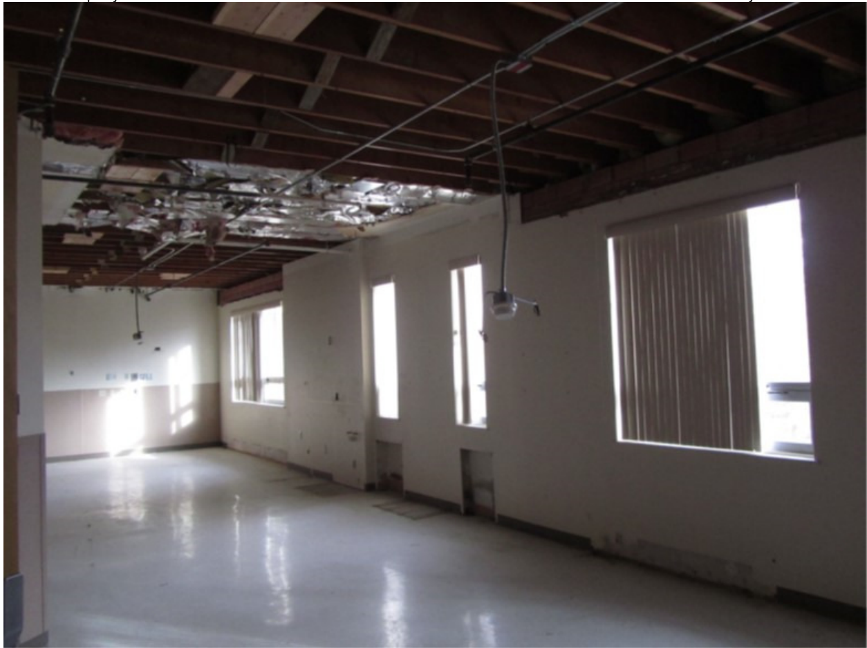
Photo 64: Maternity Corridor (SE side), Converted 4-Room Ward, Aspect: W
