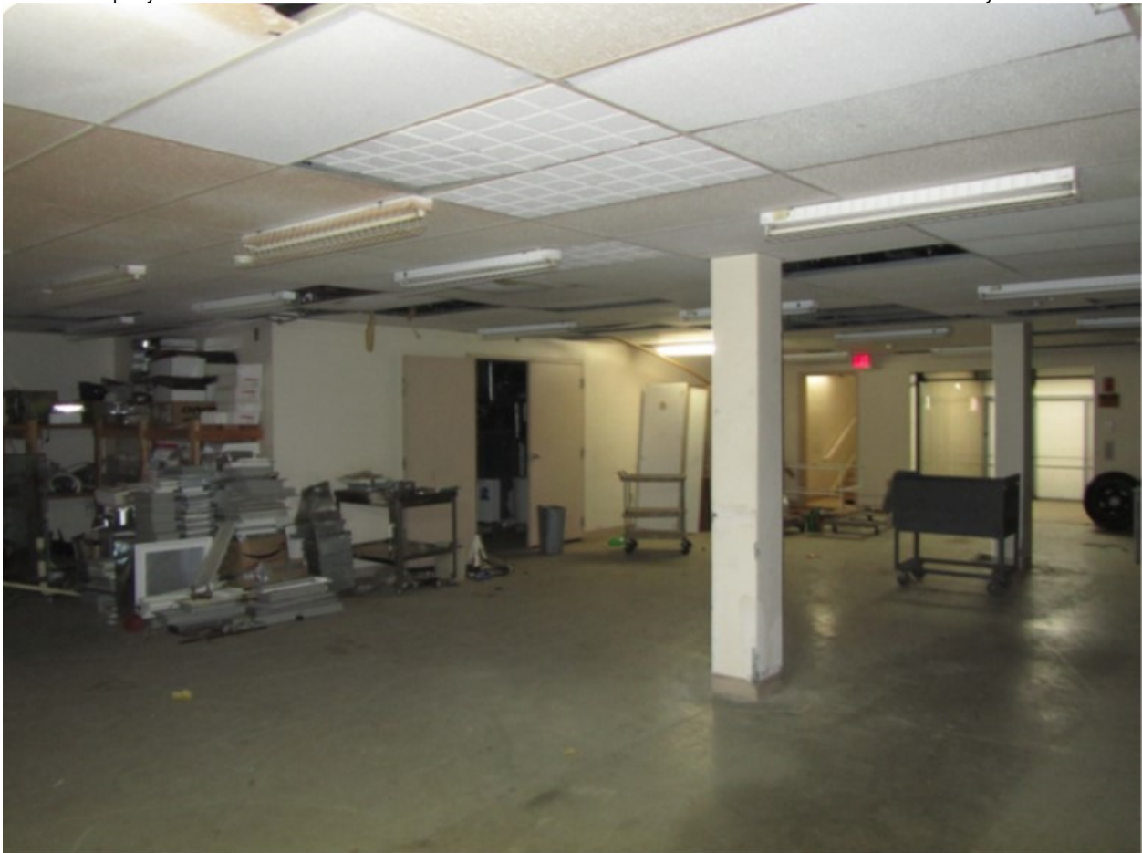
Photo 75: Basement, ER Addition, Aspect: N
