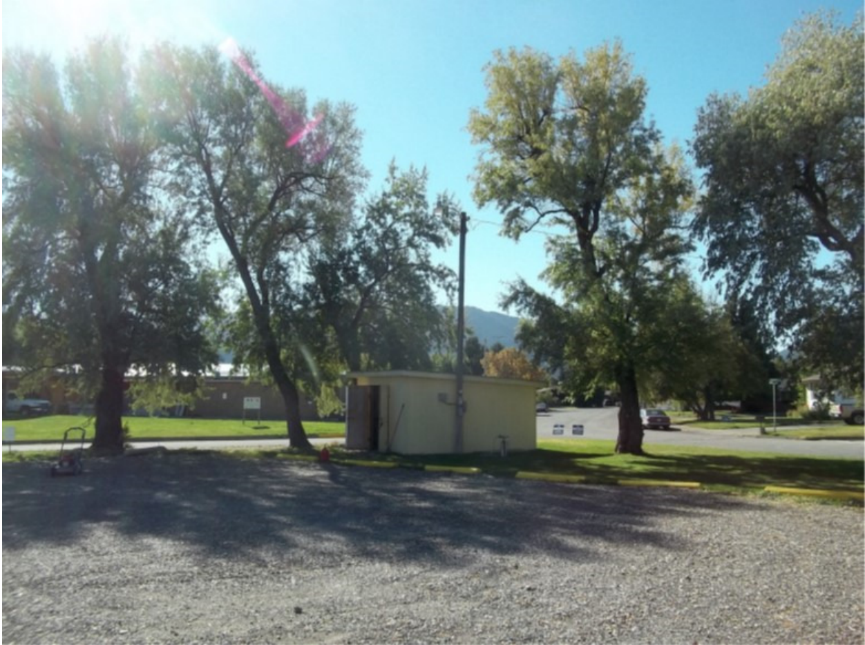
Photo 21: Groundskeeper Shed, Gravel Parking Lot and Cottonwood Trees, Aspect: SW
