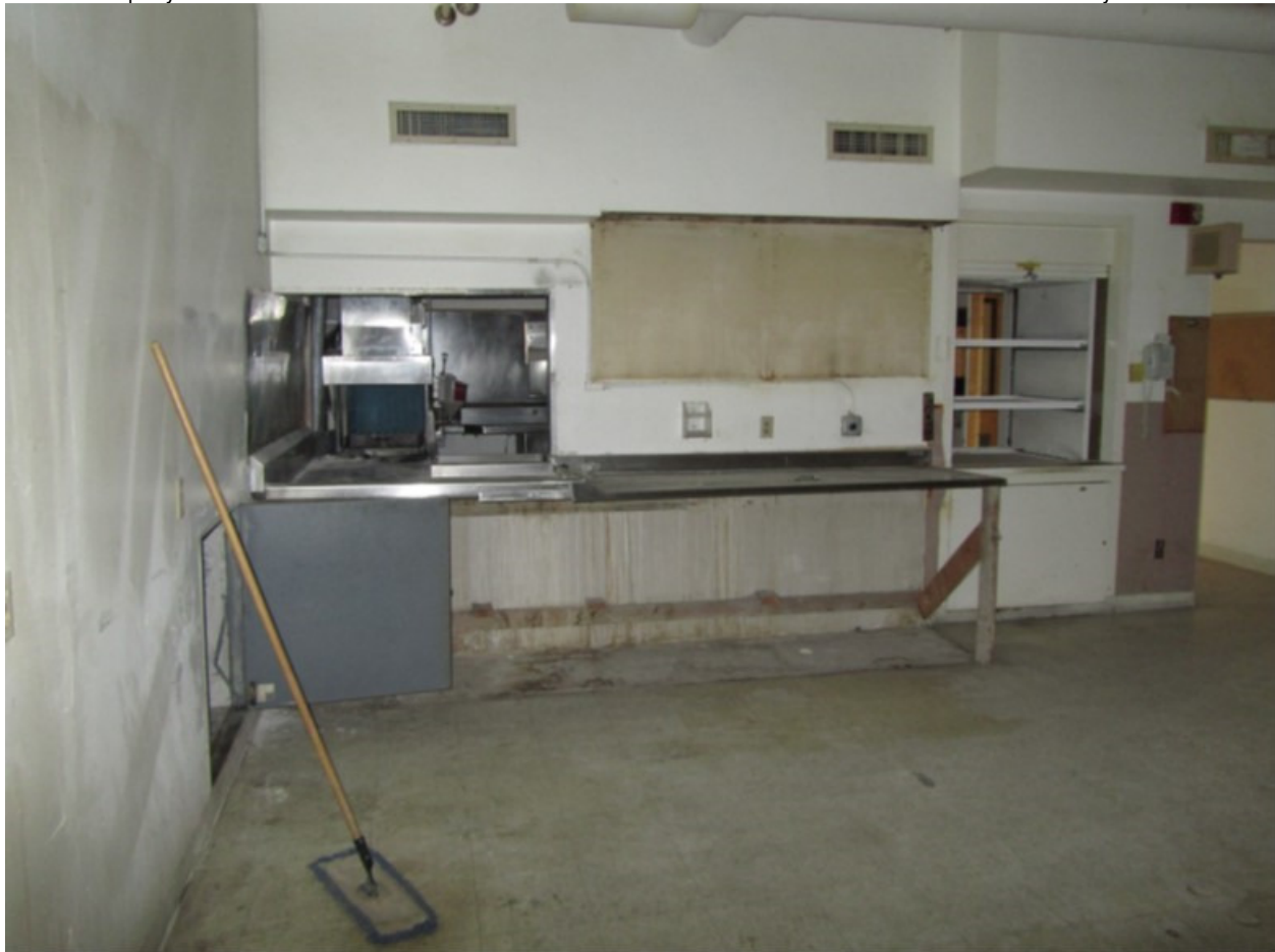
Photo 79: Basement, Primary Corridor (SW side), Cafeteria and Kitchen, Aspect: NW
