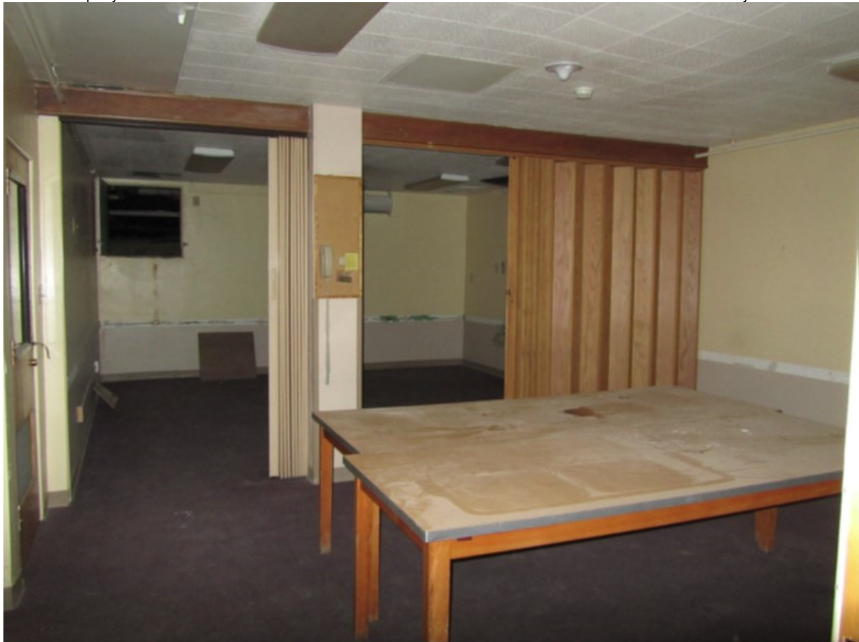
Photo 81: Basement, Primary Corridor (SW side), Lounge, Aspect: SW
