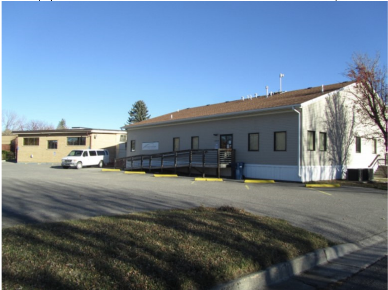
Photo 25: NW and SW Elevation of Mental Health Building and NW Elevation of Surgical Wing (background), Aspect: SE
