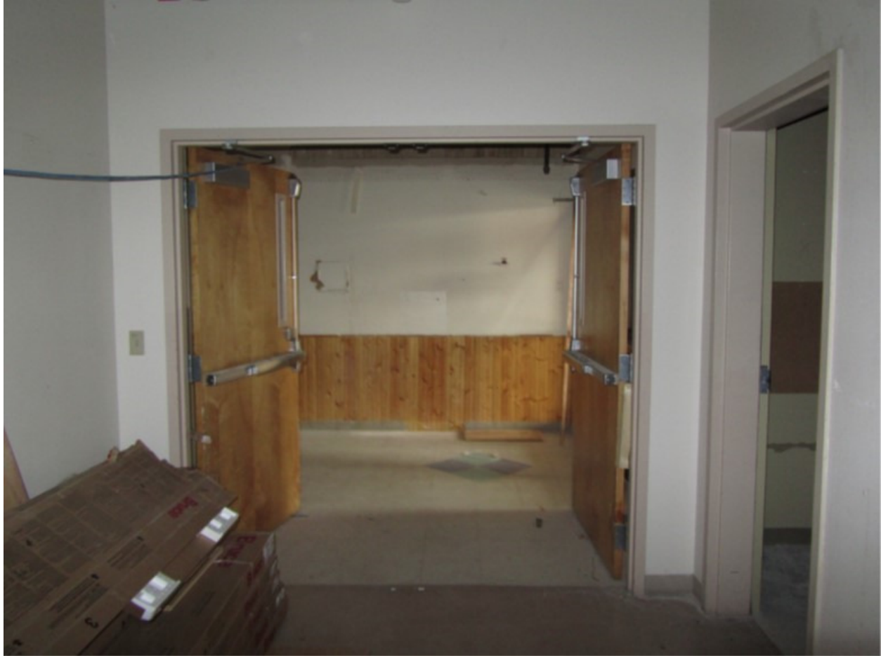
Photo 56: ER Addition, Main Entrance from Corridor, Aspect: SW
