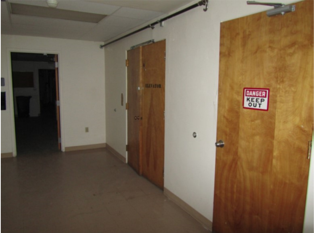
Photo 74: Basement, Administrative Wing, Secondary Corridor, Aspect: NE
