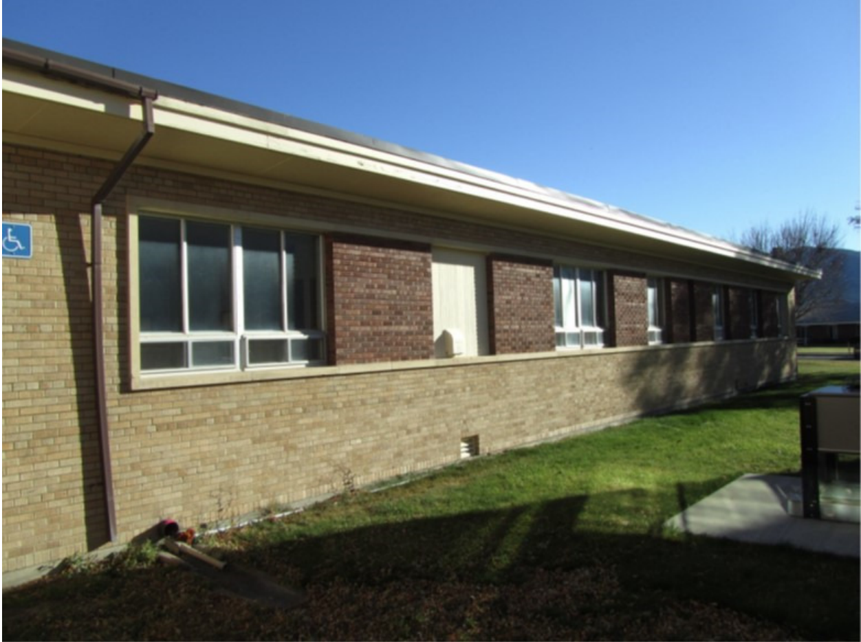
Photo 11. NW Elevation of Maternity Wing, Aspect: S
