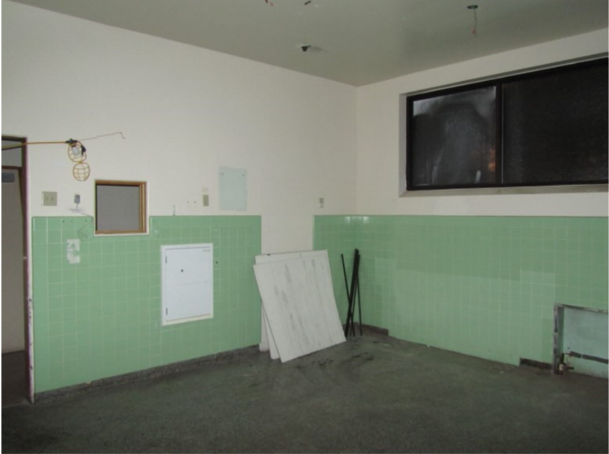
Photo 46: Primary Corridor, Surgical Wing, Delivery Room, Aspect: S
