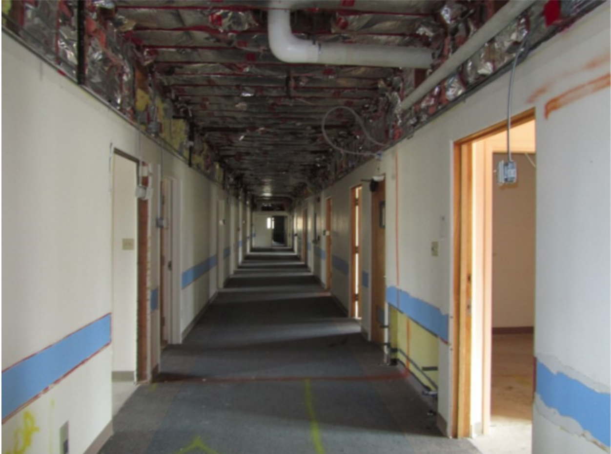
Photo 67: Nursing Corridor, Aspect: NE
