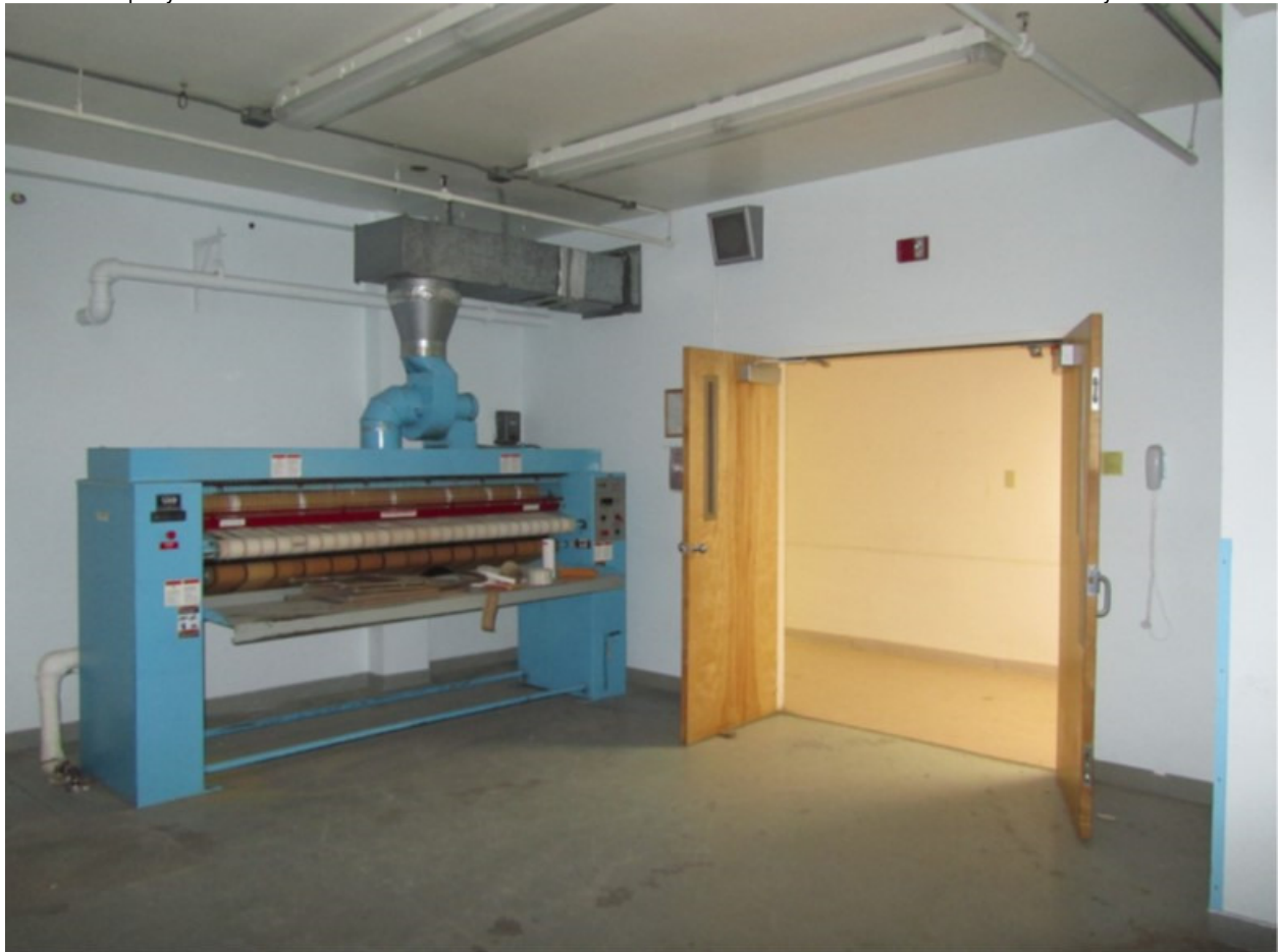
Photo 83: Basement, Primary Corridor (SW side), Laundry Room, Aspect: W
