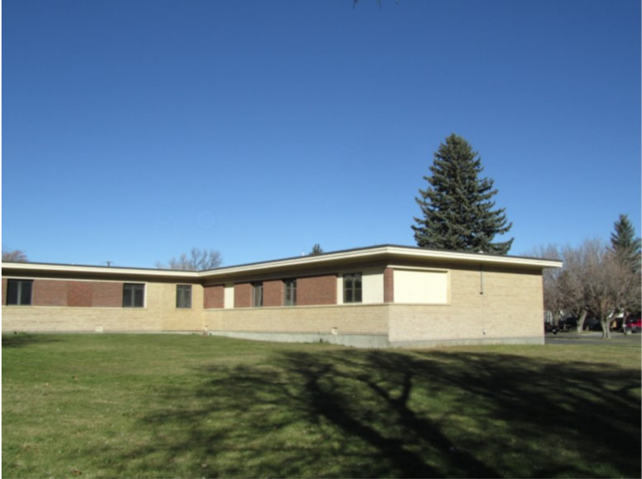
Photo 09. SE and SW Elevation of Pediatric Wing (right) and SE Elevation of Nursing Wing, Aspect: N
