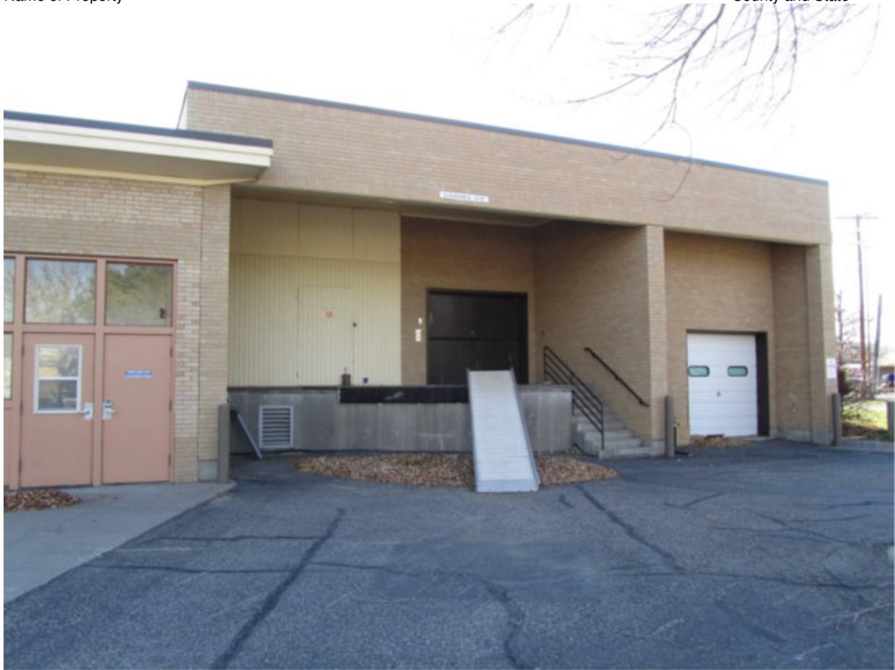
Photo 18: NE Elevation of ER Addition, Aspect: SW
