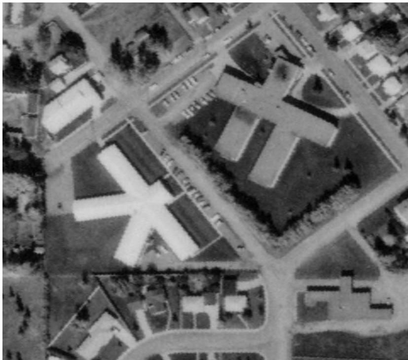
Aerial Views of Livingston Memorial Hospital, 1955 (top) and 1973 (bottom). Available at Montana Geographic Information Clearing House.
