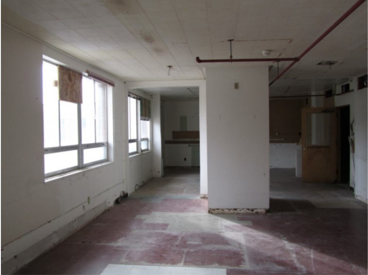
Photo 52: Administrative Corridor, Laboratory and Business Office (foreground), Aspect: SW
