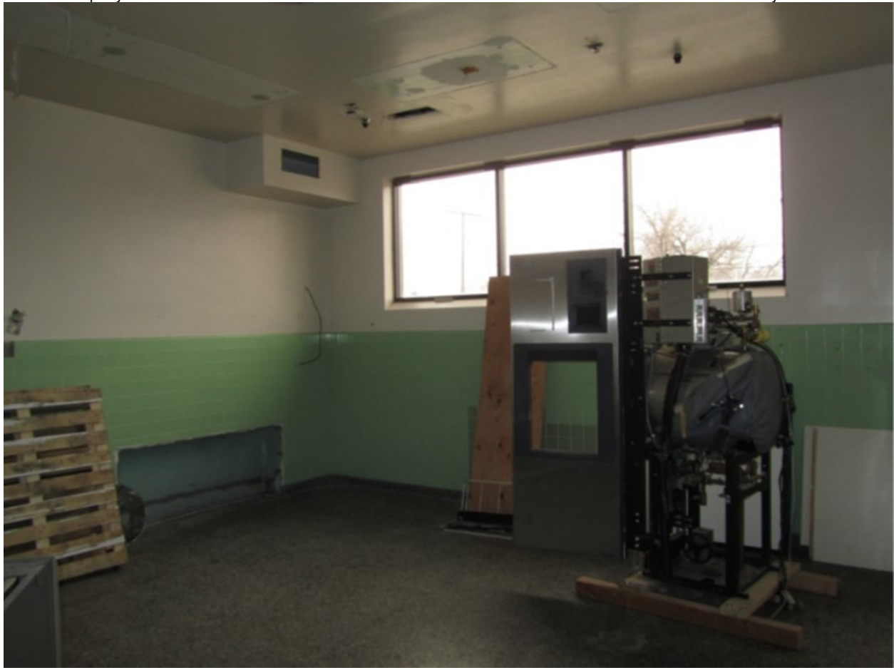
Photo 44: Primary Corridor, Surgical Wing, SW Operating Room, Aspect: W
