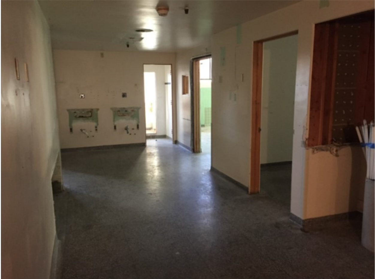
Photo 42: Primary Corridor, Surgical Wing, Aspect: NW
