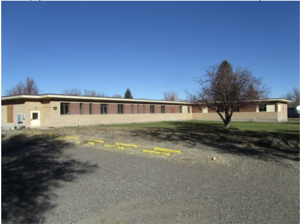
Photo 10. SE Elevation of Nursing Wing (left) and SW Elevation of Pediatric Wing, Aspect: NE
