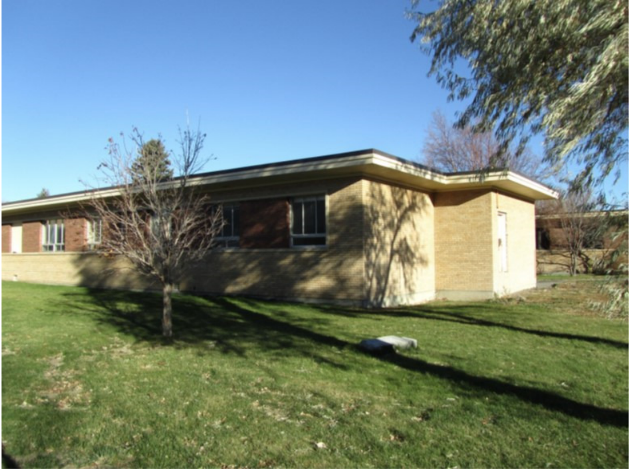
Photo 12. NW and SW Elevation of Maternity Wing, Aspect: E
