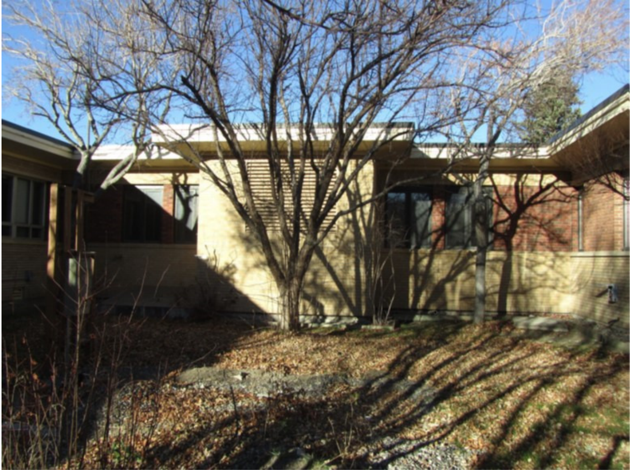
Photo 15. SW Elevation of Rooms Addition (courtyard interior), Aspect: NE
