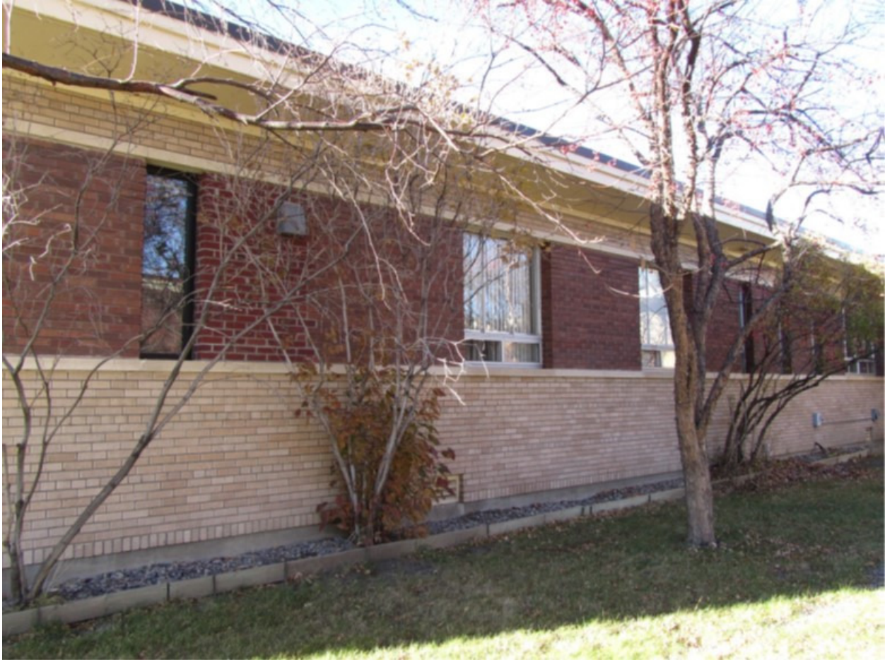
Photo 14. SE Elevation of Maternity Wing (courtyard interior), Aspect: N
