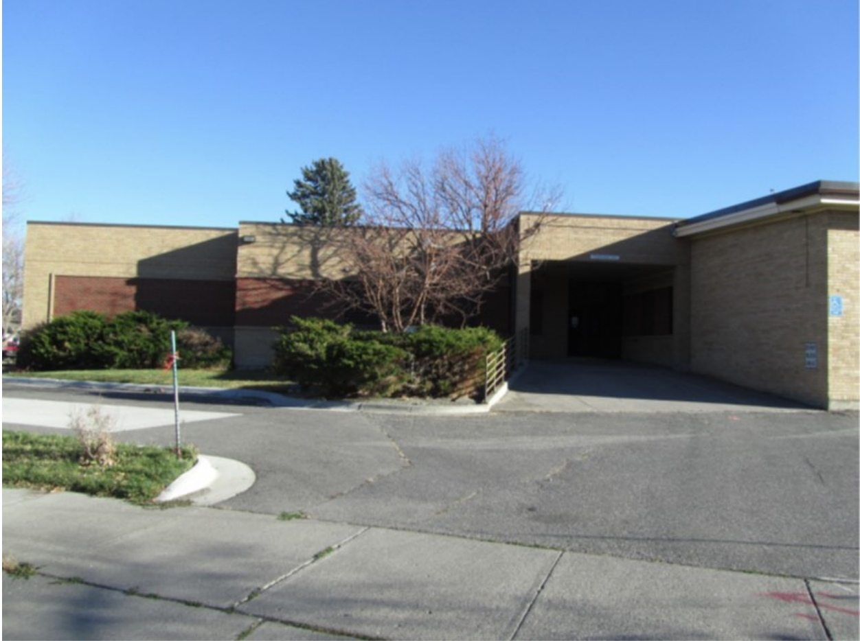
Photo 19: NW Elevation of ER Addition, Aspect: SE
