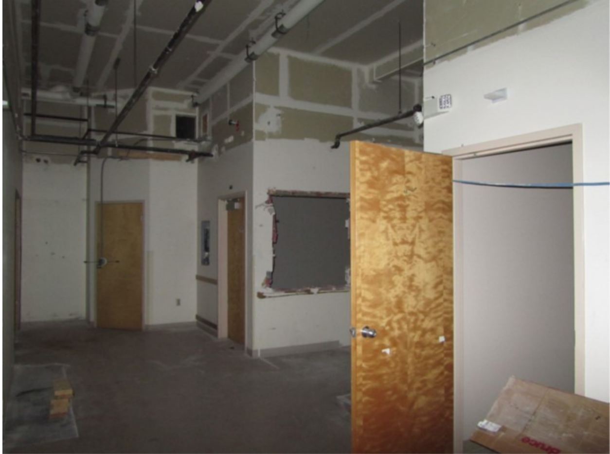
Photo 57: ER Addition, Aspect: NE
