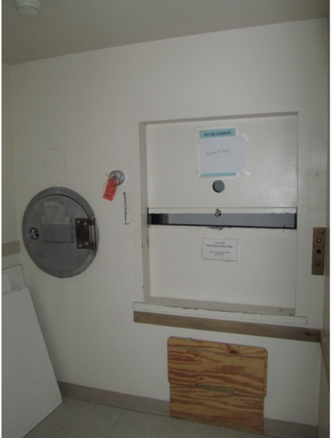
Photo 38: Primary Corridor, Hospital Core, Laundry Chute and Dumbwaiter, Aspect: NW
