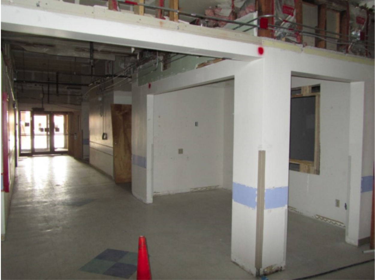
Photo 54: ER Addition Corridor with Main Entrance, Aspect: NW
