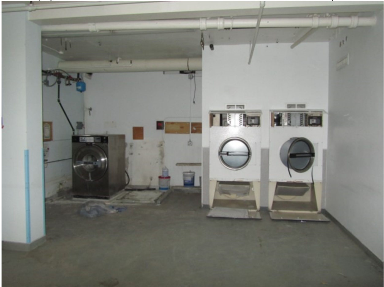
Photo 82: Basement, Primary Corridor (SW side), Laundry Room, Aspect: SW
