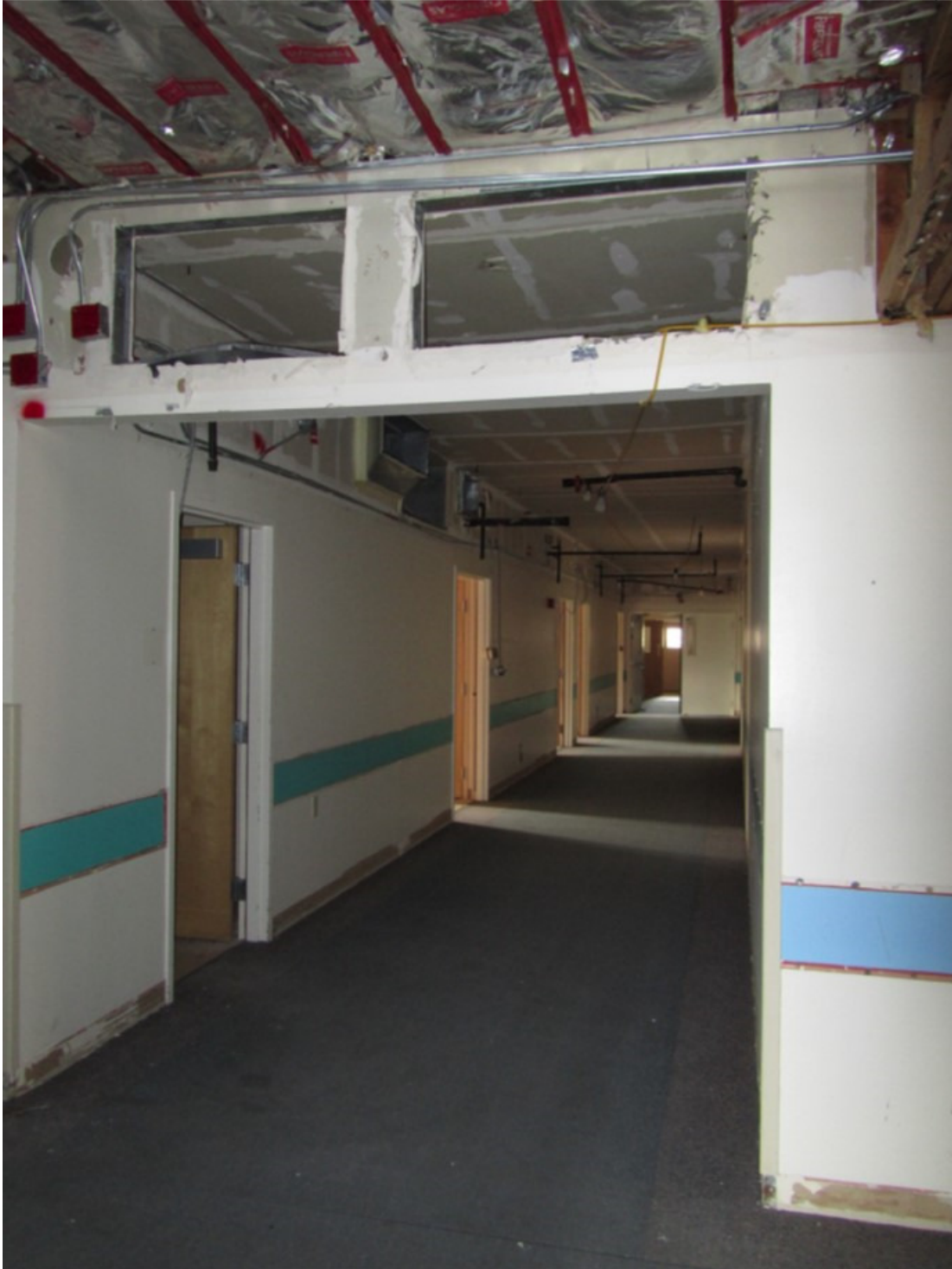
Photo 58: Rooms Addition from Nursing Corridor, Aspect: NW
