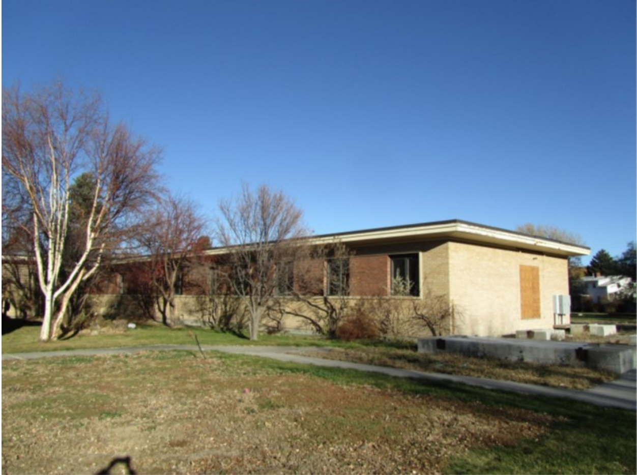
Photo 16. NW and SW Elevation of Nursing Wing, Aspect: E
