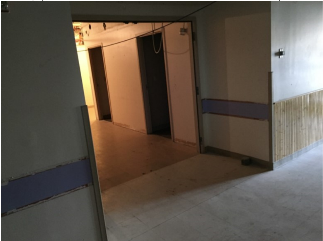
Photo 55: ER Addition Corridor, Hall to Primary Corridor, Aspect: SW
