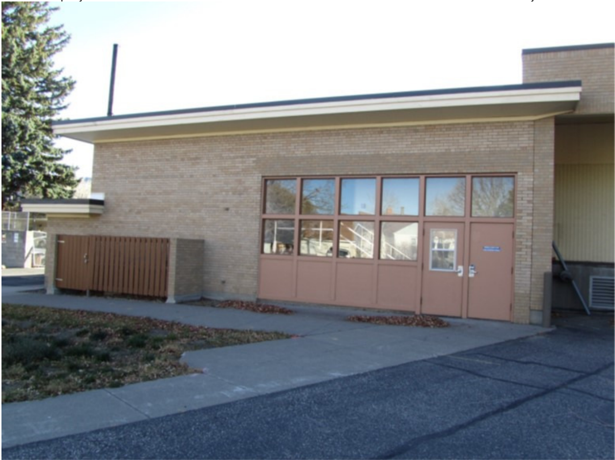
Photo 01(B). Original Main Entrance, NE Elevation of Administrative Wing, Aspect: SW
