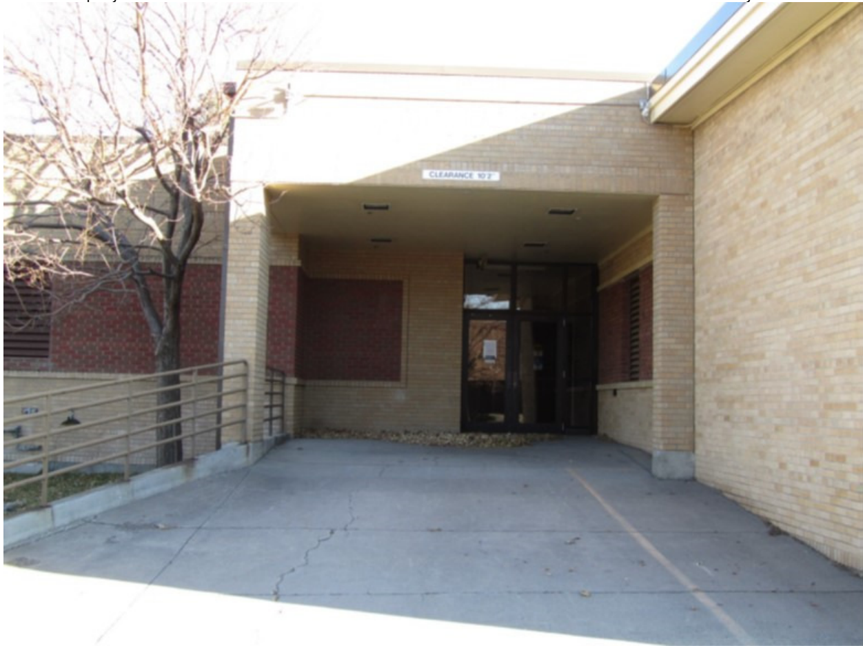
Photo 20: Main Entrance, NW Elevation of ER Addition, Aspect: SE
