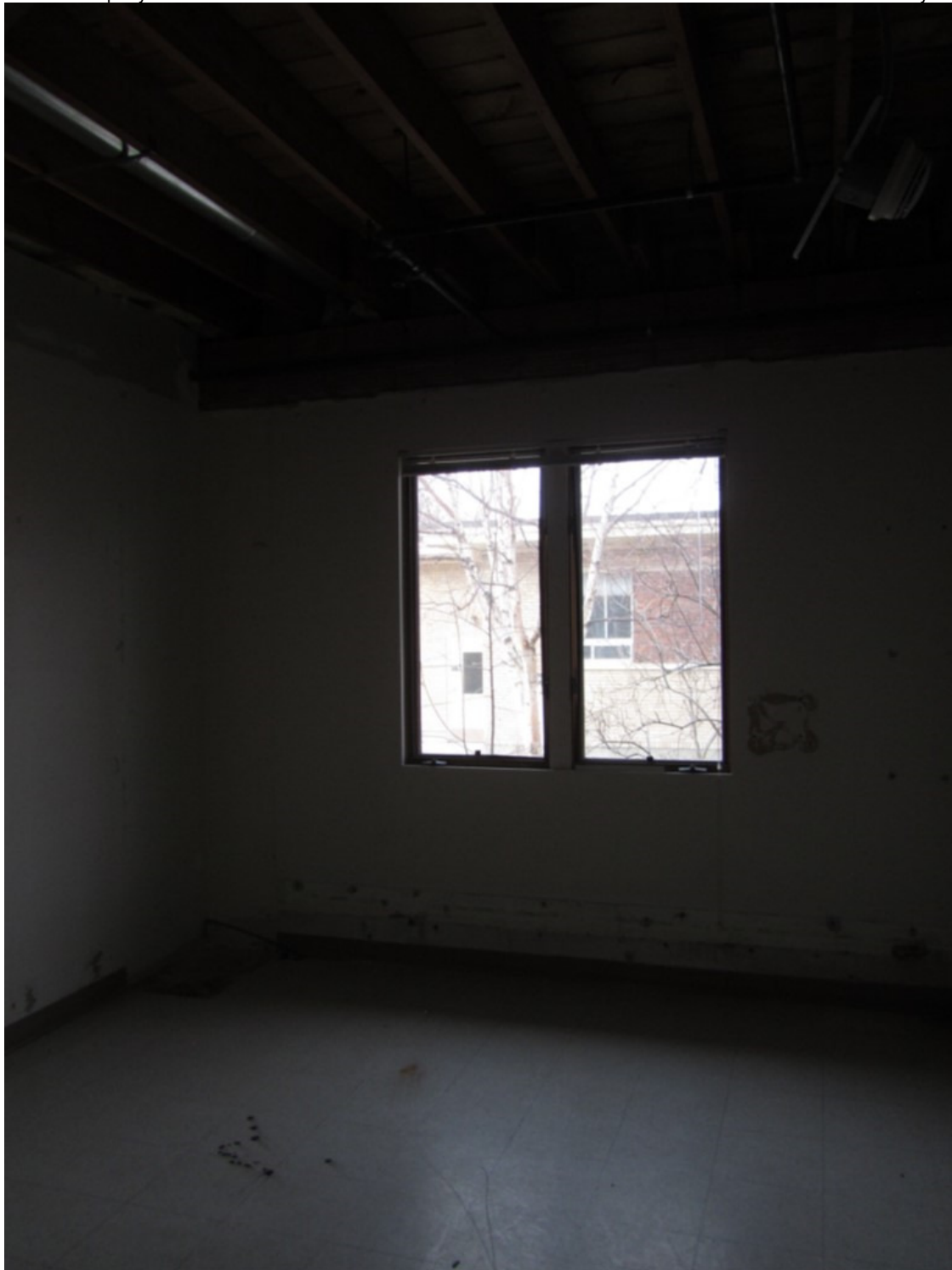
Photo 69: Nursing Corridor (SE side), Patent Room, Aspect: NW
