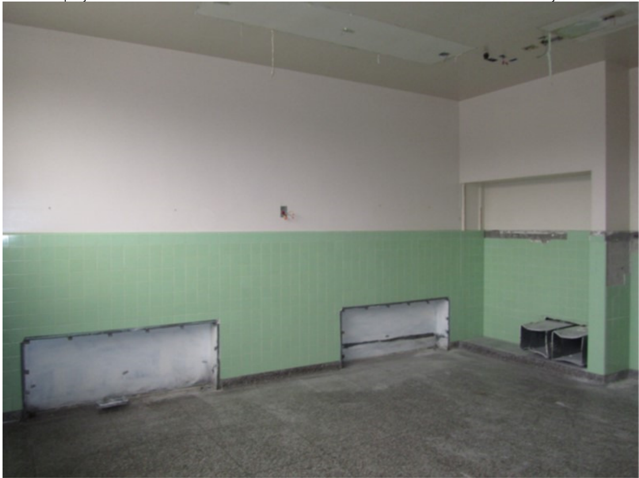
Photo 45: Primary Corridor, Surgical Wing, NE Operating Room, Aspect: E
