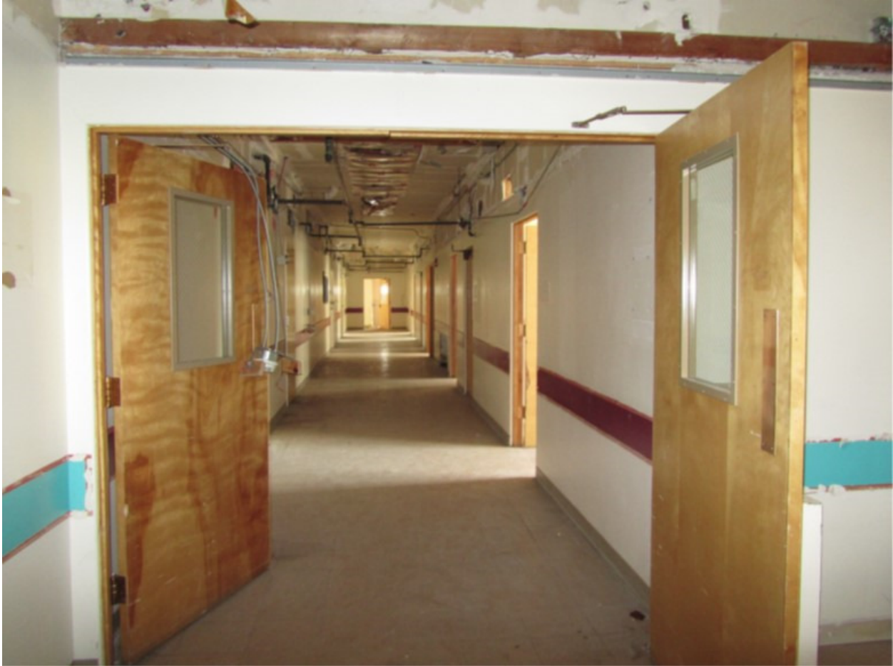
Photo 61: Maternity Corridor, Aspect: SW
