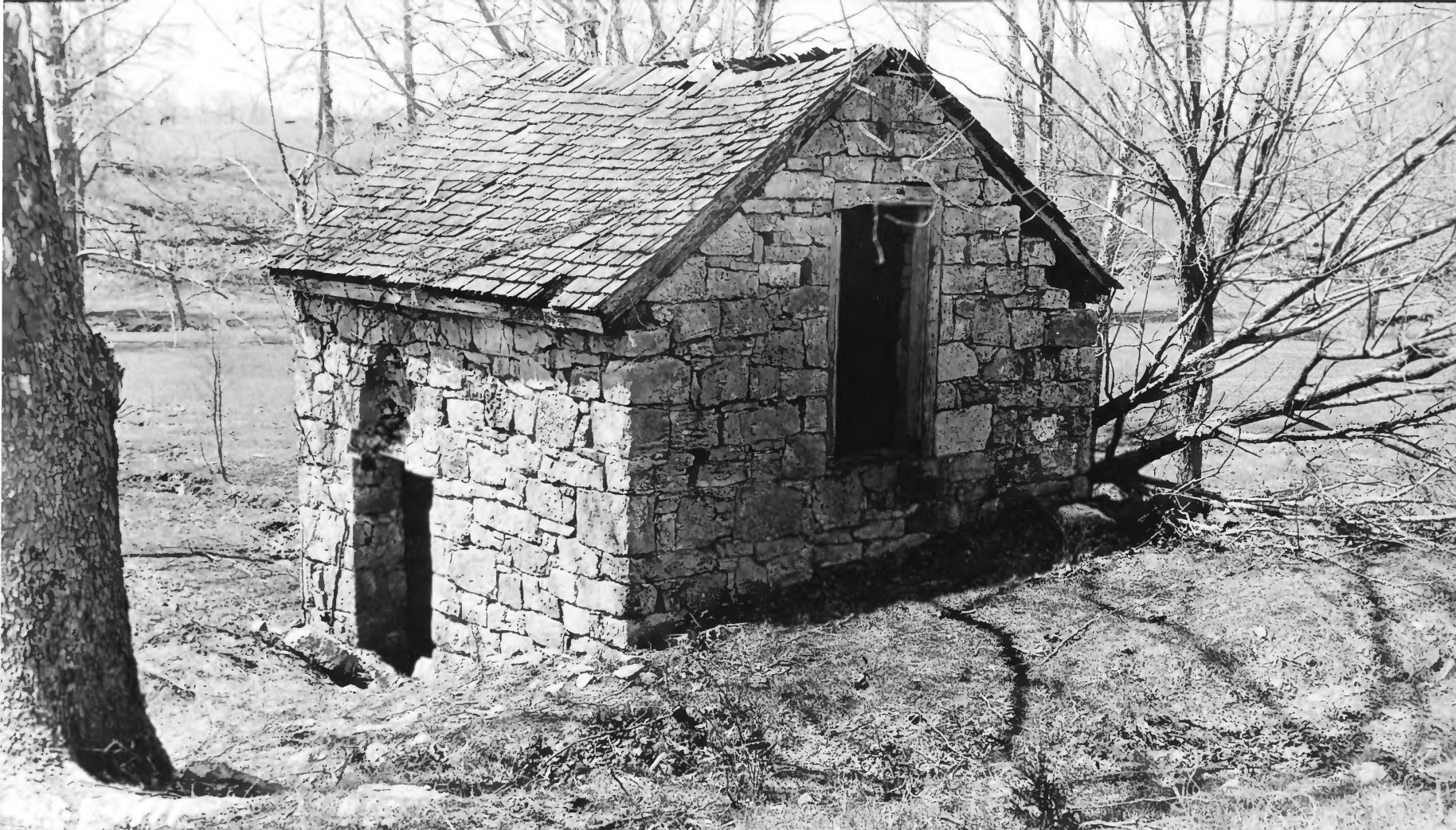
Spring Mills, where Chenoweth massacre occurred July 17, 1869
