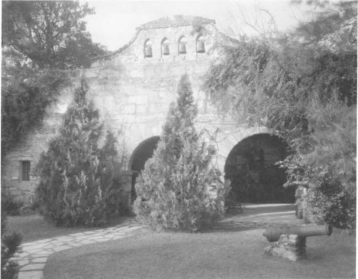
Figure 2: The photograph shows the south façade of the Spring House in the 1930s. Camera facing roughly north. (Photograph by Johnston, Frances B. 1936 or 1937. "Fountain of Youth, St. Augustine, St. Johns County, Florida." Negative, safety film, 8 x 10 in. Library of Congress: Carnegie Survey of the Architecture of the South. Accessed November 2014. http://www.loc.gov/item/csas200800426/ )
