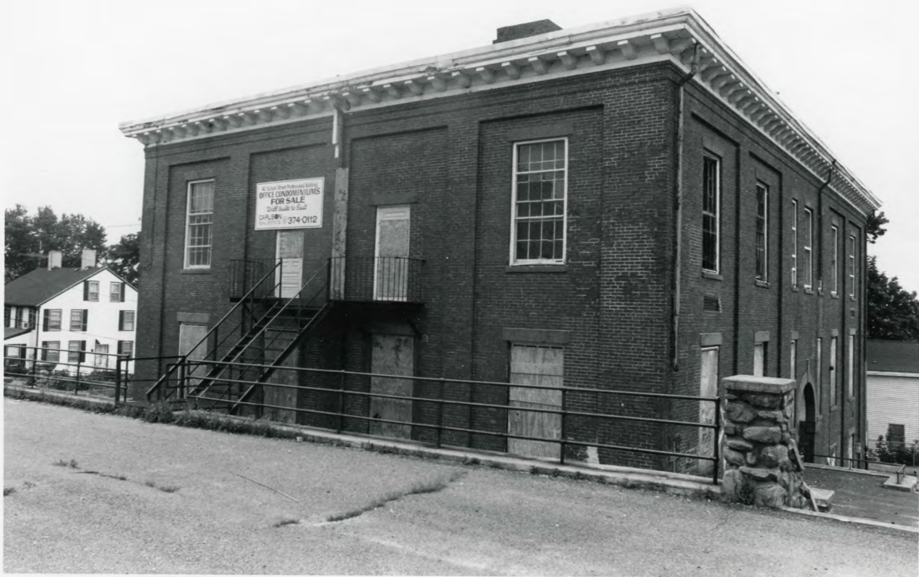
School Street School North and West Facades
