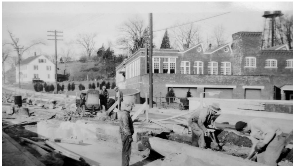
Figure 6 RI SBPR photo 108091 showing widening of Branch River Bridge No. 108 (December 1930). Former Andrews Mill office, weave shed and loading dock in background. The 2½-story residence in the rear left was a Pitts Mill worker tenement (demolished after 1949).
