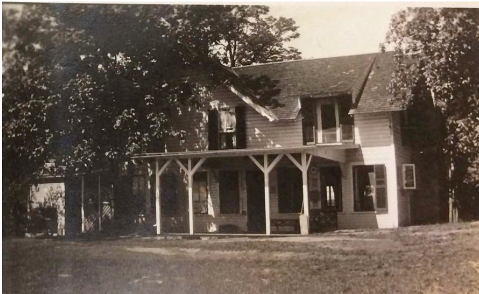
Figure 4. Main Cottage (HD #1), undated photograph Courtesy of the Vermont Historical Society.
