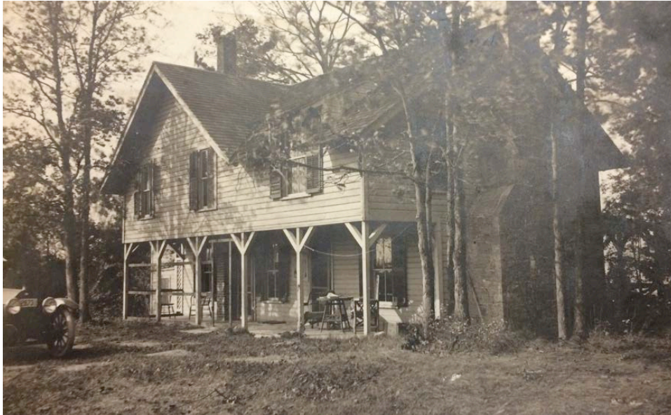
Figure 3. Main Cottage (HD #1), undated photograph Courtesy of the Vermont Historical Society.
