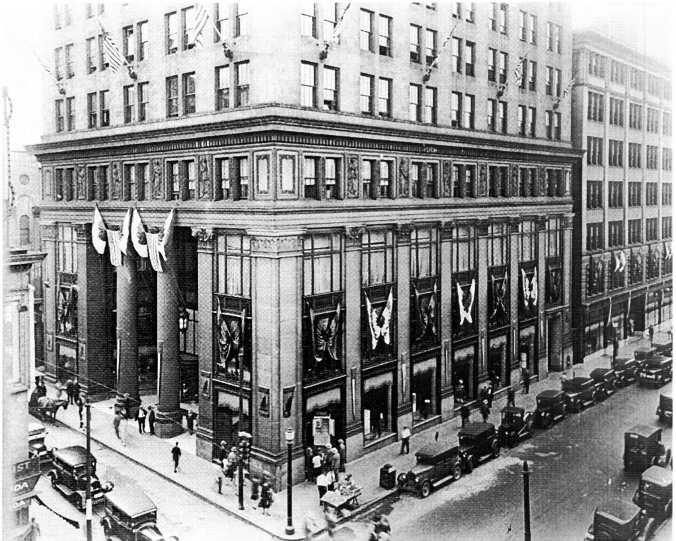
HV-6: View of street level and lower stories of the BG&E Co. Building at corner of Lexington and Liberty Streets, looking southeast, c. 1917. Courtesy of the Baltimore Gas and Electric Company Archives, Baltimore, Maryland.
