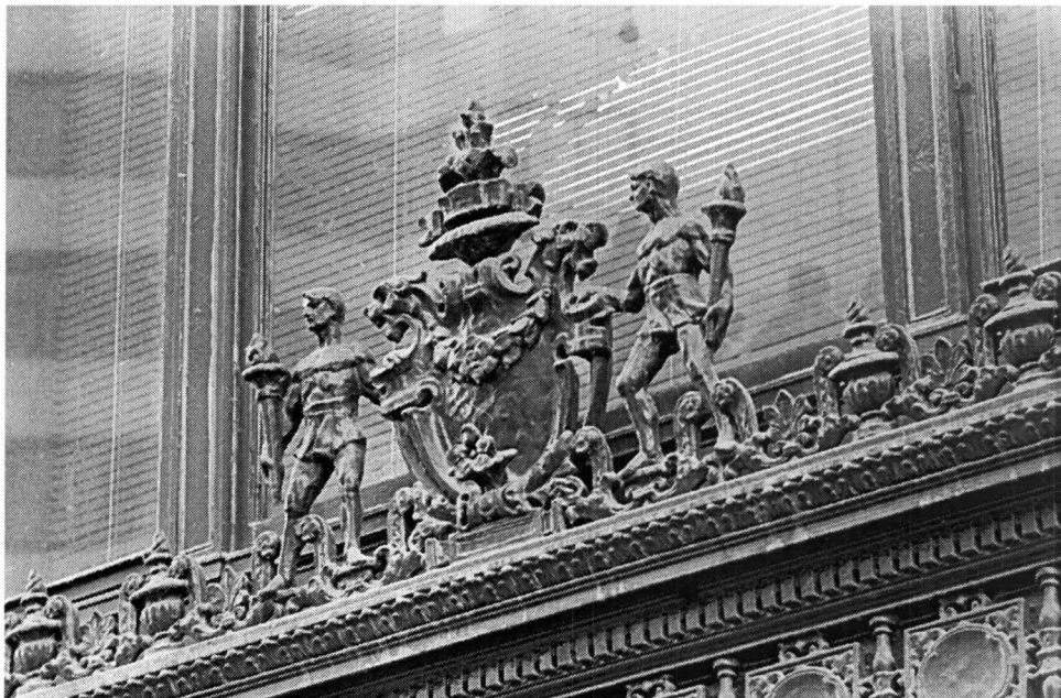
HV-12: Detail view of ironwork at window heads in exterior vestibule at Lexington Street façade, c. 1990. Courtesy of the Baltimore Gas and Electric Company Archives, Baltimore, Maryland.
