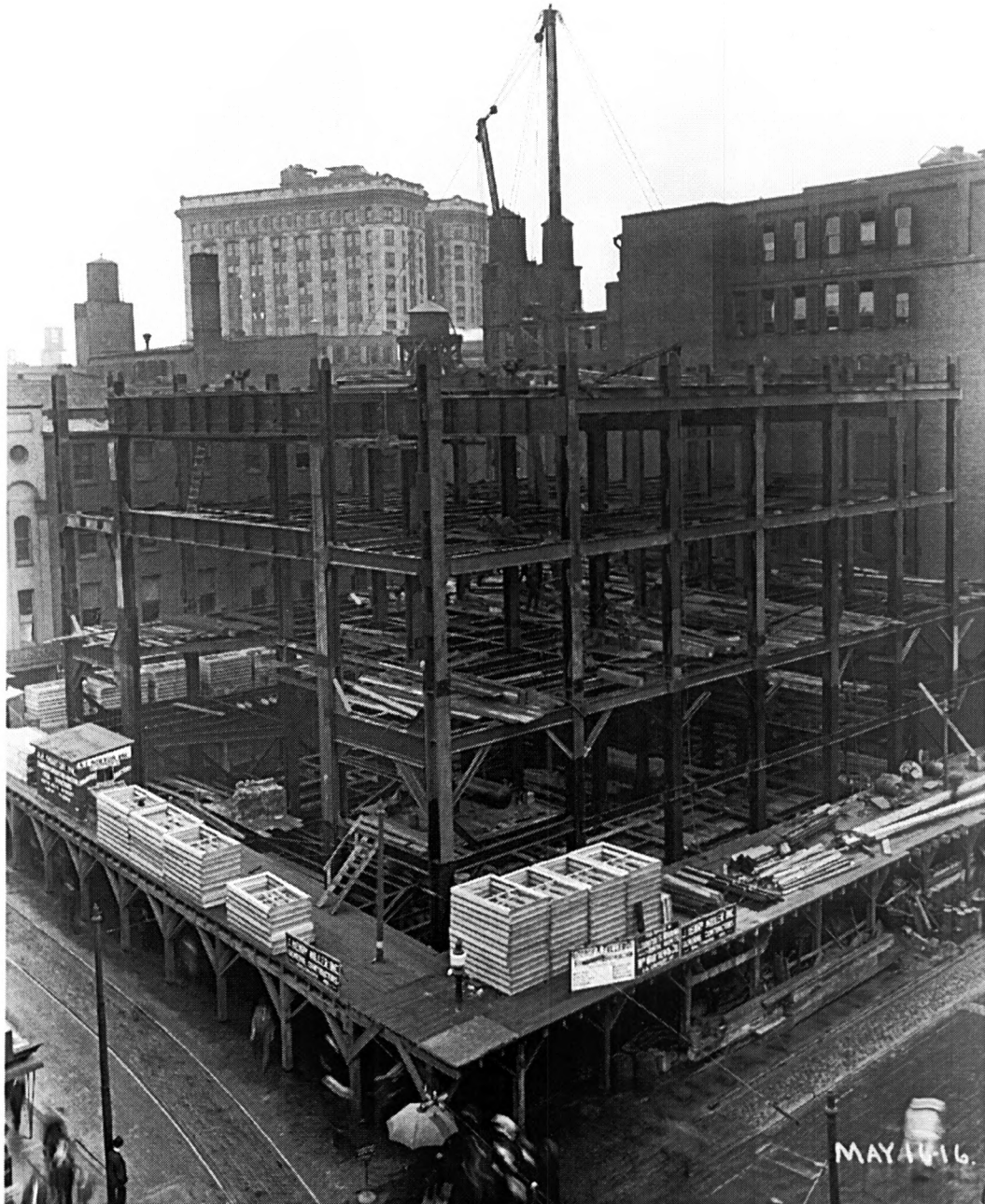
HV-2: View of BG&E Co. Building under construction, looking southeast, May 1916. Courtesy of the Baltimore Gas and Electric Company Archives, Baltimore, Maryland.
