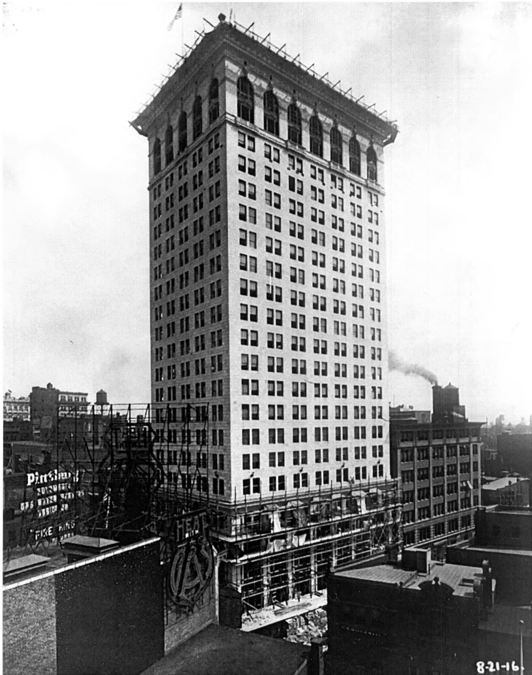
HV-5: View of BG&E Co. Building under construction, looking southeast, August 1916. Courtesy of the Baltimore Gas and Electric Company Archives, Baltimore, Maryland.
