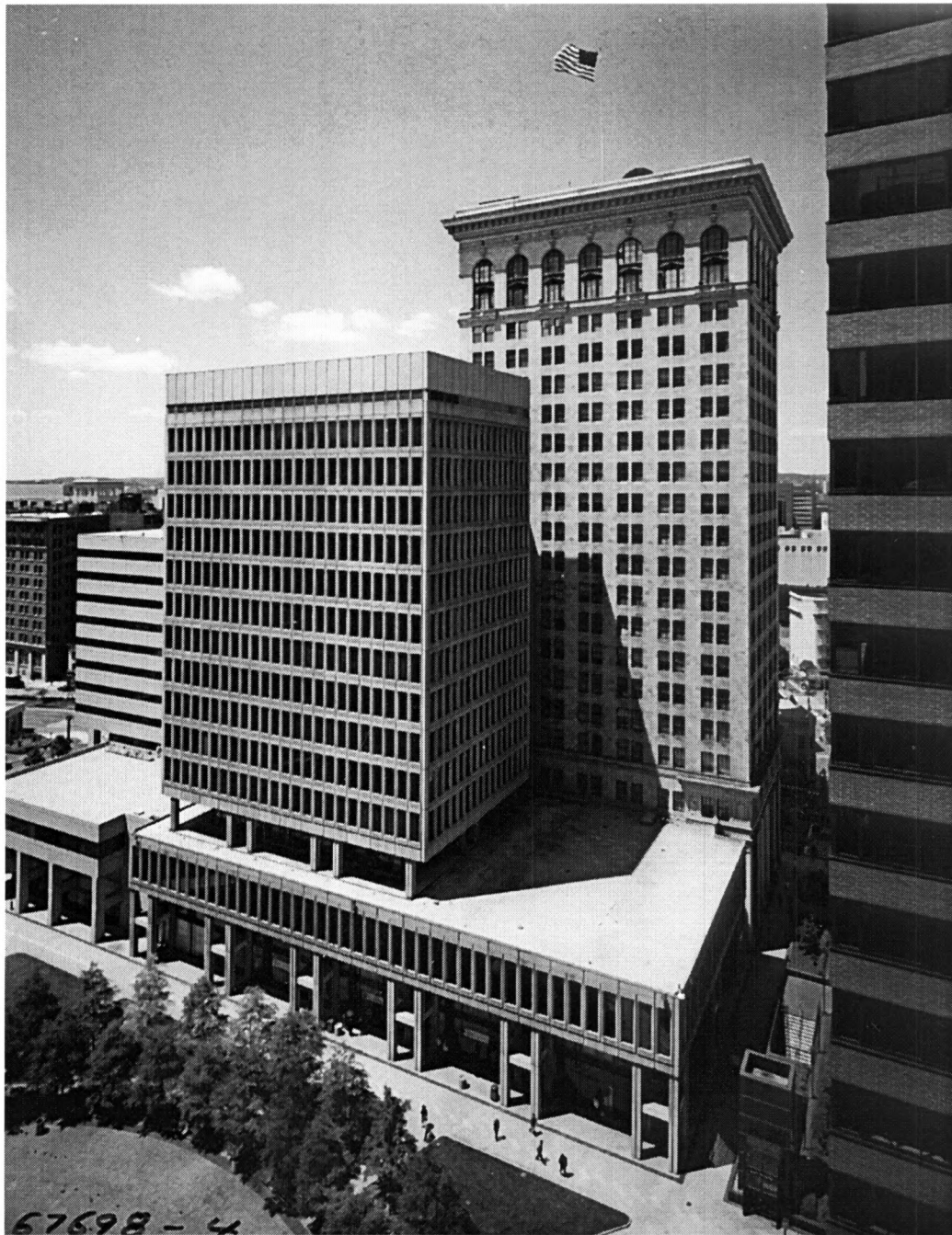
HV-22: View of south façade of BG&E Co. Building, looking north, c. 1998. The 1966 office tower addition by Fisher, Nes, Campbell and Partners in foreground. Courtesy of the Baltimore Gas and Electric Company Archives, Baltimore, Maryland.
