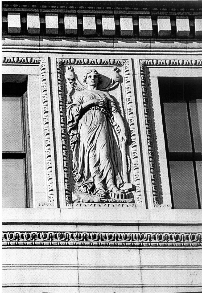
HV-9: Detail view of bas-relief marble figure at Third Floor frieze, c. 1990. It is one of four ornamental designs symbolizing Knowledge, Light, Heat and Power. The figure represented here signifies "Power." Courtesy of the Baltimore Gas and Electric Company Archives, Baltimore, Maryland.
