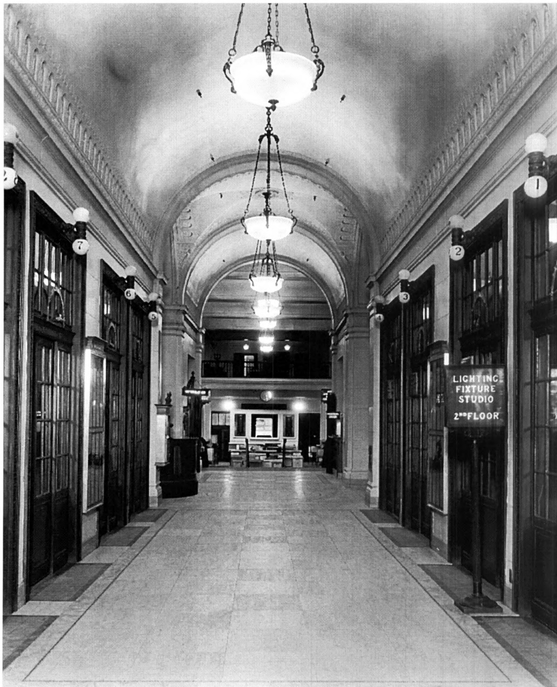
HV-18: Interior view of First Floor elevator lobby, looking south, c. 1917. The interior of the Yakel Building Annex can be seen in the background beyond the archways. Courtesy of the Baltimore Gas and Electric Company Archives, Baltimore, Maryland.
