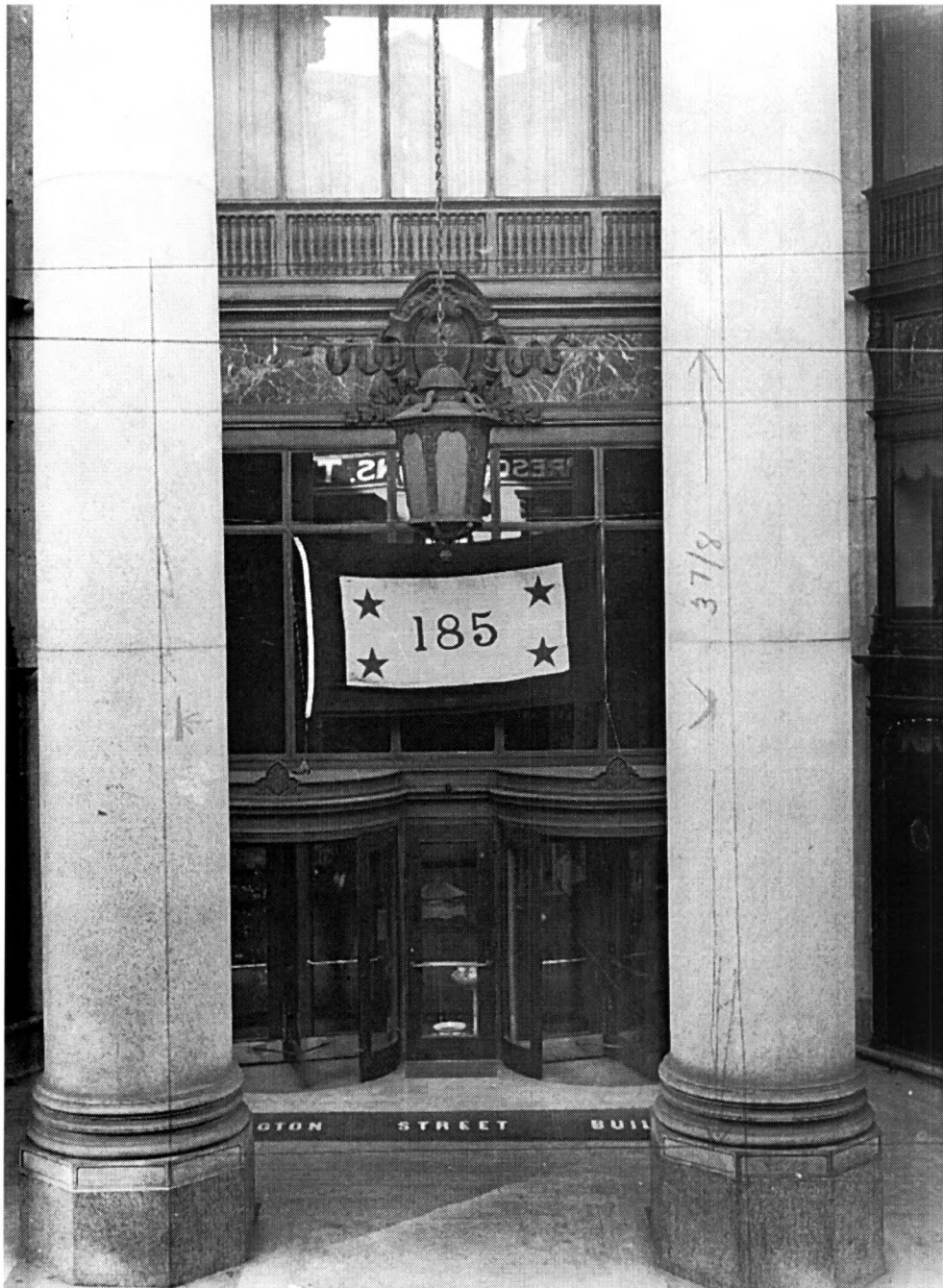
HV-10: Detail view of entrance portico and exterior vestibule at Lexington Street façade, looking south, c. 1920. Courtesy of the Baltimore Gas and Electric Company Archives, Baltimore, Maryland.
